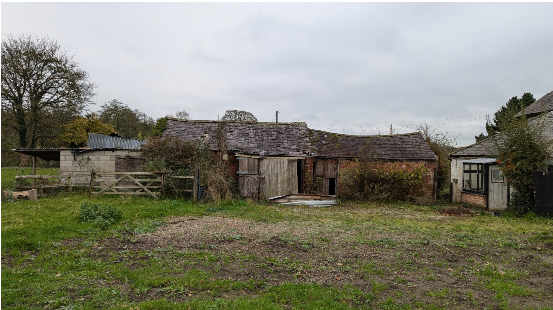
Plate 4: The west elevation showing bays C, D and E
