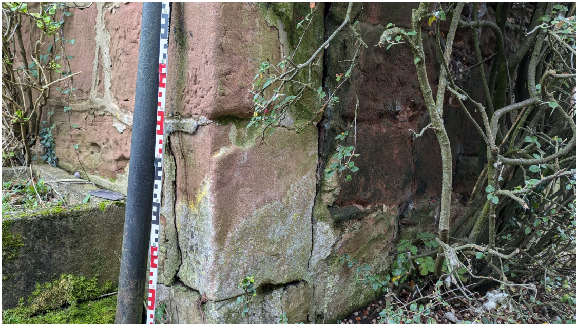
Plate 13: Southern elevation, showing junction of sandstone blockwork
