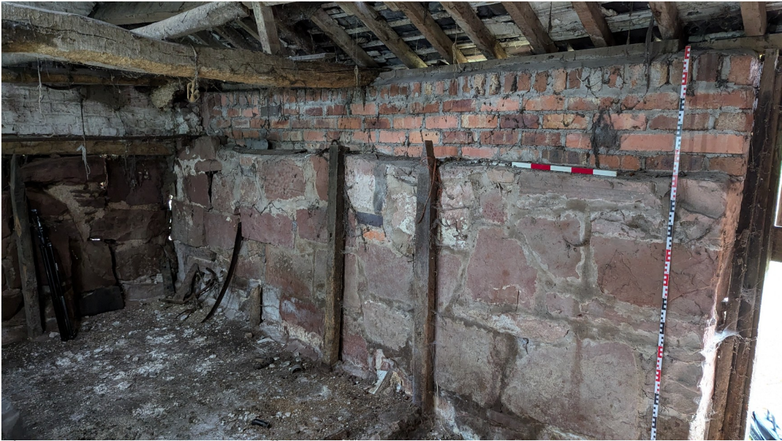
Plate 32: Room C upper western wall
