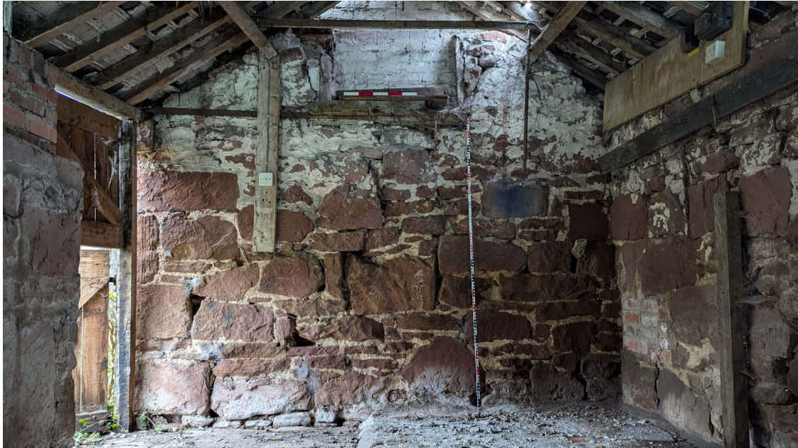
Plate 35: Room C north wall
