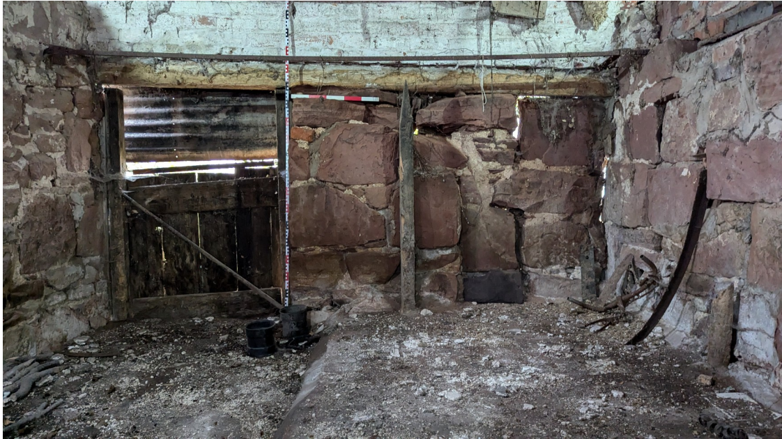
Plate 30: Room C lower section of southern wall
