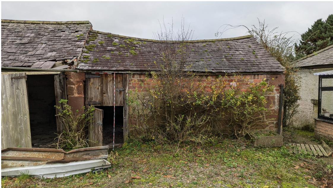
Plate 5: The west elevation of the southern bay
