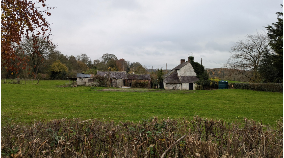
Plate 1: The setting of the structure, looking east
