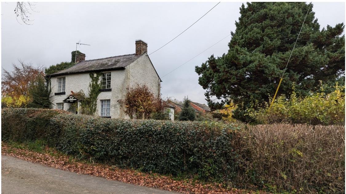
Plate 2: The setting of the structure, looking northwest
