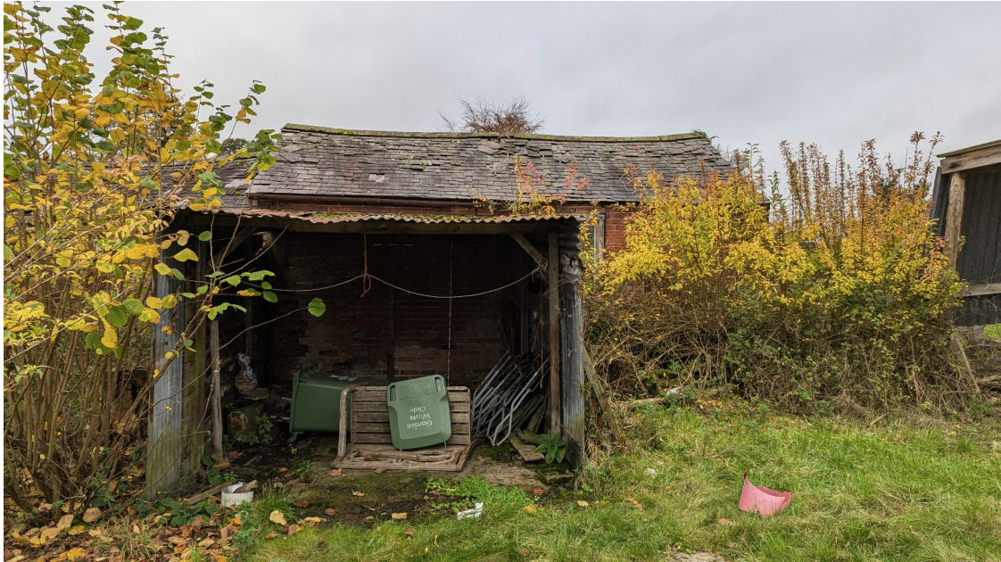
Plate 26: Room B looking west
