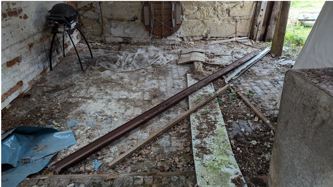
Plate 47: Room D floor looking south
