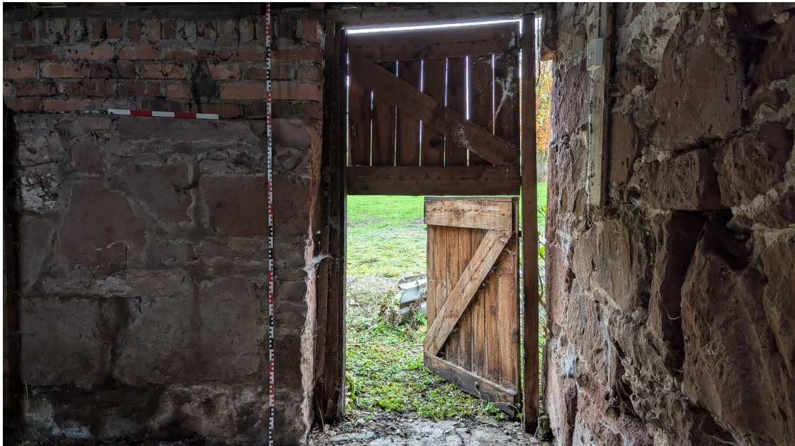
Plate 34: Room C access
