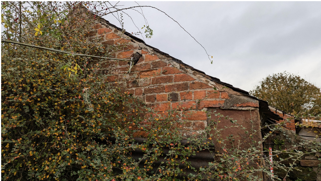
Plate 12: Southern elevation, showing brick gable, sandstone edge and corrugated metal shuttering
