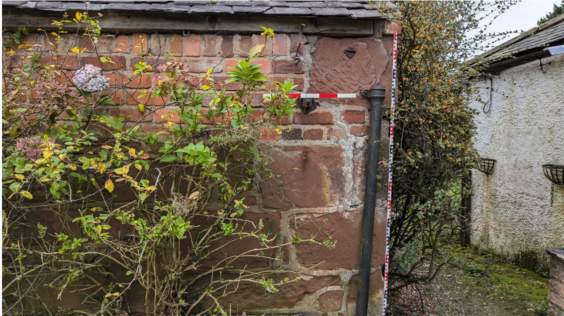
Plate 6: The southwest corner of the structure
