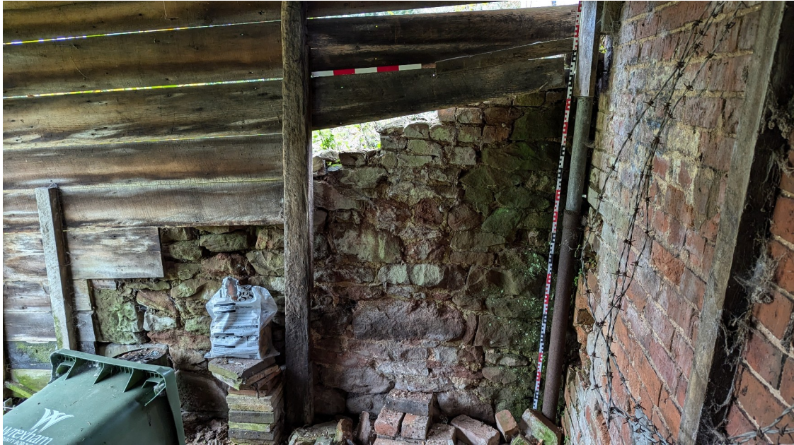
Plate 28: South wall of Room B
