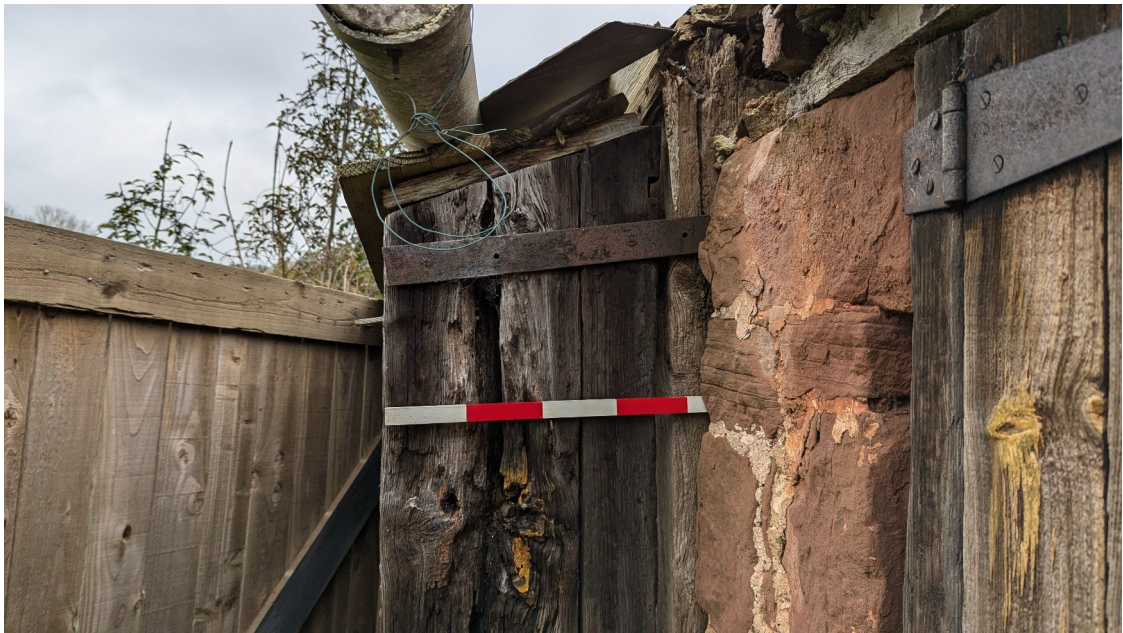
Plate 8: Timber framework for 20 th century door to Room D
