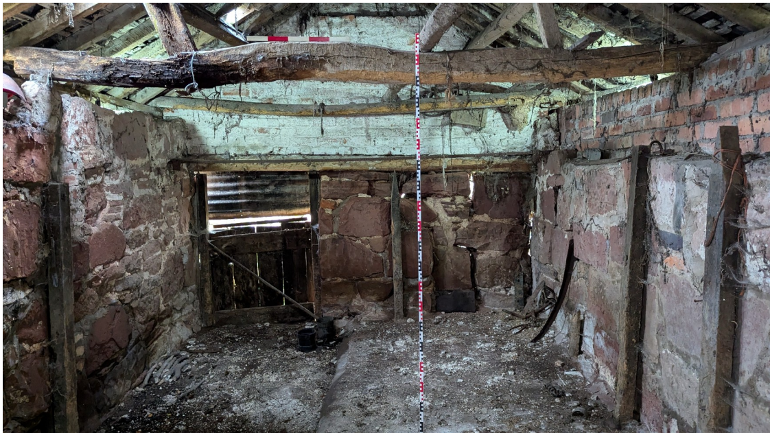
Plate 29: Room C looking south
