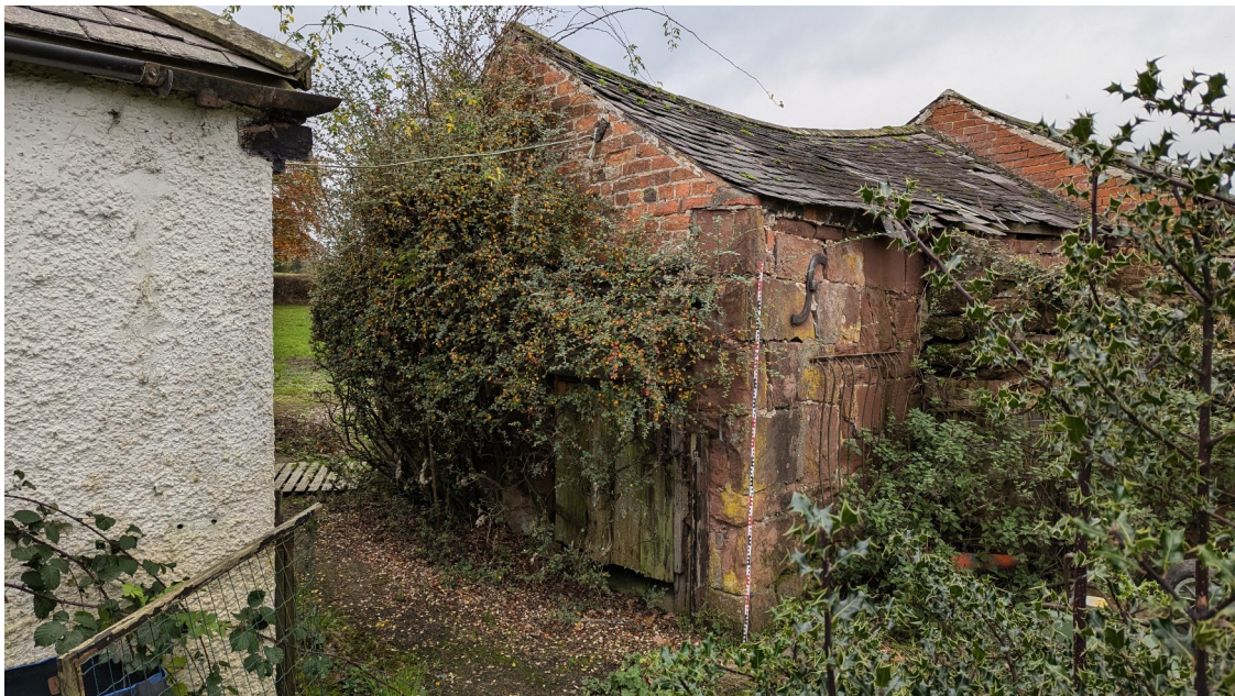
Plate 11: Southern elevation, looking west
