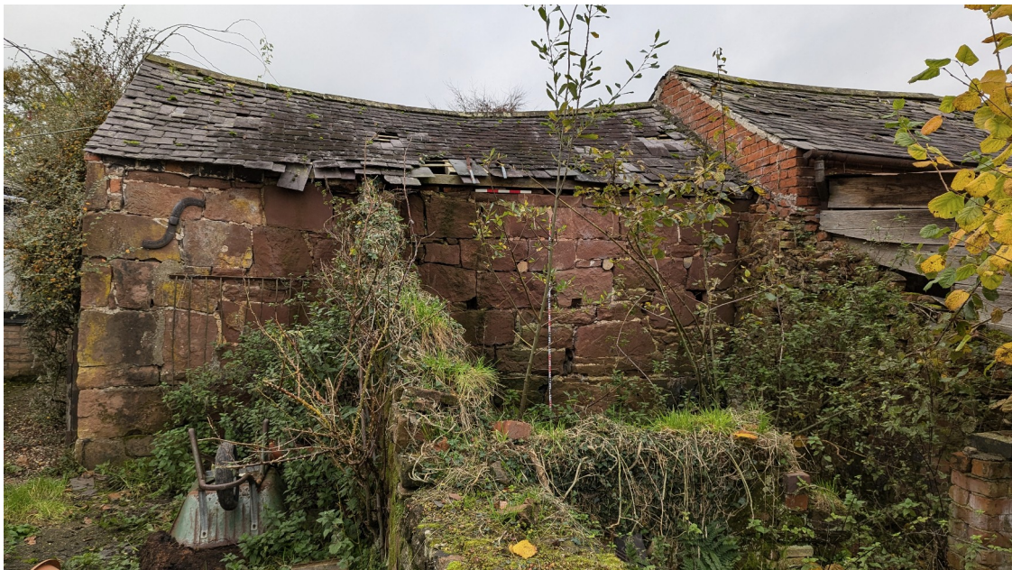
Plate 18: Eastern elevation, southern bay
