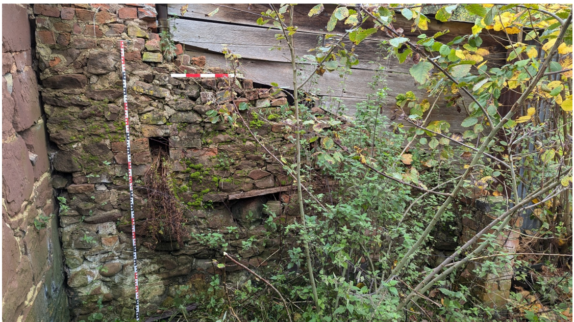
Plate 20: Wall between Rooms A and B
