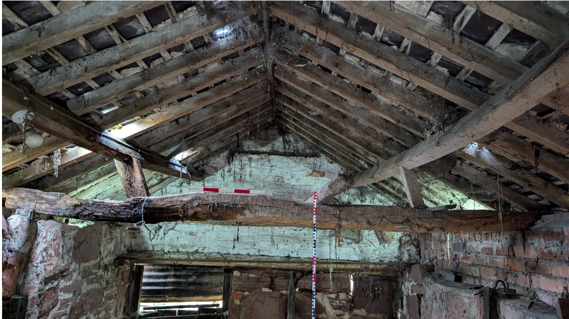
Plate 33: Room C roof structure
