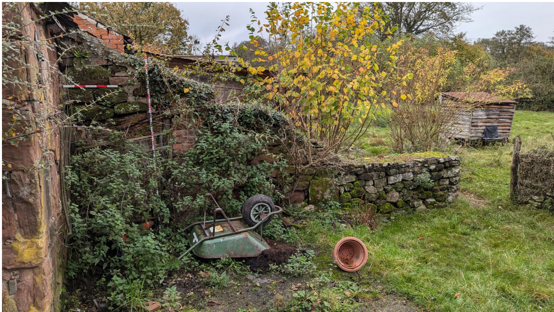
Plate 14: Southern elevation, showing Room A and garden wall
