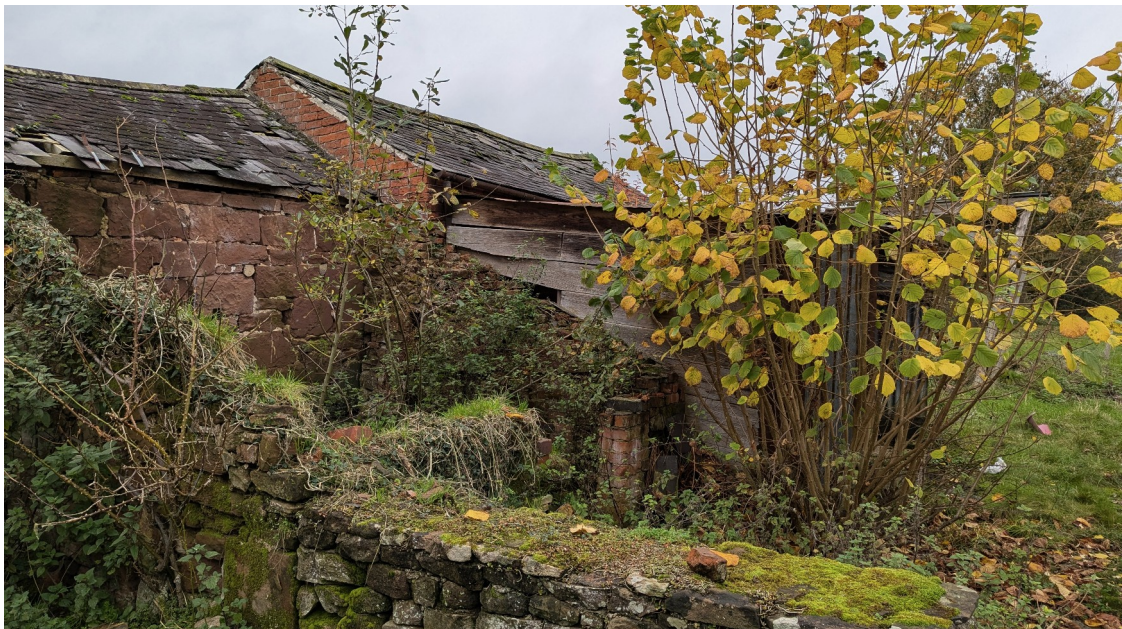
Plate 24: Room A looking northwest
