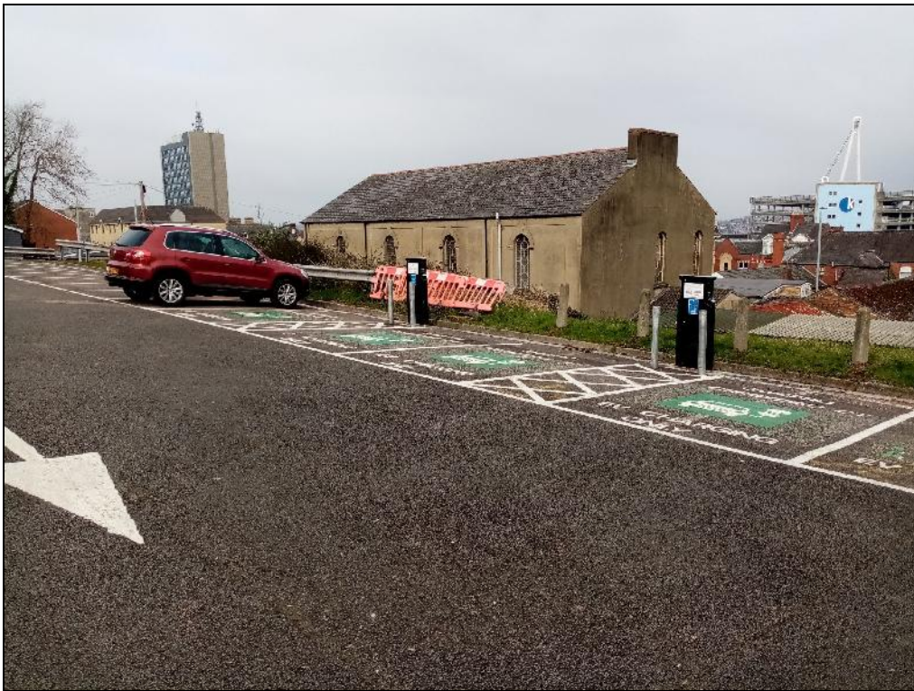
Plate 18: A view of Mount Zion chapel from within Hill Street Car Park. Note the high-rise modern buildings now dominating the skyline beyond. Looking northeast.
