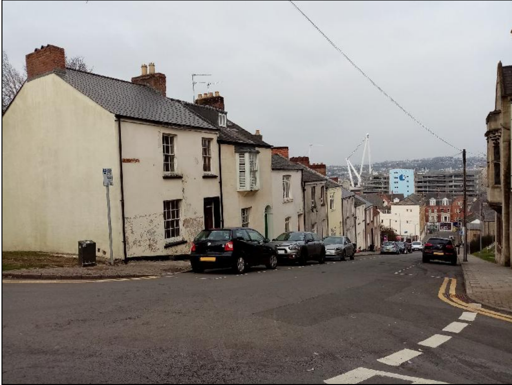
Plate 41: A view down Hill Street towards Commercial Street. This is a key view of the listed terraces houses of No.13 and No.14 Hill Street, at the top of the row to the left. The proposed development would not affect this view. Note the modern structures dominating the long view beyond Commercial Street. Looking northeast.
