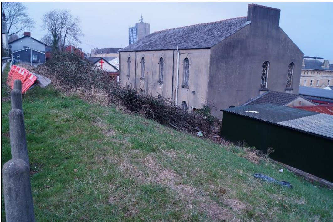
Plate 28: A view of the space between the Hill Street Car Park and Mount Zion chapel showing the fall in ground level between the two sites. Looking north.
