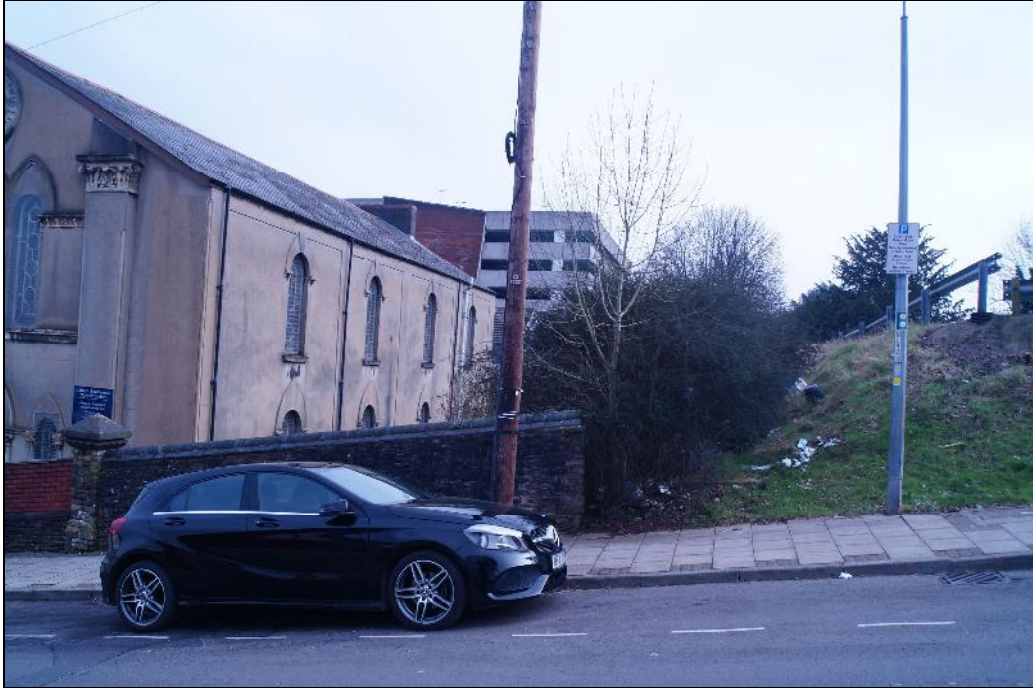
Plate 13: A view of the gap between Mount Zion chapel to the left and the bottom of Hill Street Car Park to the right. This shows the considerable depth of material added to level up the Hill Street Car Park on the steeply sloping ground which formerly existed here. Looking south-southeast.
