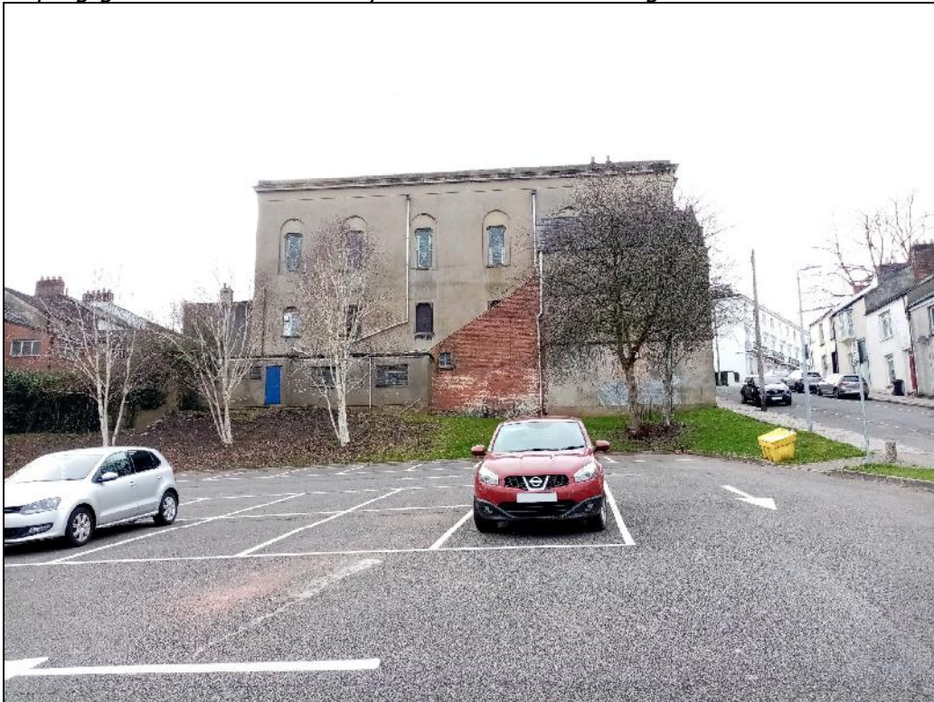
Plate 14: A view within Hill Street Car Park looking towards Victoria Road Chapel. The south terrace of Victoria Place (Listed Building 3045) is seen to the right and the listed No.13 and No.14 (Listed Buildings 23150 and 23151) at the end of Hill Street. Looking west-southwest.
