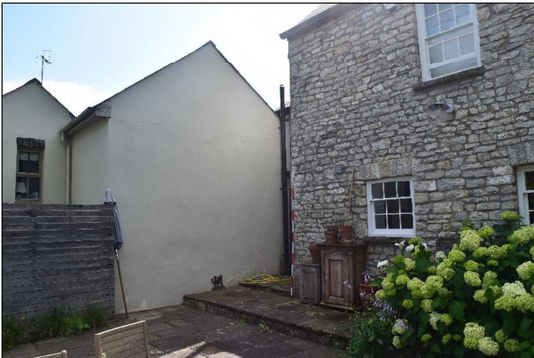
Plate 3: KCM2021_003 A view looking southeast towards where the "boot room" is to be in a location that on the 1877, 1899, 1919 and 1971 1:2500 Ordnance Survey maps was occupied by a porch or conservatory which wrapped around the end of the house. The window centre right was formerly a doorway and has been blocked in.
