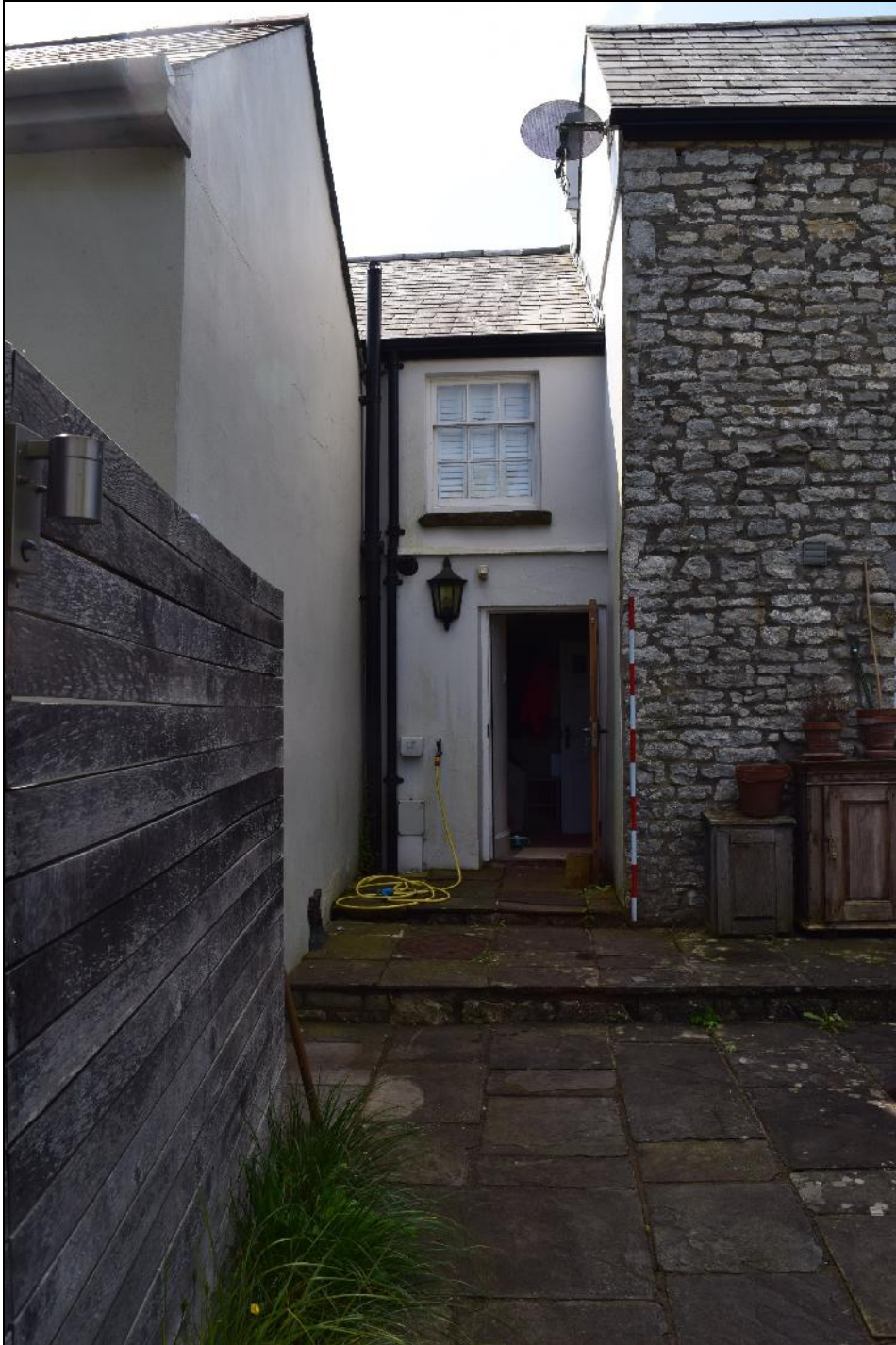
Plate 1: KCM2021_001 The rear of the property looking south-southeast where the "boot room" would be located. The corner of the main building is bare stone with no obvious quoin stones apart from towards the top of the wall where a repair has been made. The infilling structure is the modern two storey extension, although the lower wall is older and part of the range of domestic and farm buildings attached to the house. The gable of a former outbuilding is seen to the left, which has been heightened in modern times but which was originally connected to the house by a porch or conservatory which stood in the area shown here.
