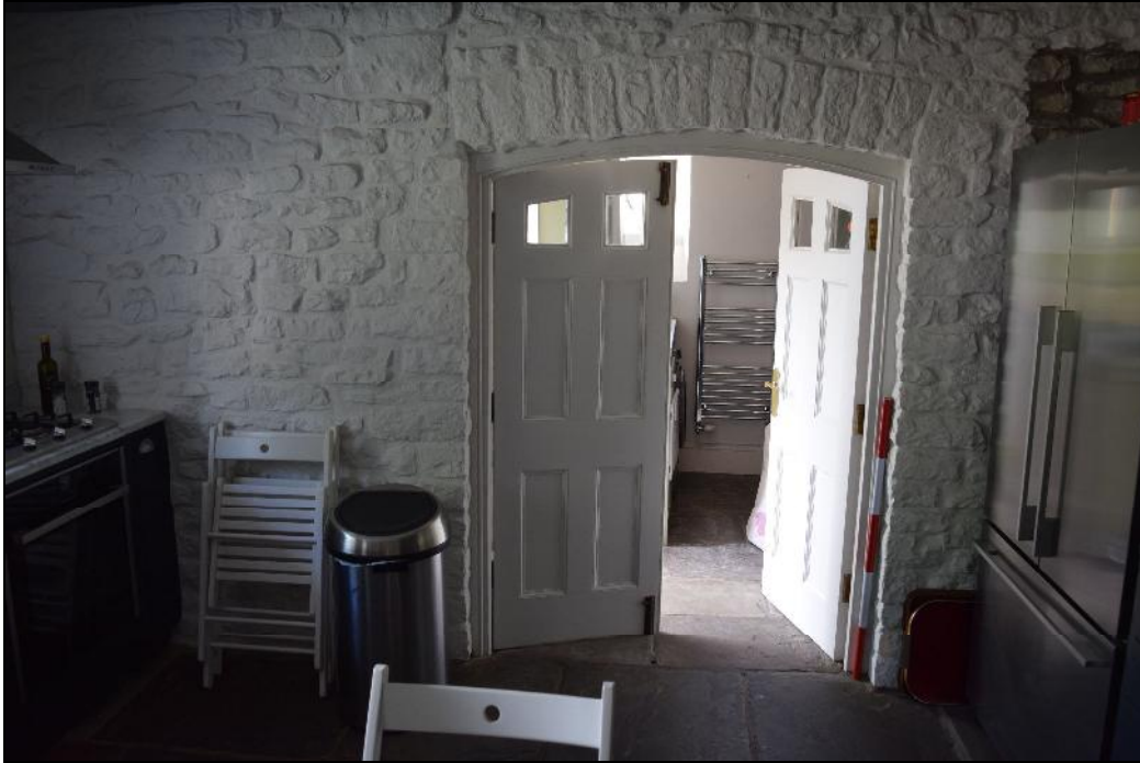
Plate 12: KCM2021_012 A view east-northeast from the kitchen towards the current double doors into the utility room. The stonework around the door suggests some alteration has happened here in the past, whether the insertion of a new door, or alteration to an existing door.
