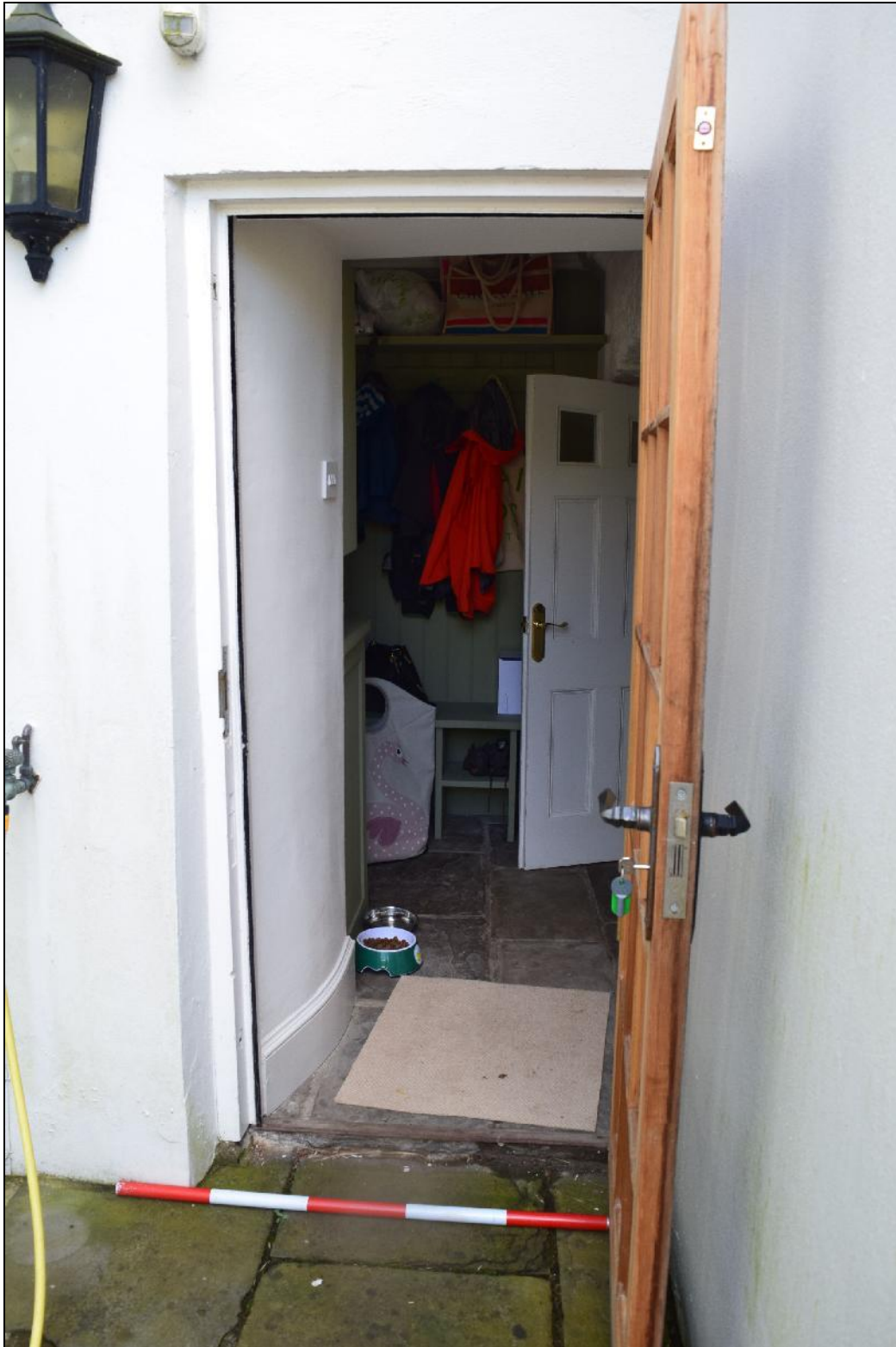
Plate 8: KCM2021_008 A view looking south-southeast through the external door into the utility room. The thickness of the wall here suggests that this was an earlier wall and not built during the modern two storey extension. The doorway is thought to be modern, as the original entrance to the kitchen has been partly blocked up and turned into a window.
