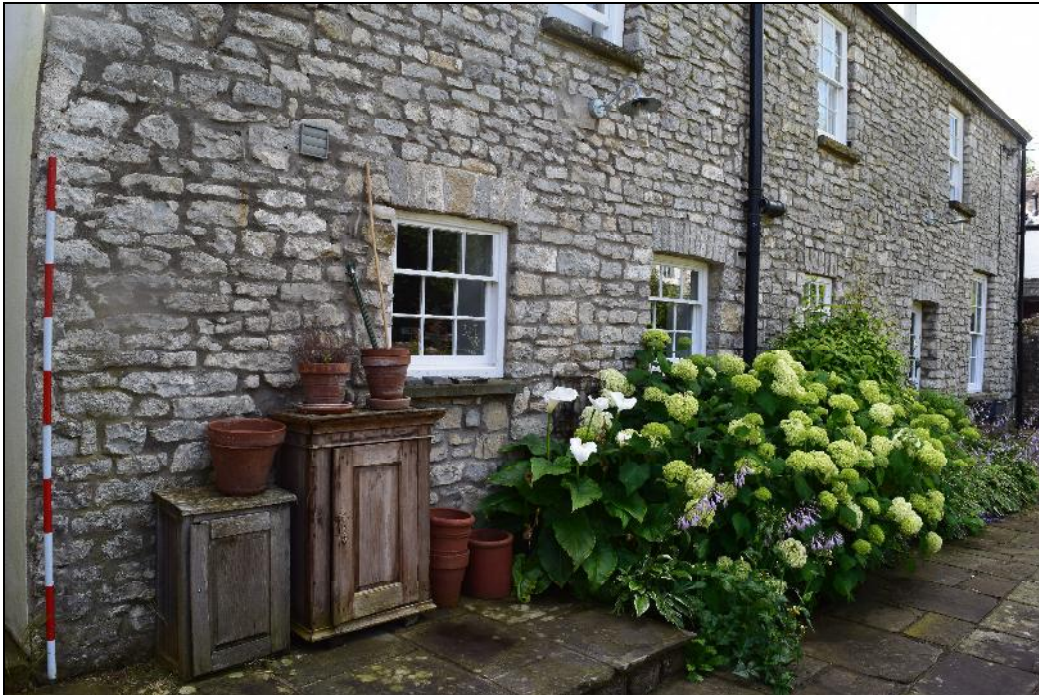
Plate 5: KCM2021_005 The rear of the house looking south-southwest. A straight joint below the window to the left of centre is evidence of its earlier use as a doorway. The 19 th century porch or conservatory may have extended beyond this doorway which would have given access from the kitchen into the lost porch.
