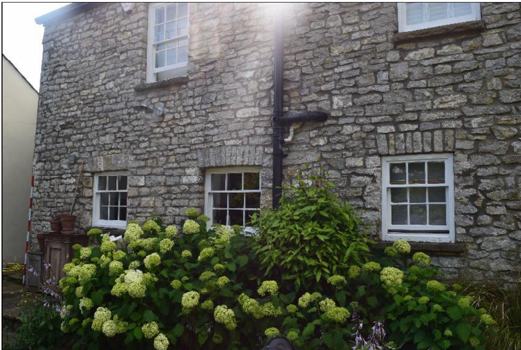
Plate 4: KCM2021_004 The rear of the house looking south-southeast the window centre right appears to have been added or altered as can be seen by the stone work and pointing around it. The window farthest to the left is the former blocked-in door.
