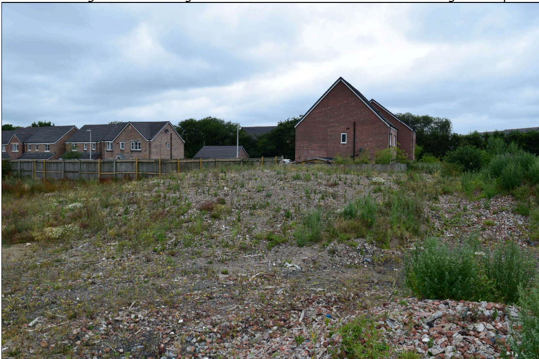
Plate 2: MYT2022_002 A view across the development site taken from the top of a mound of rubble, looking northeast towards the existing development on Maes Pedr. The Carmarthen Cattle Breeding Centre buildings have been demolished and the remains ground up.
