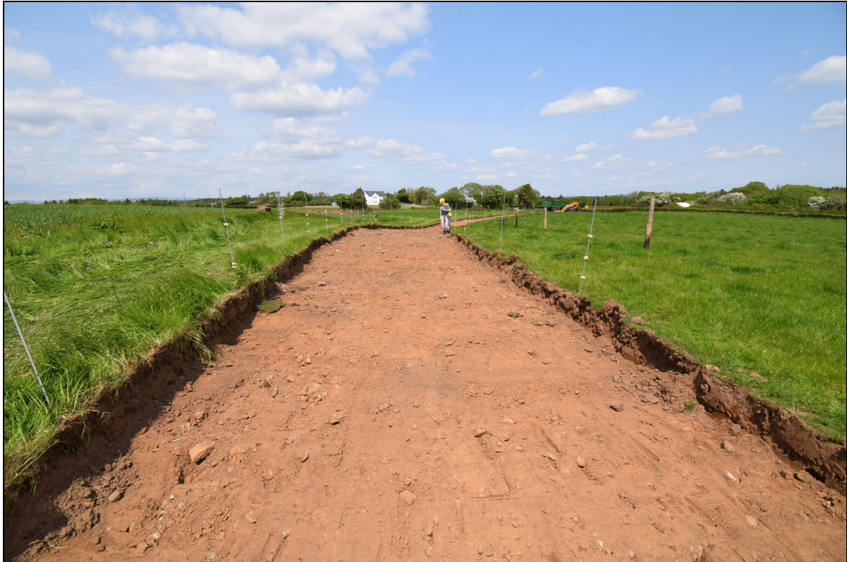
Plate 7: MYW2023_107: View after (001) and (002) removed taken from ST0372775435, looking north.
