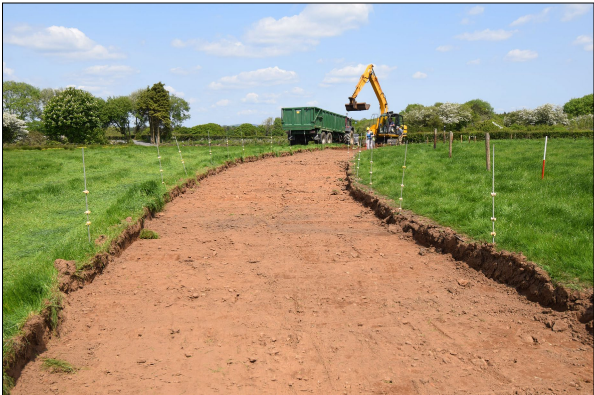
Plate 10: MYW2023_110: View after (001) and (002) removed taken from ST0375075500, looking east-northeast.
