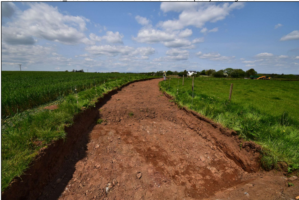
Plate 6: MYW2023_106: View after (001) and (002) removed taken from ST0373575416, looking north-northwest
