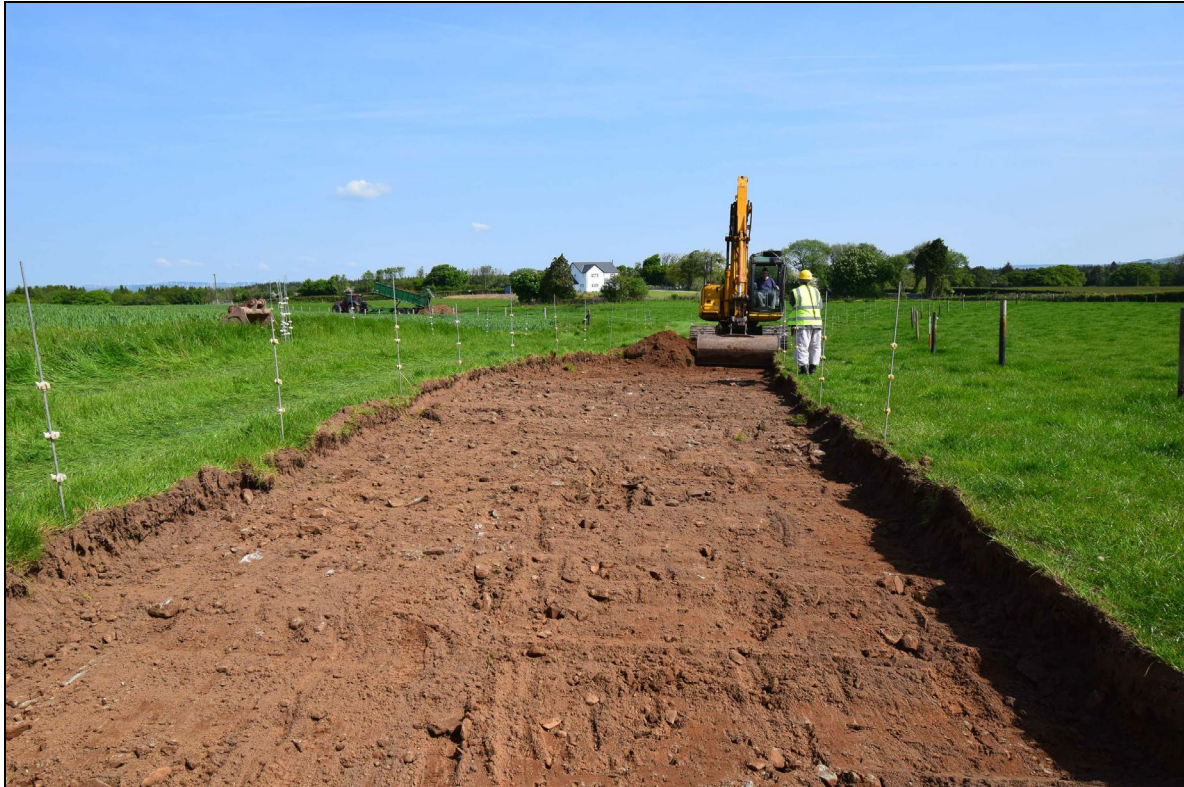
Plate 5: MYW2023_105: General view of the removal of (001) looking north.
