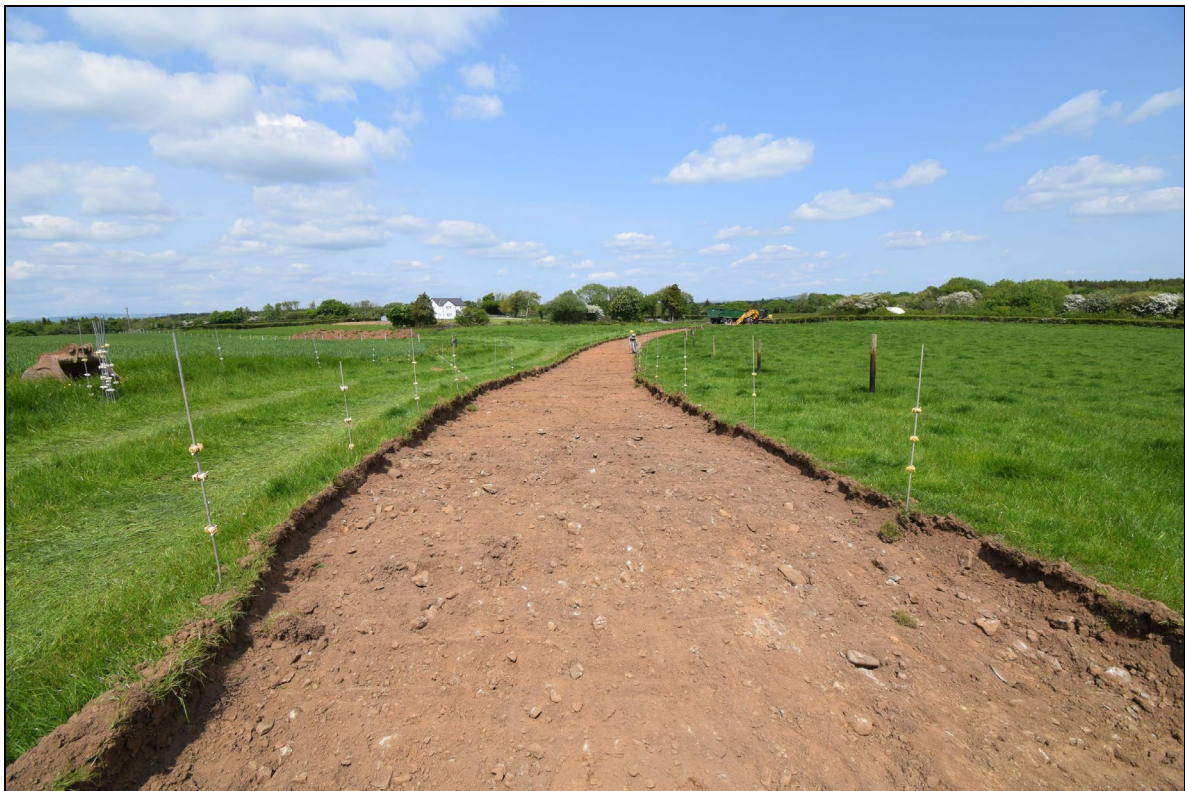
Plate 8: MYW2023_108: View after (001) and (002) removed taken from ST0373875480, looking north.
