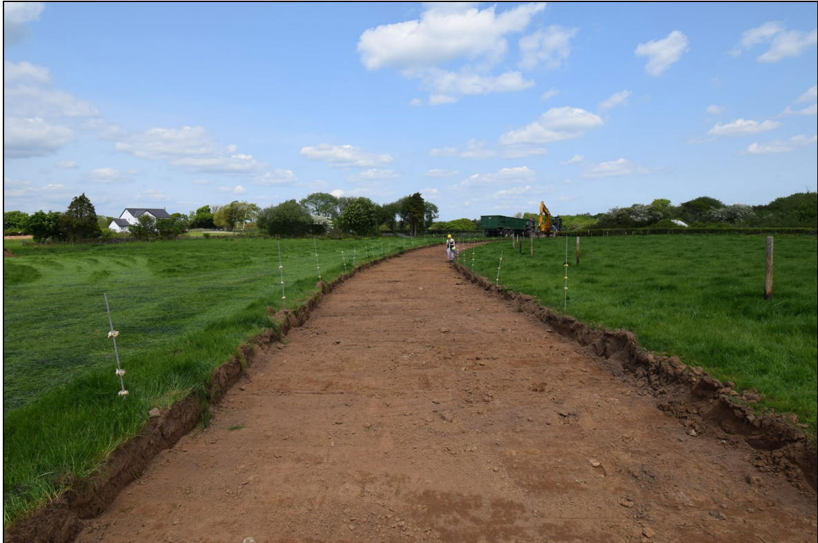
Plate 9: MYW2023_109: View after (001) and (002) removed taken from ST0373875480, looking northeast.
