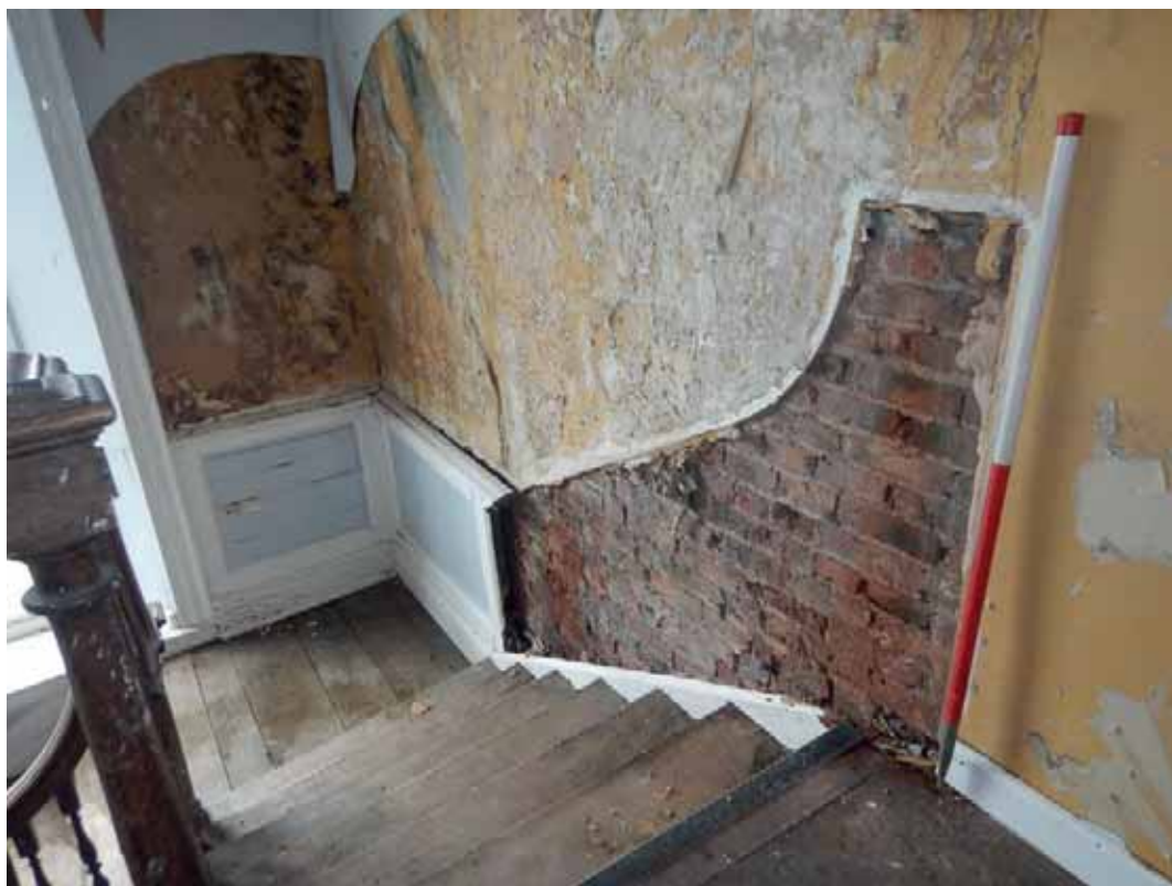
Plate 21. Exposed brick under damaged panelling to the top flight of the main staircase, looking south-east. 1m scale.
