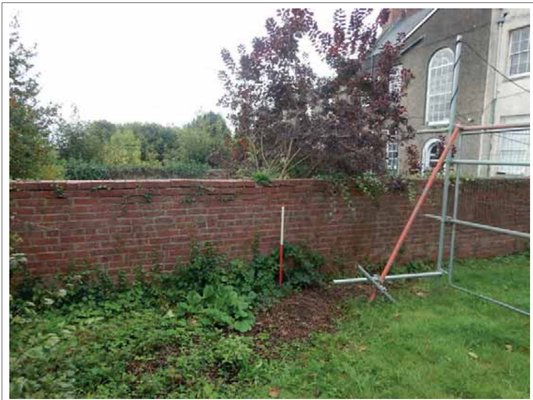
Plate 235. 20th century replacement of a central section of the walled garden. 1m scale.
