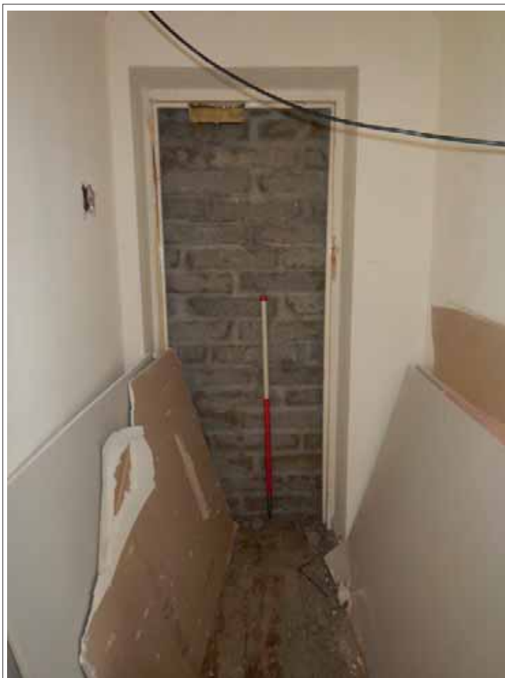
Plate 48. Room 1.3, looking north, showing blocked doorway through to north annex. 1m scale.
