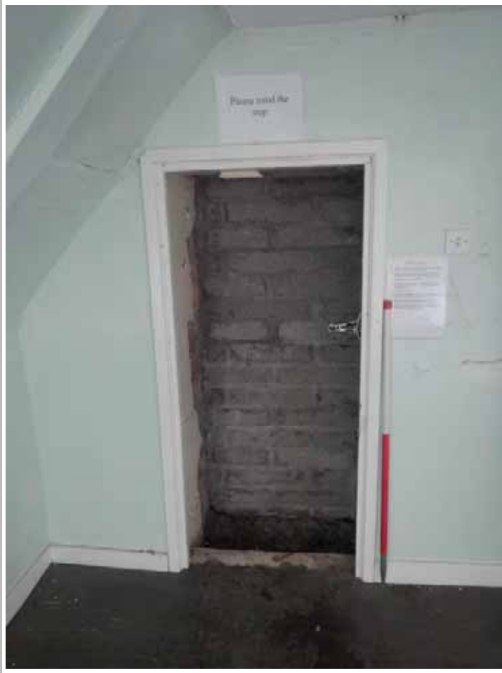
Plate 87. Blocked up doorway to north annex in Room 2.8, looking north. 1m scale.
