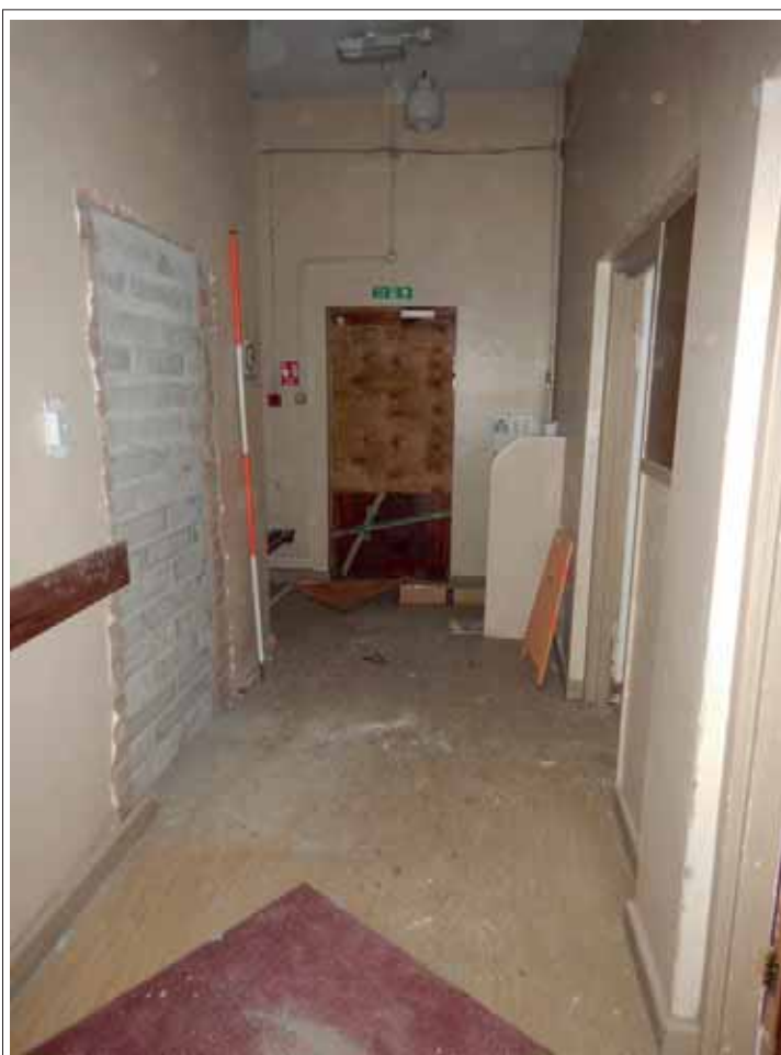
Plate 188. South hallway, looking west, showing blocked up doorway to the original house to the left. 2m scale.
