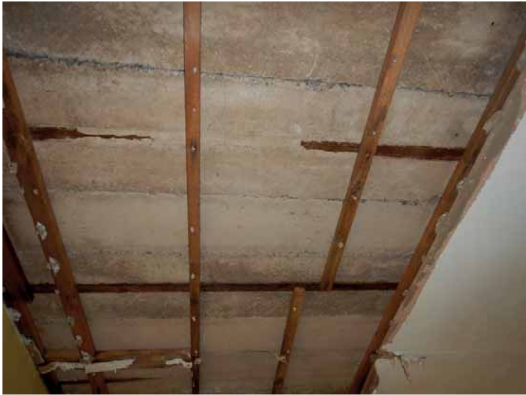
Plate 173. Detail of damaged ceiling in ground floor washroom revealing concrete beam construction.
