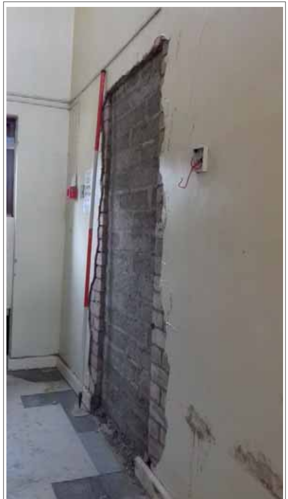
Plate 210. Blocked doorway through to original house, looking south-east. 2m scale.
