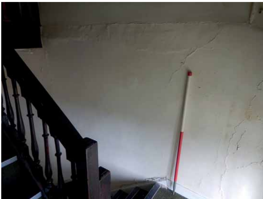
Plate 61. North wall of Room 1.13, showing scar of removed first floor ceiling to the top of the image. 1m scale.
