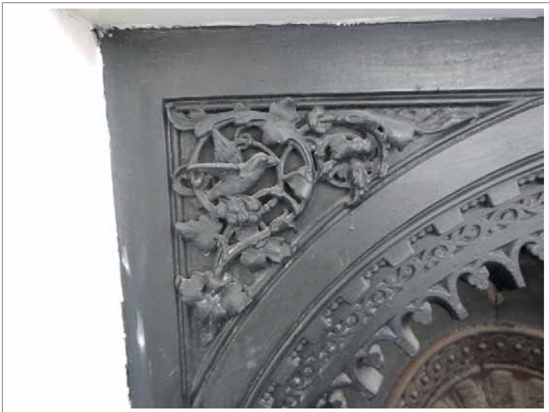
Plate 36. Detail of cast iron fireplace in Room 0.3.
