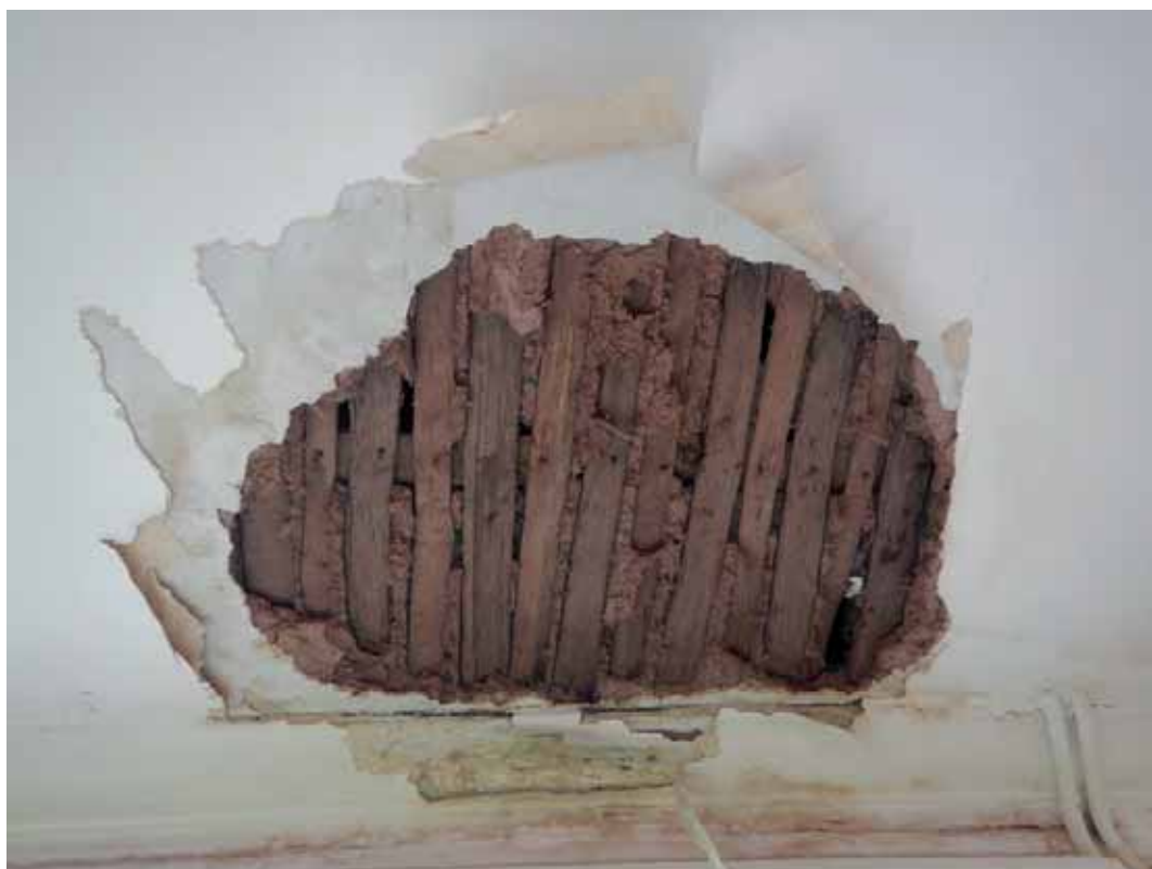
Plate 50. Damaged ceiling in Room 1.2, showing original ceiling construction.
