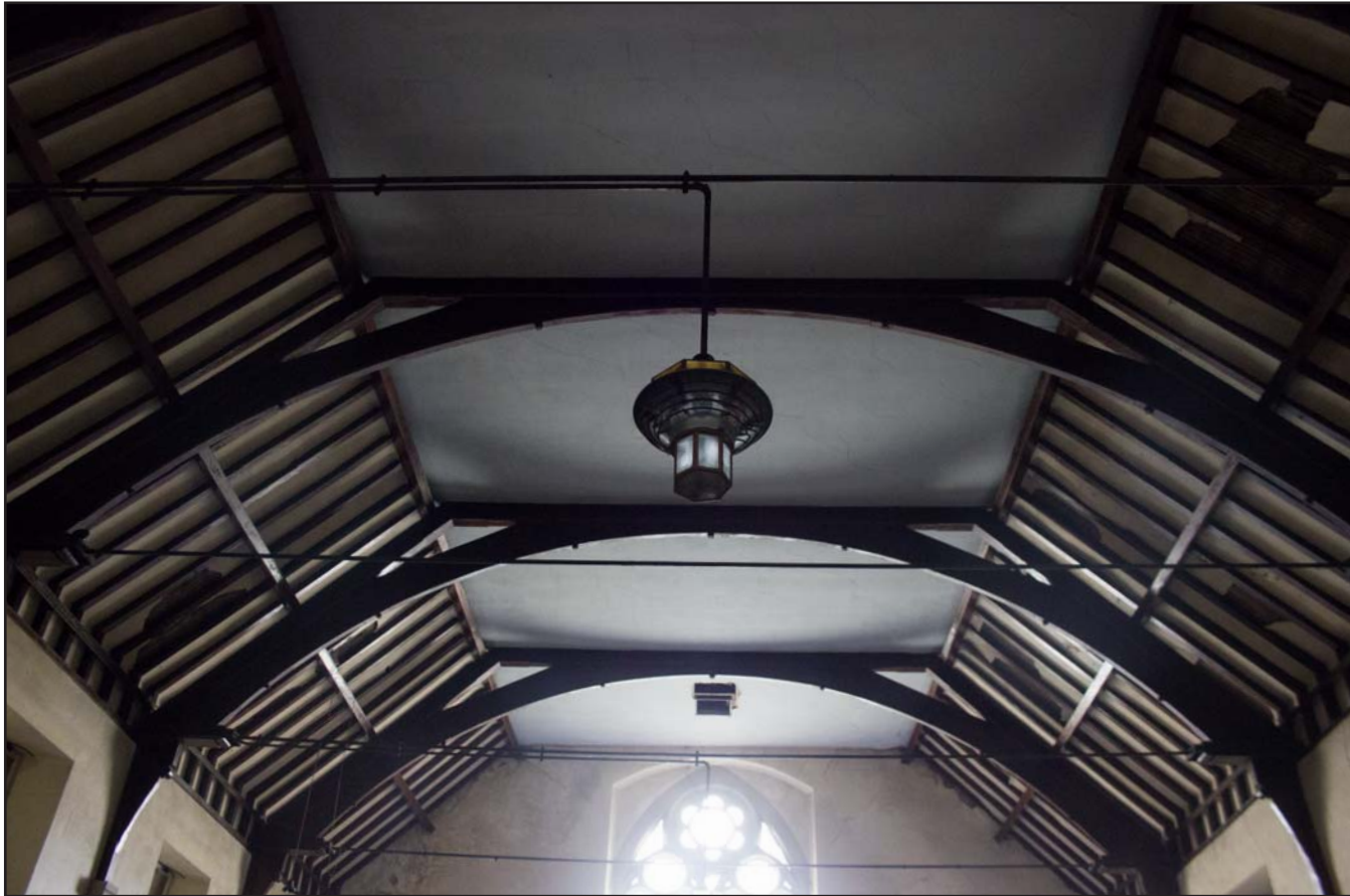
Plate 14: Chapel ceiling showing hammer beam truss, from the west.
