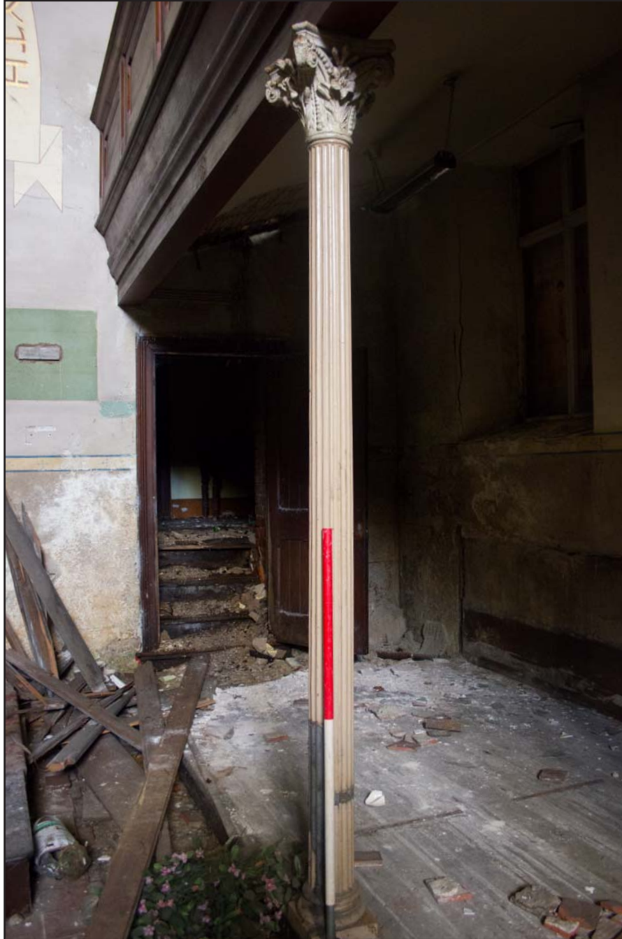
Plate 24: Chapel showing cast-iron gallery column, from the southeast. Scale 1.0m.
