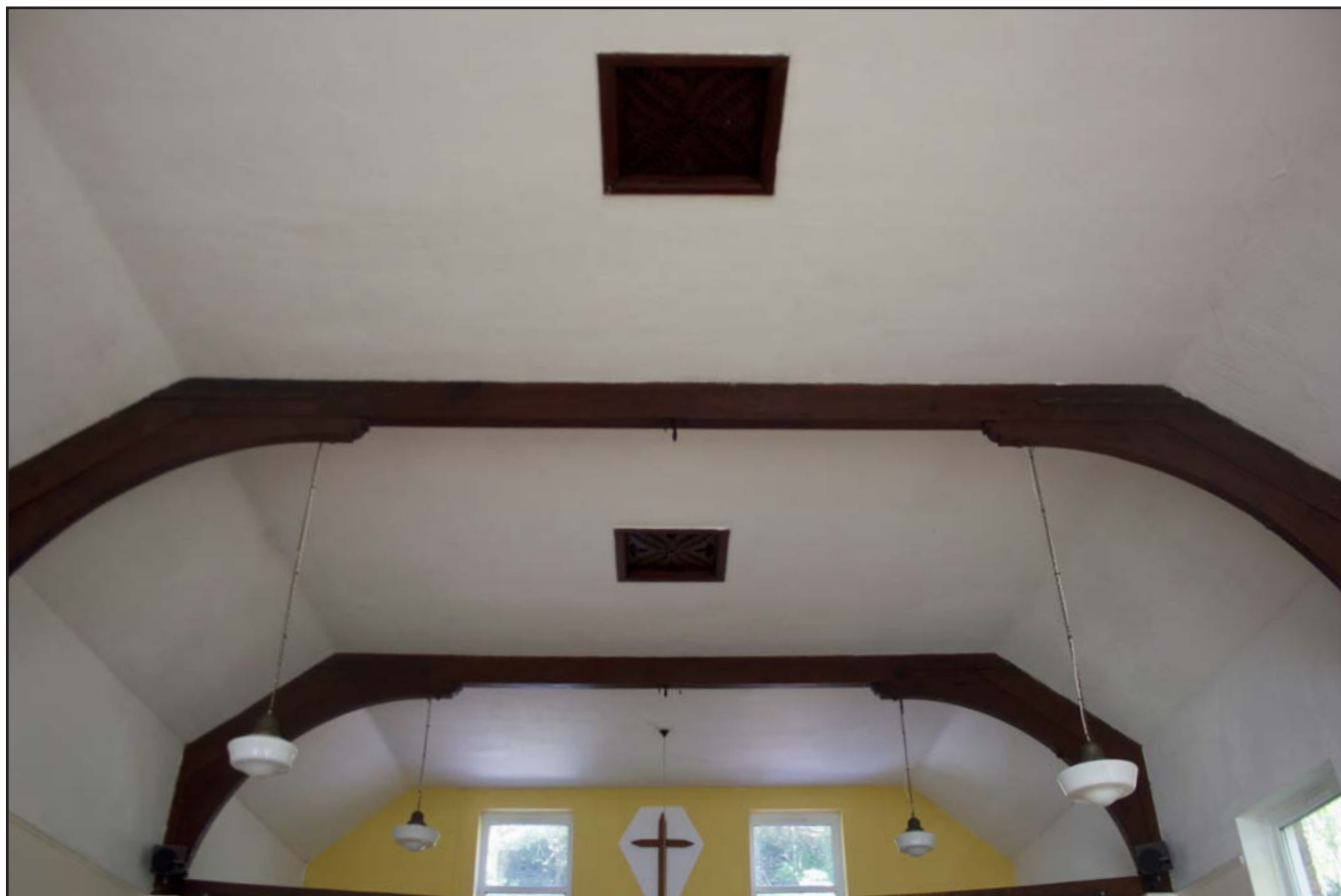
Plate 28: Chapel showing ceiling trusses with arched braces, from the east.
