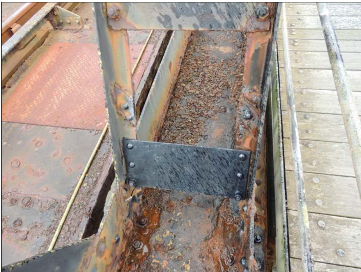
Plate 35. Plan shot of rectangular metal plate with rivets replacing corroded lattice work on hogback lattice trusses on the spans of the viaduct.
