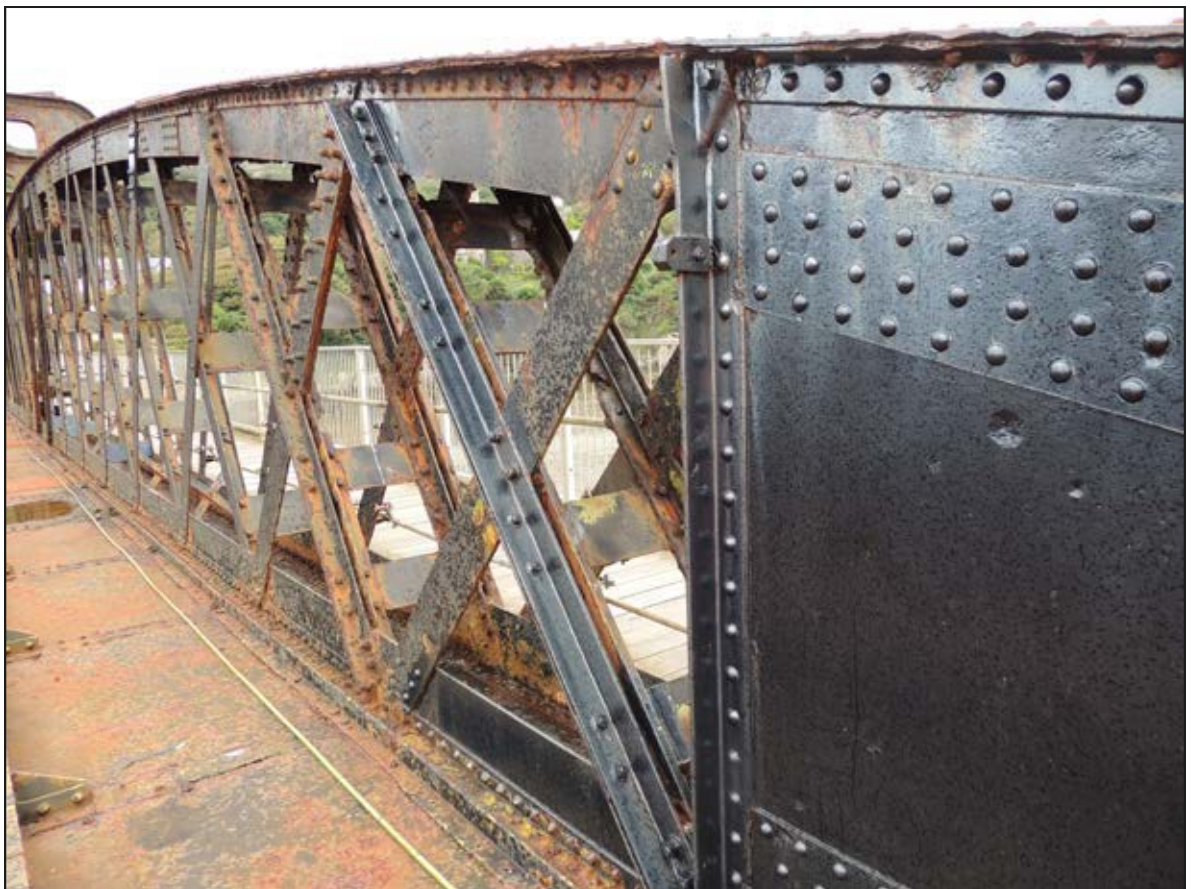
Plate 28. N facing shot of replacement metalwork on the hogback lattice trusses on the span of the viaduct.
