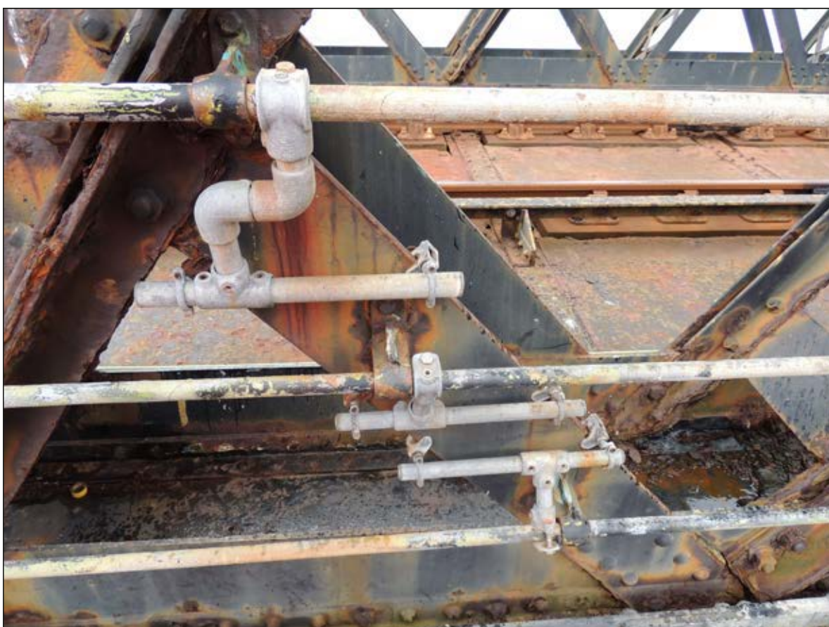
Plate 32. SW facing shot of stainless steel handrail clamps attached to corroded lattice trusses on the spans of the viaduct.
