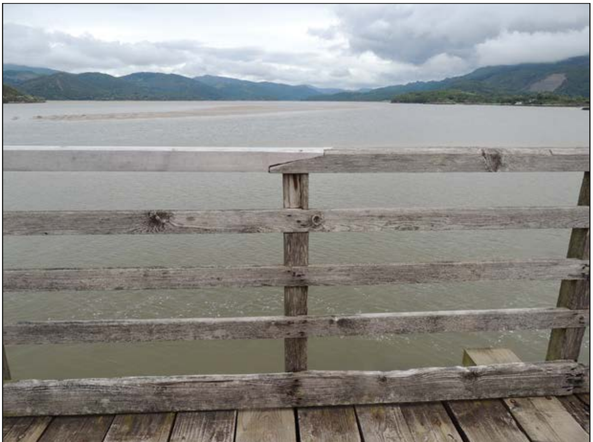
Plate 16. NE facing shot of repaired timber hand rail of walkway at trestle 14.
