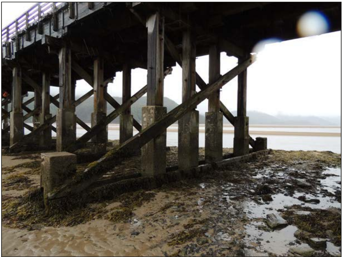
Plate 45. N facing shot showing verticle piles with reinforced concrete pile casing and diagonal beam & horizontal waling of trestle 2.
