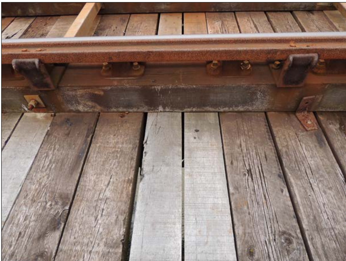
Plate 17. Plan shot of replacement transverse deck planks at trestle 15.
