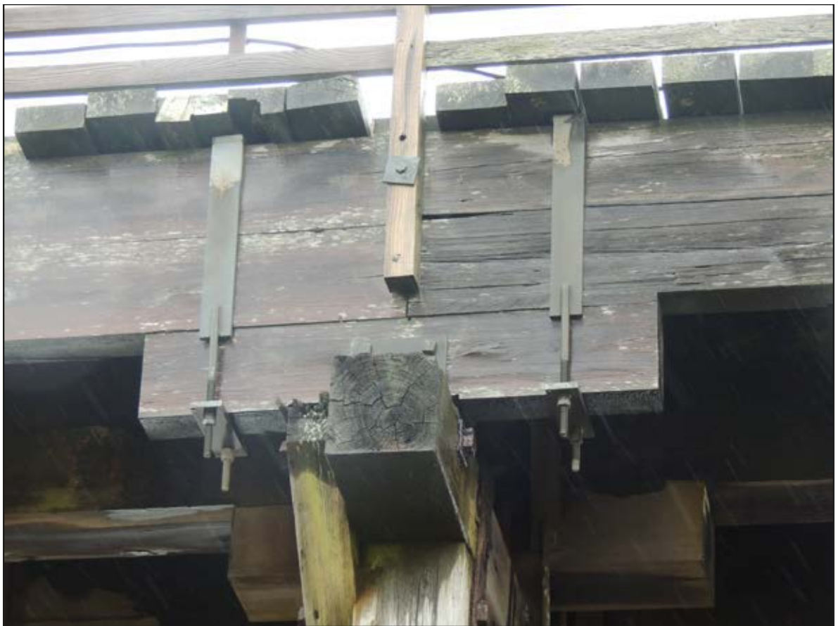
Plate 59. Shot of galvanised steel straps attached to longitudinal outer beam above trestle 87.
