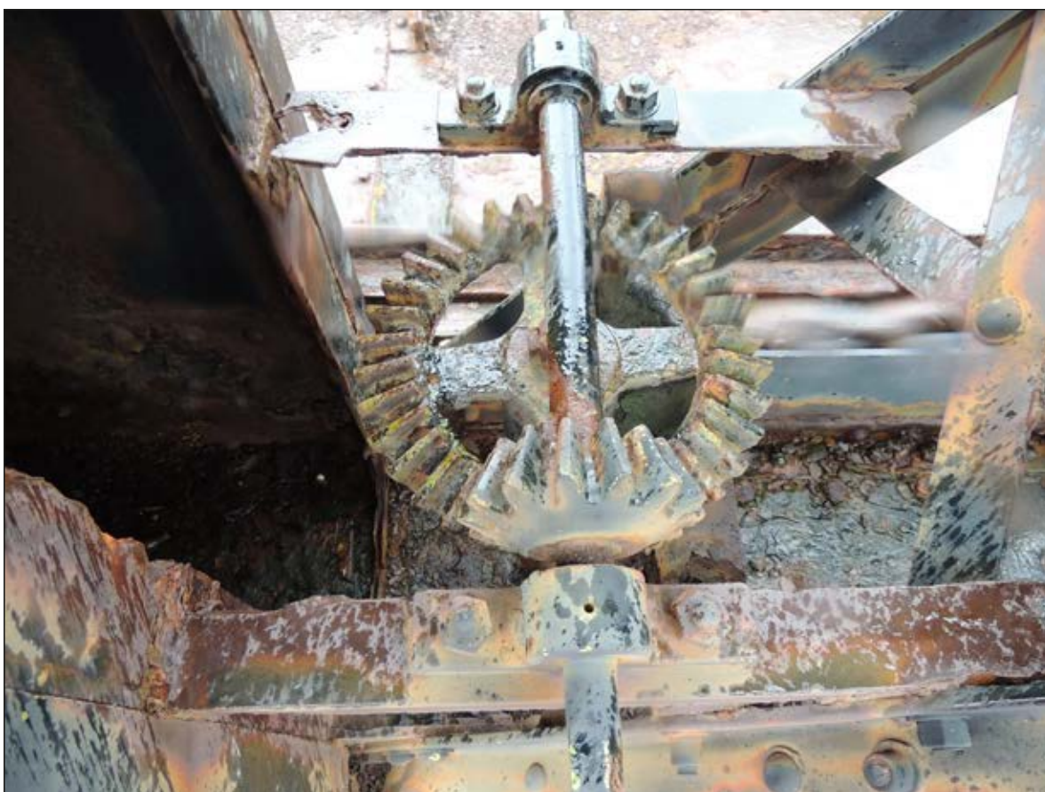
Plate 38. Plan shot of handcrank mechanism on the NE elevation of hogback lattice trusses on the spans of the viaduct.
