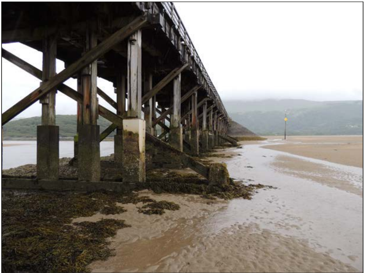
Plate 47. ESE facing shot of trestle 14 showing vertical pile with a protective covering over concrete pile casing.
