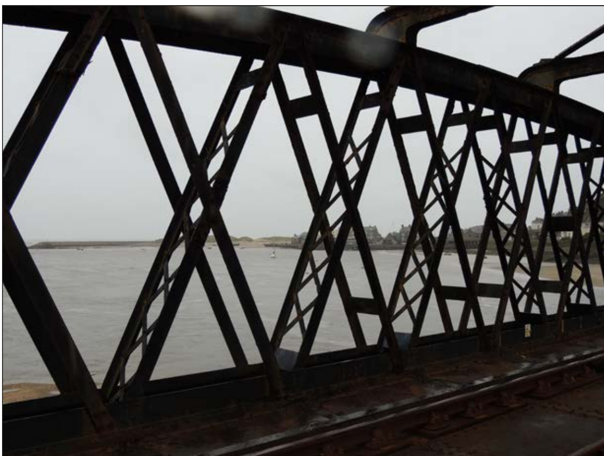
Plate 36. WNW facing shot of intact latticework on the hogback lattice trusses on the SW elevation of the spans of the viaduct.
