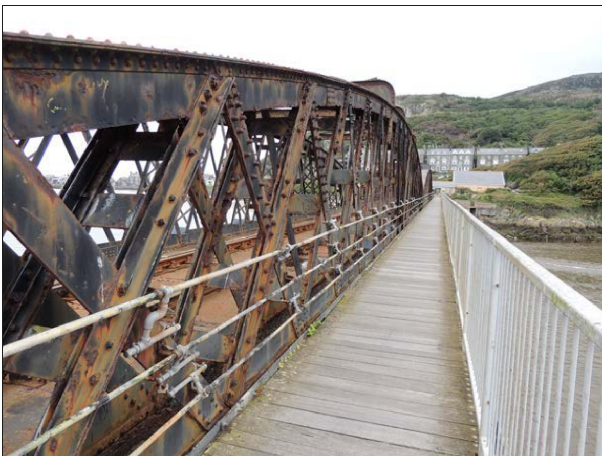
Plate 30. NNW facing shot of hogback lattice trusses on the span of the viaduct from the walkway.
