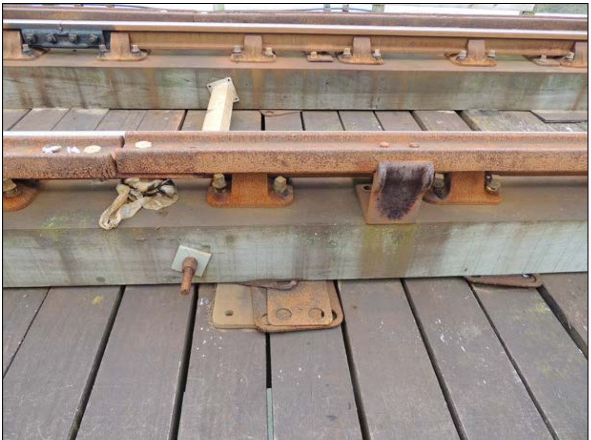
Plate 24. SW facing shot of metal plates supporting the track due to slumping of the transverse deck planks at trestle 81 and 82.
