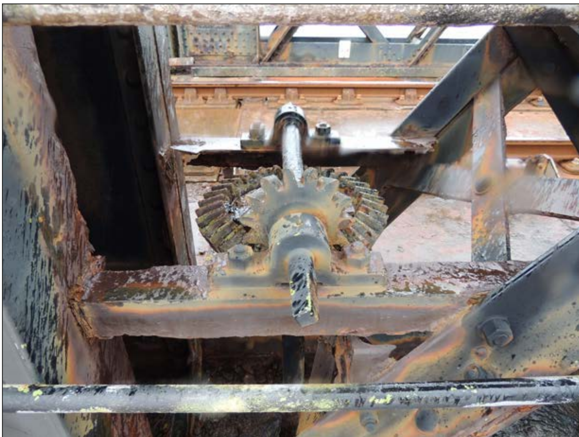
Plate 37. SW facing shot of hand crank mechanism of the swing bridge on NE elevation of hogback lattice trusses on the spans of the viaduct.
