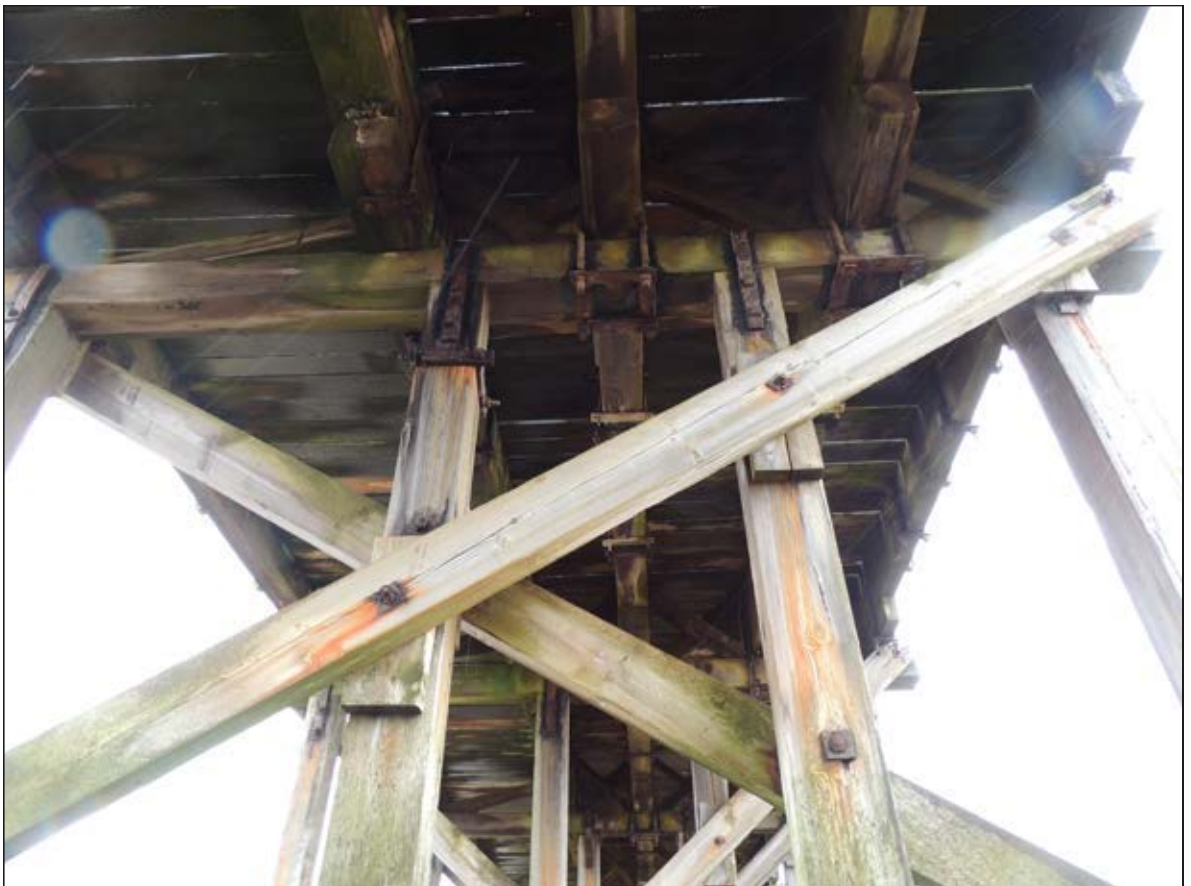
Plate 48. Shot of earlier steel straps attached to support beams for transverse deck planks, trestle 22.
