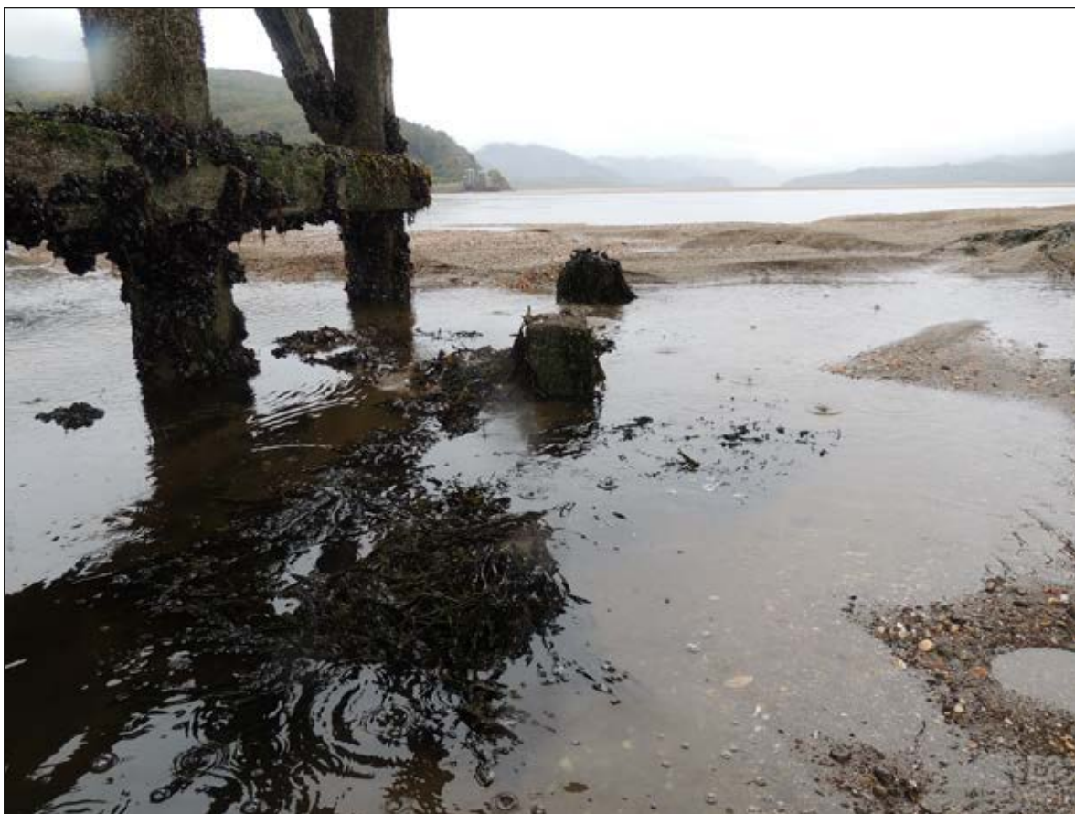
Plate 53. NNE facing shot of remains of verticle pile stumps under trestle 55.
