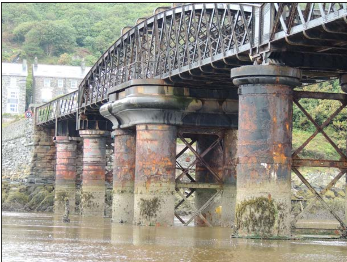
Plate 63. NNE facing of cluster of the cylindrical iron piers to support the turn table of swing bridge.
