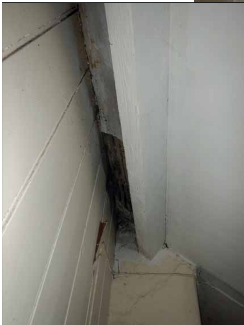
Plate 55. Exposed lathes in Landing ceiling.
