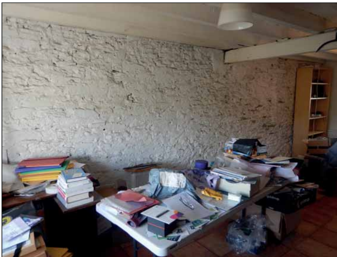
Plate 24. South wall of Dining Room, showing rubble stone construction, looking south-west.
