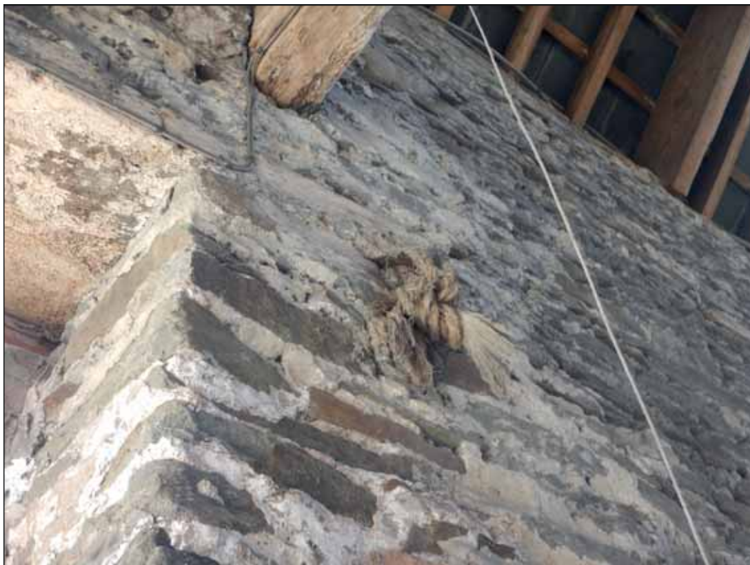
Plate 48. Horseshoe mortared into east wall as tie ring, looking south-east.
