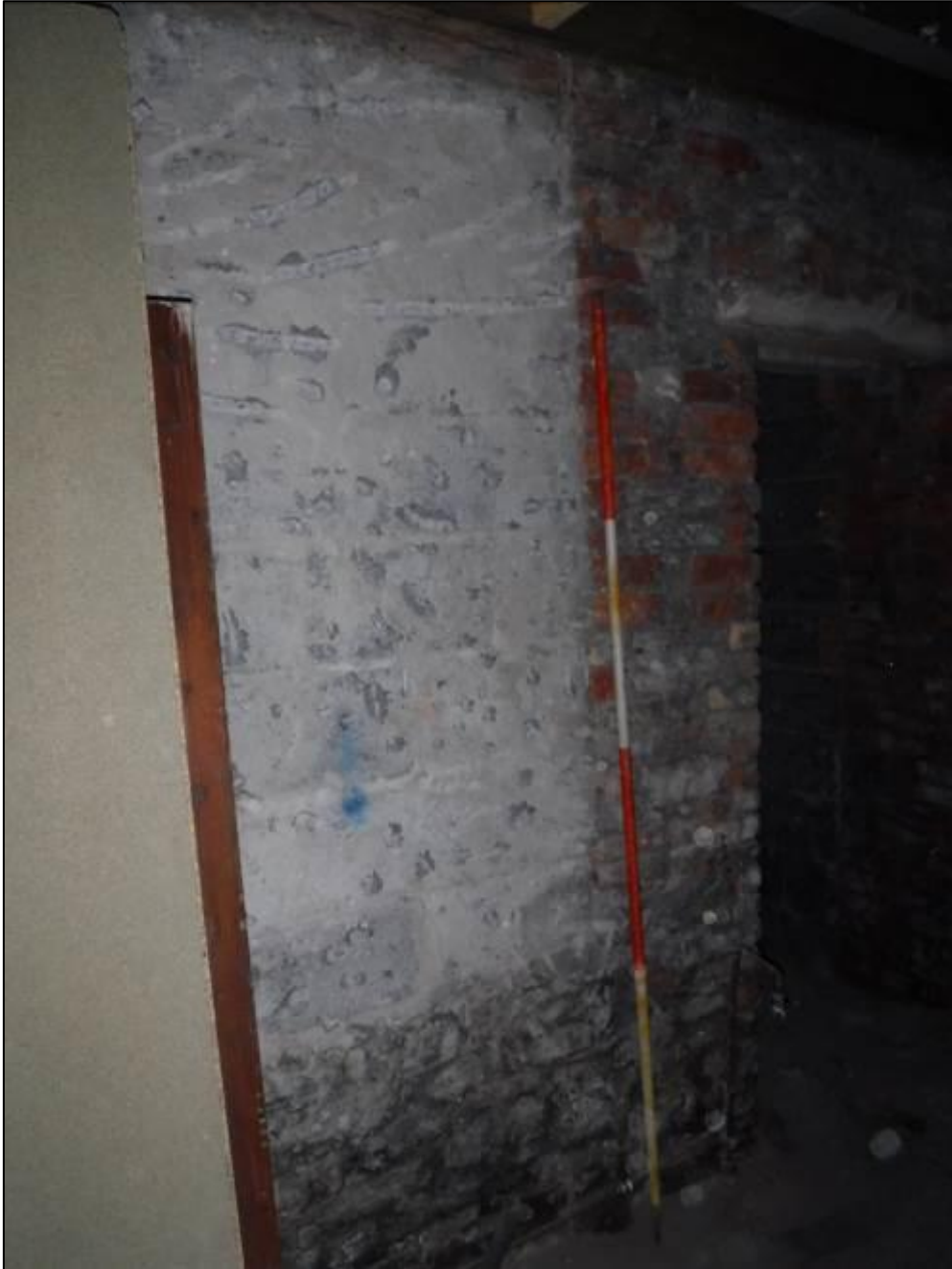
Plate 65. Ground floor, Room 5: eastern wall and original exterior wall of building, with blocked window clearly visible, alongside doorway to Room 4, south-east facing, 2m scale
