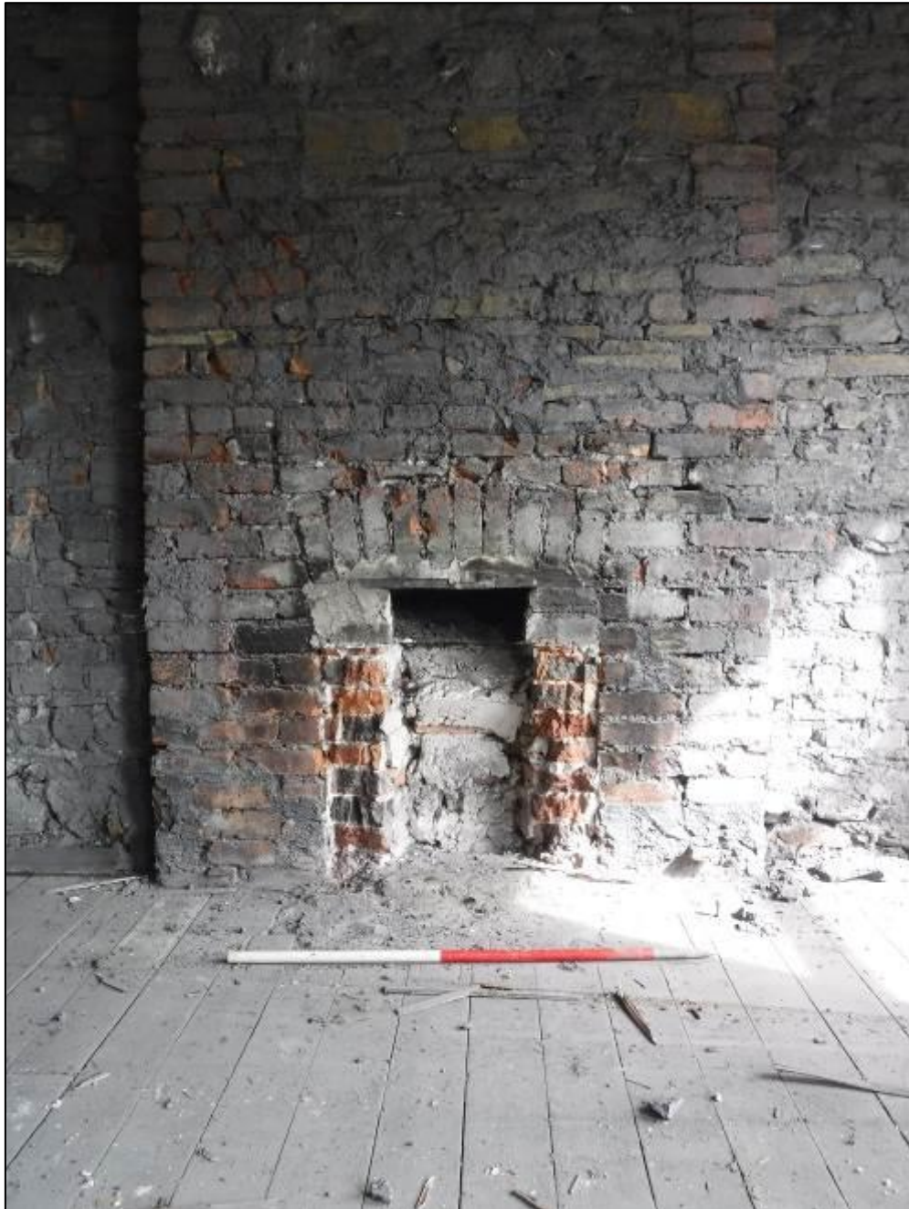
Plate 24. First Floor, northern wall, chimney breast with blocked fireplace, facing north, 1m scale
