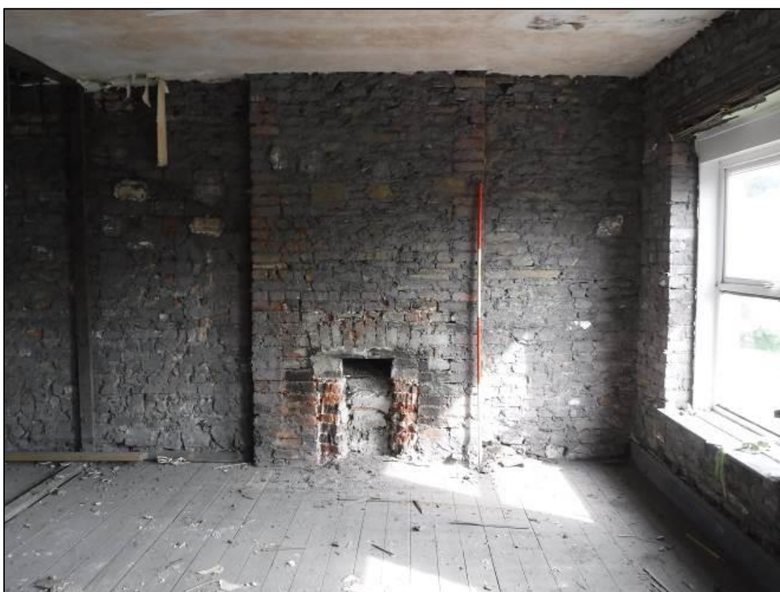
Plate 23. First Floor, northern wall, chimney breast with blocked fireplace, facing north, 2m scale
