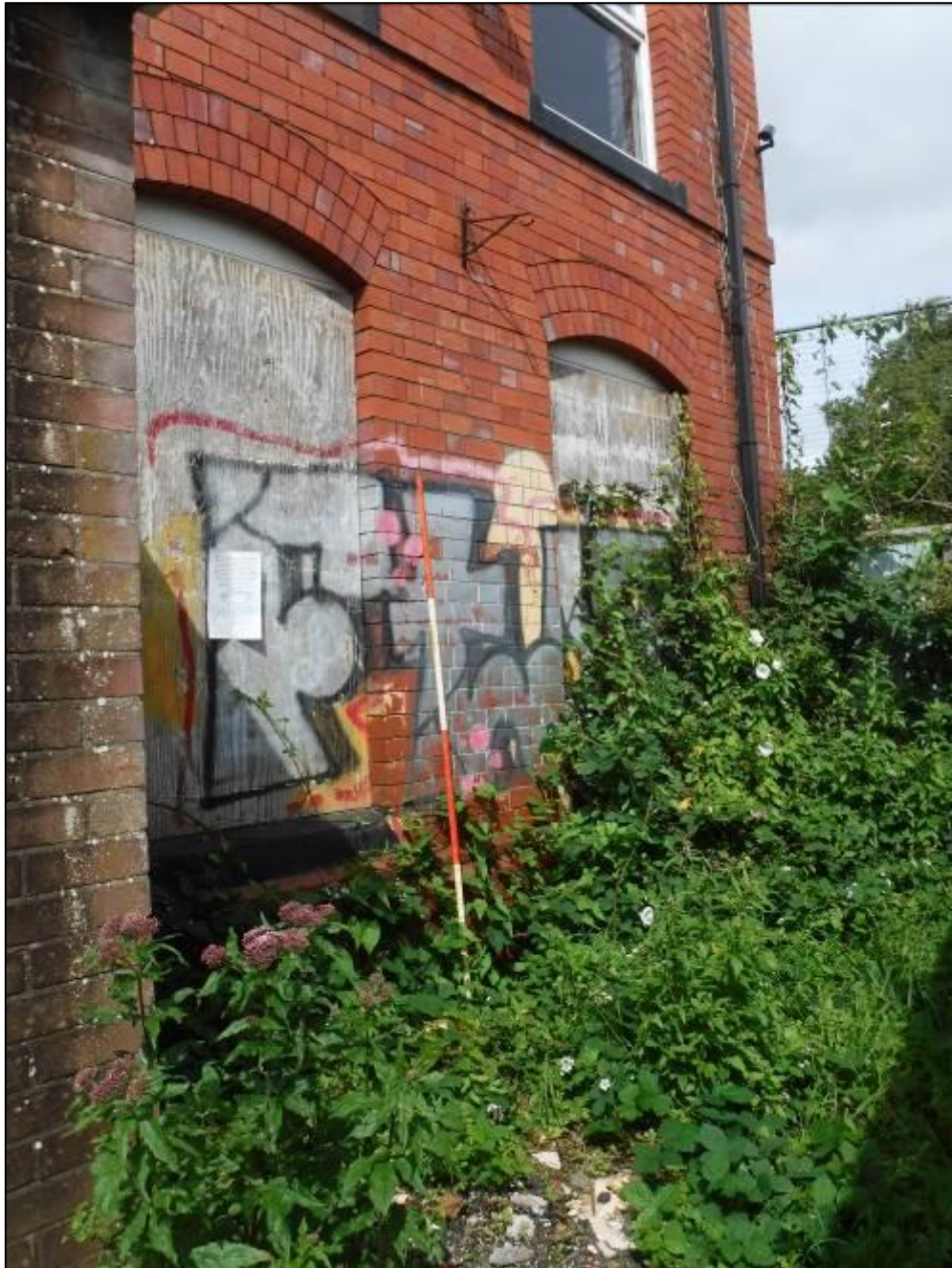
Plate 3. Two windows on ground floor of front elevation, with segmental arches and stone lintels, north-west facing, 2m scale.
