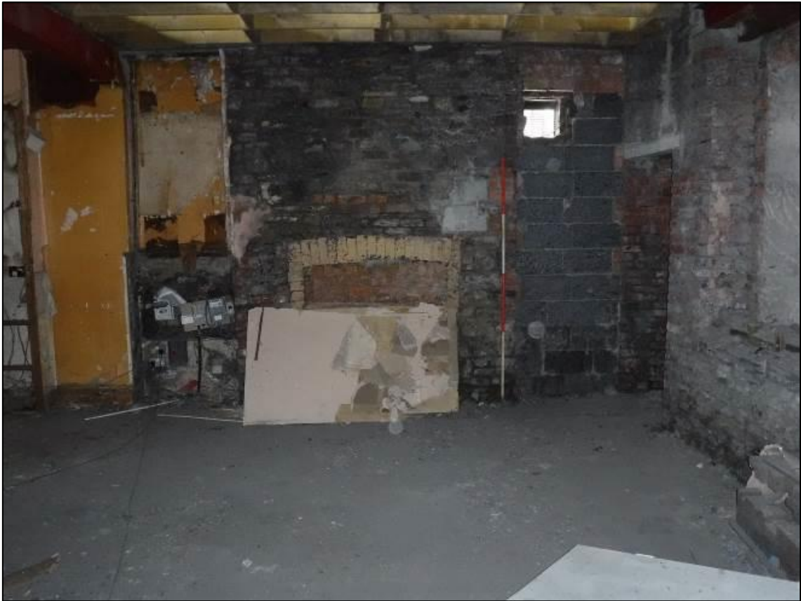
Plate 61. Ground floor, Room 4: southern wall with chimney breast and bricked-up fireplace, south facing, 2m scale
