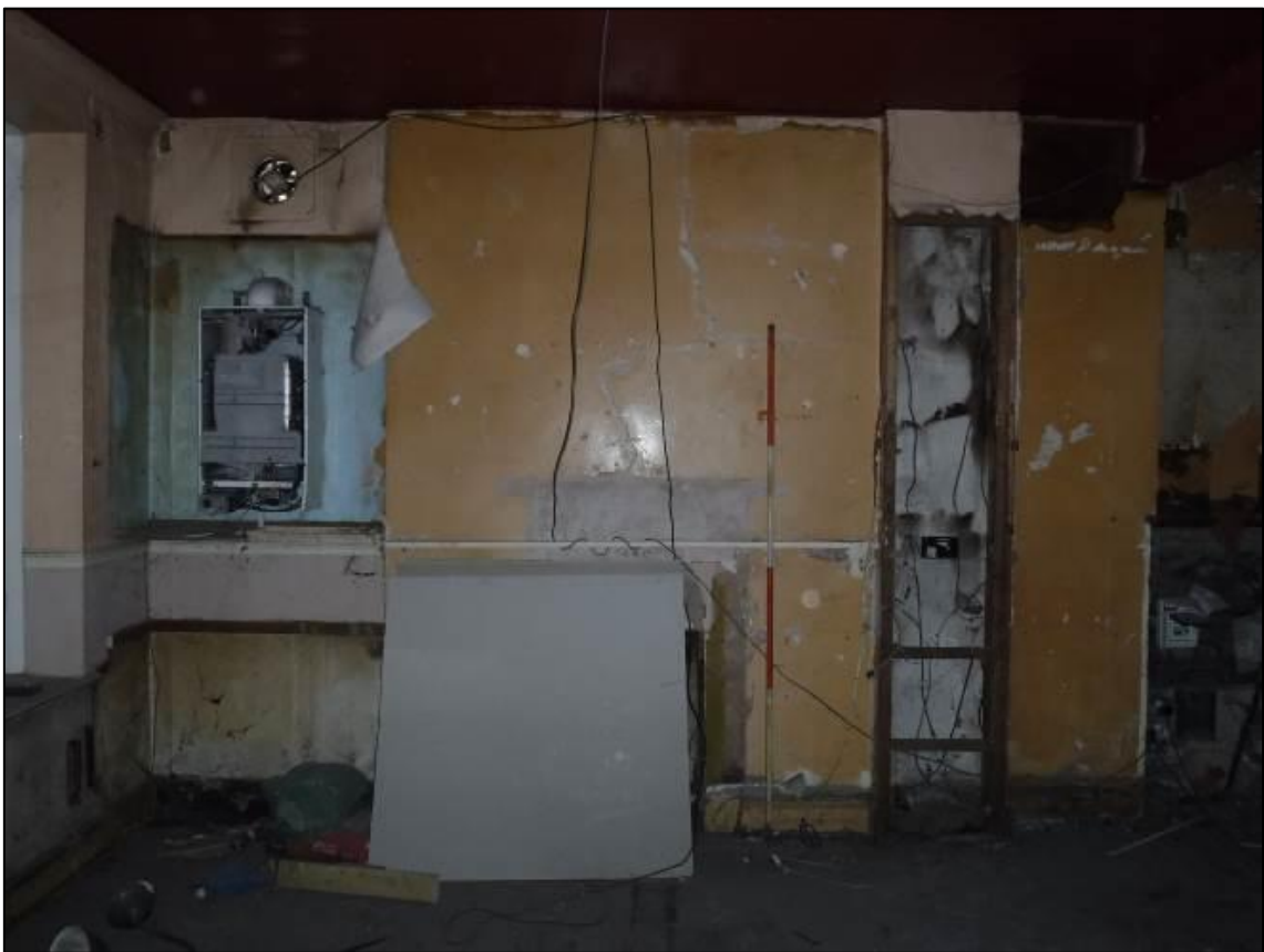
Plate 62. Ground floor, Room 4: southern wall with chimney breast with fireplace covered up by plaster and paint, south facing, 2m scale
