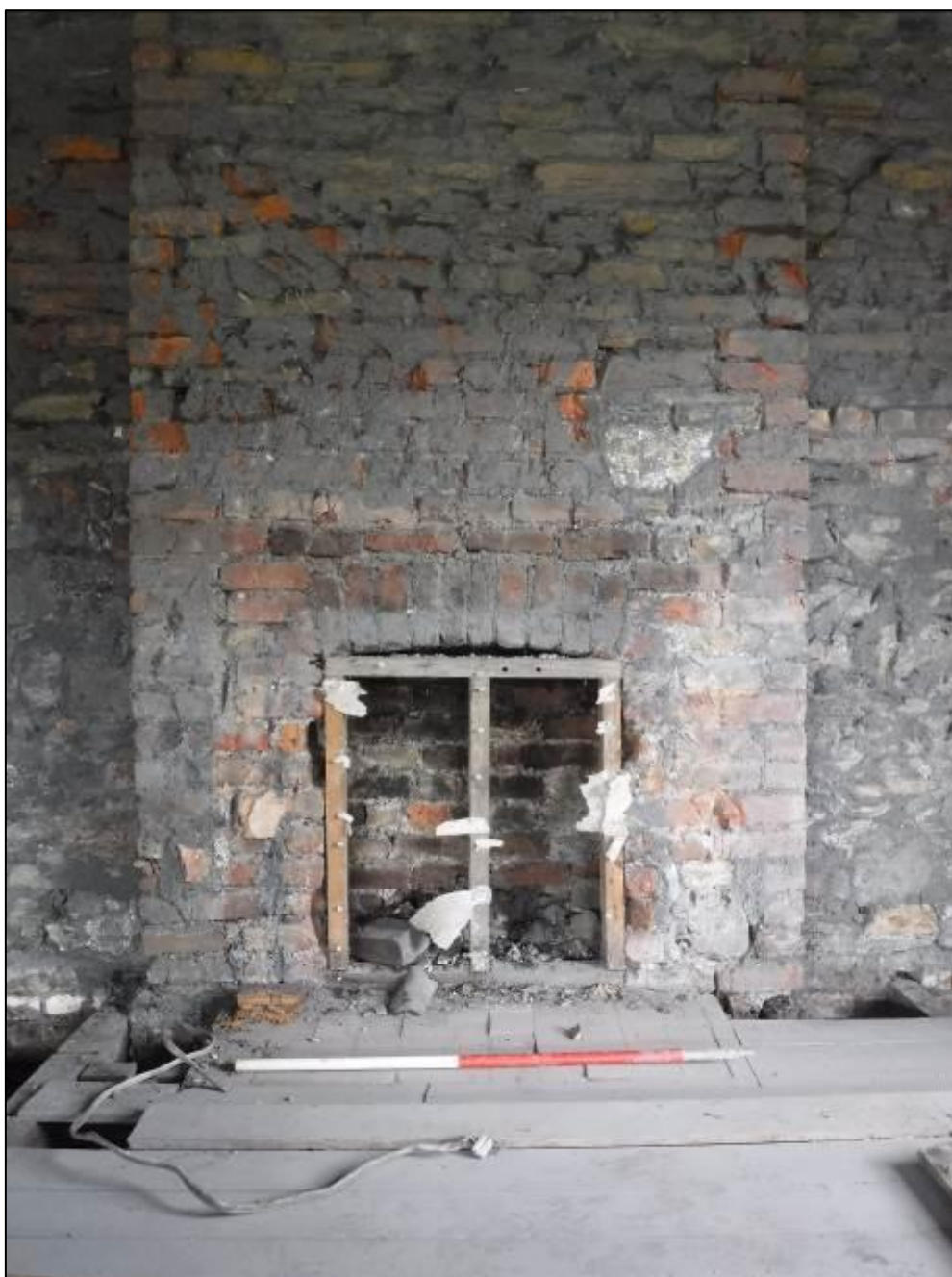
Plate 21. First floor: western wall, chimney breast previously had been blocked by a wooden framed partition, facing west, 1m scale
