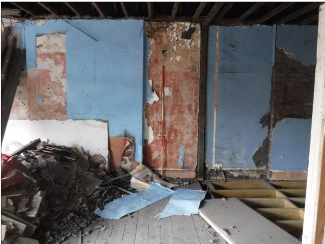
Plate 30. First floor: southern wall, chimney breast behind debris and covered by plaster and wallpaper, south facing, 2m scale
