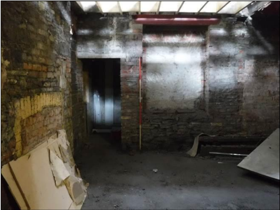
Plate 63. Ground floor, Room 4: view towards western wall, original window can clearly be seen blocked up with concrete blocks, with doorway to Room 5 adjacent to window, west facing, 2m scale
