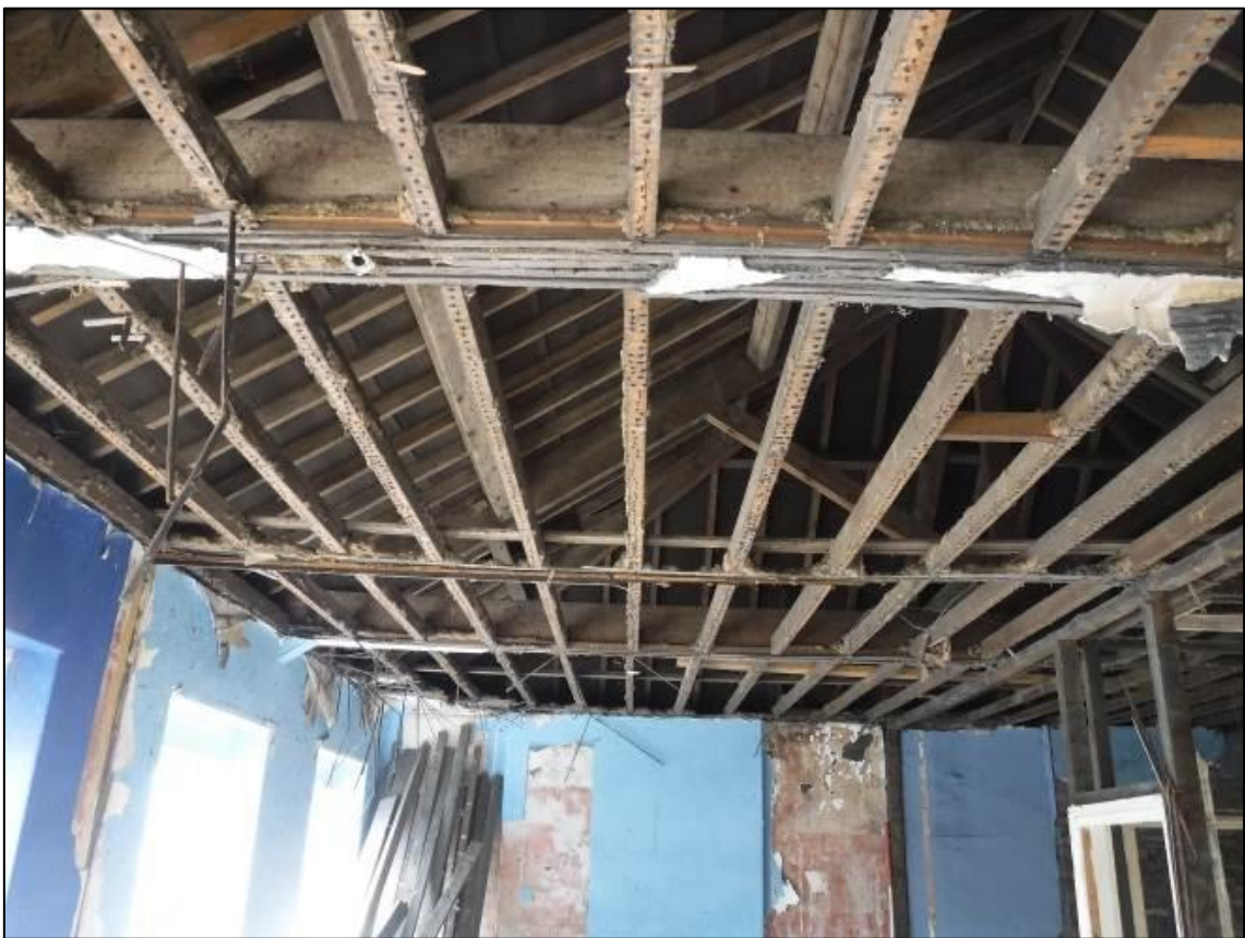
Plate 47. First floor: view of attic space and exposed ceiling joists, south facing
