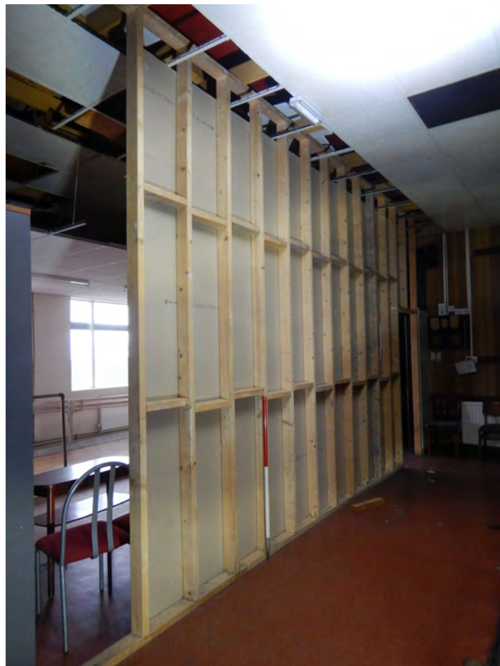
Plate 92. Recently added stud wall, Room 8, looking south
