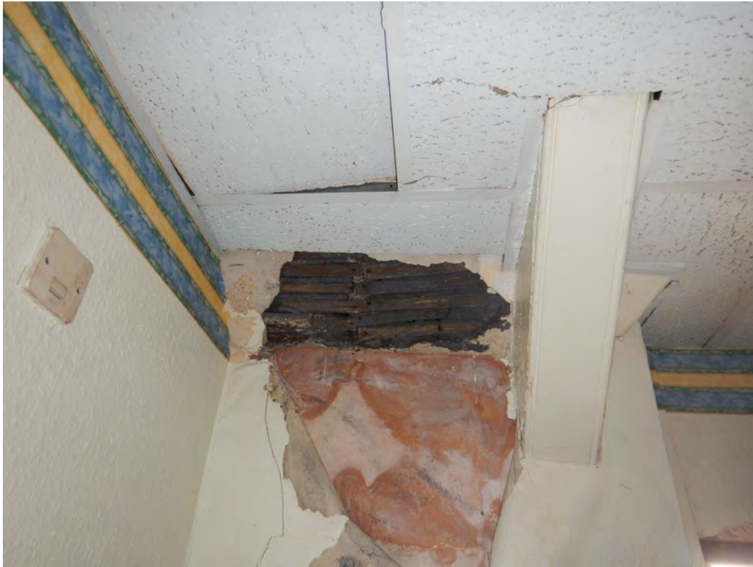
Plate 195. Exposed lathes in the east corner of the Artist's Room, looking east
