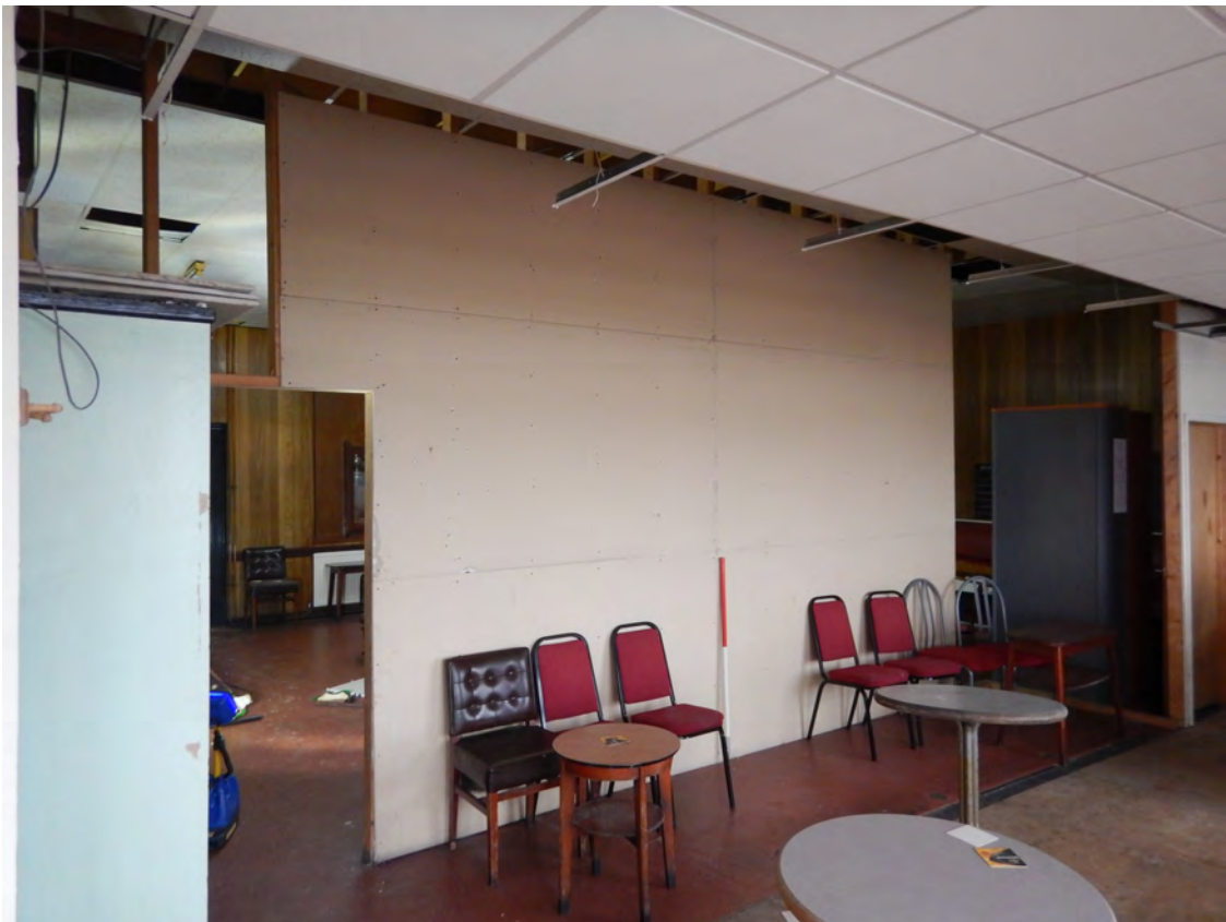
Plate 88. Recently added stud wall, Room 7, looking north
