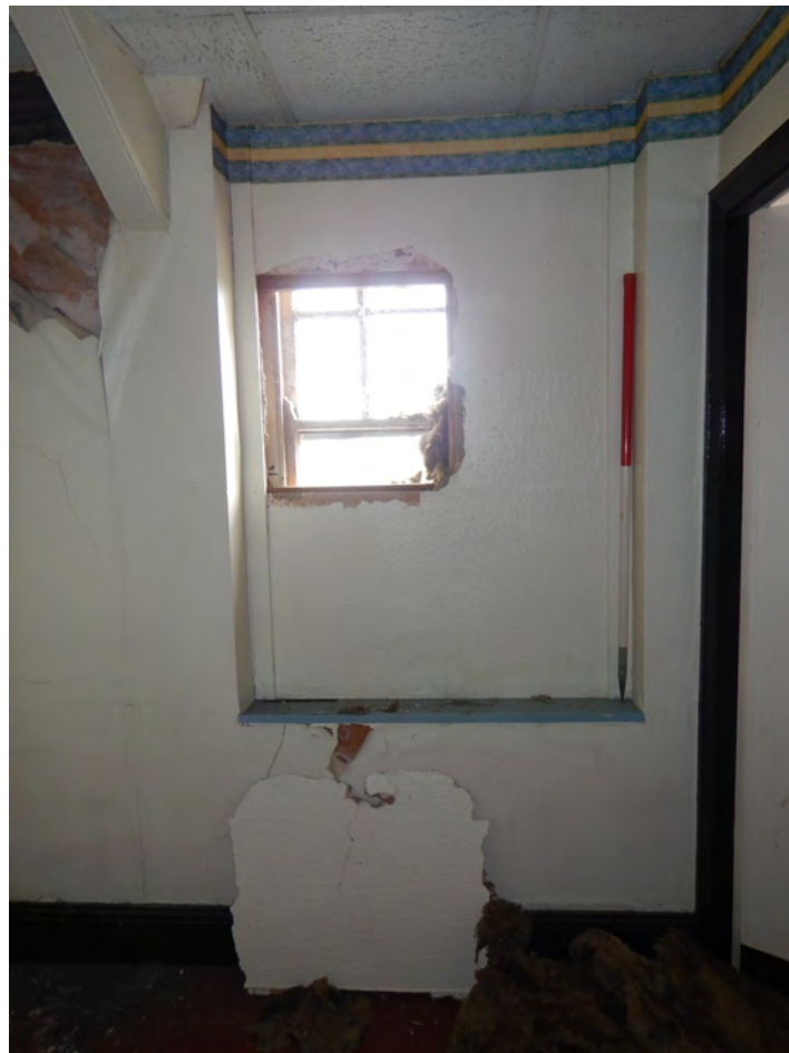
Plate 196. Blocked window on south-east wall of Artist's Room, looking south-east
