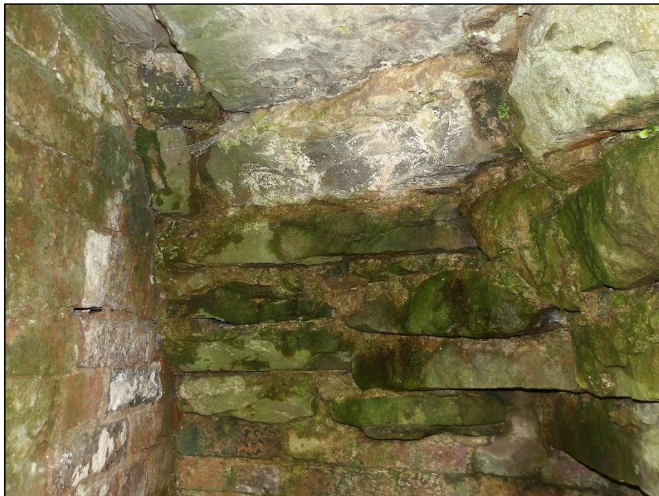
Plate 30: Corbelled roof. Staircase interior
