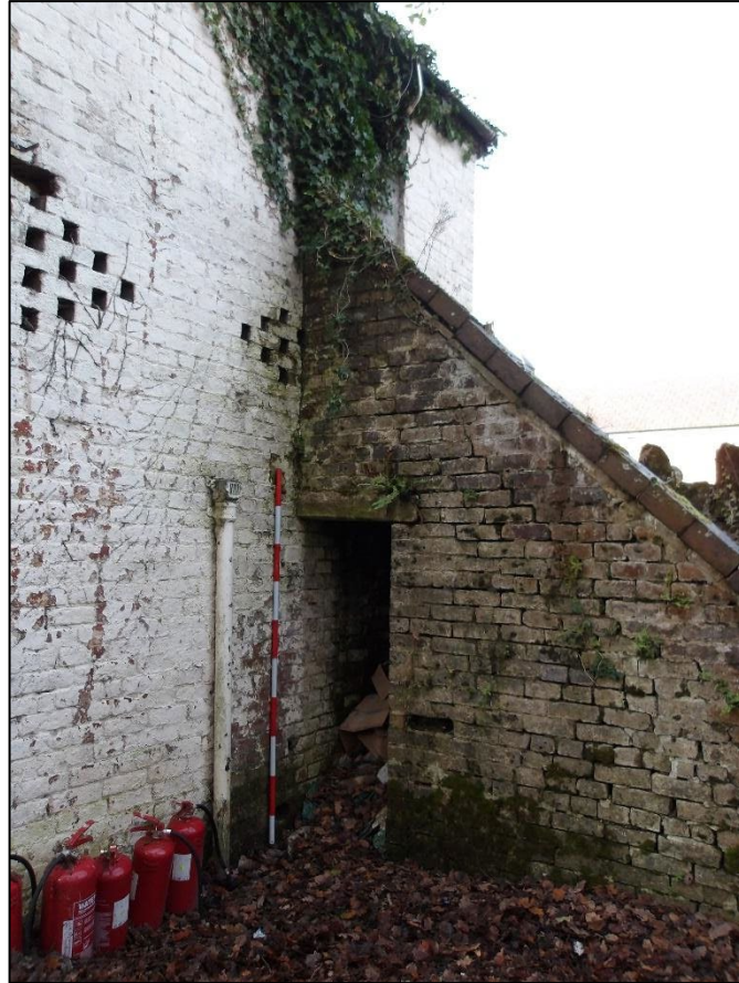
Plate 27: Diamond-shaped ventilation openings blocked by staircase. Northeast facing section of coach house. 2m scale
