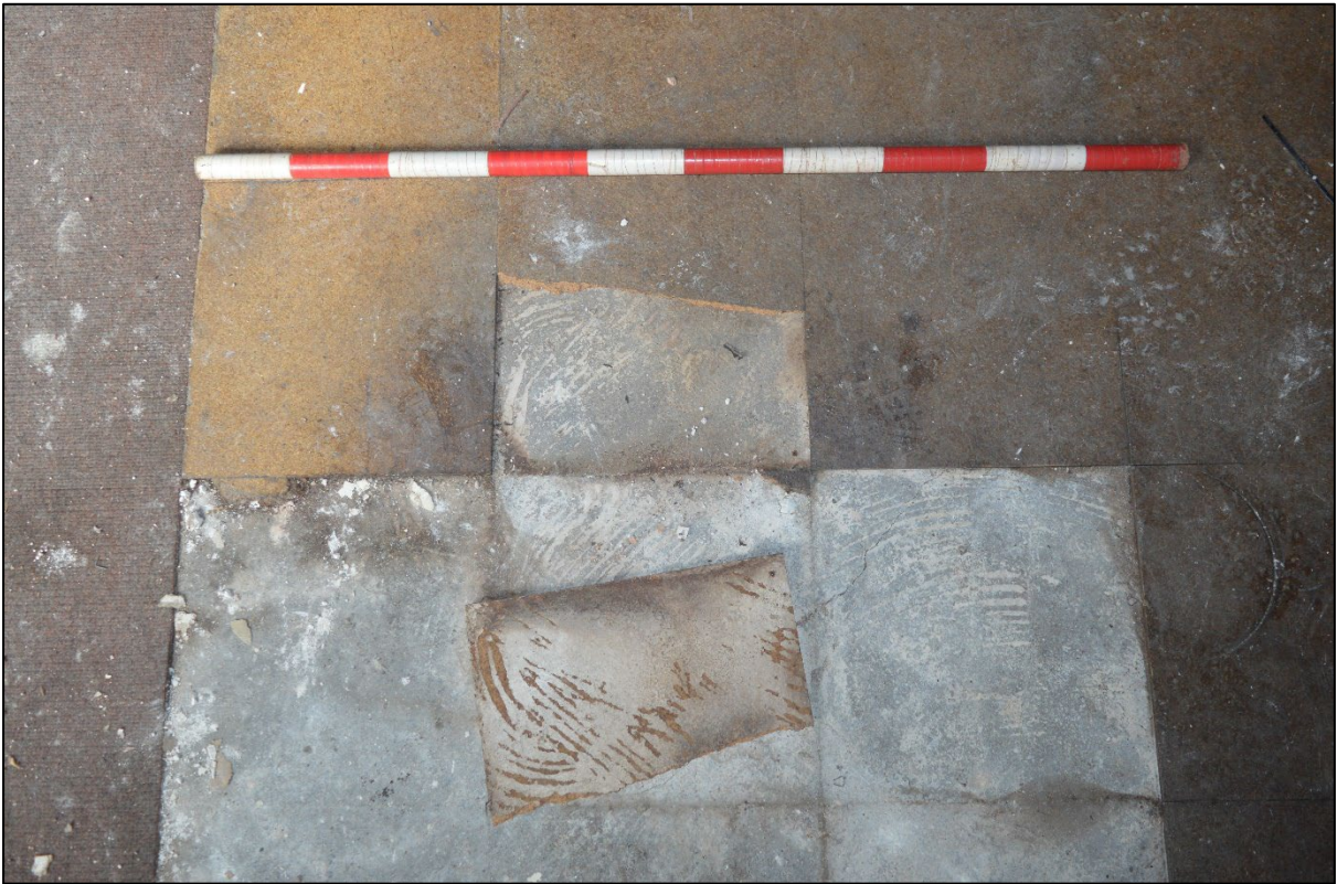
Plate 27: Damaged area of cork tiles within main library floor
