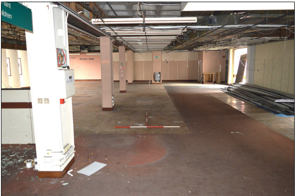
Plate 18: Cork tiles on main library floor, central area, looking north
