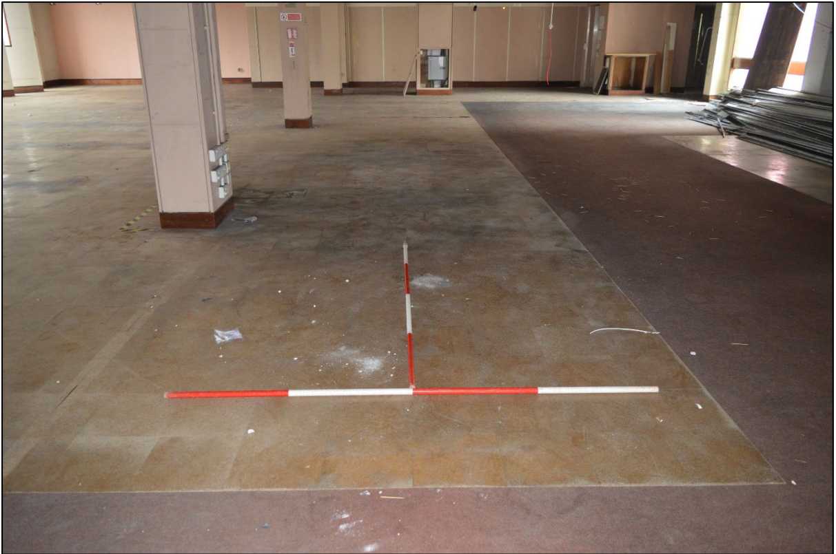
Plate 19: Cork tiles on main library floor, central area, looking north
