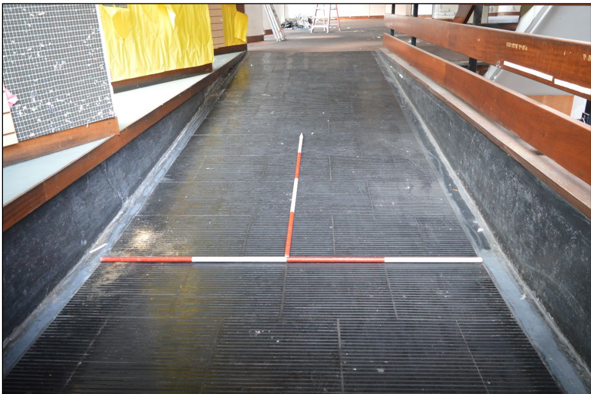
Plate 4: Detail of black rubberised surface, entrance ramp, looking west
