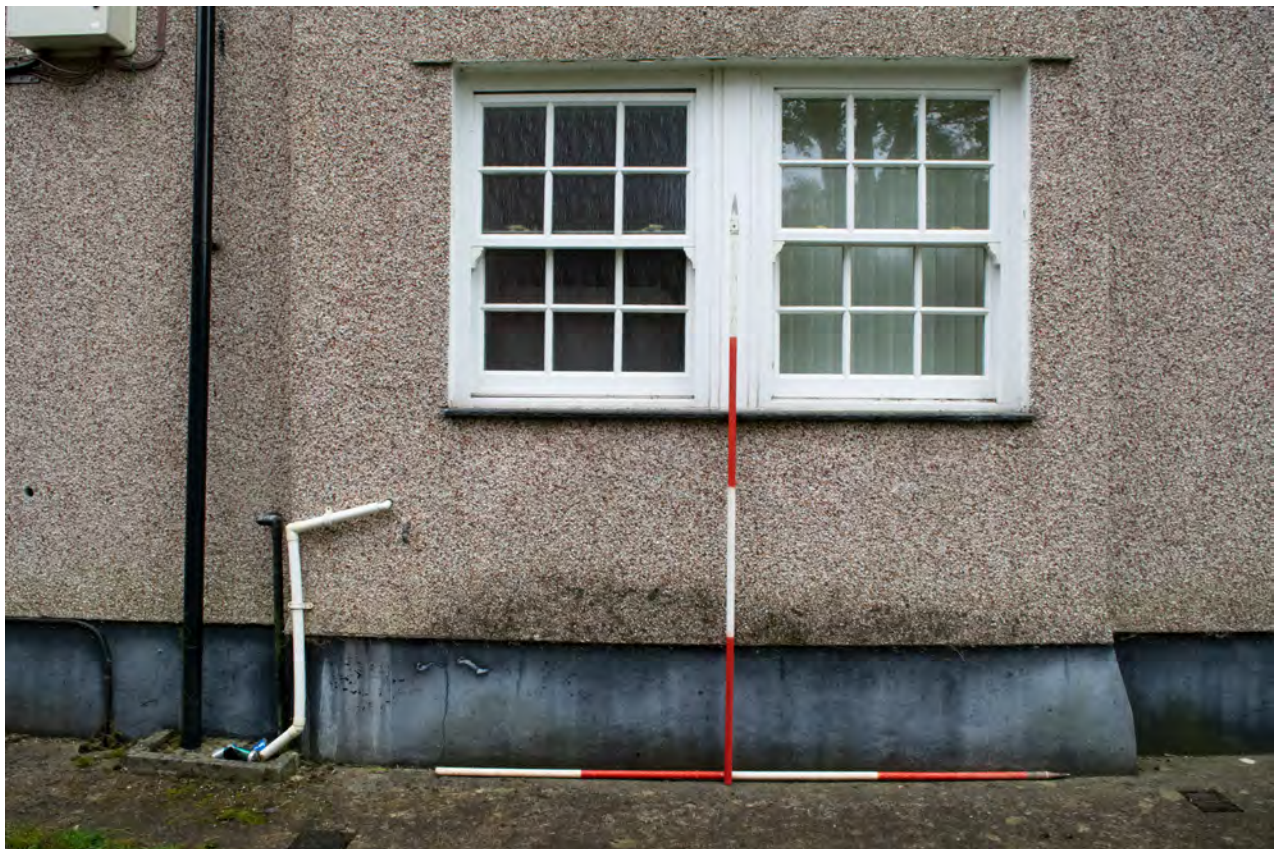
Plate 12. Close up of double hung sash window on northern elevation. 2x2m scale.
