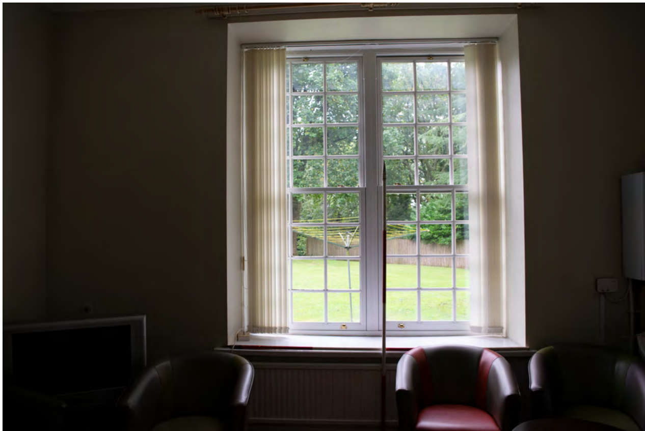
Plate 41. Double hung sash windows on eastern wall of piano lounge. 2x2m scale.
