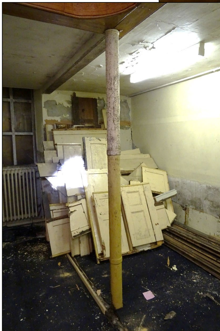
Plate 43: Cast iron post supporting gallery, looking south-west.
