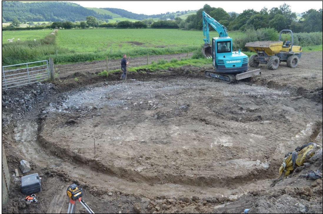
Fig. 4: The ring foundation for the new slurry store. Photo HENEB PD24-088-007
