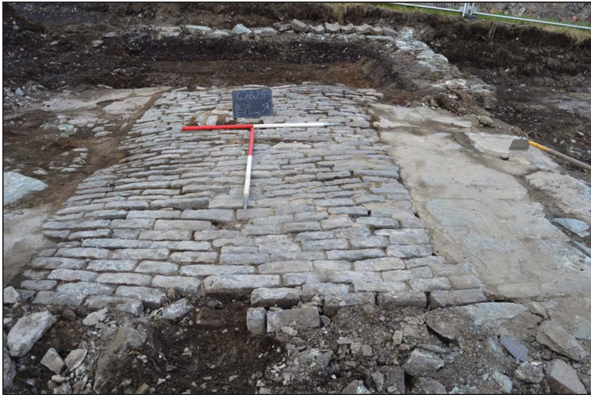
Plate 44. Floor with setts (107) and slabs (110) after concrete has been removed. View from south-east, scales 1m (archive reference: G2825_270)
