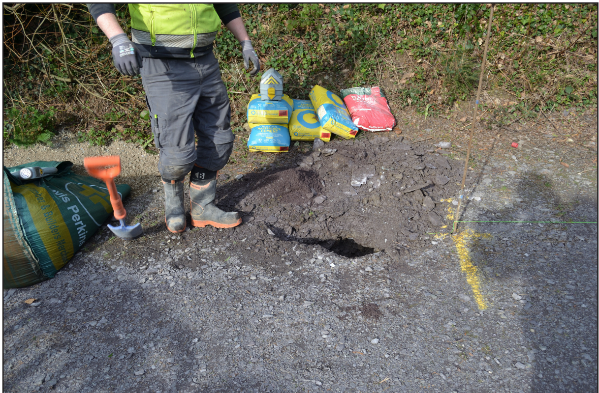
Plate 6: - Working shot of test pit being dug to find existing cable duct; scale not used; view from SE (archive reference: E49185_06).
