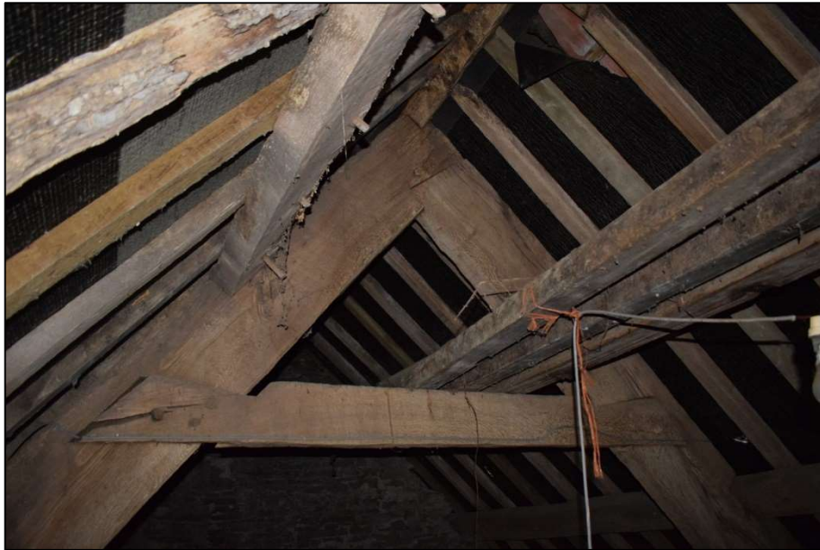
Fig. 12 Upper southern truss viewed from the north and loose collar tie. Photo HENEB PD24-063-050
