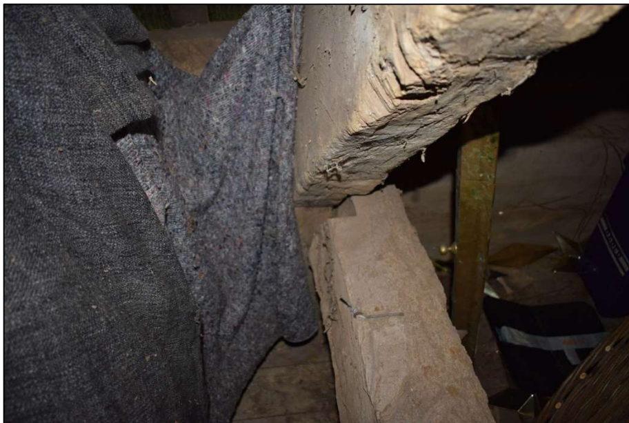
Fig. 13 Lower northern truss (top) and partially dislocated tie beam Photo HENEB PD24-063-047
