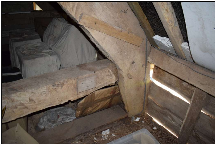
Fig. 15 Detail of the lower cruck, tie beam and wall plate viewed from the south-west Photo HENEB PD24-063-046
