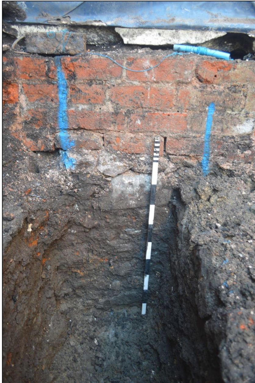
Figure 13: Base of wall at southwest end of trench, with brick and stone wall on top of the clay layer (7). Facing southwest. CPAT 2752_040
