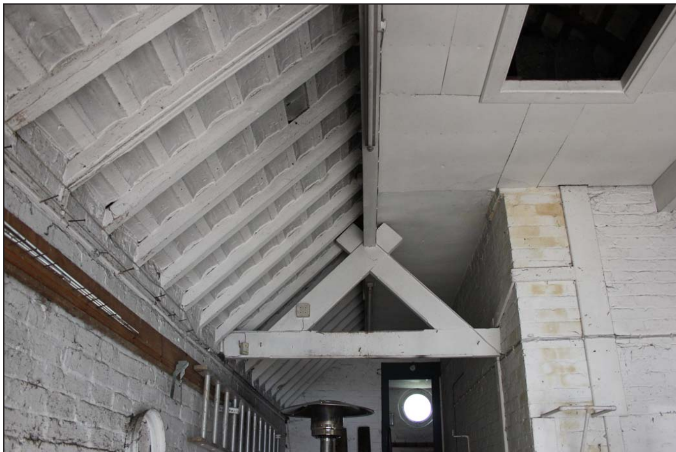
Plate 14: Ceiling in garage with possible truncated queen-post truss - from the southwest - scale 1m
