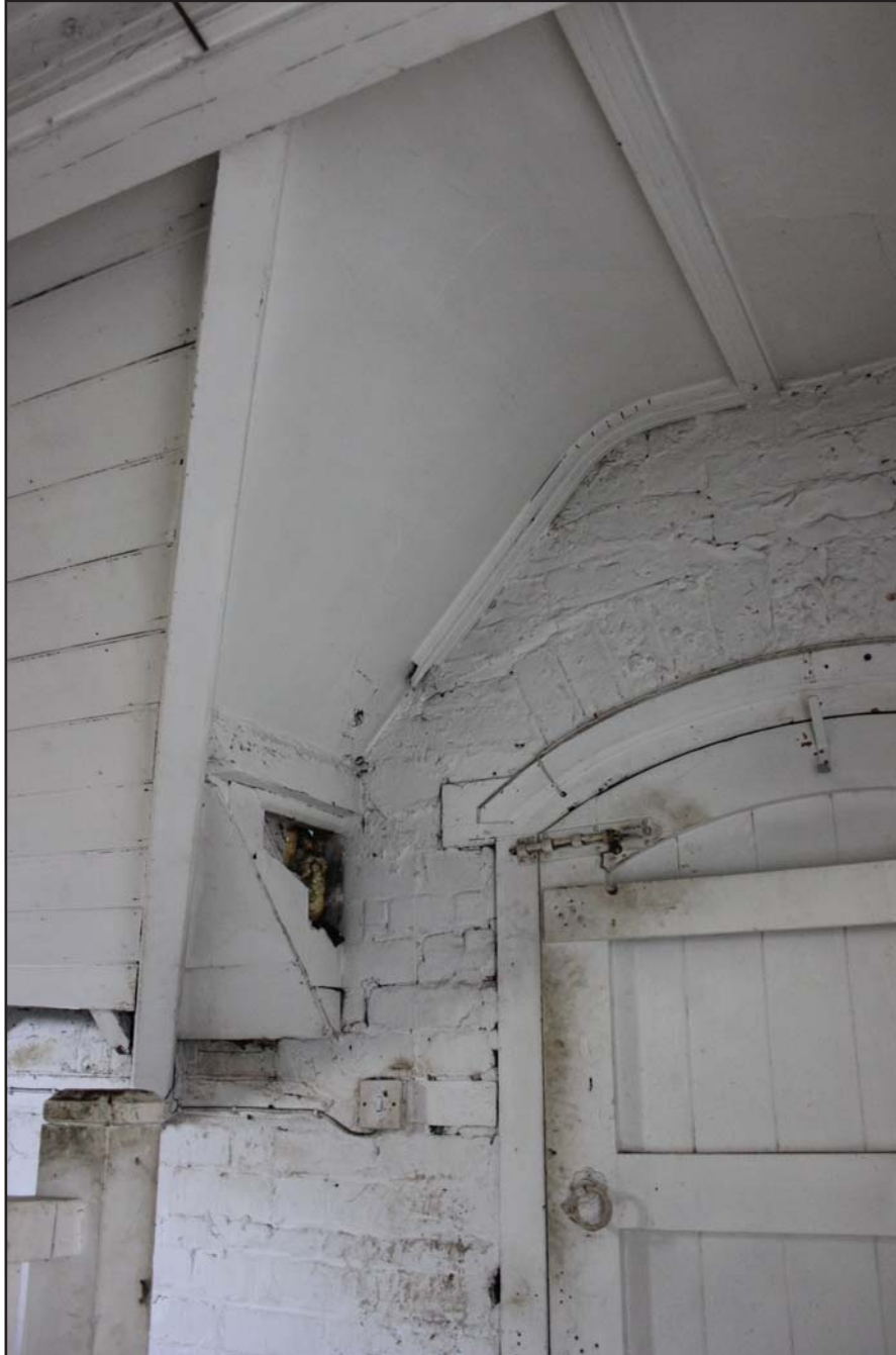
Plate 21: Timber dormer construction within ceiling construction to upper left of 3/4 door - from the west - n/a scale
