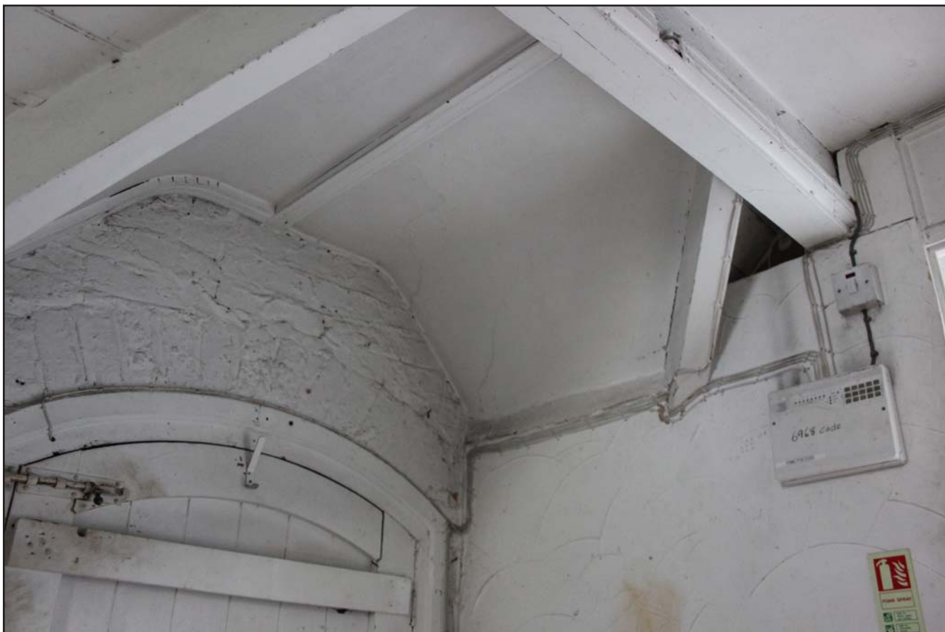
Plate 22: Timber dormer construction within ceiling construction to upper right of 3/4 door - from the north - n/a scale
