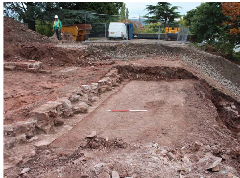
Garden walk way and demolition deposit 1035, looking south (1m scale)
