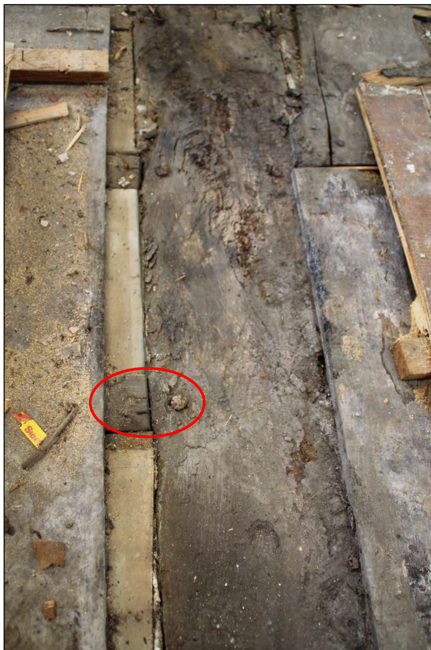
Photo 9 View of one of the beams with areas of aging, dowels to joists (circled) and boarding between joists
