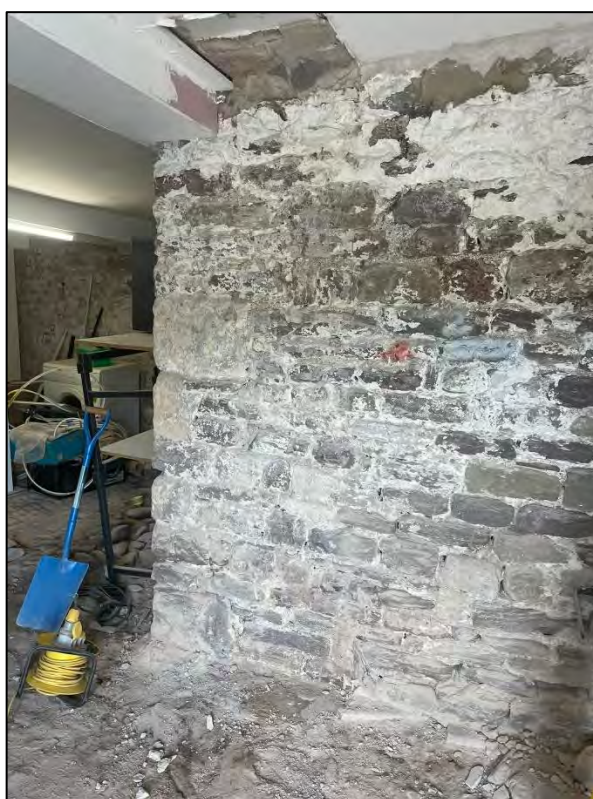
Photo 20 The undisturbed cellar wall after the concrete pier was removed
