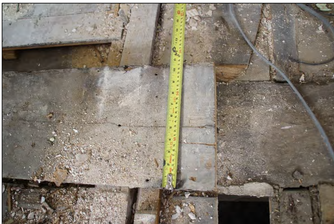
Photo 6 The oak floorboards present as the first layer over the beams and joists
