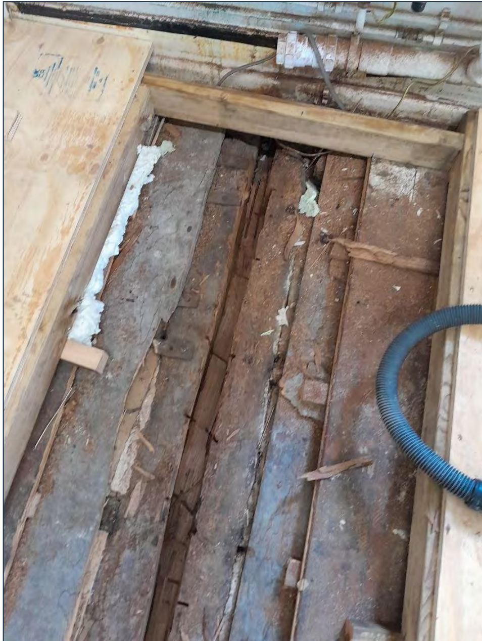
Photo 11 View of the one of the beams with central valley ready to receive the T steel section
