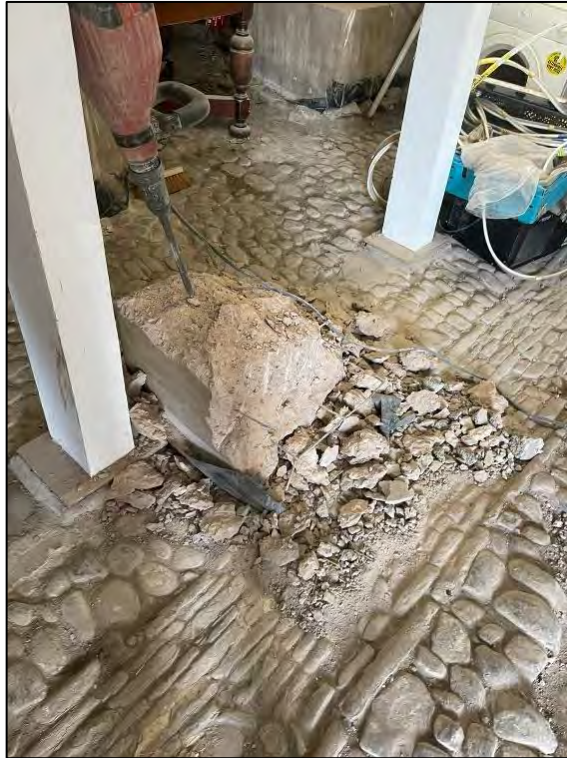
Photo 17 Part way through removal of the concrete pad
