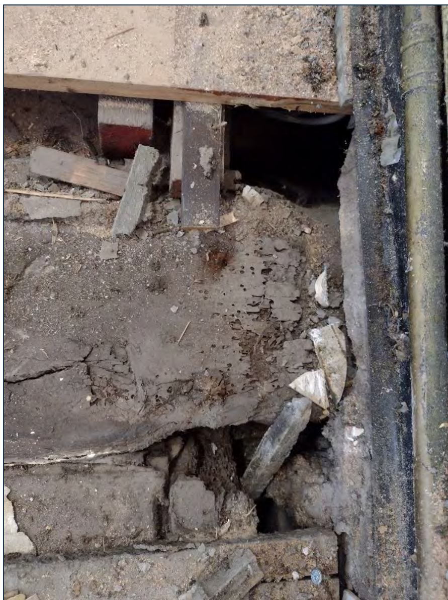
Photo 10 Image of the rotted southern beam end of the western beam at the bearing of the wall plate
