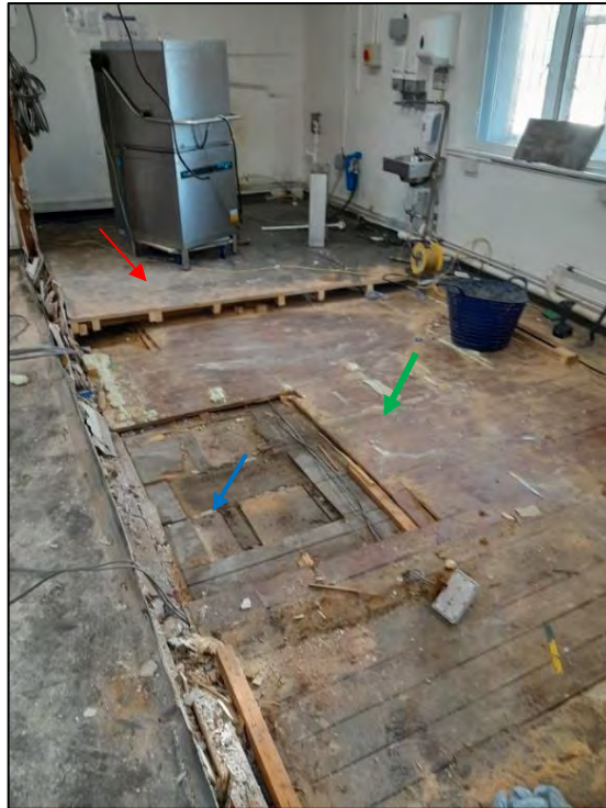
Photo 4 The floor surface during early uncovering (red arrow denotes plywood layer, green arrow the tongue and groove layer, and blue the wide oak boards)
