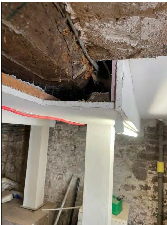
Photo 18 View of the chamfered western beam uncovered as part of the removal
