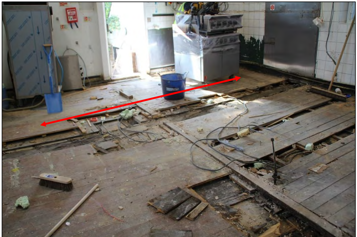
Photo 5 Following removal of the plywood layer and showing the pine tongue and groove layer with areas of removal to reveal the two beams (arrowed)
