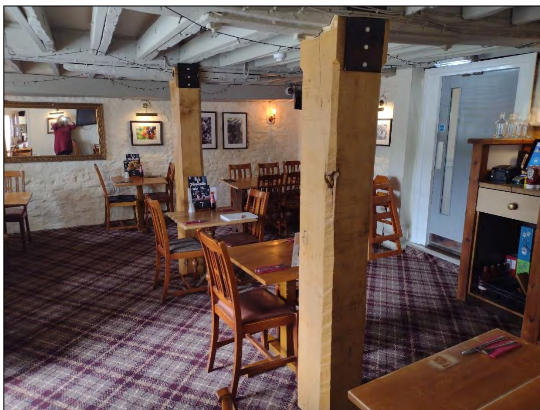
Photo 2 The ground floor restaurant with unauthorised piers
