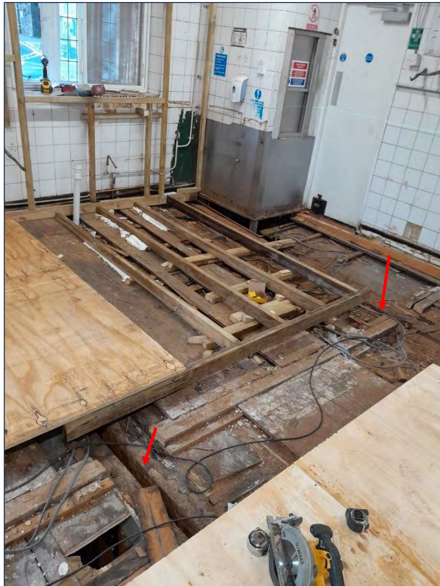
Photo 12 Both beams ready to receive the T steel section
