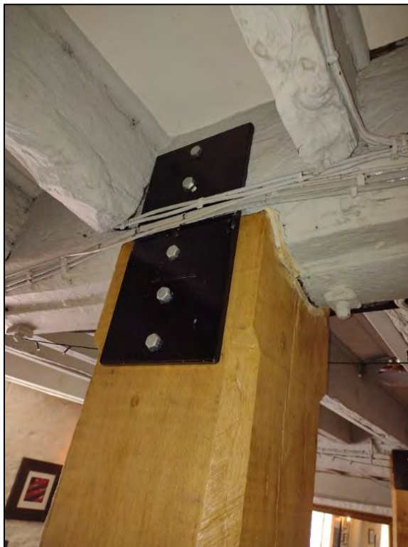
Photo 15 The interface of the to-be-removed pier and steel plate to the underside of the eastern primary beam on the ground floor
