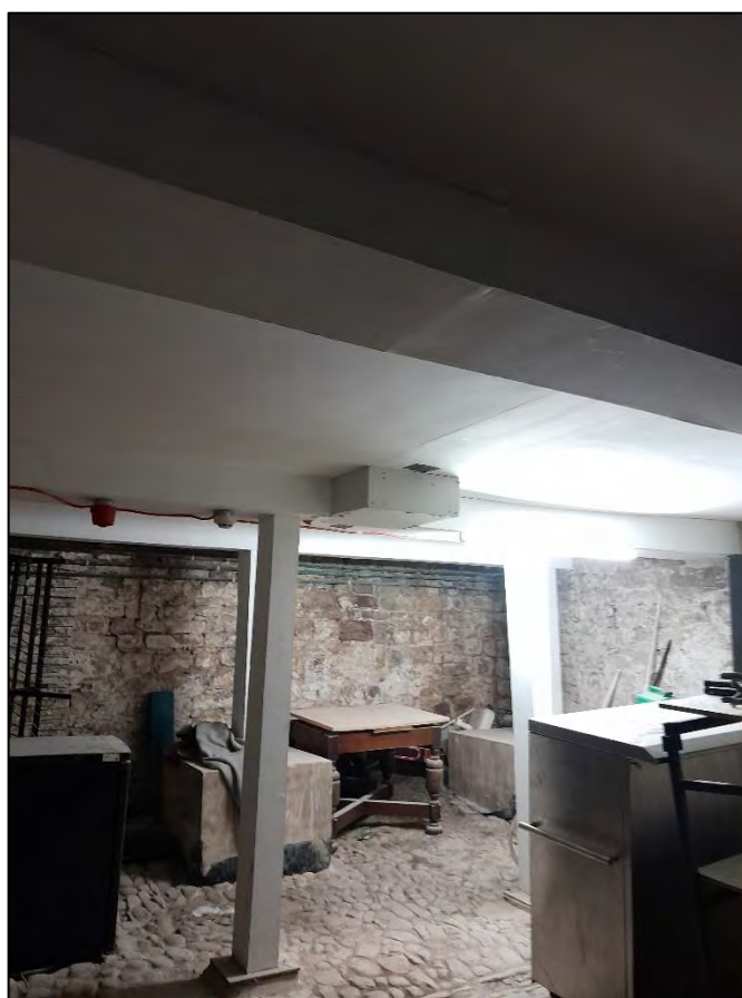
Photo 21 The basement level with piers removed
