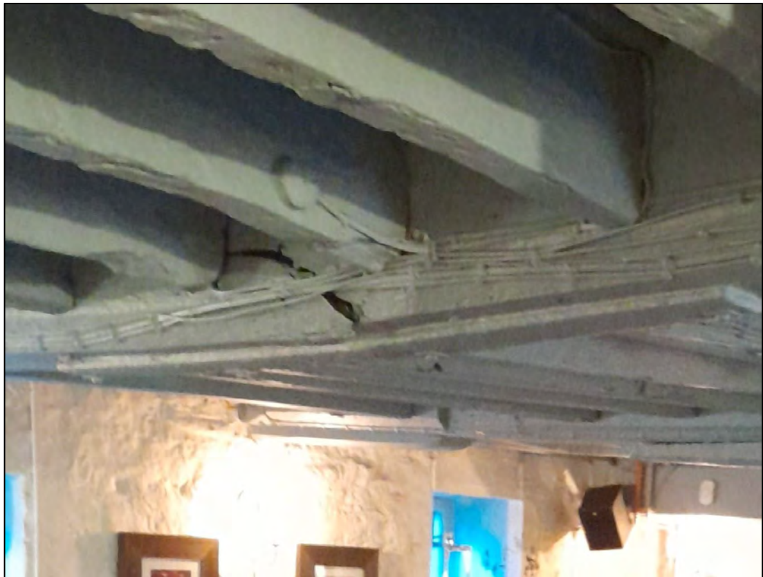
Photo 16 The eastern side of the beam with eastern pier removed
