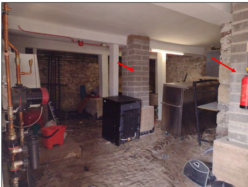
Photo 3 The unauthorised piers in the basement (arrowed)
