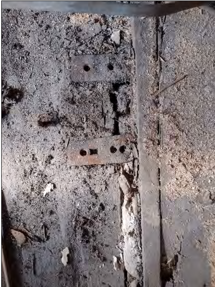
Photo 8 Evidence of previous structural additions, possibly joist brackets
