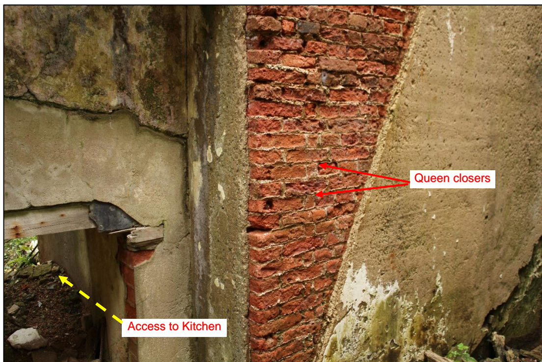
Photo 105: Detail of queen closer bricks at east extent of recessed opening within the north wall of West Stair Hall, ground floor of Cell F
