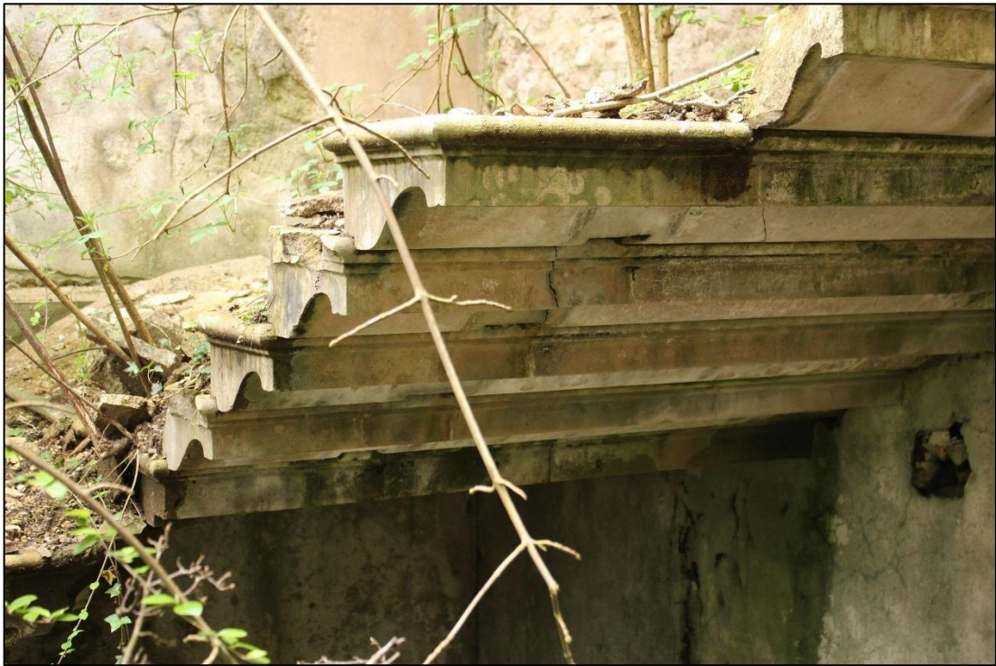
Photo 66: Detail of cantilever stair treads, west wall of Cell B
