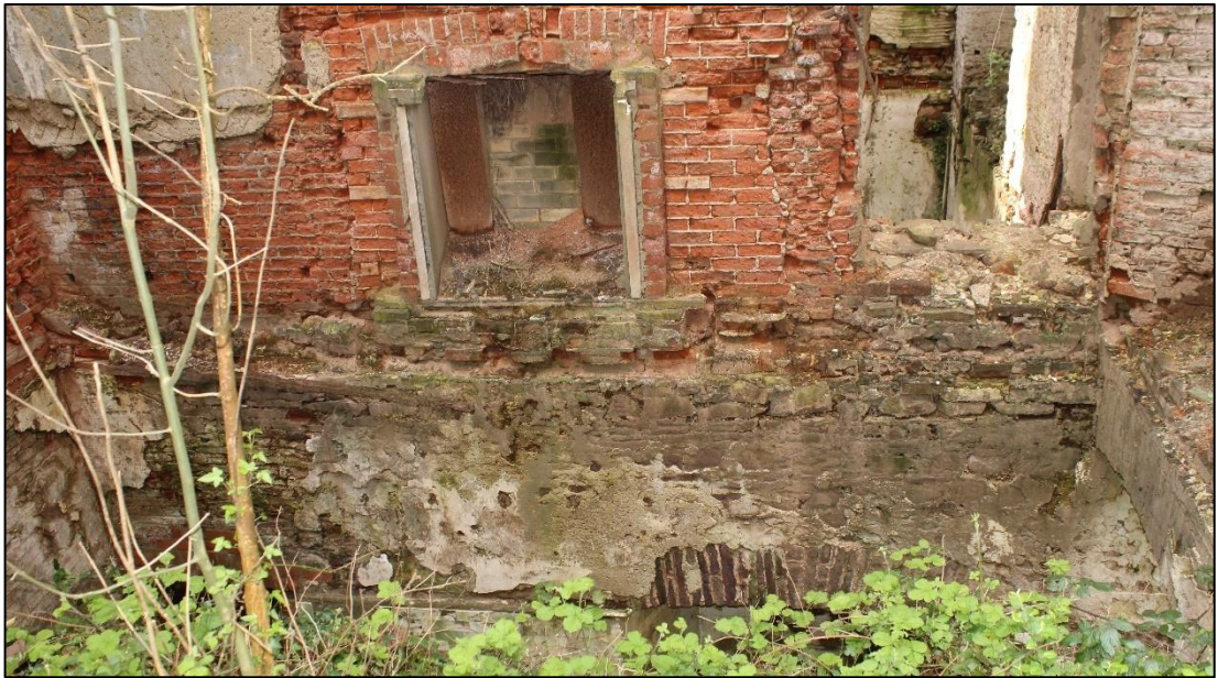
Photo 82: Collapsed floor at western extent of Smoking Room
