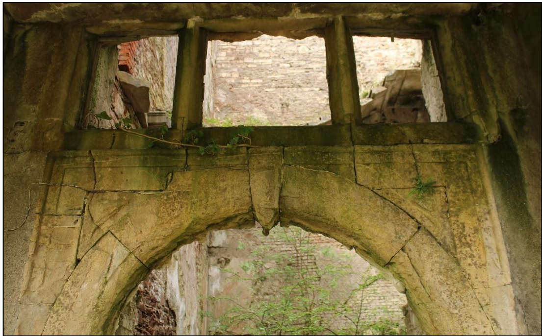
Photo 26: Detail of upper portion of early 17th-century door surround in east elevation, within the early 20th-century porch
