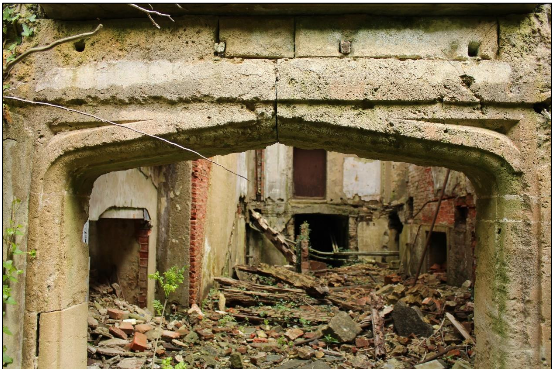
Photo 113: Detail of four-centred door head of original west entrance to the building
