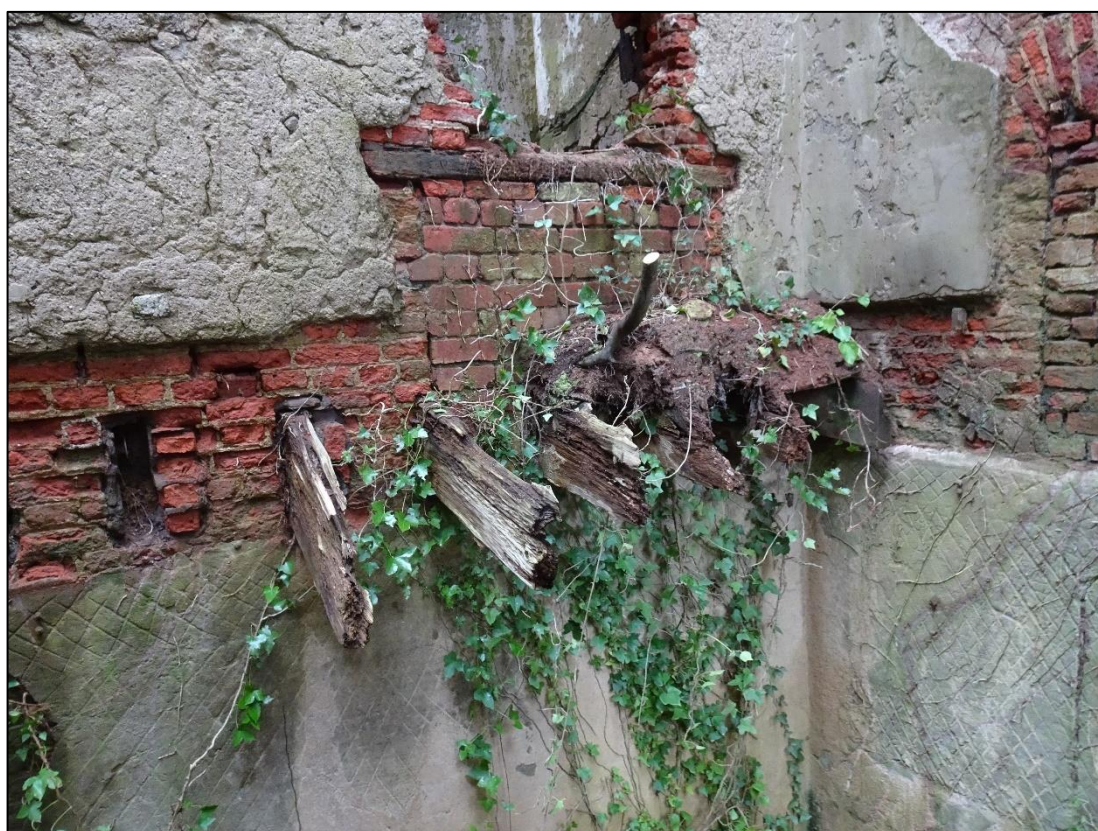
Photo 121: Infilled doorway at halfway landing height within north wall of Butler's Pantry
