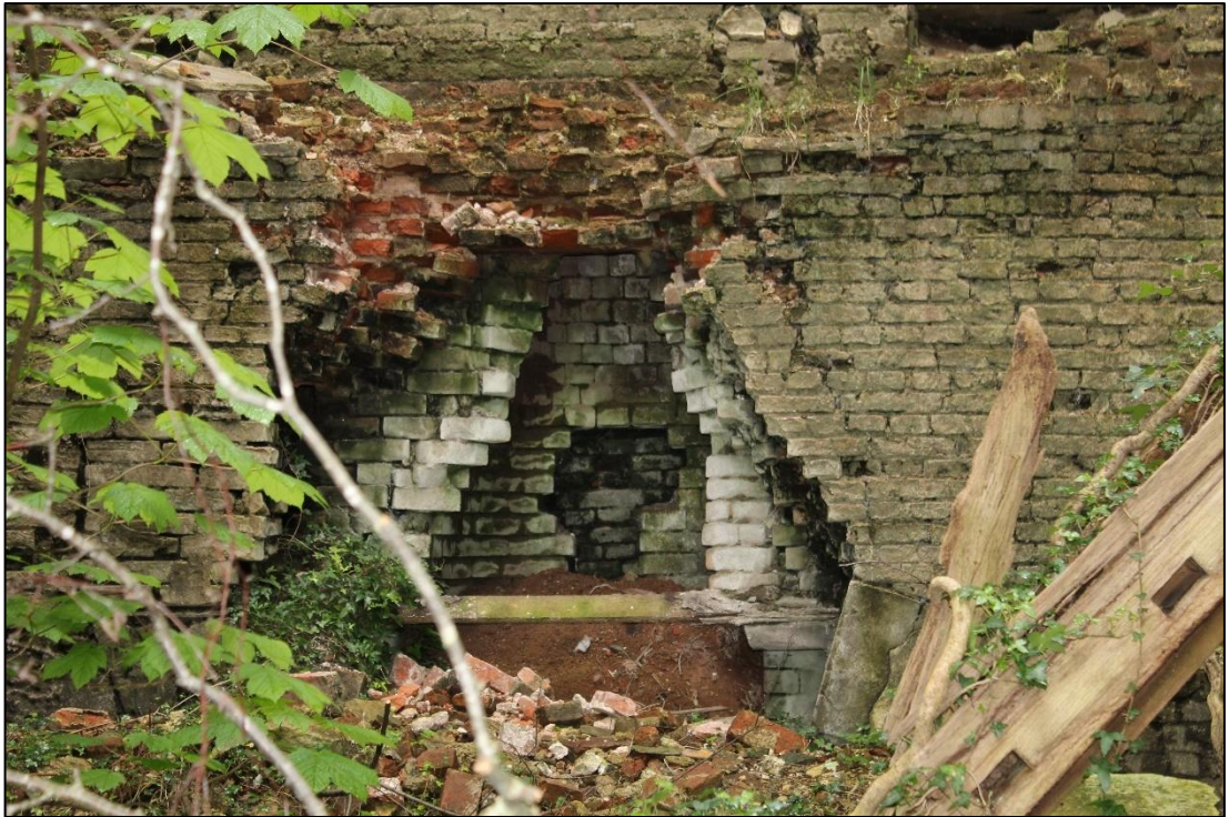
Photo 87: Detail of collapsed brickwork above fireplace in Scullery, south wall
