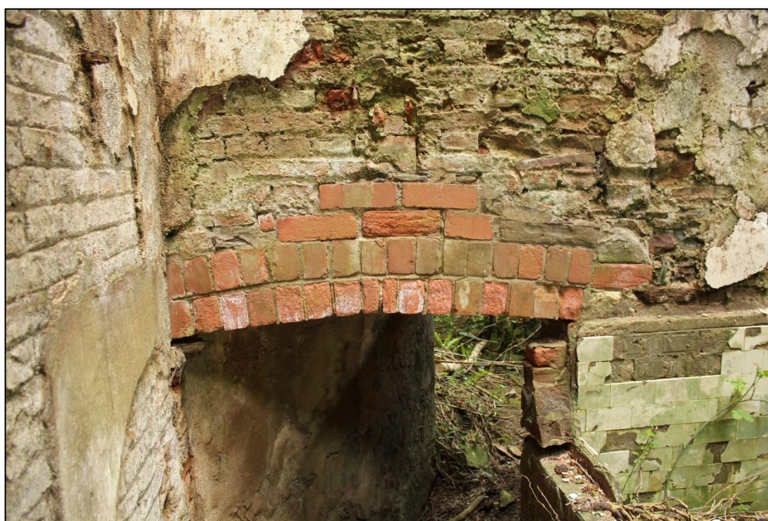
Photo 84: Detail of early 20th-century brick segmental head above passageway door
