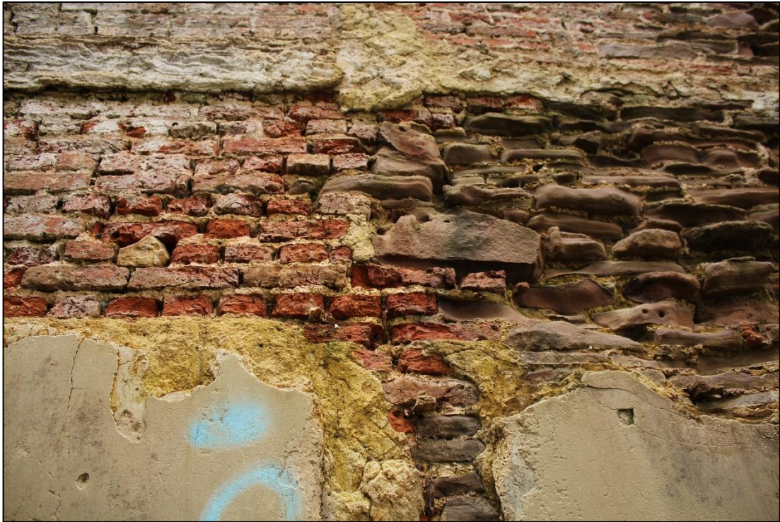
Photo 43: Detail of brickwork and rubblestone within north wall of Dining Hall
