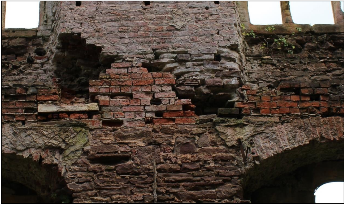
Photo 50: Detail of red brick repairs within the south wall of Cell A
