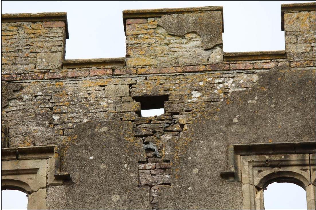
Photo 21: Detail of exposed masonry at parapet level
