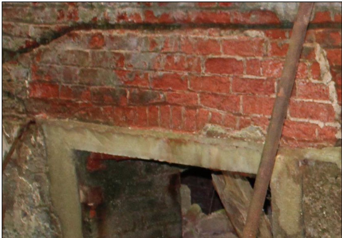
Photo 107: Detail of altered brickwork above central doorway of south wall of West Stair Hall
