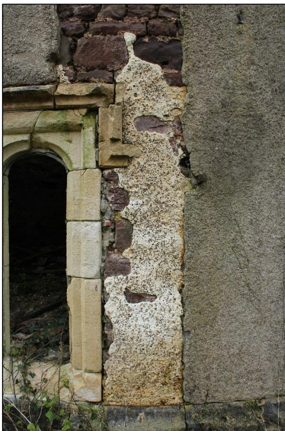
Photo 29: Evidence of patch repair following removal of wall, north-east tower
