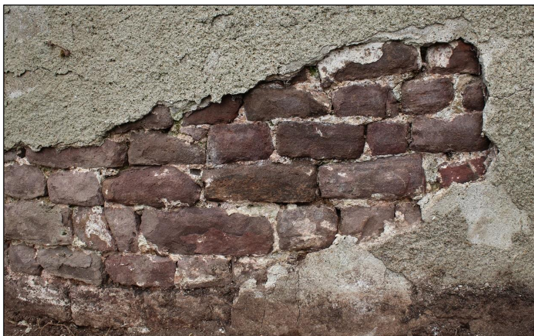
Photo 3: Exposed course of old red sandstone, south-west tower
