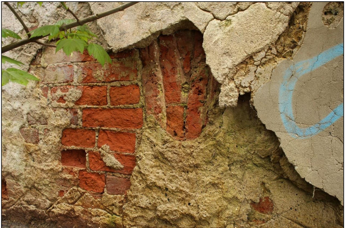
Photo 42: Detail of plasterwork and brick construction above fireplace in Dining Hall
