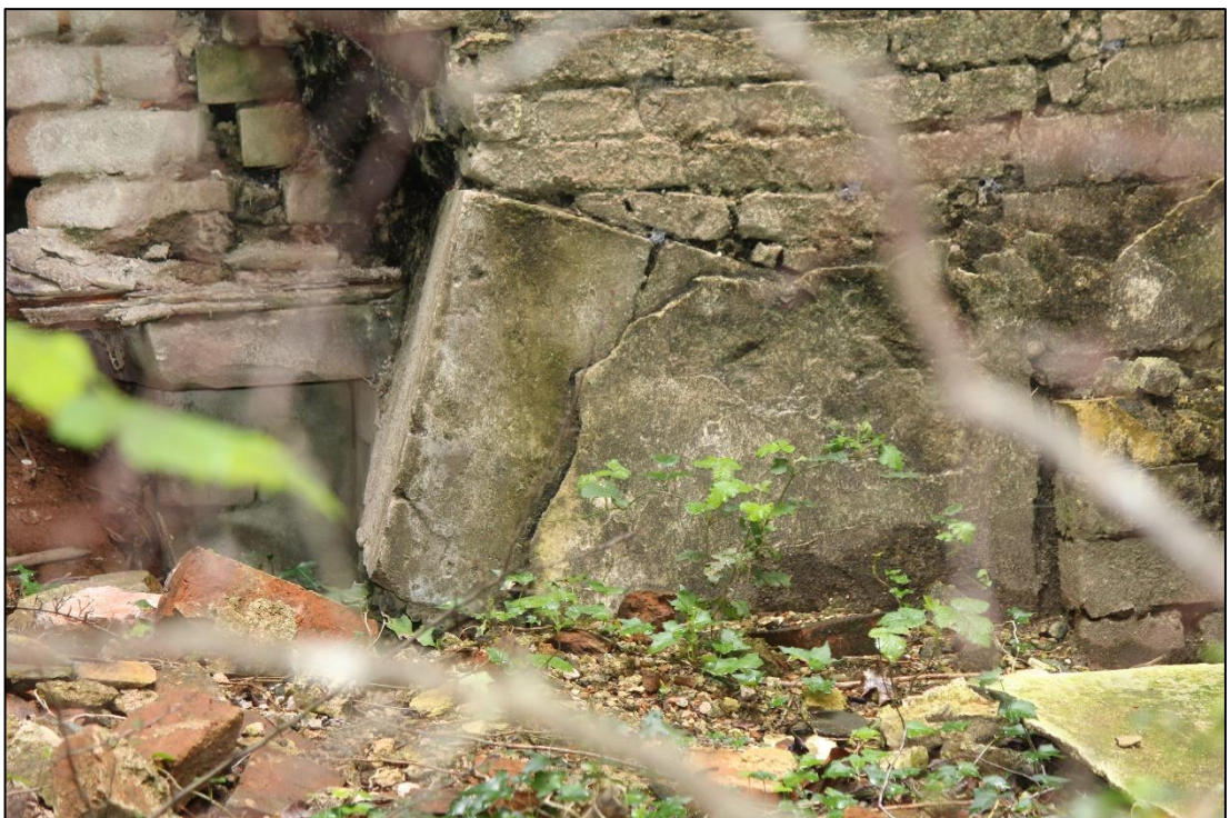
Photo 88: Detail of ashlar voussoir remains forming head of fireplace in Scullery, south wall
