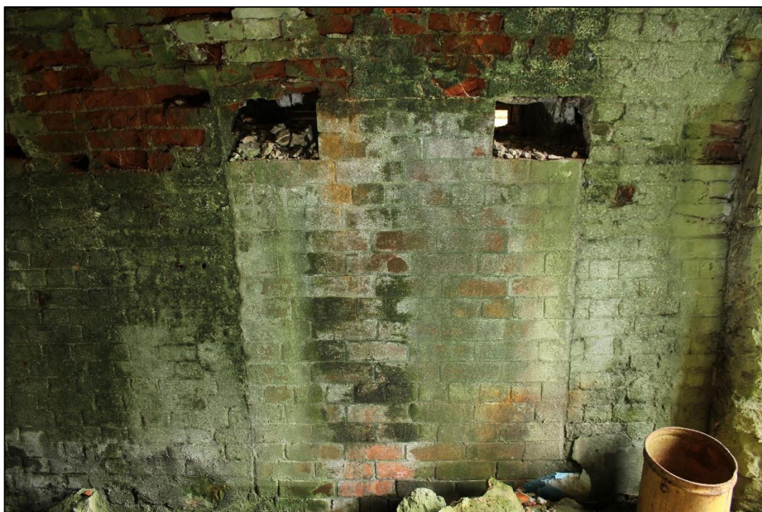
Photo 139: Infilled doorway between West and East Larders
