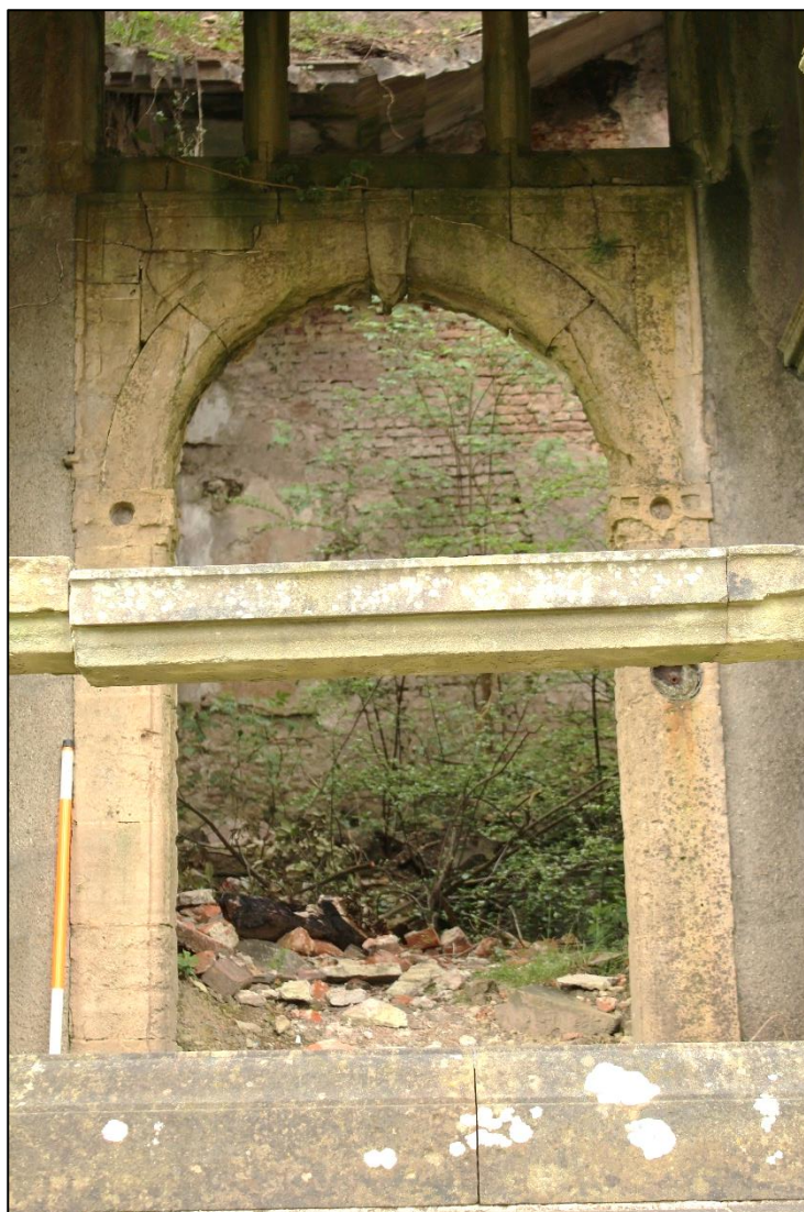
Photo 25: Detail of early 17th-century door surround in east elevation, within the early 20th-century porch
