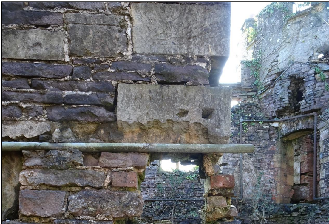
Photo 112: Detail of ashlar quoins at third floor level, south wall of Cell F
