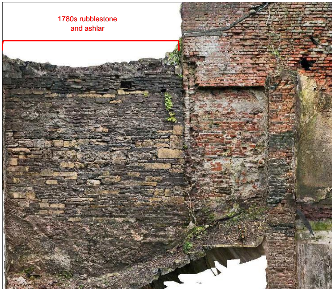
Fig. 49: Detail of rubblestone and brickwork within west wall of Cell B, third floor
