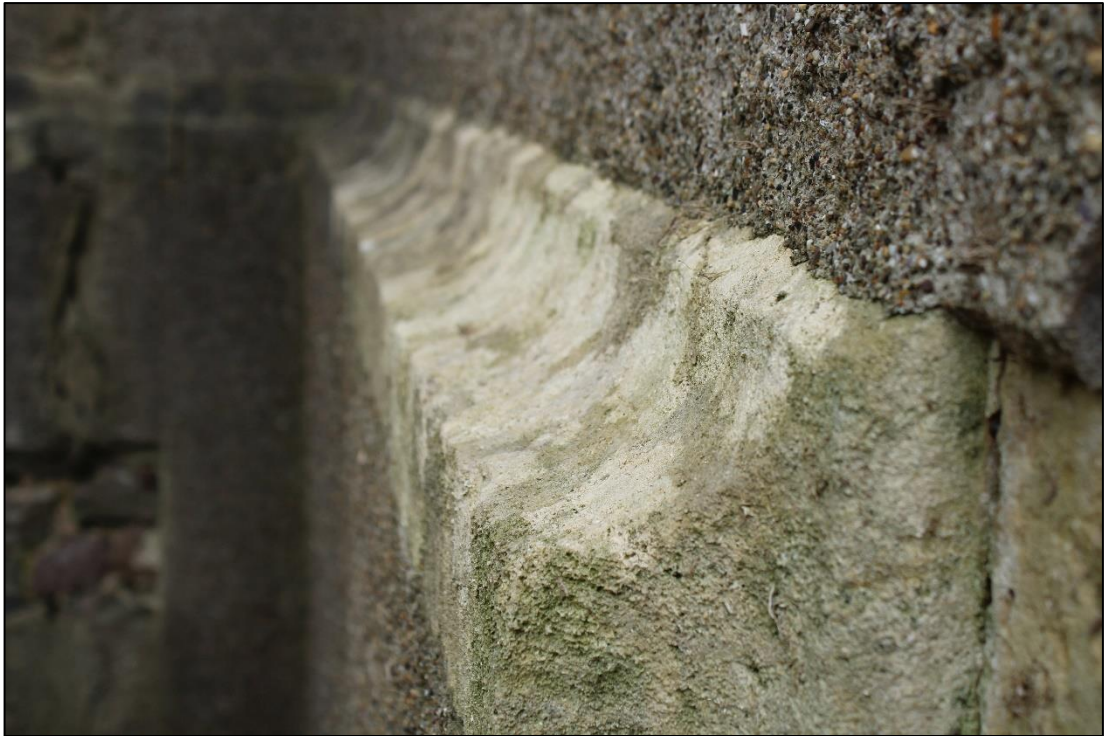
Photo 7: Detail of cavetto moulding atop plinth, porch on south elevation
