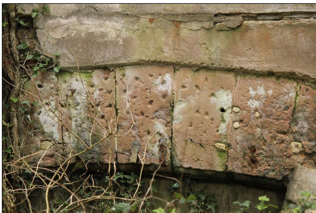
Photo 97: Detail of stone voussoirs above Kitchen hearth
