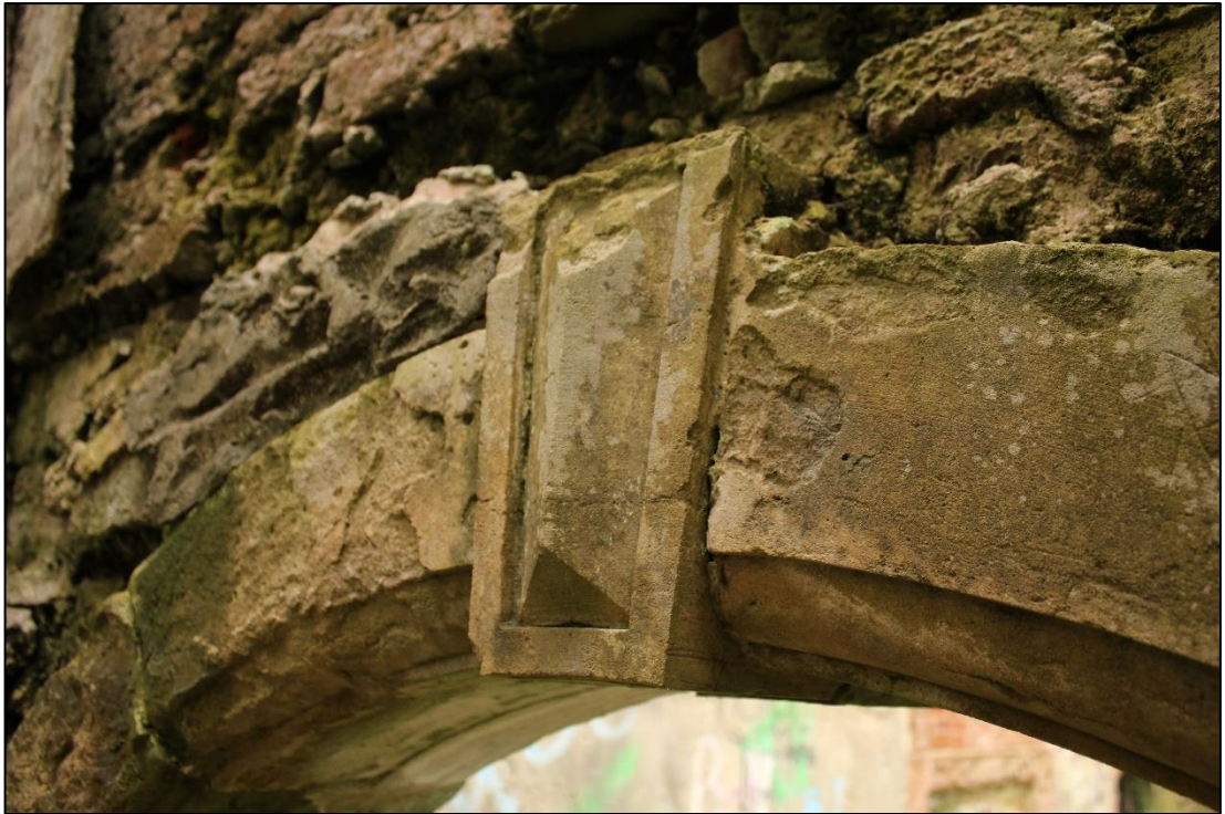
Photo 53: Keystone on reverse of door at west extent of south wall of Cell A
