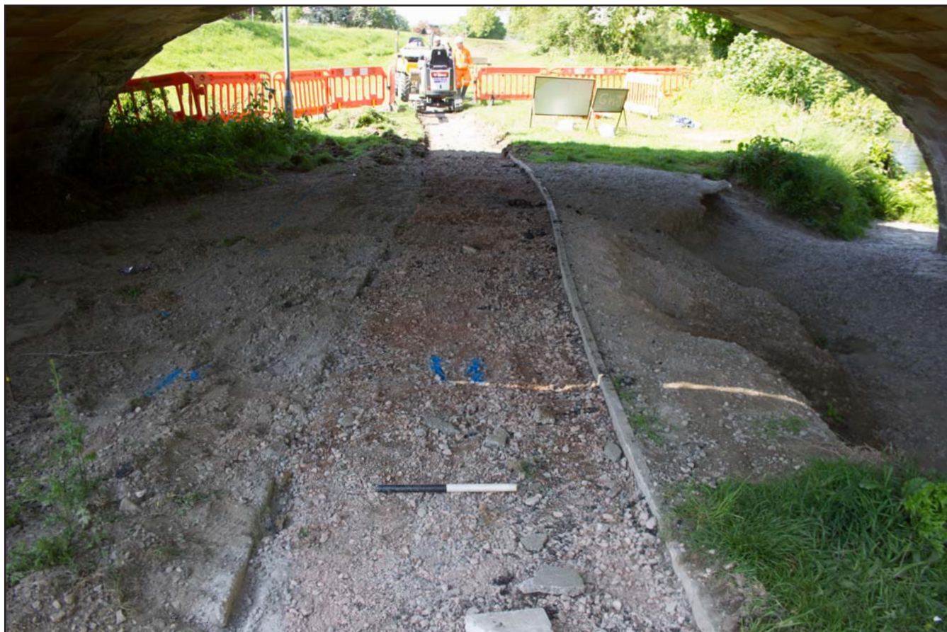
Plate 07: Removal of existing pathway, from the south. Scale 0.5m.
