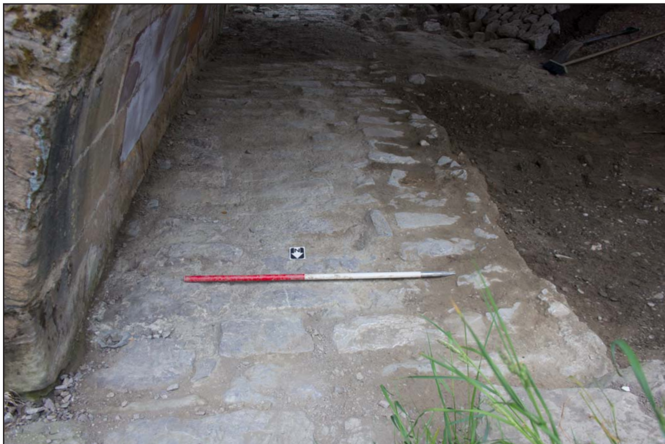
Plate 29: Removal of remaining silt exposing bridge plinth (102), from the north. Scale 1.0m.
