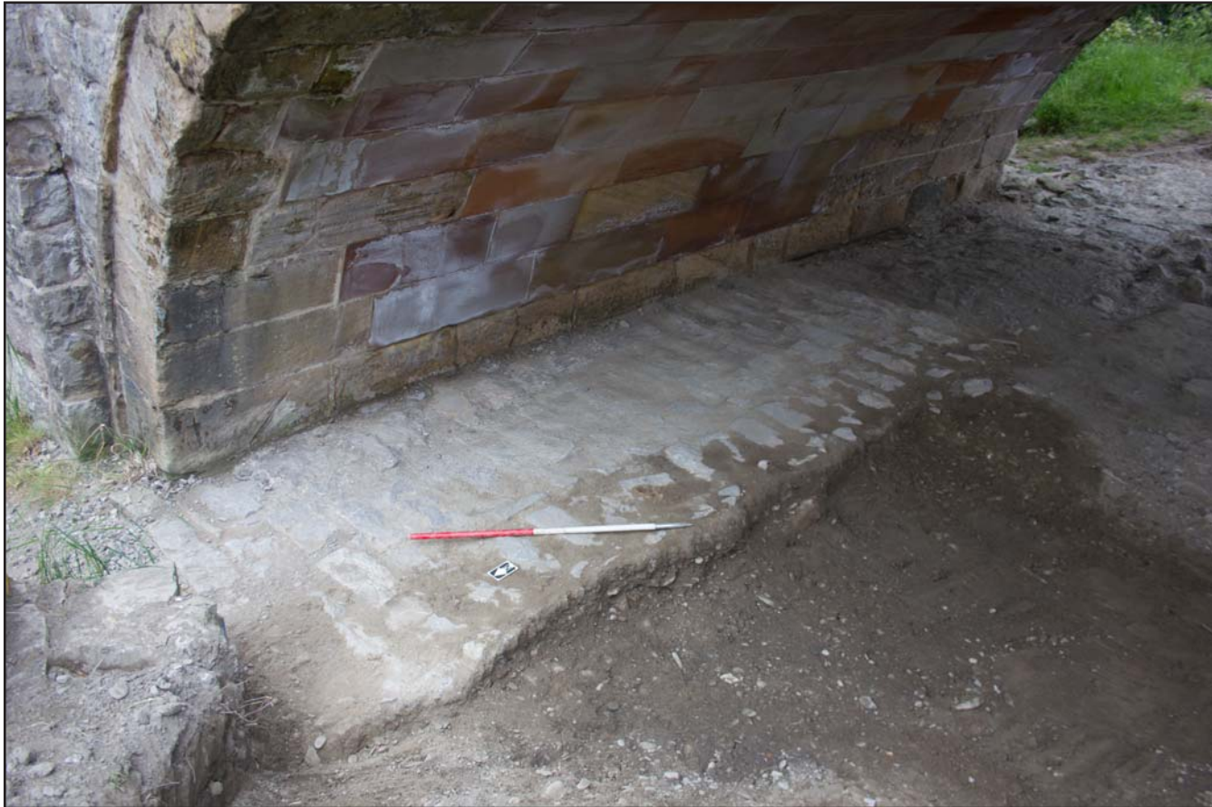
Plate 30: Removal of remaining silt exposing bridge plinth (102), from the northwest. Scale 1.0m.
