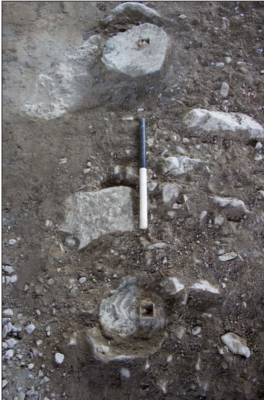
Plate 22: Iron railing bases inserted into pitching stones (101), from the north. Scale 0.5m.
