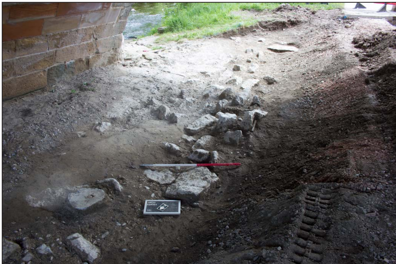
Plate 16: Removal of loose mid/light grey silt revealing pitching stones (101), from the northwest. Scale 1.0m.
