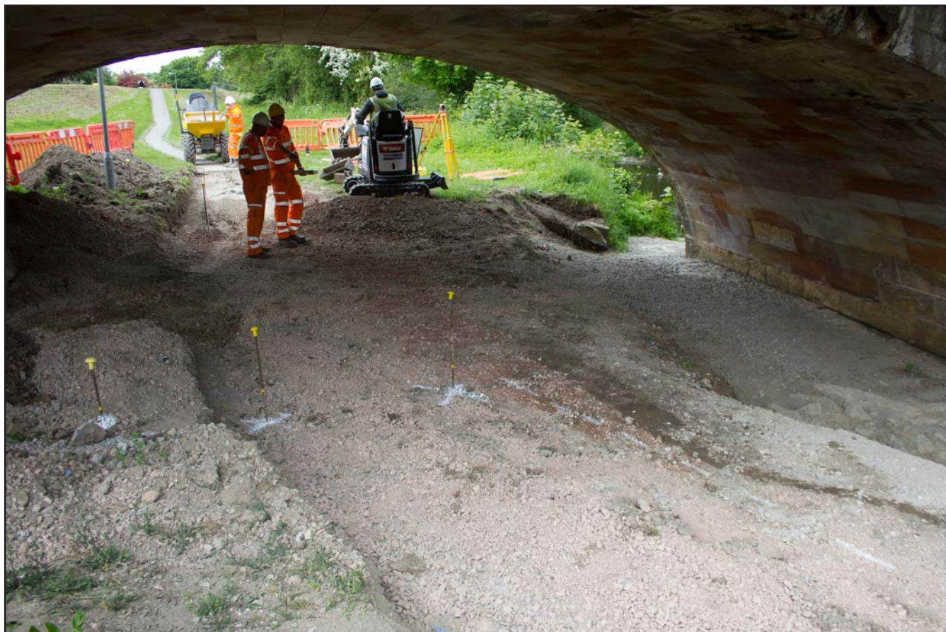
Plate 09: Removal of existing sub-base to east of pathway, from the southwest.
