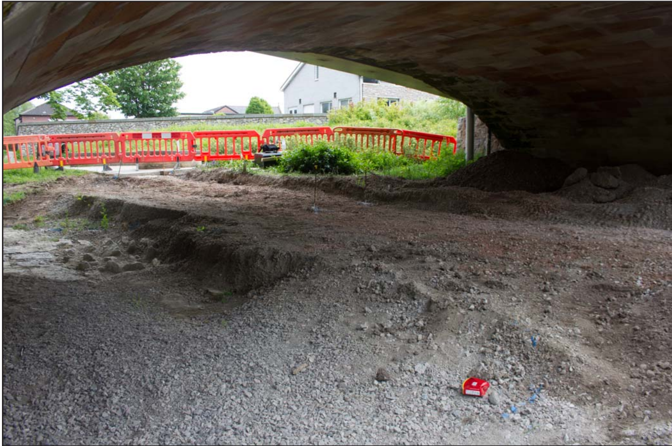
Plate 10: Removal of existing sub-base to east of pathway, from the northwest.
