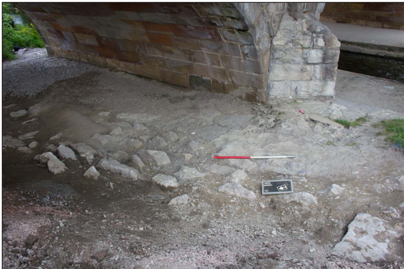
Plate 14: Removal of loose mid/light grey silt revealing pitching stones (101), from the southwest. Scale 1.0m.
