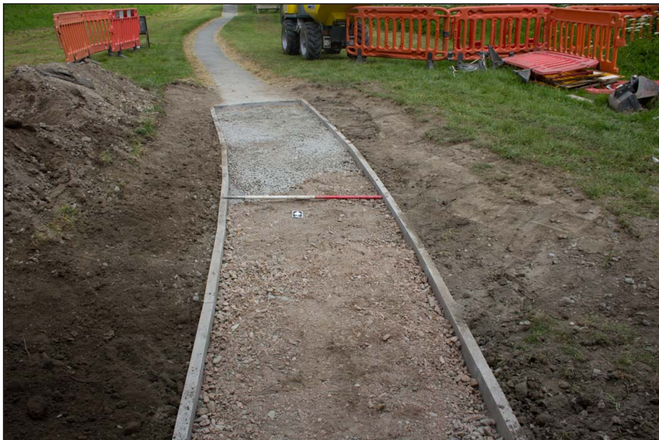
Plate 33: Reduction of bank either side of new pathway to the north of the bridge, from the south. Scale 1.0m.
