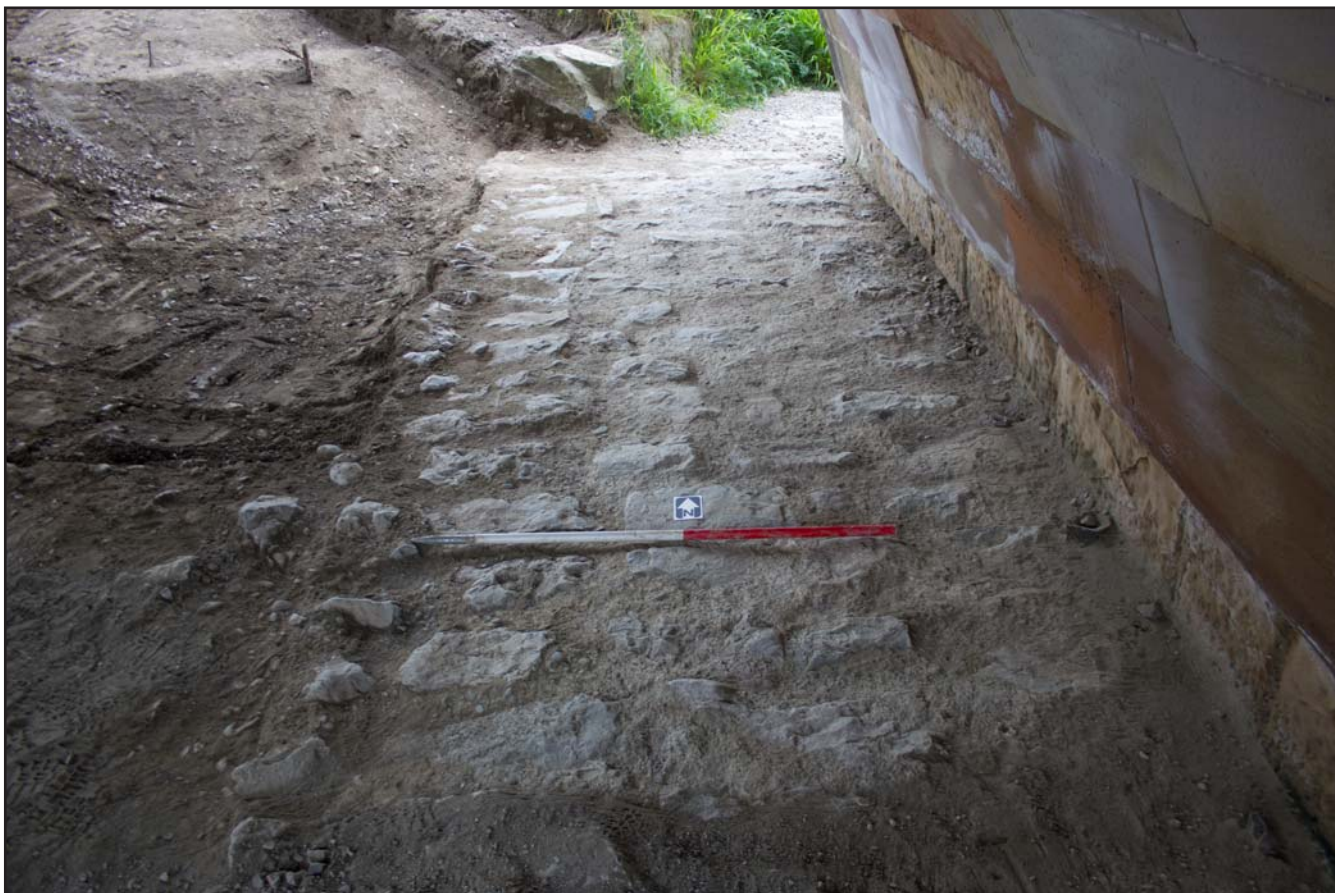
Plate 28: Removal of remaining silt exposing bridge plinth (102), from the south. Scale 1.0m.
