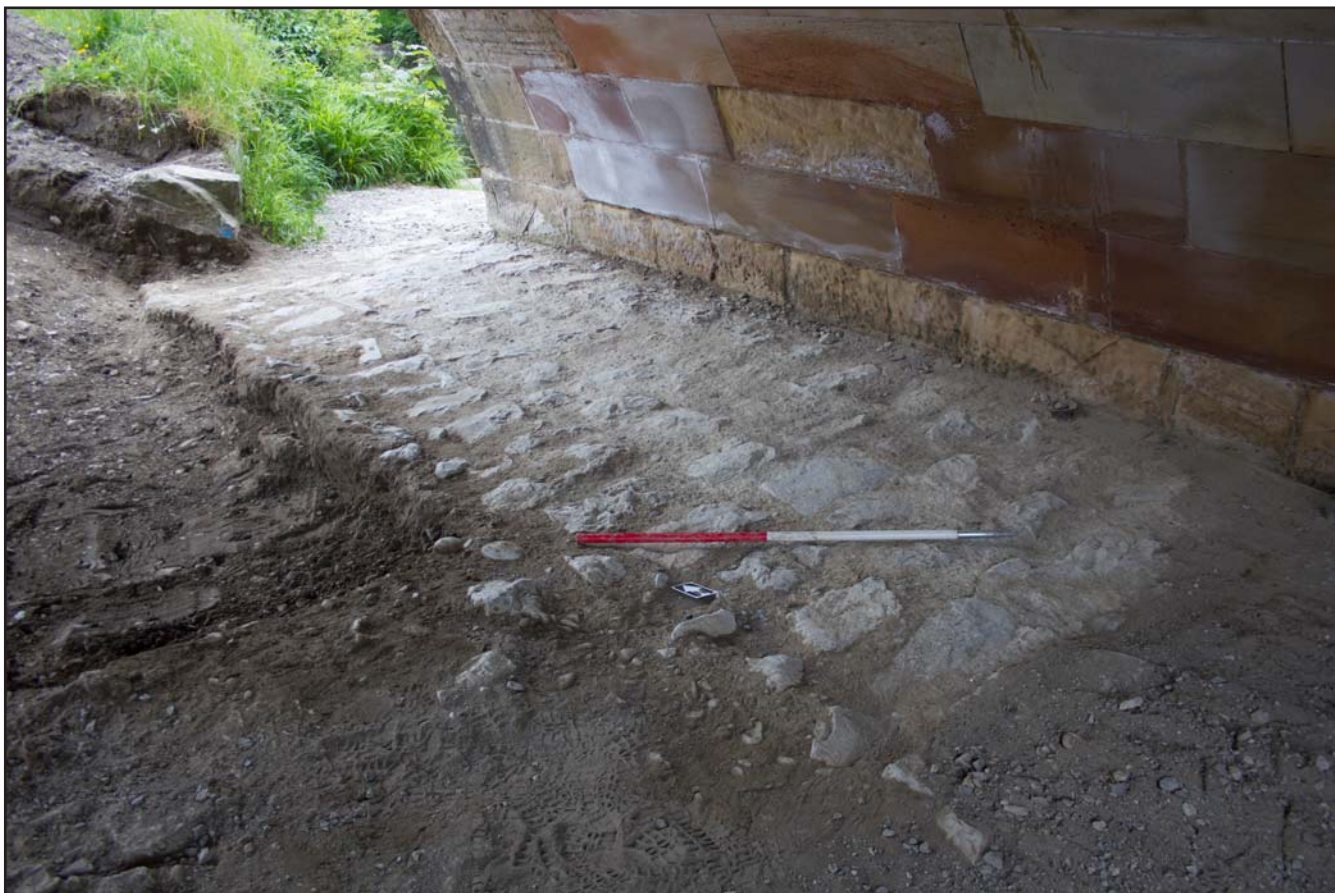
Plate 32: Removal of remaining silt exposing bridge plinth (102), from the southwest. Scale 1.0m.
