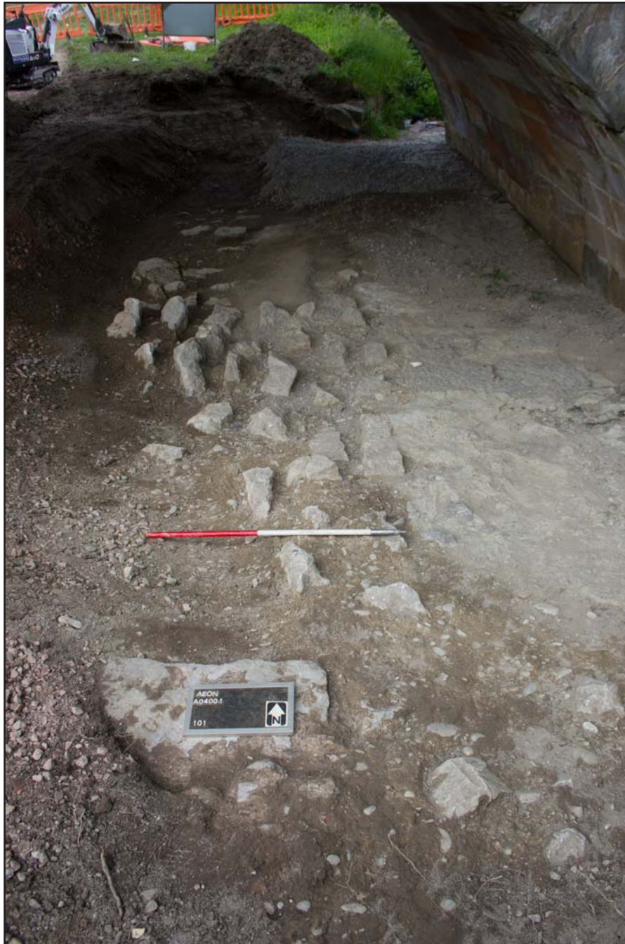
Plate 12: Removal of loose mid/light grey silt revealing pitching stones (101), from the south. Scale 1.0m.
