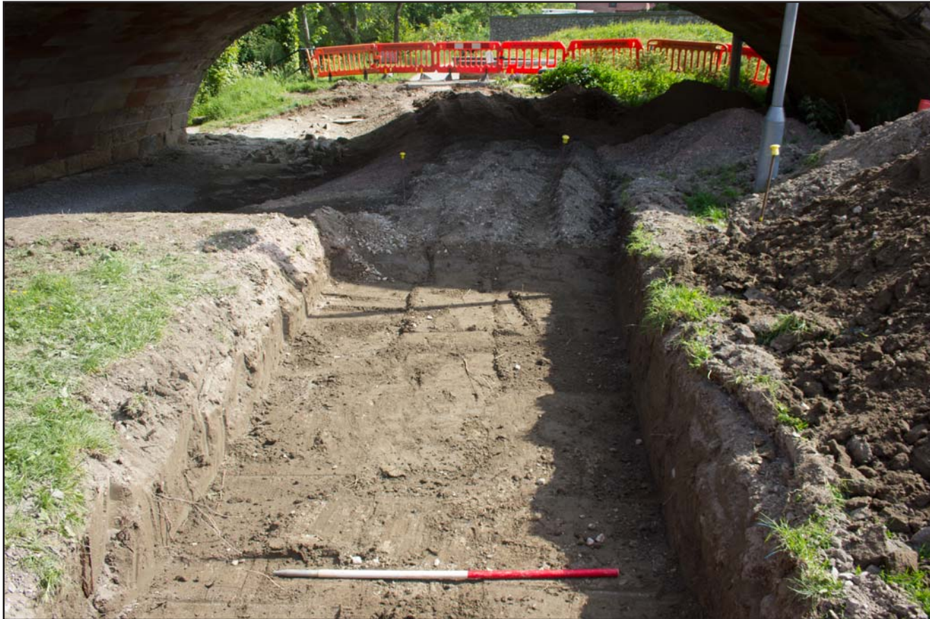
Plate 27: Removal of existing trackway and excavation of undelying sub-base and subsoil to the north of the bridge arch, from the north. Scale 1.0m.
