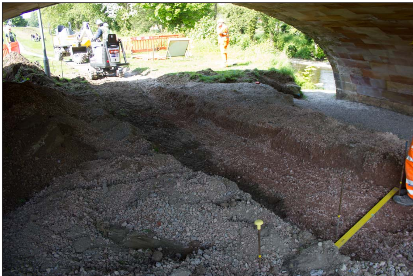
Plate 08: Removal of existing sub-base beneath pathway, from the southwest.
