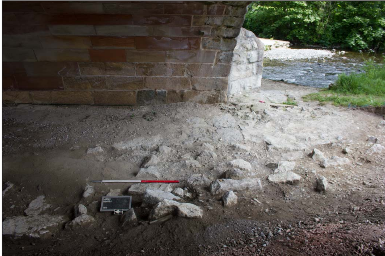
Plate 15: Removal of loose mid/light grey silt revealing pitching stones (101), from the west. Scale 1.0m.
