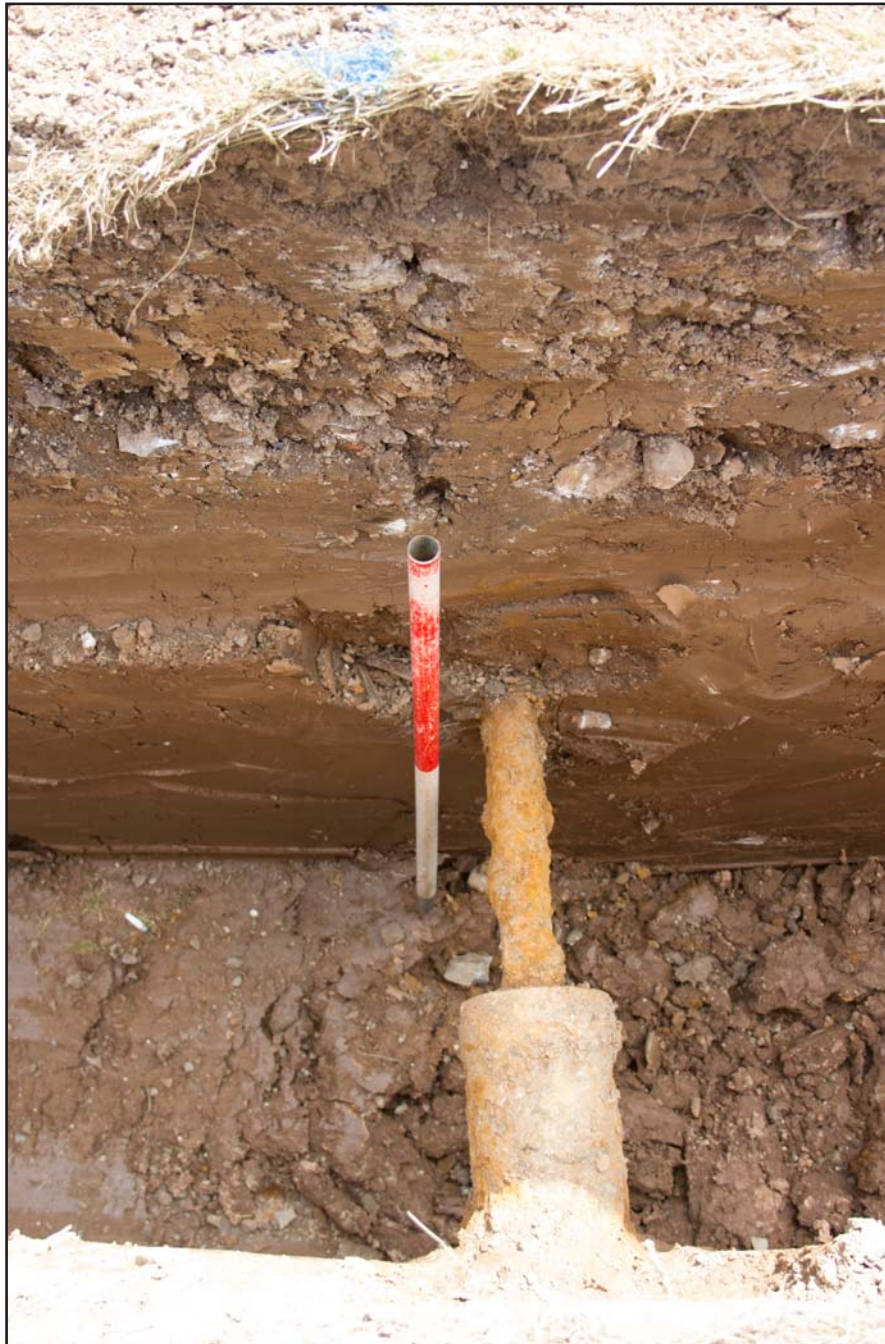
Plate 24: Cast iron drainage pipe running northwest - southeast toward former pond, Glascoed to Bodelwyddan DCWW - from the south-southeast - 1.00m scale
