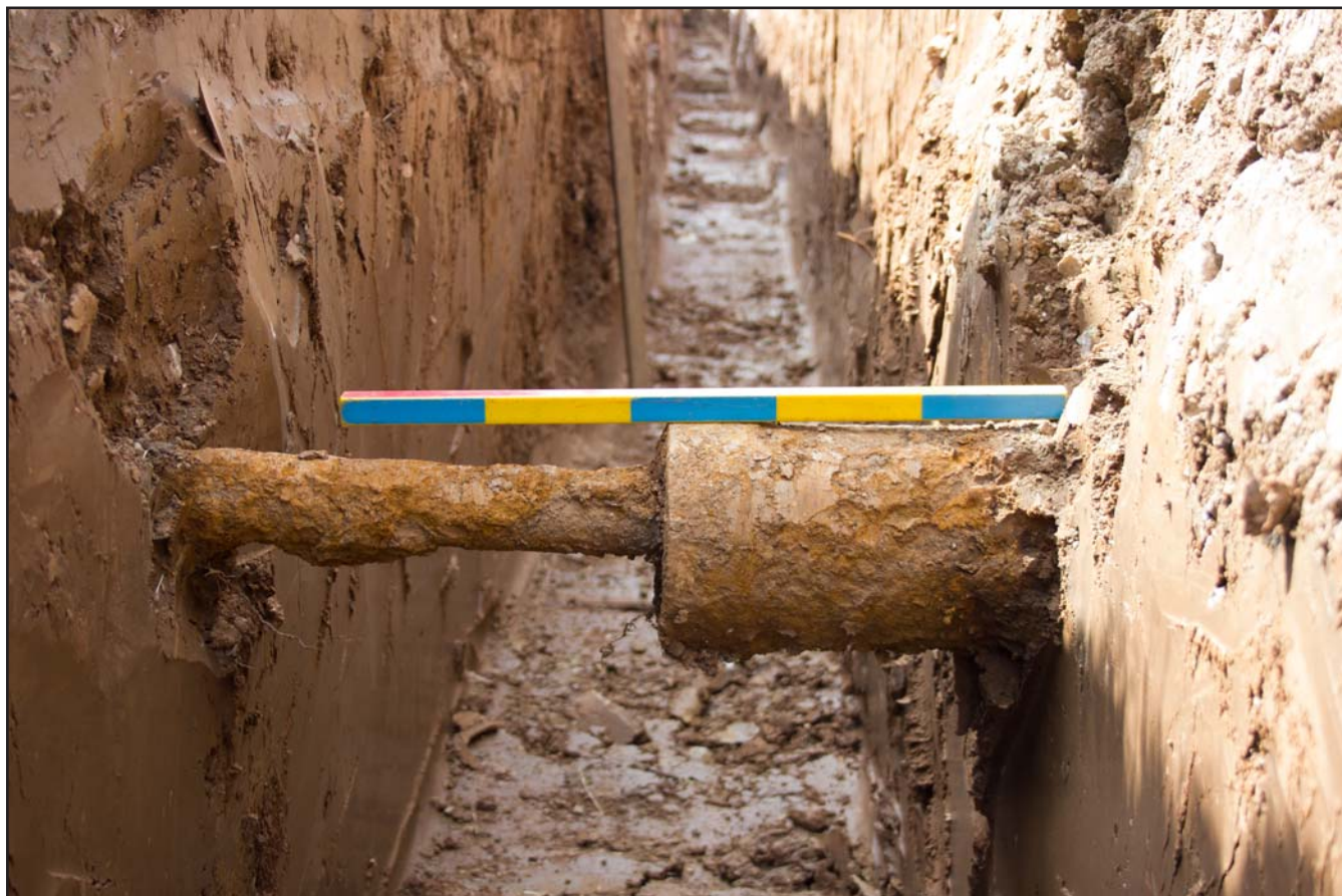
Plate 25: Cast iron drainage pipe running northwest - southeast toward former pond, Glascoed to Bodelwyddan DCWW - from the south-southeast - 1.00m scale
