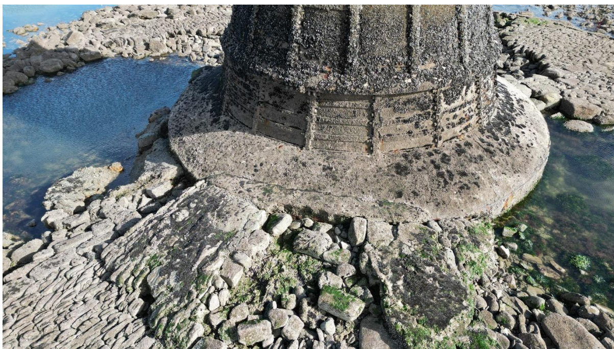
Figure 2.6: Surviving sections of the upper apron on the western side of Whitford Point Lighthouse, photographed on 17/10/2024 (© Crown Copyright: RCAHMW).
