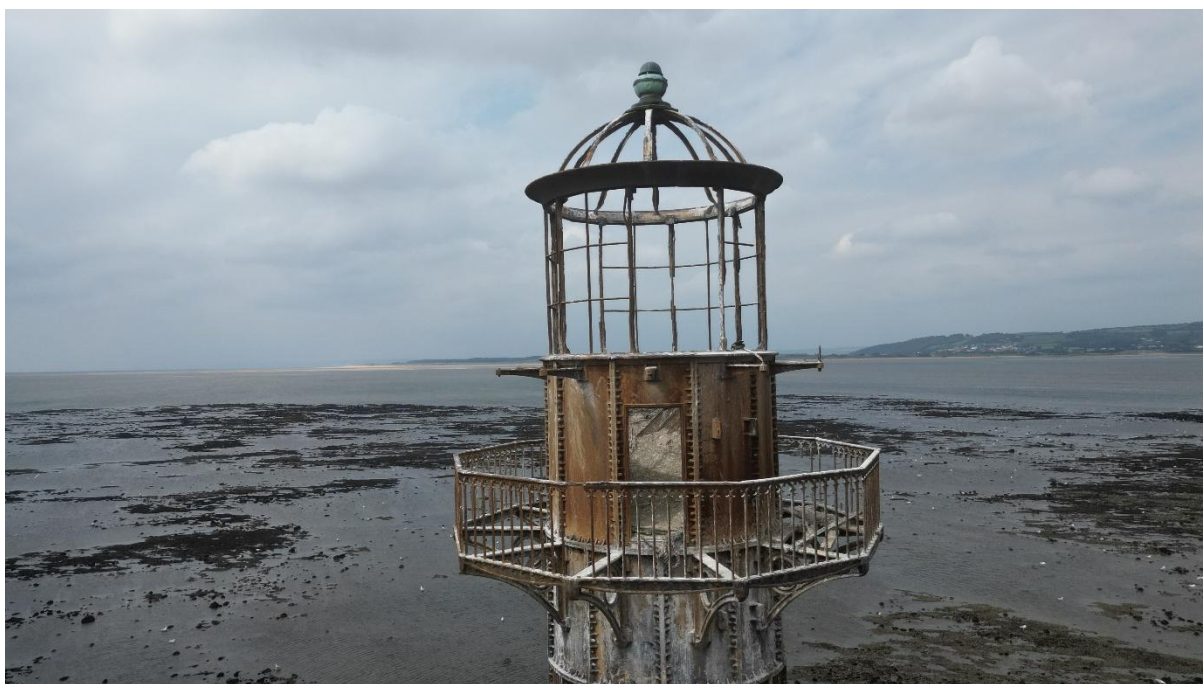
Figure 2.3: The upper sections of Whitford Point Lighthouse on 17/08/2024, including the living-room, lantern, dome and balustrades (© Crown Copyright: RCAHMW).
