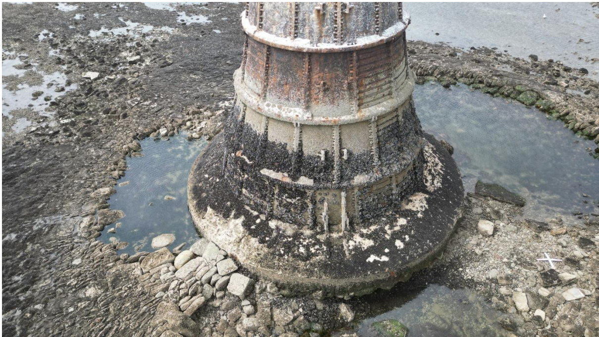
Figure 2.2: The lower cast-iron sections, collar and surrounding apron of Whitford Point Lighthouse on 17/08/2023 (© Crown Copyright: RCAHMMW).
