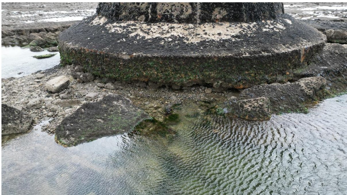
Figure 2.5: The collar surrounding the base of the lowest cast-iron ring of Whitford Point Lighthouse, photographed on the 17/08/2023 (© Crown Copyright: RCAHMMW).
