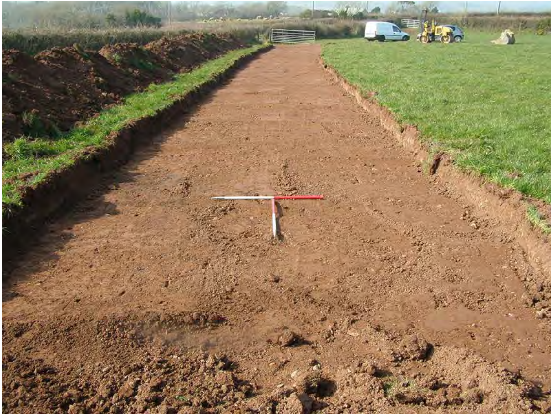
Photo 1: Initial topsoil strip of trackway, removing the upper 0.3m. Facing NNW, 1m scales.
