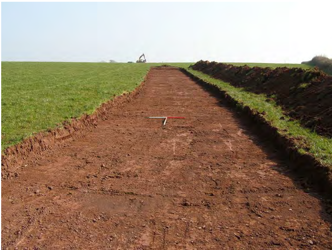
Photo 2: Initial topsoil strip of trackway, removing upper 0.3m. Facing SSE, 1m scales.
