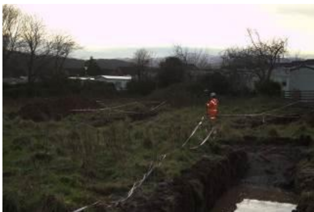
Working shot: Surveying of Site
