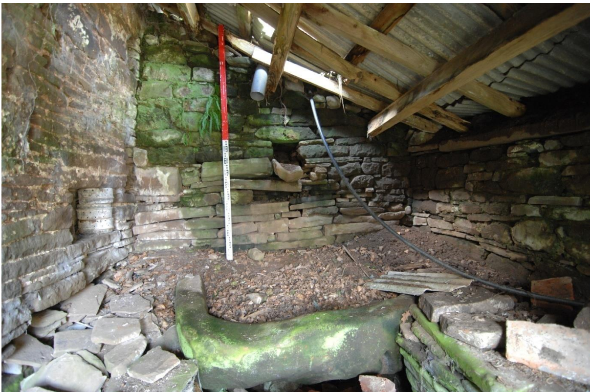
Pl.13: The interior of the Lean-to, showing the trough and water supply at the rear, or west, of the building where it is built into the bank.
