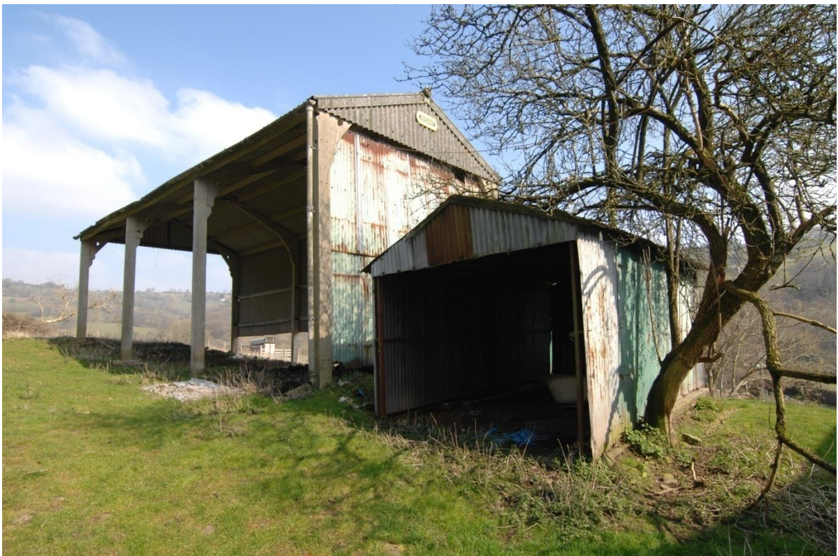
Pl.59: Modern concrete portal framed Dutch barn and slightly earlier sheeted garage to the north of the farmhouse.
