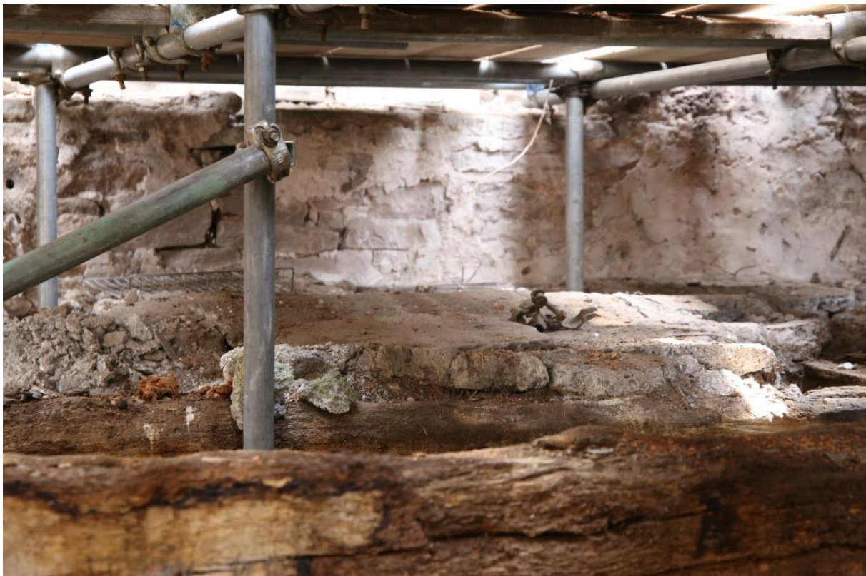
Pl.11a: Remnants of secondary thick plaster floor laid onto the loft floor boards of the Store, taken after initial clearance (courtesy of Sam Hale).
