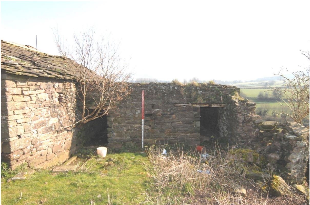
Pl.34: The north wall of the Piggery (Building H) showing the openings to the sties; the yard walls in front have largely been removed.
