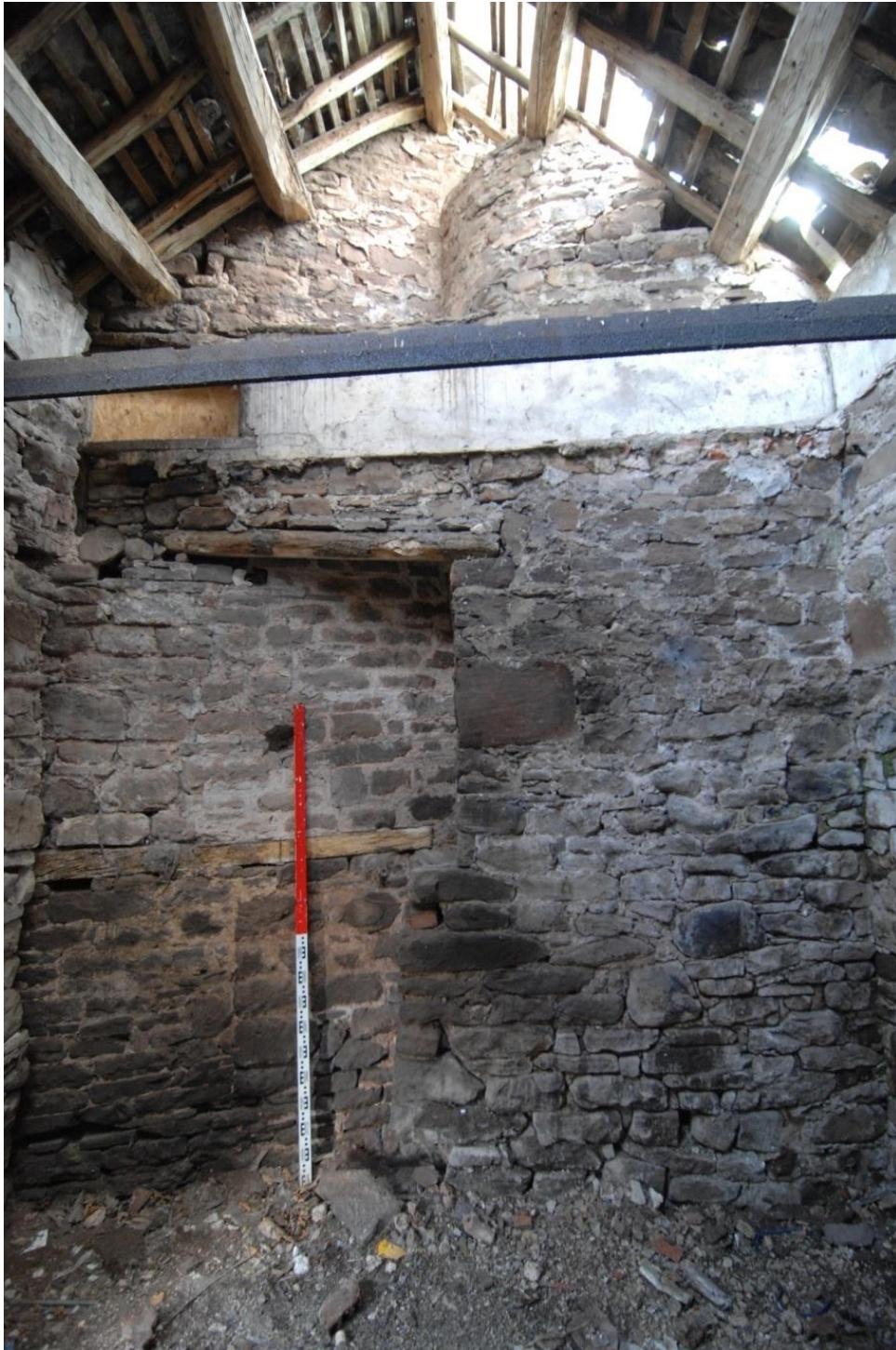
Pl.3: The interior of the Infill Range, looking south to the end gable of the Solar wing of the main house; note the blocked windows in the original building at both floor levels.
