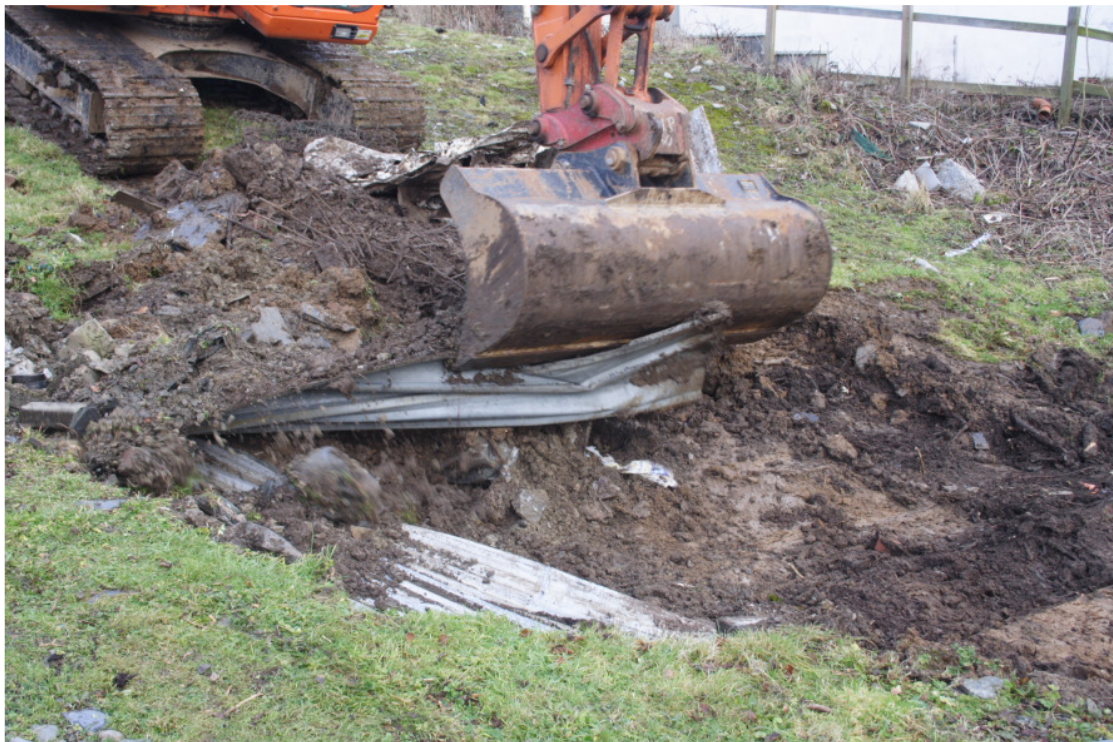
Photo 2: Photo showing removal of modern debris.
