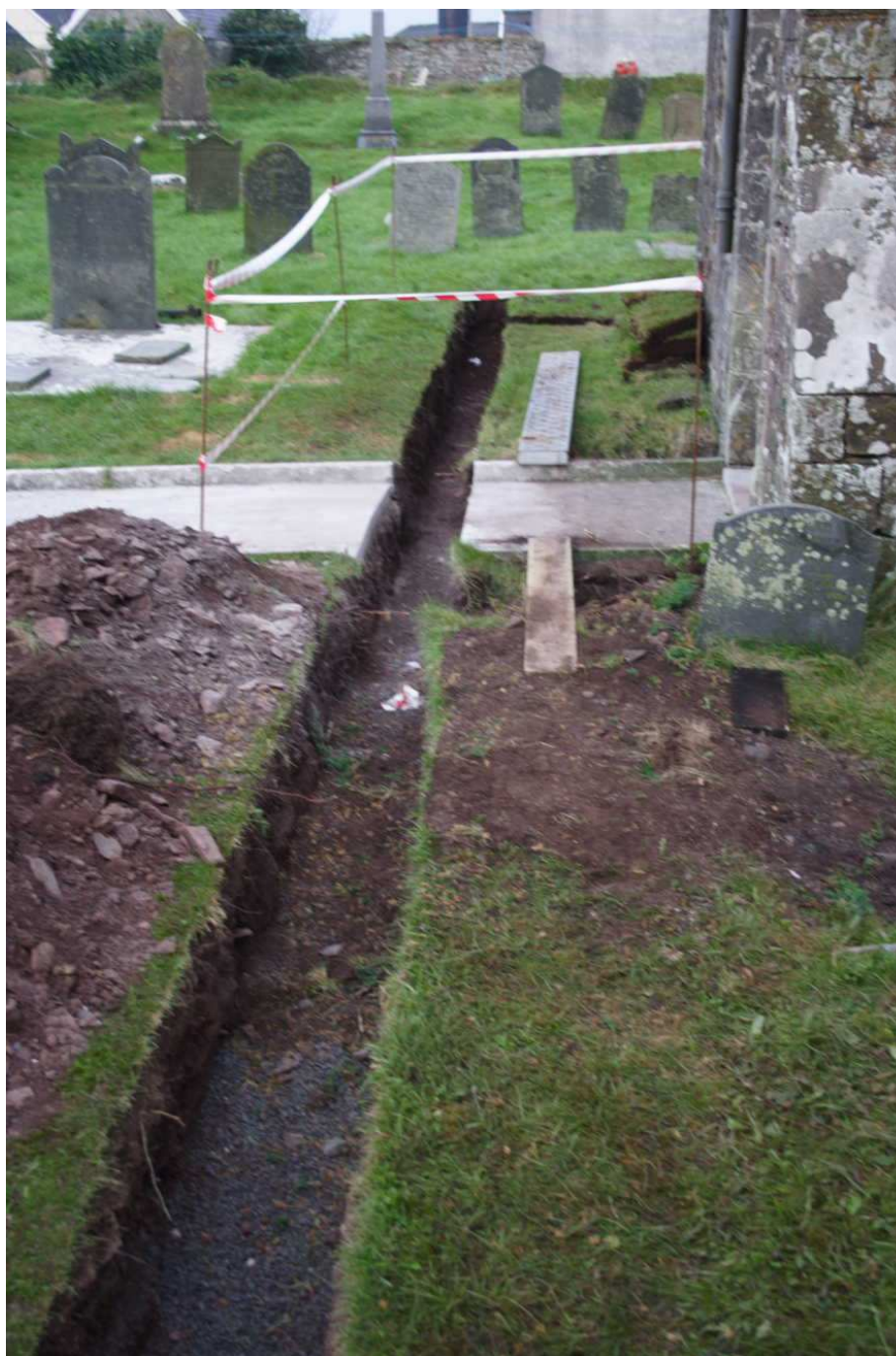
Photo. 1: West facing section of Drainage pipe cut.
