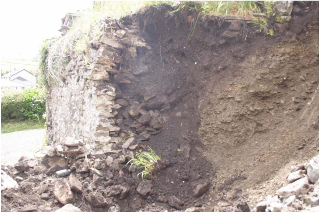
Plate 1: Section through retaining wall following demolition.
