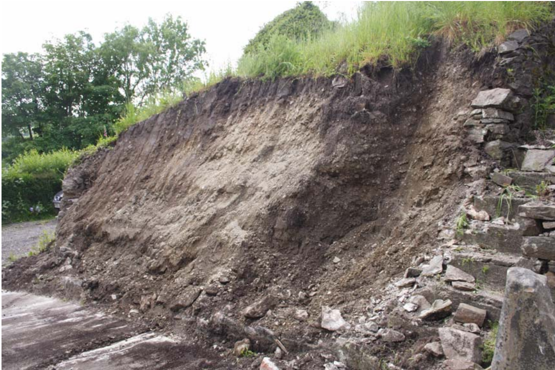
Plate 4: Section through garden following demolition of retaining wall.
