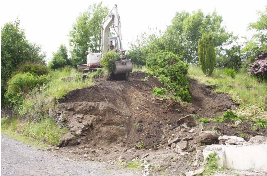
Plate 5: General working shot showing site stripping in progress.
