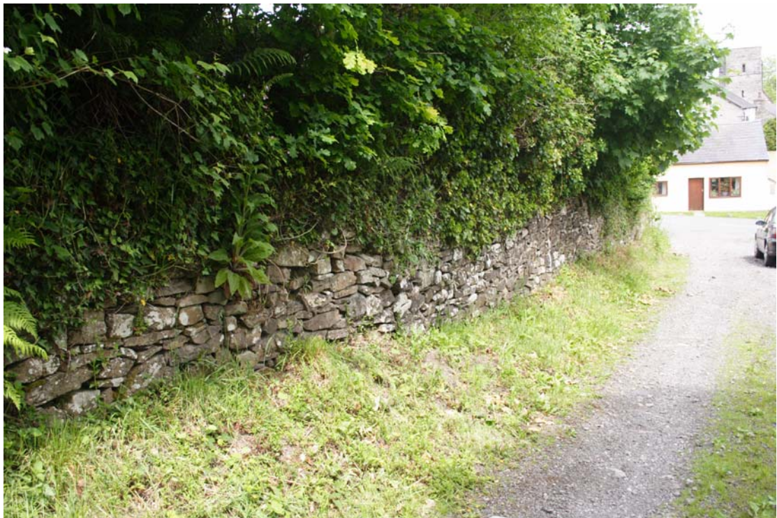
Plate 2: Surviving length of retaining wall alongside former main road into Llansawel.
