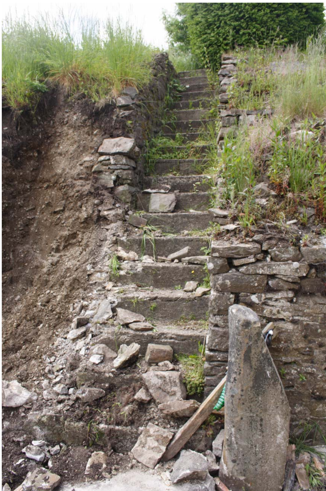
Plate 3: Modern steps prior to demolition.
