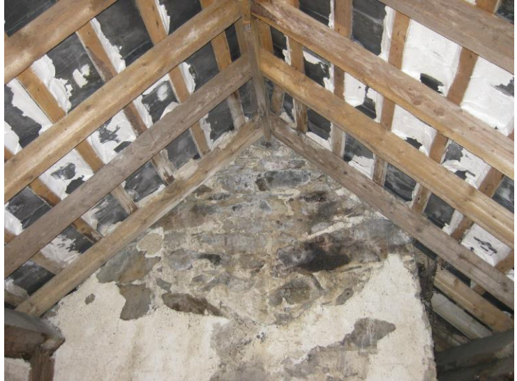
The attic showing the end chimney
