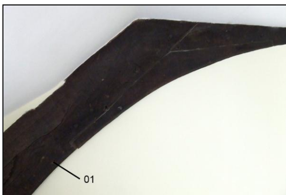
Figure 1: West cruck of central truss
