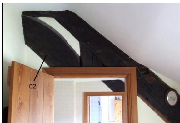
Figure 2: Timber above door, central truss
