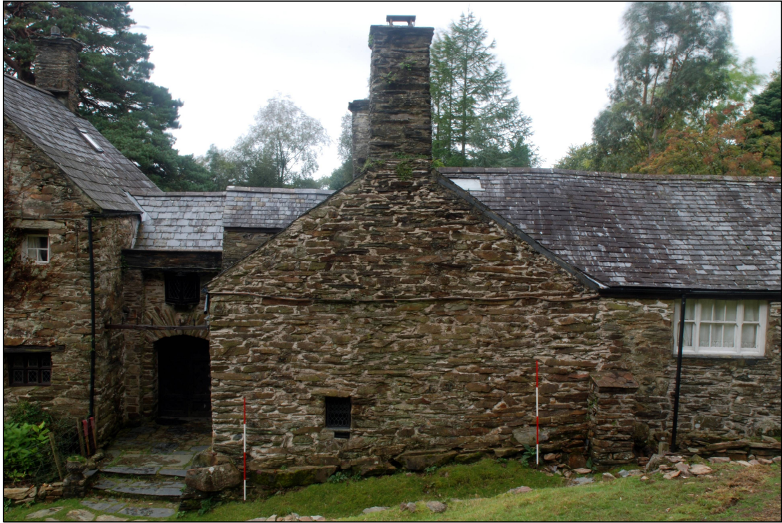
Plate 7: The front elevation of the northern range.
