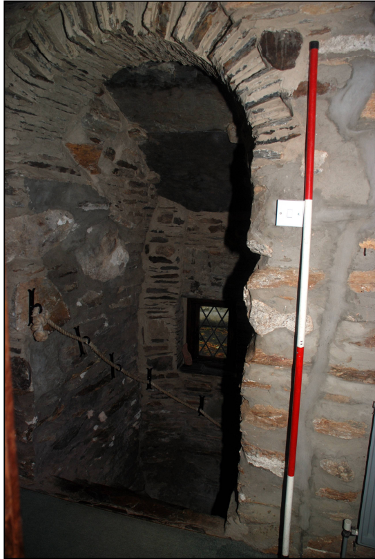
Plate 27: First floor access to the staircase
