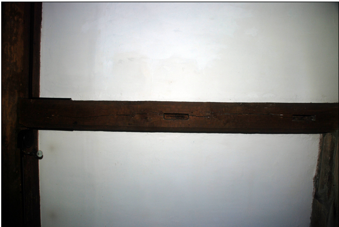
Plate 20: Mortice holes for the partition in the parlour
