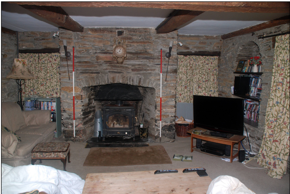
Plate 16: The chimney breast in the parlour
