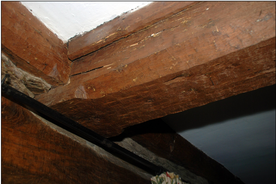
Plate 18: The chamfer and stop on the transverse beam in the parlour
