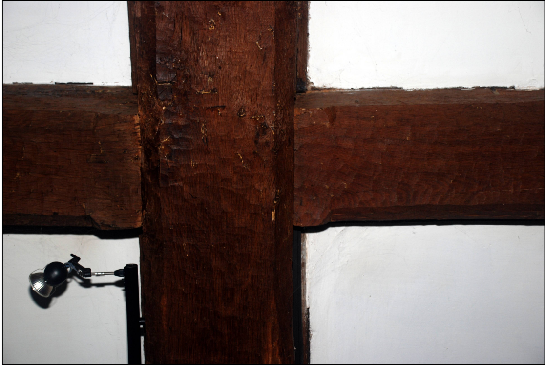
Plate 17: Chamfer and stops on ceiling beams of the parlour
