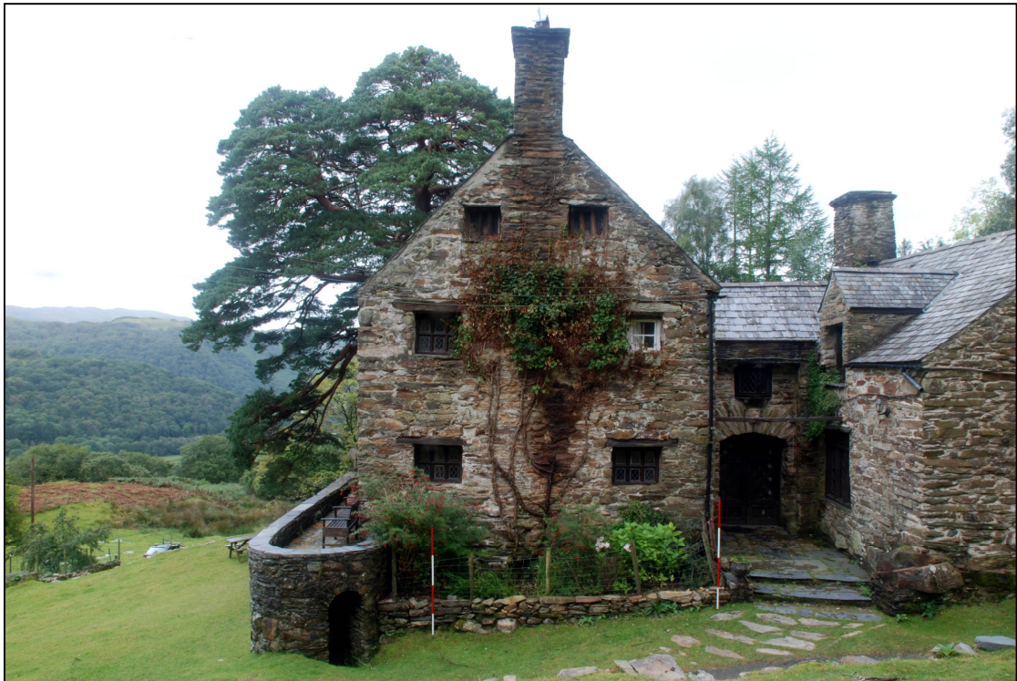
Plate 2: The north eastern elevation of the southern range
