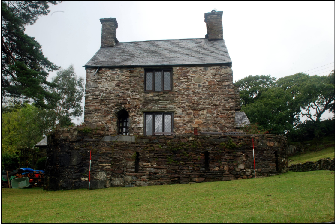
Plate 3: The south eastern elevation of the southern range
