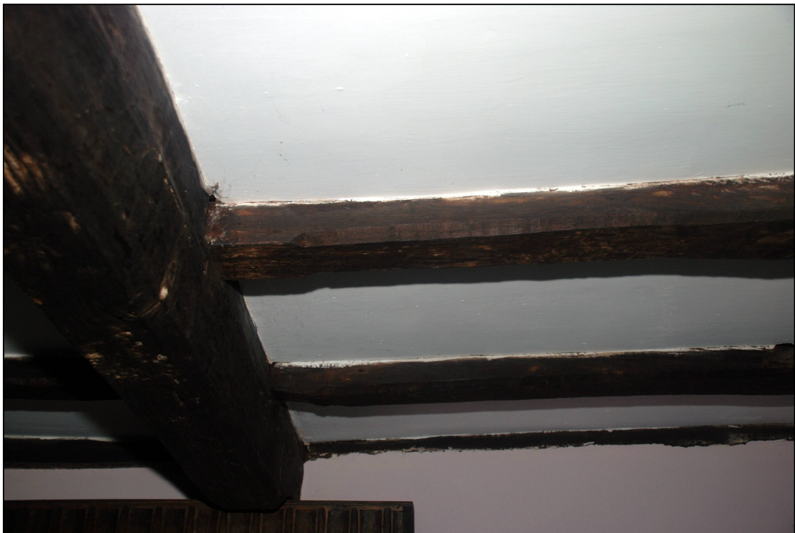
Plate 30: The joists in the first floor bedroom of the parlour block
