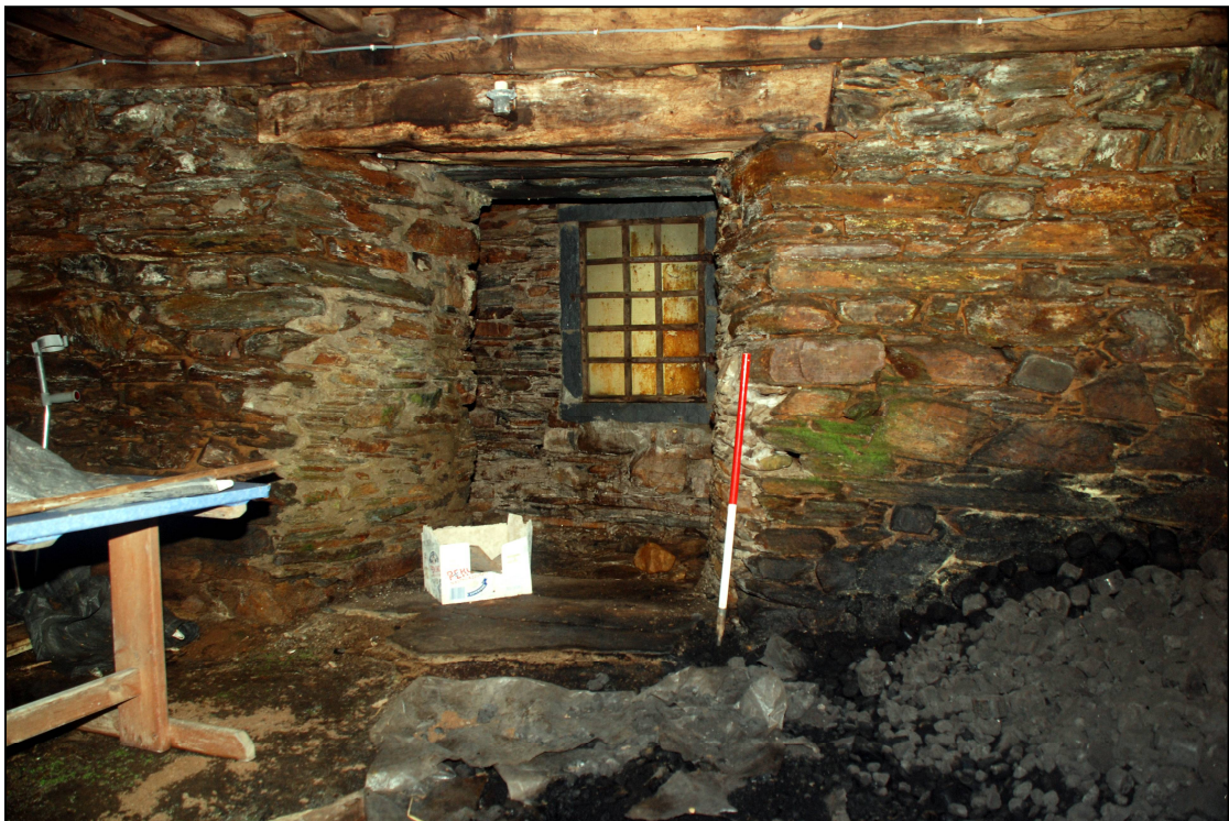
Plate 14: The “doorway” between the two cellars
