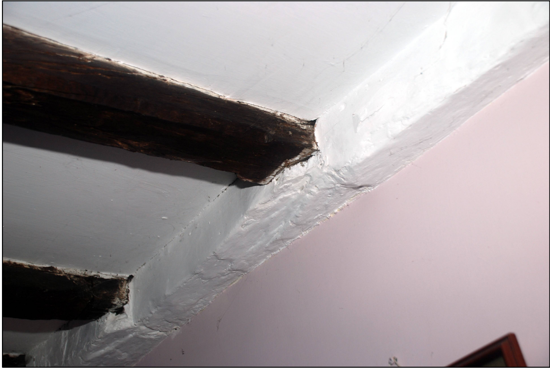
Plate 31: The beams in the first floor bedroom of the parlour block
