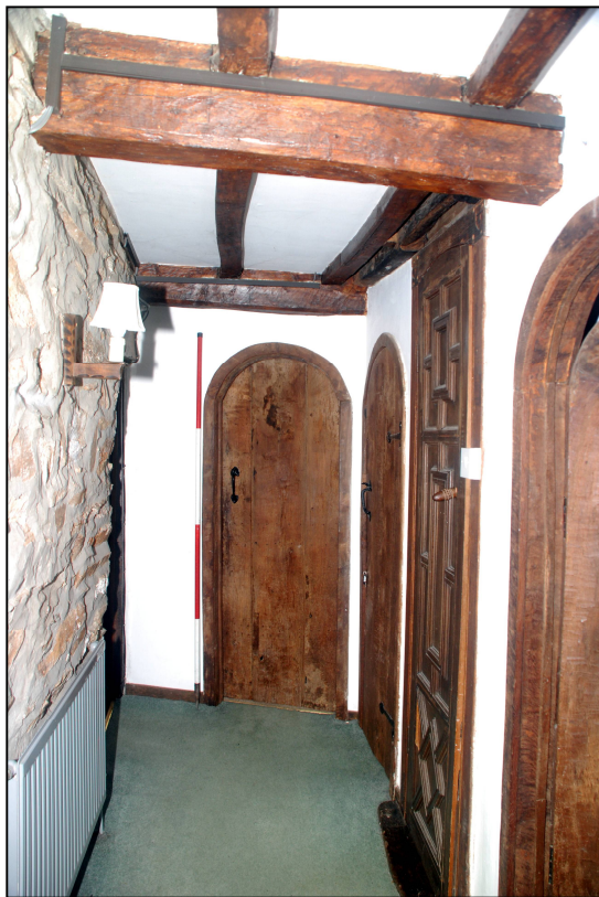
Plate 28: The first floor corridor in the parlour block
