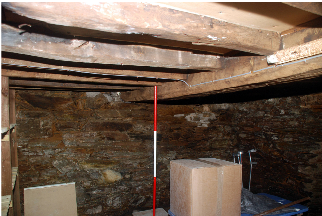
Plate 12: The cellar ceiling
