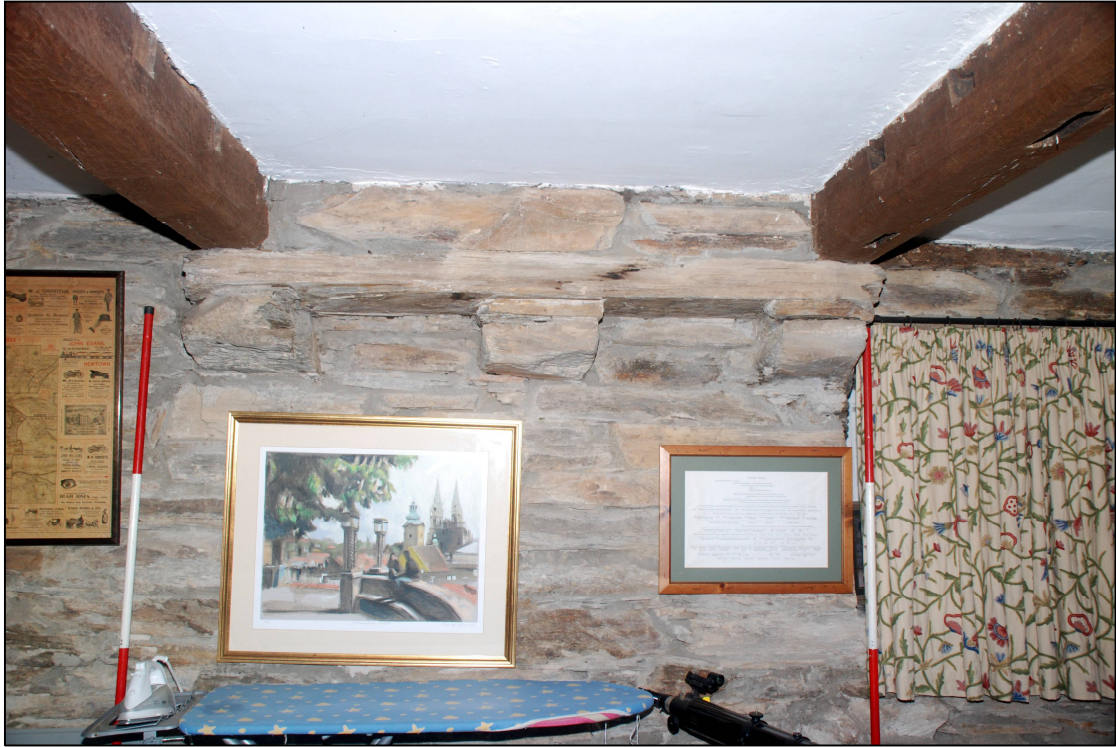
Plate 21: The corbelled support for the longitudinal beams in the parlour
