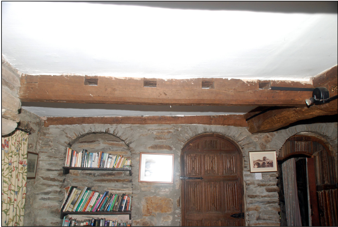
Plate 19: Mortice holes for joists in the parlour
