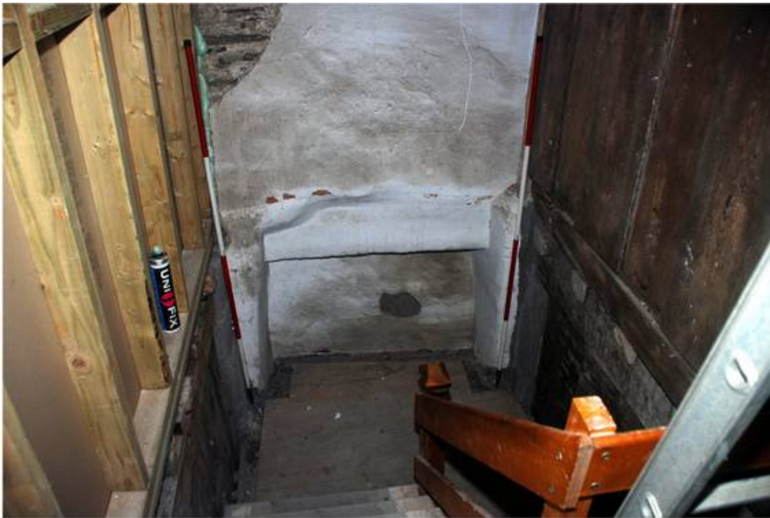
Plate 6: The blocked doorway seen in the stairwell.
