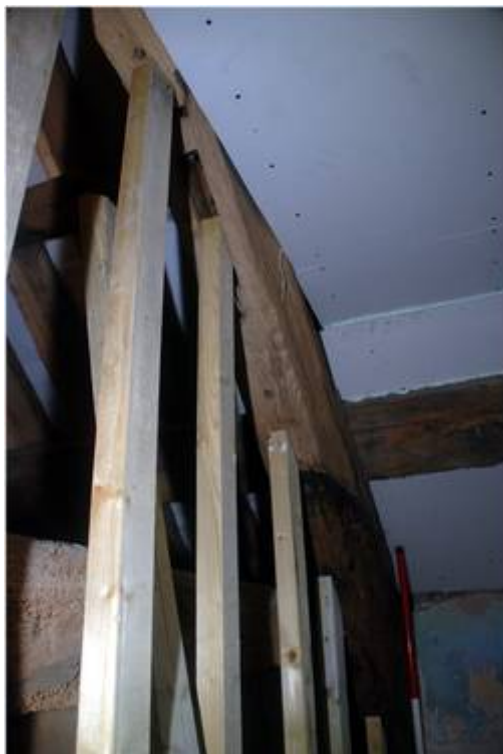
Plate 22: Mortice and dowel holes below northern principal rafter of Truss 2
