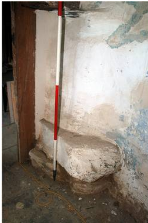
Plate 16: Remains of the stone staircase, looking SW
