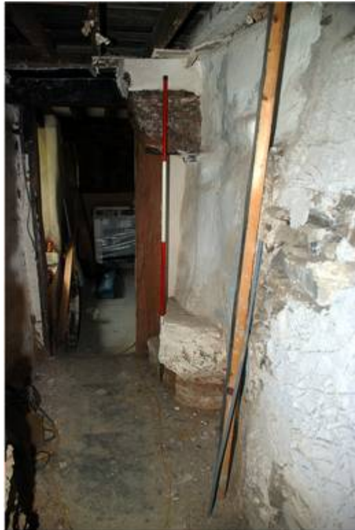
Plate 11: The end of the brussummer extending into the passage between main rooma and the lean too.
