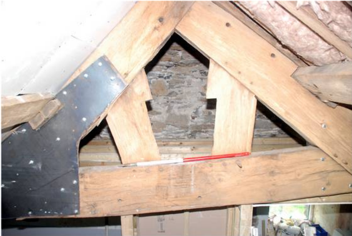
Plate 23: Truss 1, looking SW
