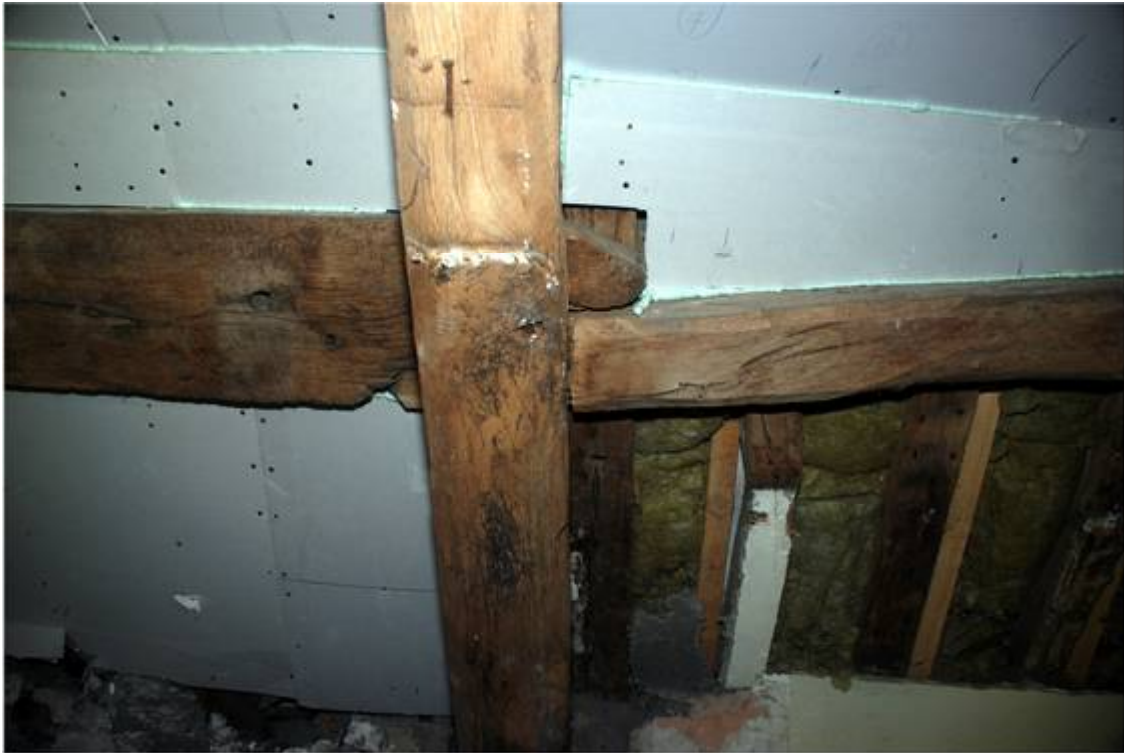
Plate 27: Detail of overlapping purlins above Truss 3
