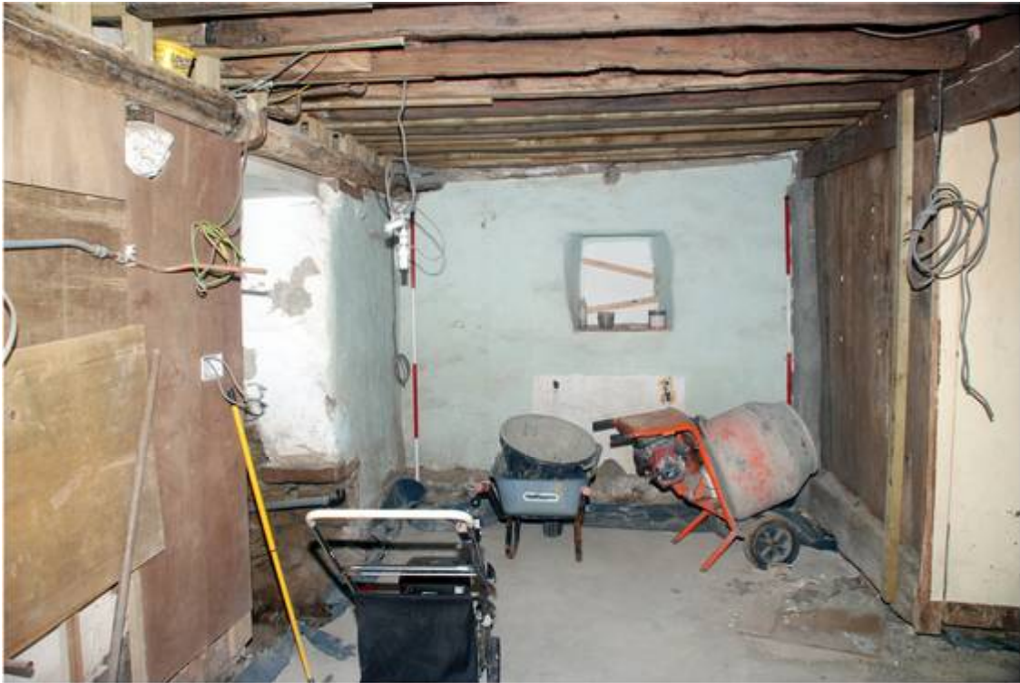
Plate 19: General view of the western ground floor room, looking NW
