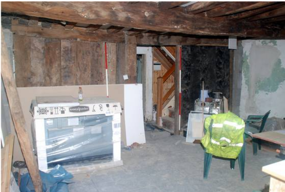
Plate 12: The partition in the main room, looking west
