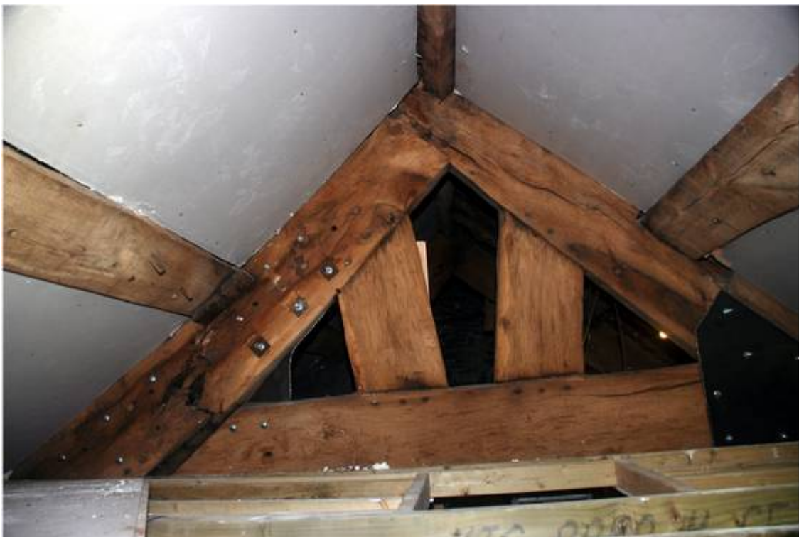
Plate 24: Truss 2, looking NE
