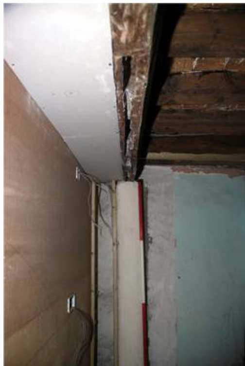
Plate 18: Socket for a post and plank partition in the ground floor, western room, looking SE
