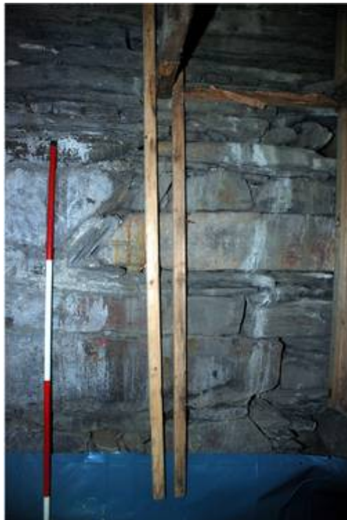
Plate 8: Stone work in north eastern gable of house
