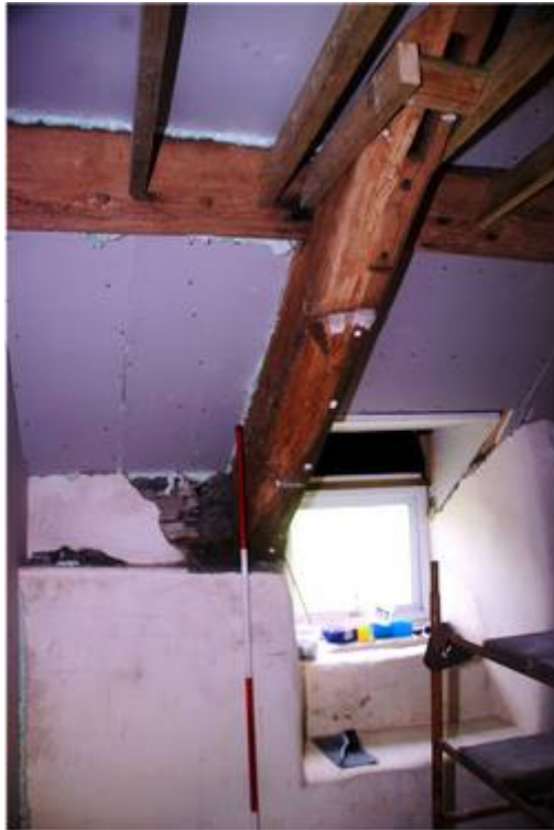
Plate 21: Mortice and dowel holes below the southern principal rafter of Truss 2
