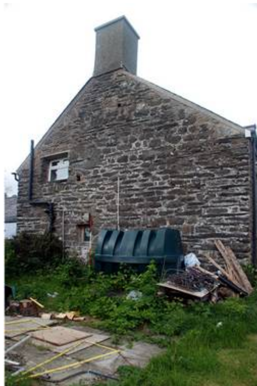
Plate 2: South western gable end
