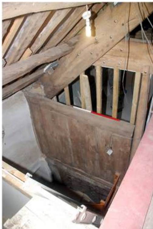
Plate 20: The relationship between the first floor partition and Truss 2
