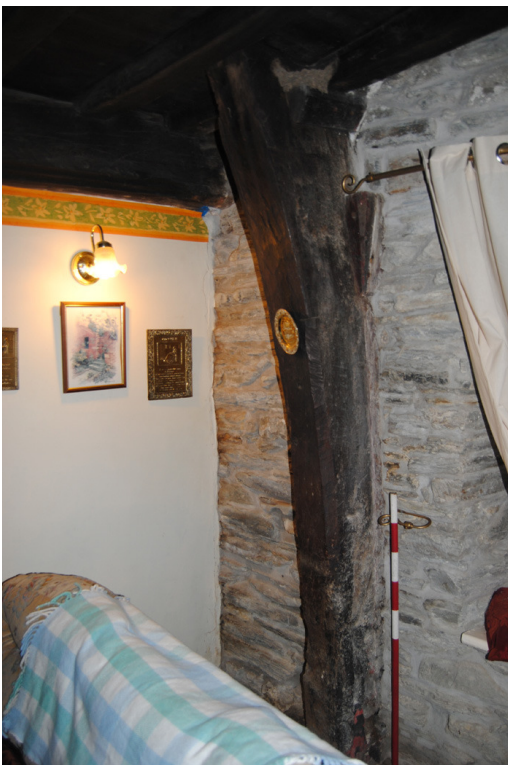
Plate 12: Eastern cruck blade visible in [GF02].
