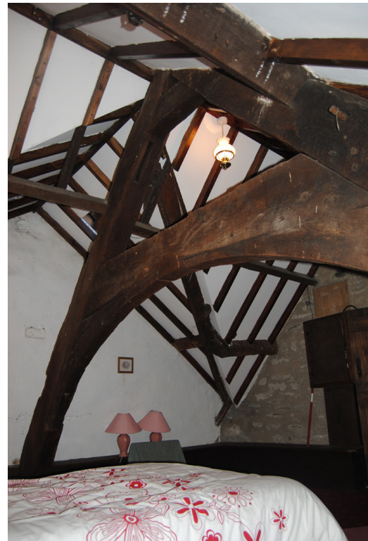
Plate 22: Room [1F01]; upper cruck looking NW.
