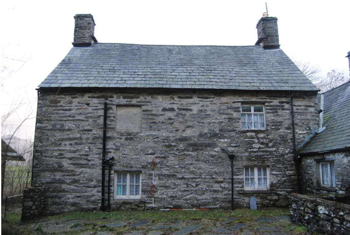
Plate 30: West Range; south elevation.
