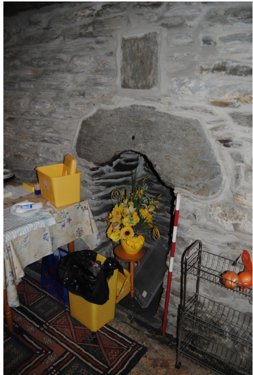
Plate 20: Small FP in rear of inserted stack.
