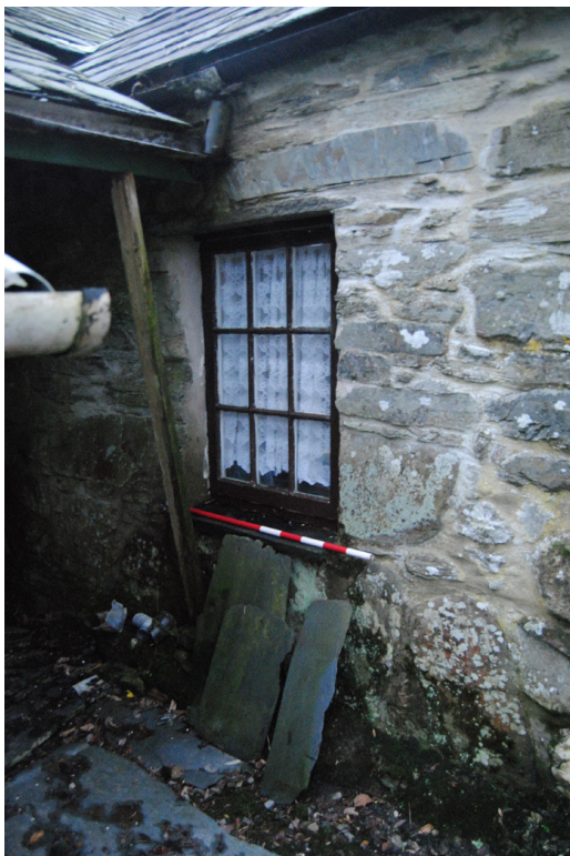
Plate 4: Reduced window opening.
