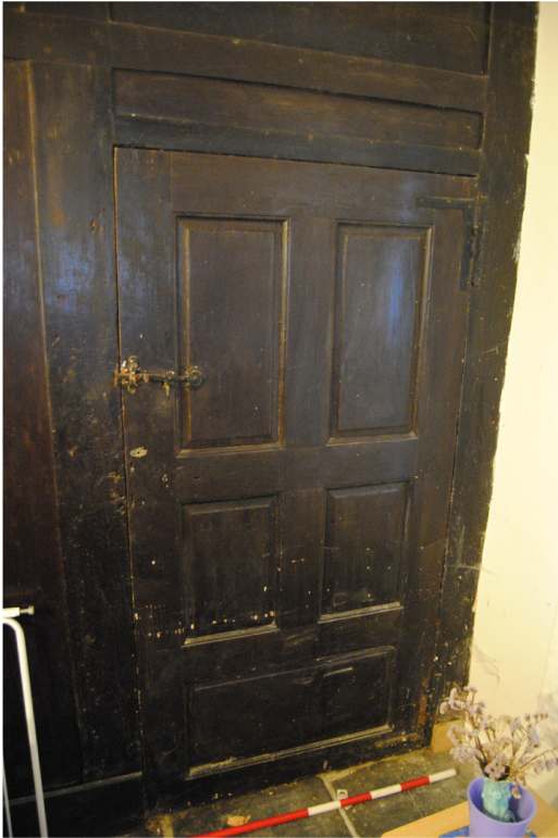
Plate 35: 5-panel door to understair cupboard.
