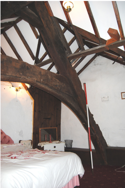
Plate 21: Room [1F01]; upper cruck looking SW.
