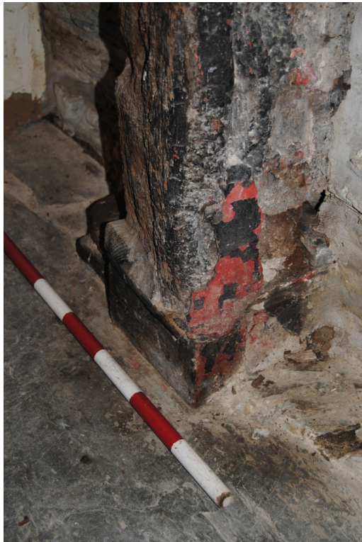
Plate 14: Foot of eastern cruck blade.
