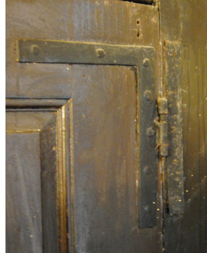
Plate 36: L-hinge to understair door.
