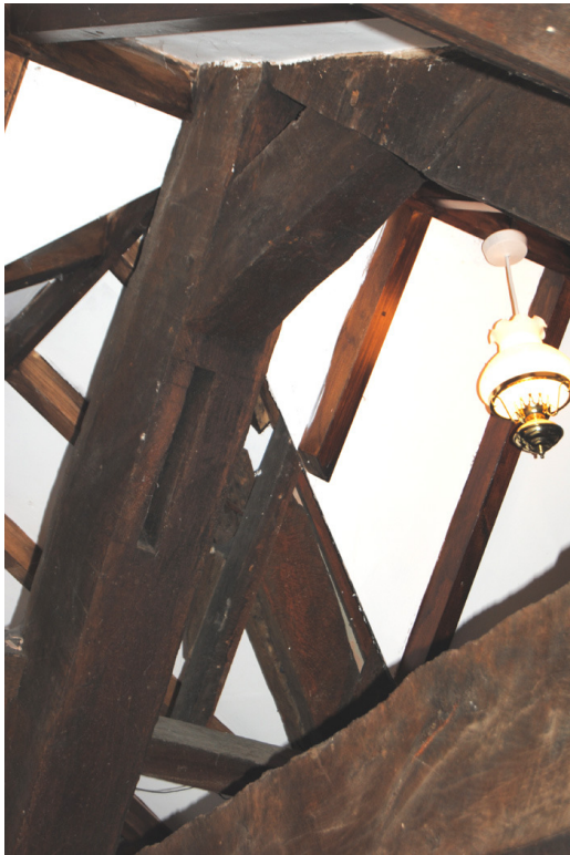
Plate 25: Redundant mortices (unpegged) for v-strutting above collar; note upper yoke.
