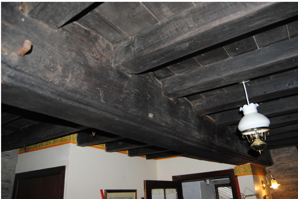
Plate 16: [GF02], inserted floor structure over former open hall.
