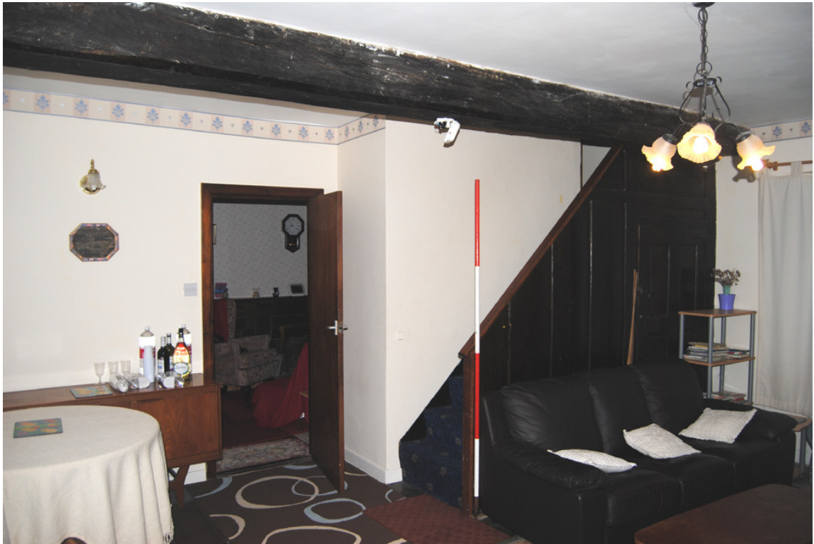
Plate 33: West Range; Room [GF07] looking south-east.
