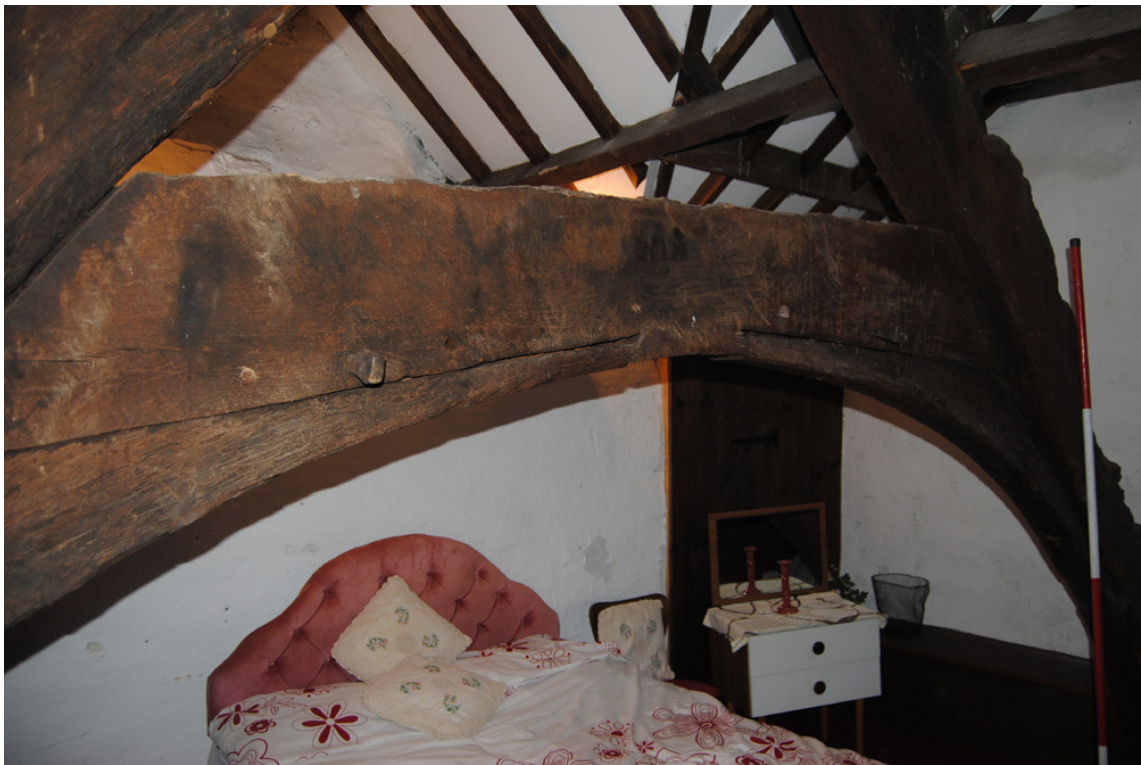
Plate 23: Cranked collar of open cruck truss.
