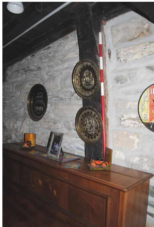
Plate 13: Western cruck blade visible in [GF02].
