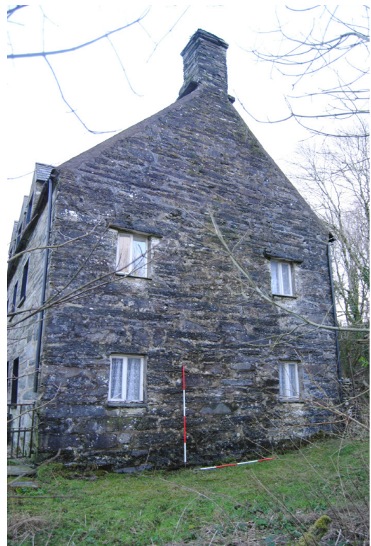
Plate 29: West Range; west elevation
