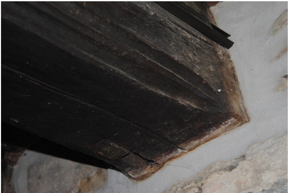
Plate 17: Decorated chamfer run-out to west end of main transverse beam of inserted floor.
