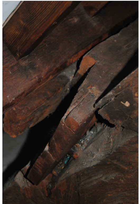
Plate 26: Detail of purlin scarf; splayed with squared abutments, single pegged.
