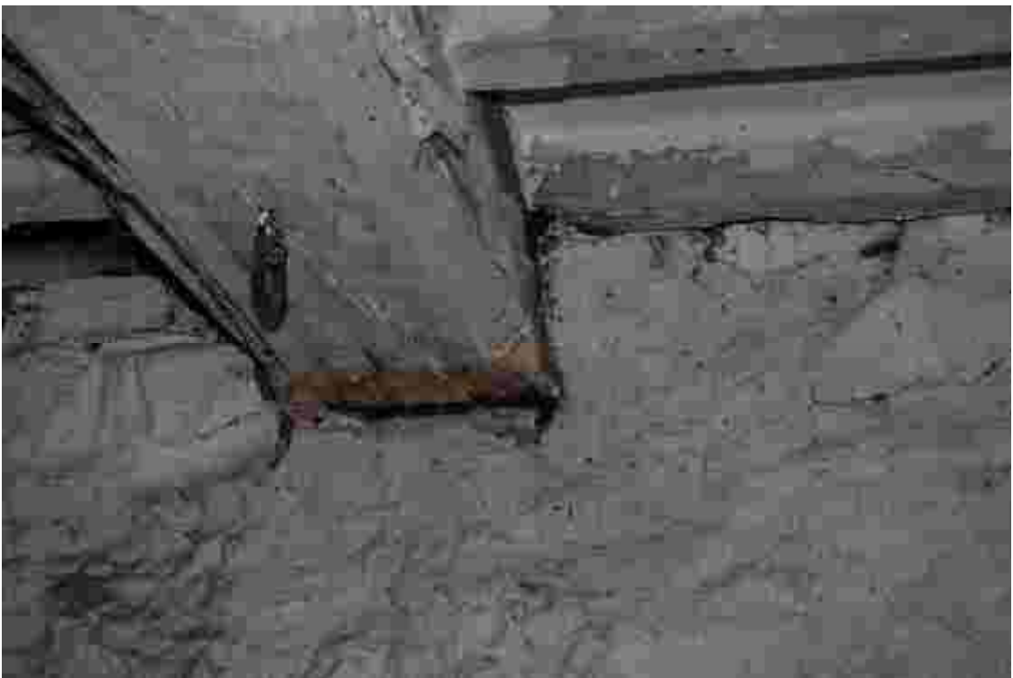
Plate 16: Beam in the northern ground floor room
