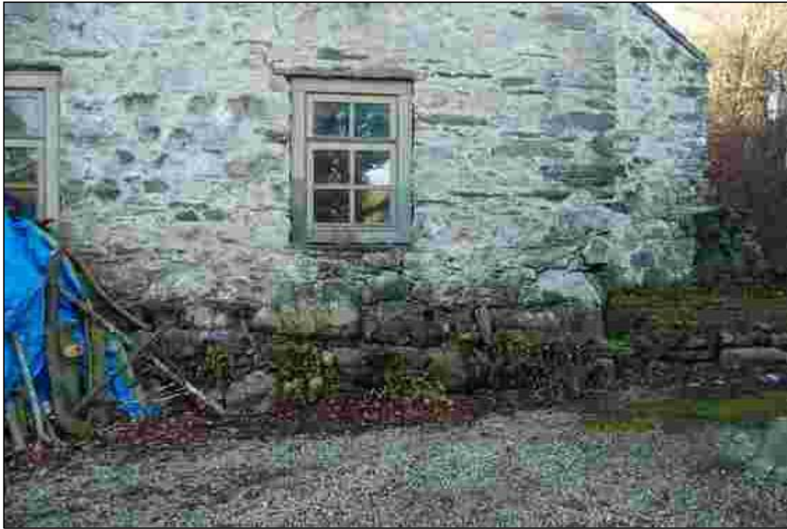
Plate 3: Exposed footings at the northern end of the eastern elevation
