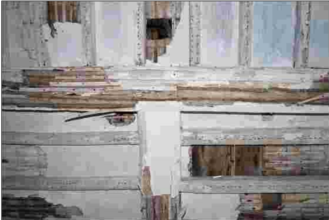
Plate 17: Sockets for the partition below the northern ground floor beam
