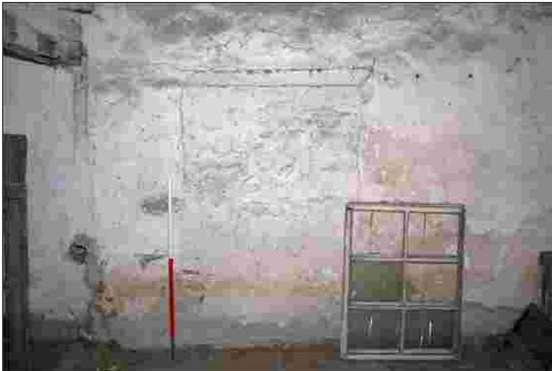
Plate 21: Block opening on the first floor
