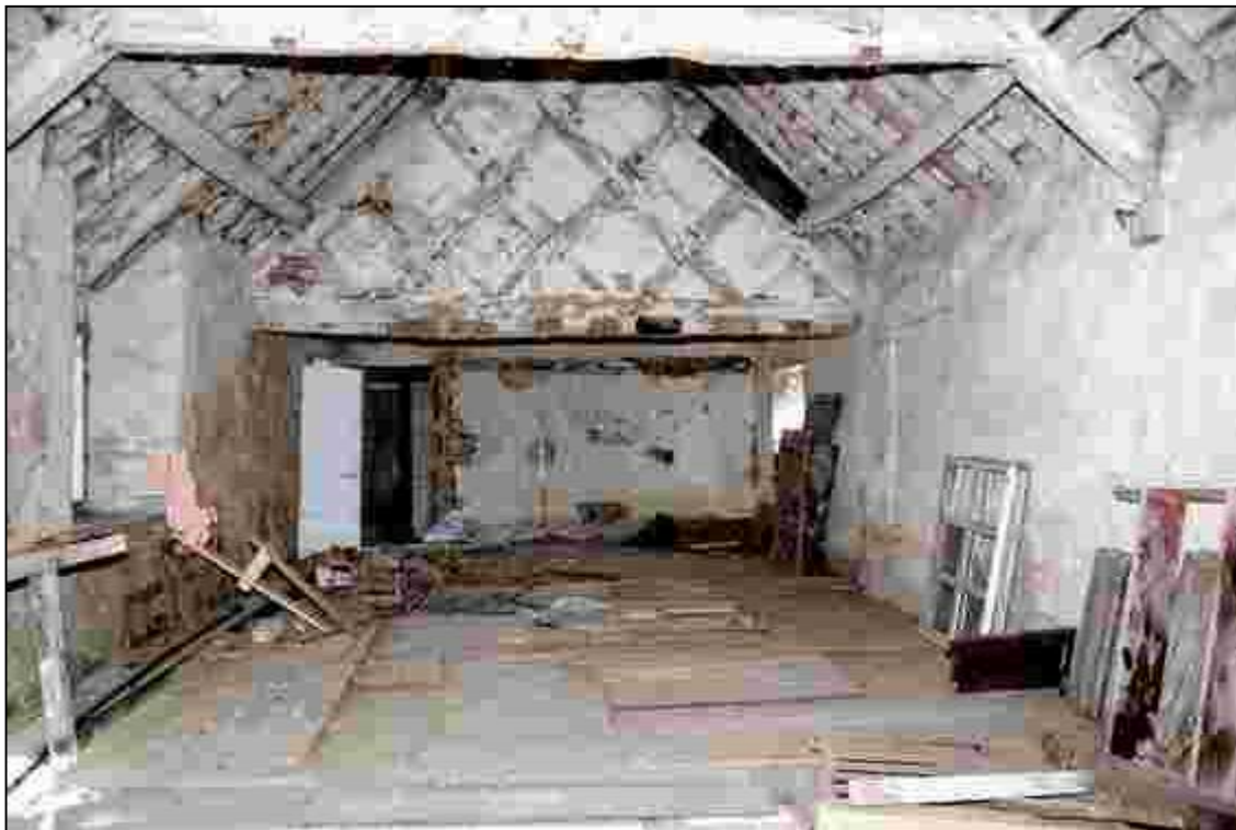
Plate 20: Southern, first floor room, looking north
