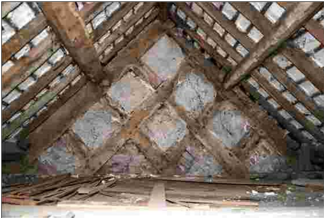
Plate 24: Rear face of Truss 2
