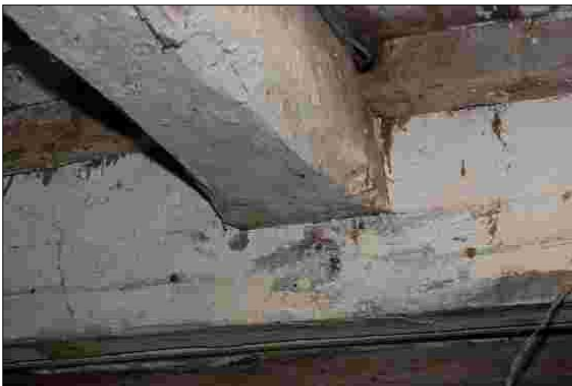
Plate 14: Northern beam in the southern ground floor room
