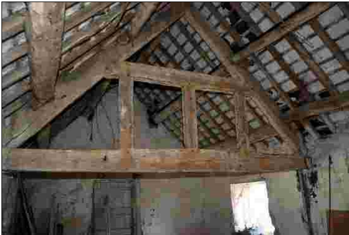
Plate 32: Truss 4, looking north
