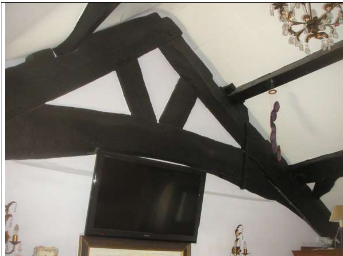
Plate 1 Truss 1 (E face)
