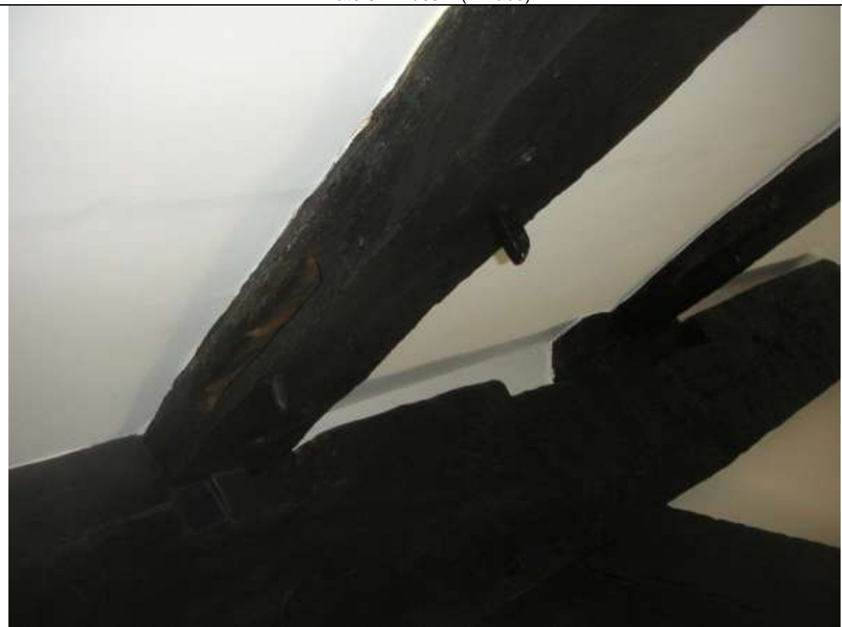
Plate 4 Truss 2 (slots and cut-outs for wind-braces)
