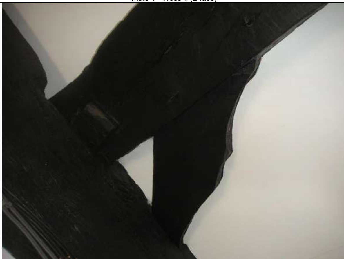
Plate 2 Surviving wind-brace on Truss 1 (E face, N end)
