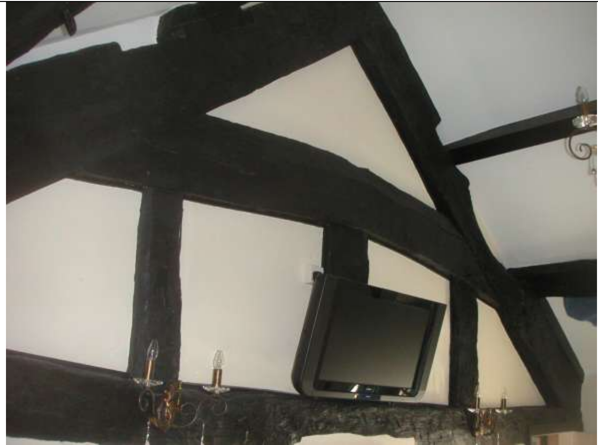
Plate 3 Truss 2 (W face)
