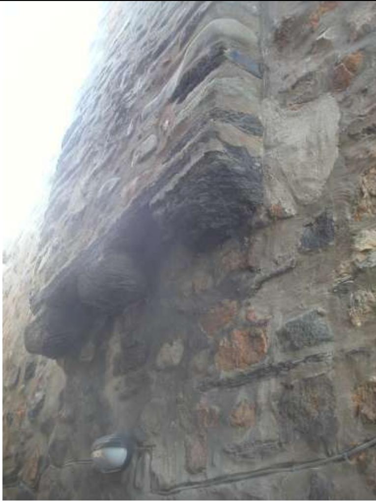
Plate 5 corbelled chimney at E gable
