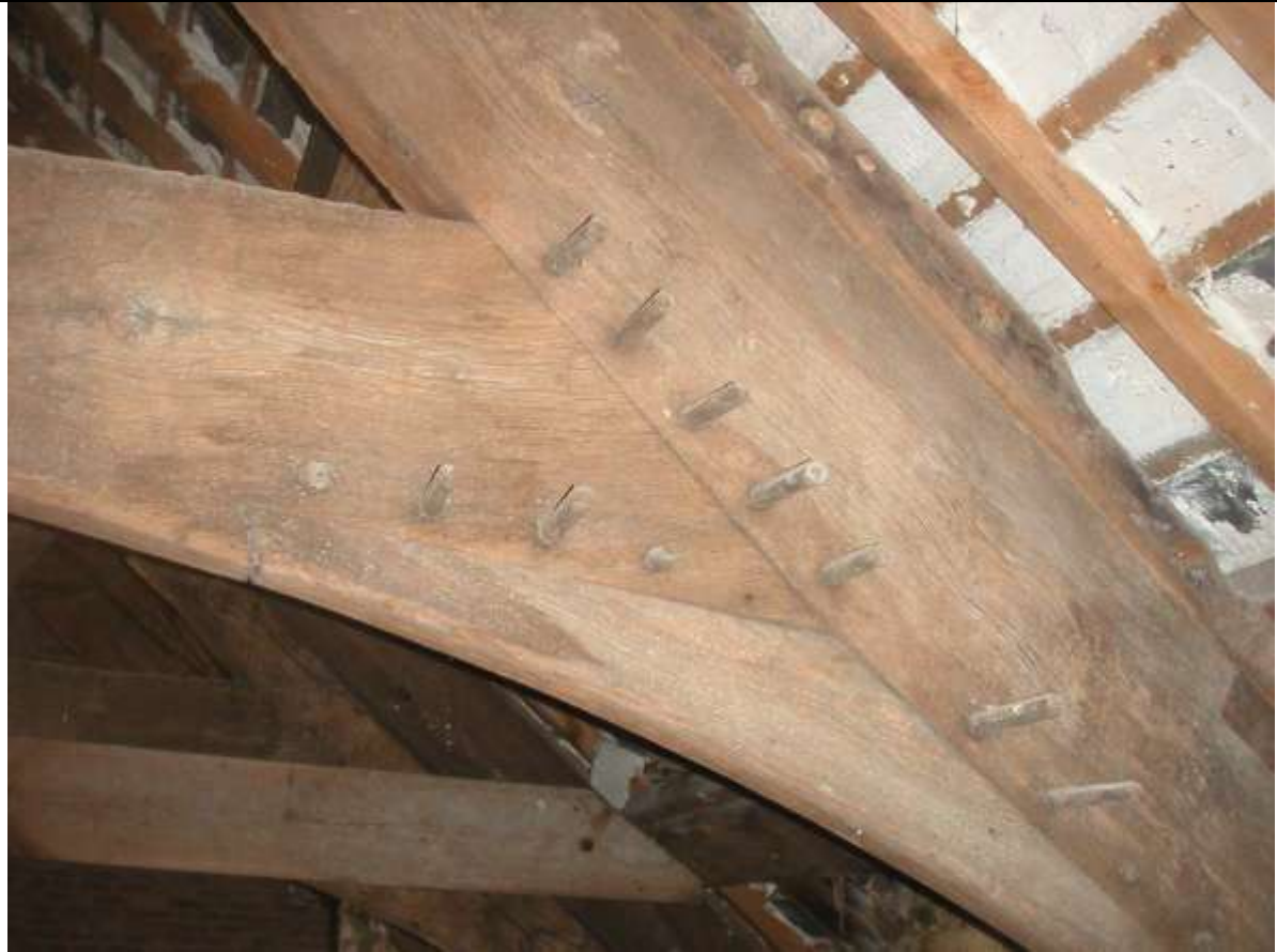
Plate 9 Truss T3, from west, showing pegged joint
