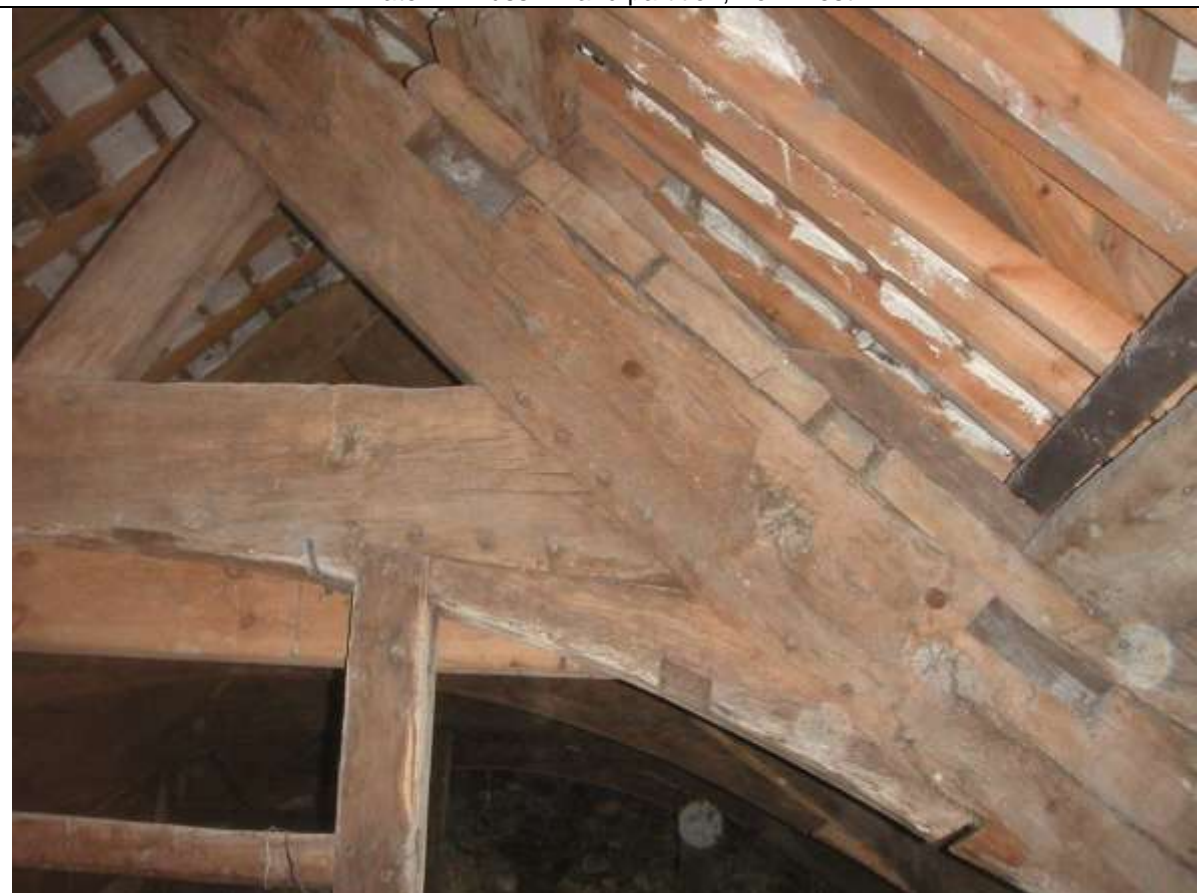
Plate 8 Truss T4, from east
