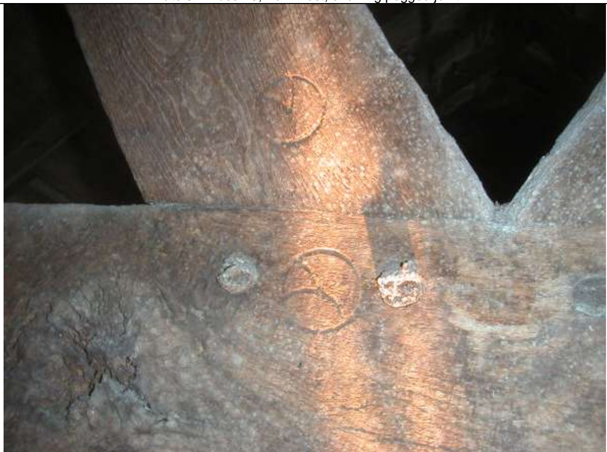
Plate 10 Truss T3, showing carpenter's marks on west face
