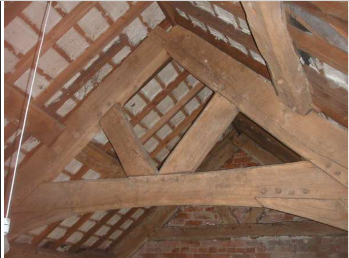
Plate 11 Truss T7, looking north (in north-west wing)
