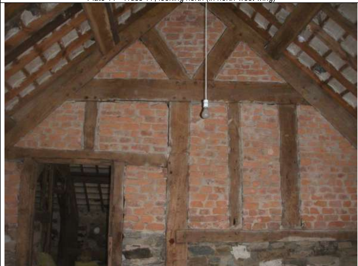
Plate 12 Truss T6, looking south, between north-west wing and original part
