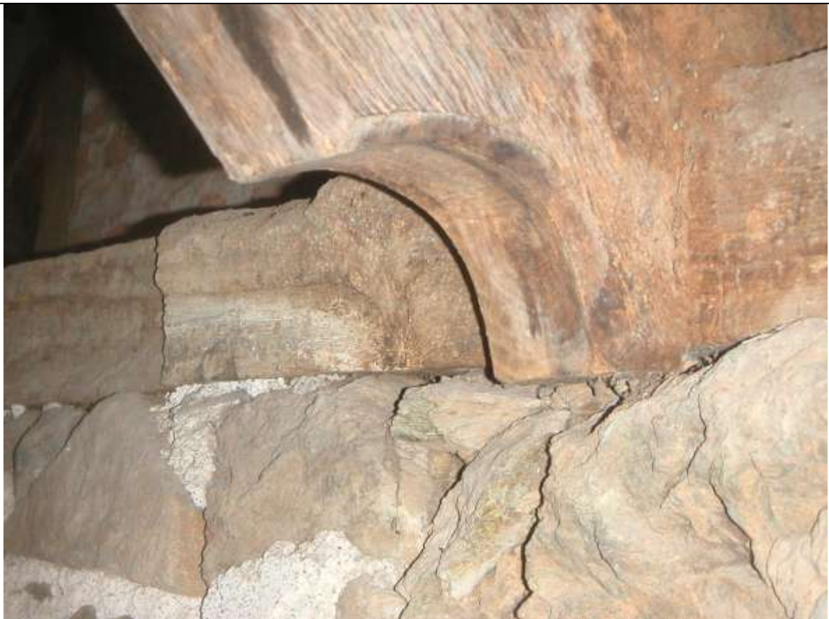
Plate 6 Cusp at foot of Truss T1 (north end)
