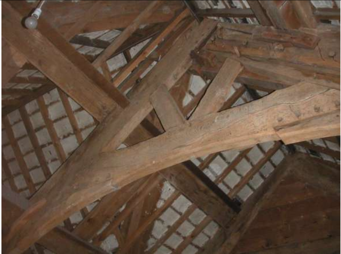
Plate 5 Truss T1, from west
