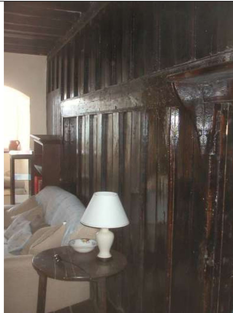
Plate 13 Post-and-panel partition at west end of ground floor
