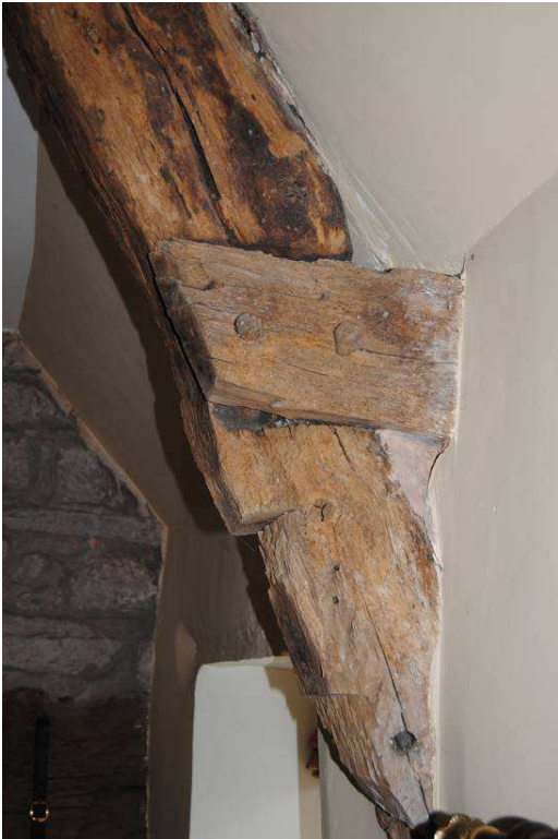
Plate 12: Cruck [T3] (W); truncated tie.
