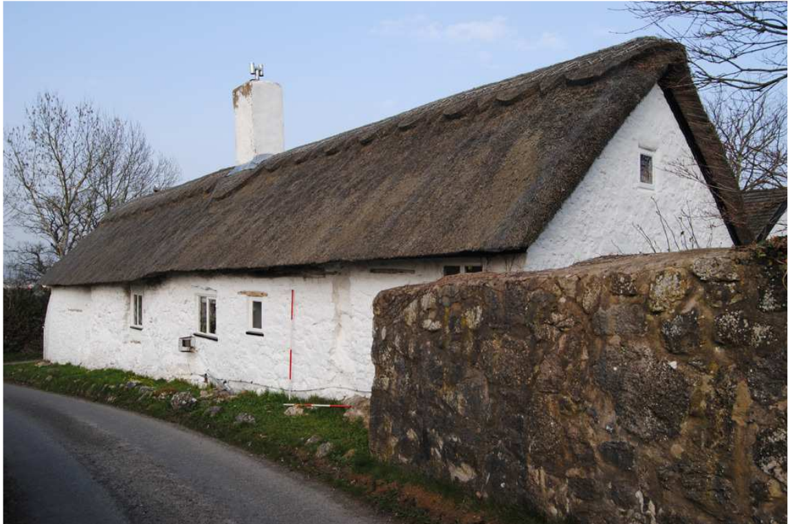
Plate 2: West elevation, oblique, looking north-east.
