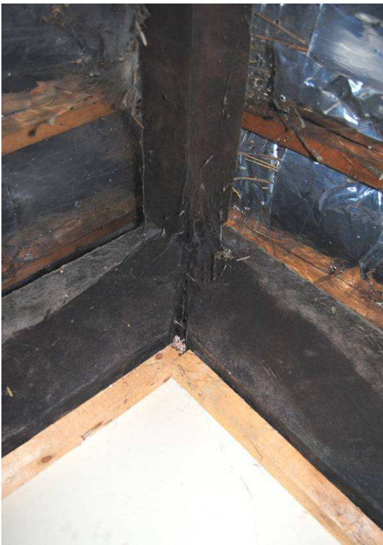
Plate 20: Cruck [T1], apex detail.
