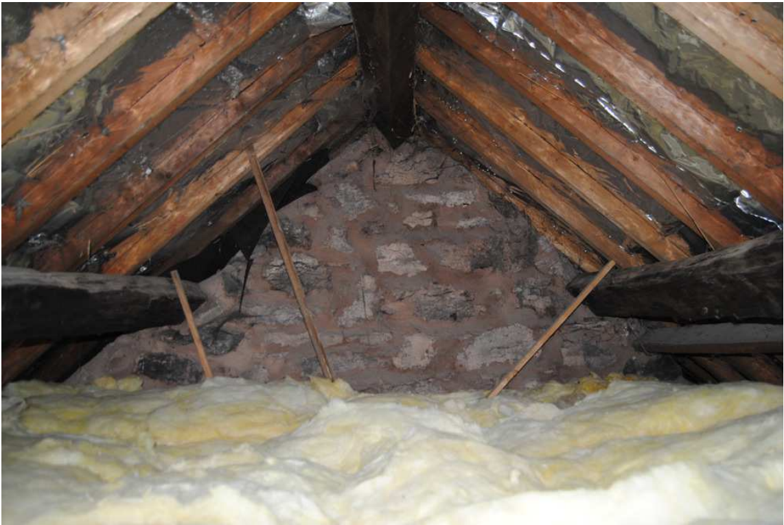
Plate 19: Roofspace over [GF03] showing upper purlin and square-section ridge piece.
