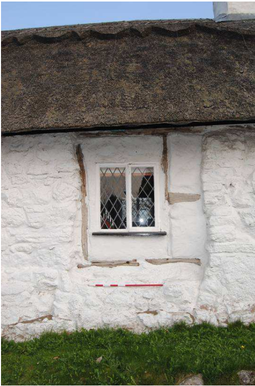
Plate 3: Section of primary wall framing visible within west elevation.
