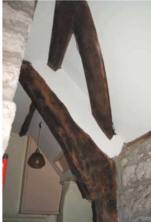
Plate 15: Cruck [T2] (E); wind-bracing to lower purlin.
