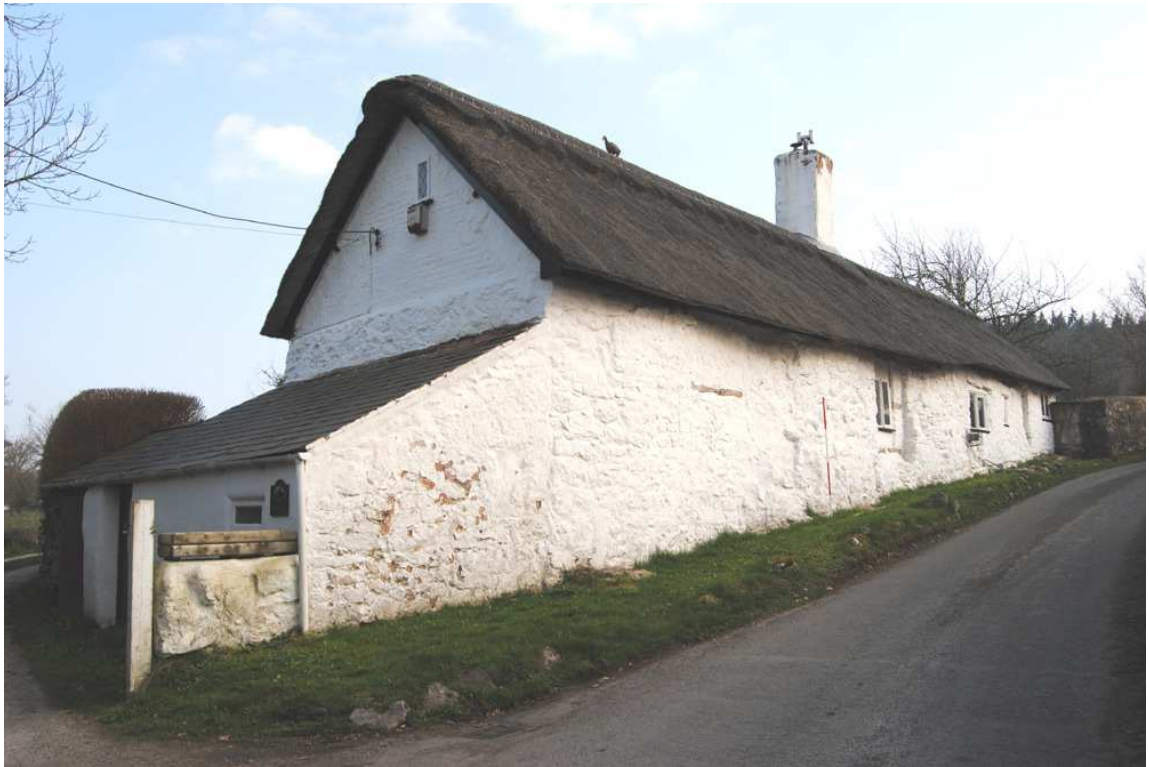
Plate 1: West elevation, oblique, looking south-east.
