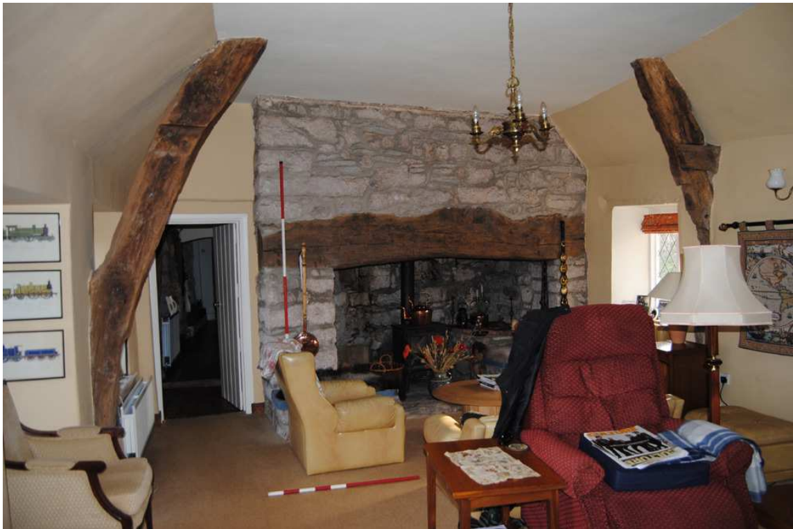
Plate 10: Cruck [T3] looking south towards inserted stack.
