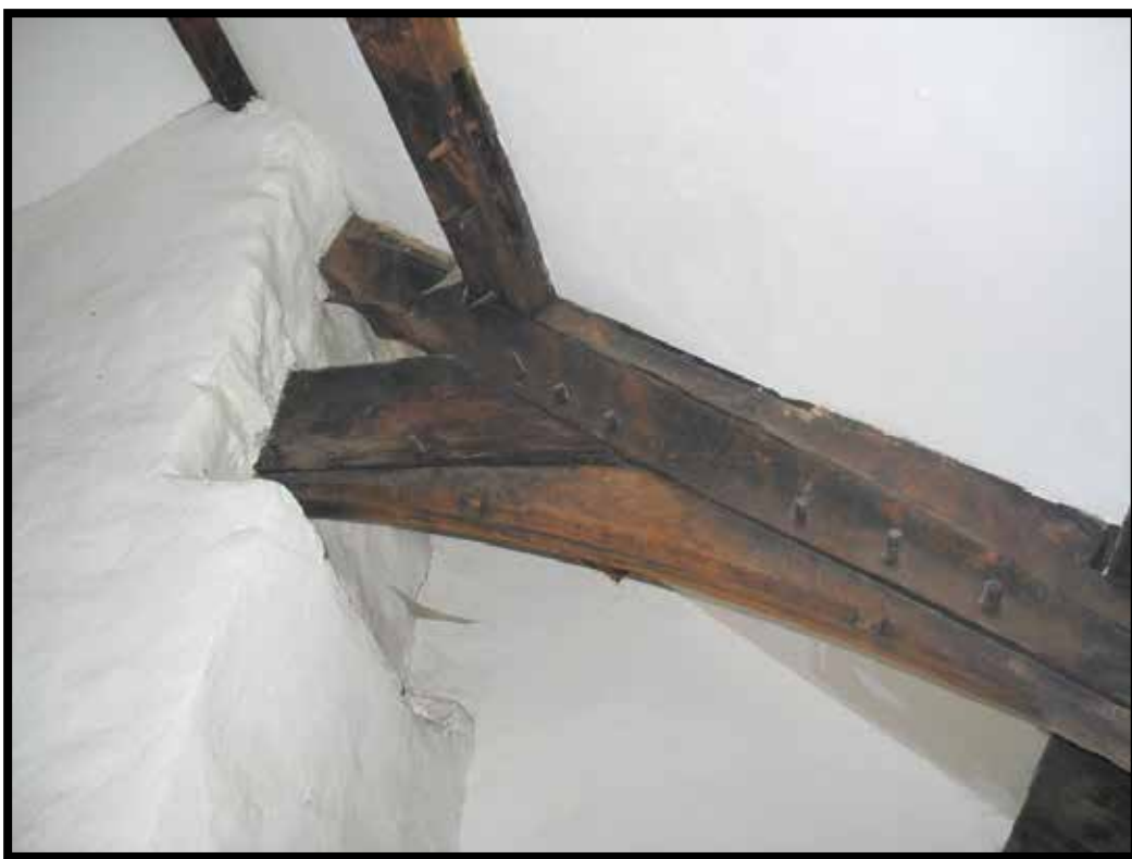
Plate 25: T2W: Pegs, wind brace mortise; smoke black
