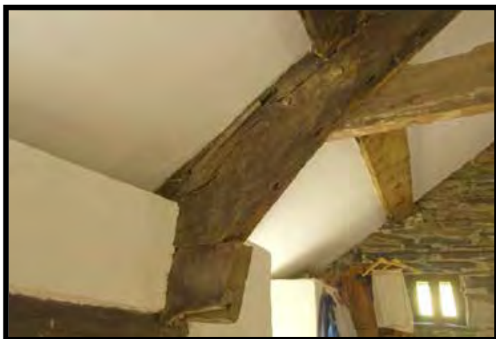
Plate 22: T1 – truncated tie beam
