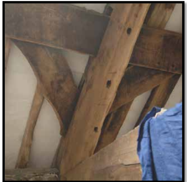
Plate 30: T3: wind braces and stave holes
