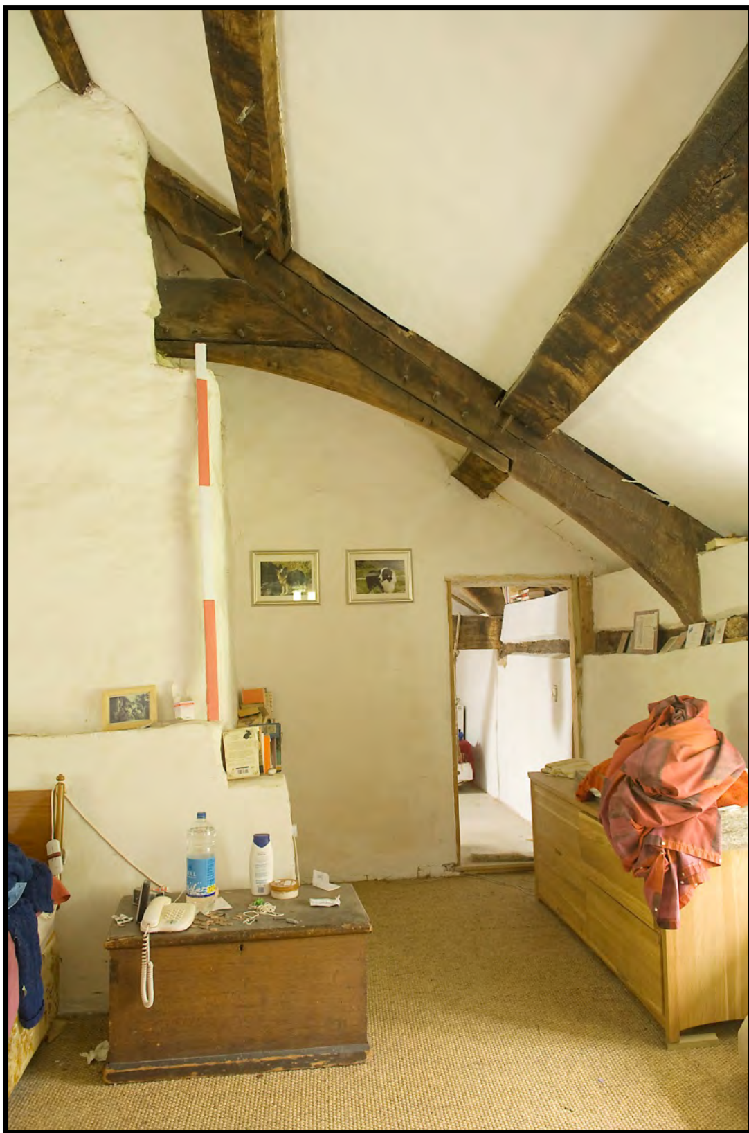
Plate 24: T2W: arch-braced truss from north east
