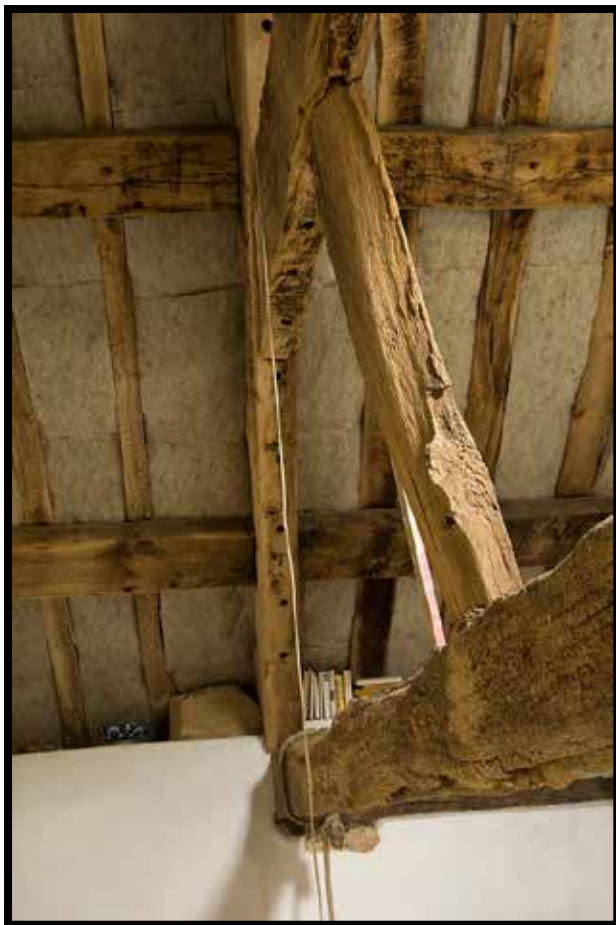
Plate 29: T3: truss showing erosion, stave holes
