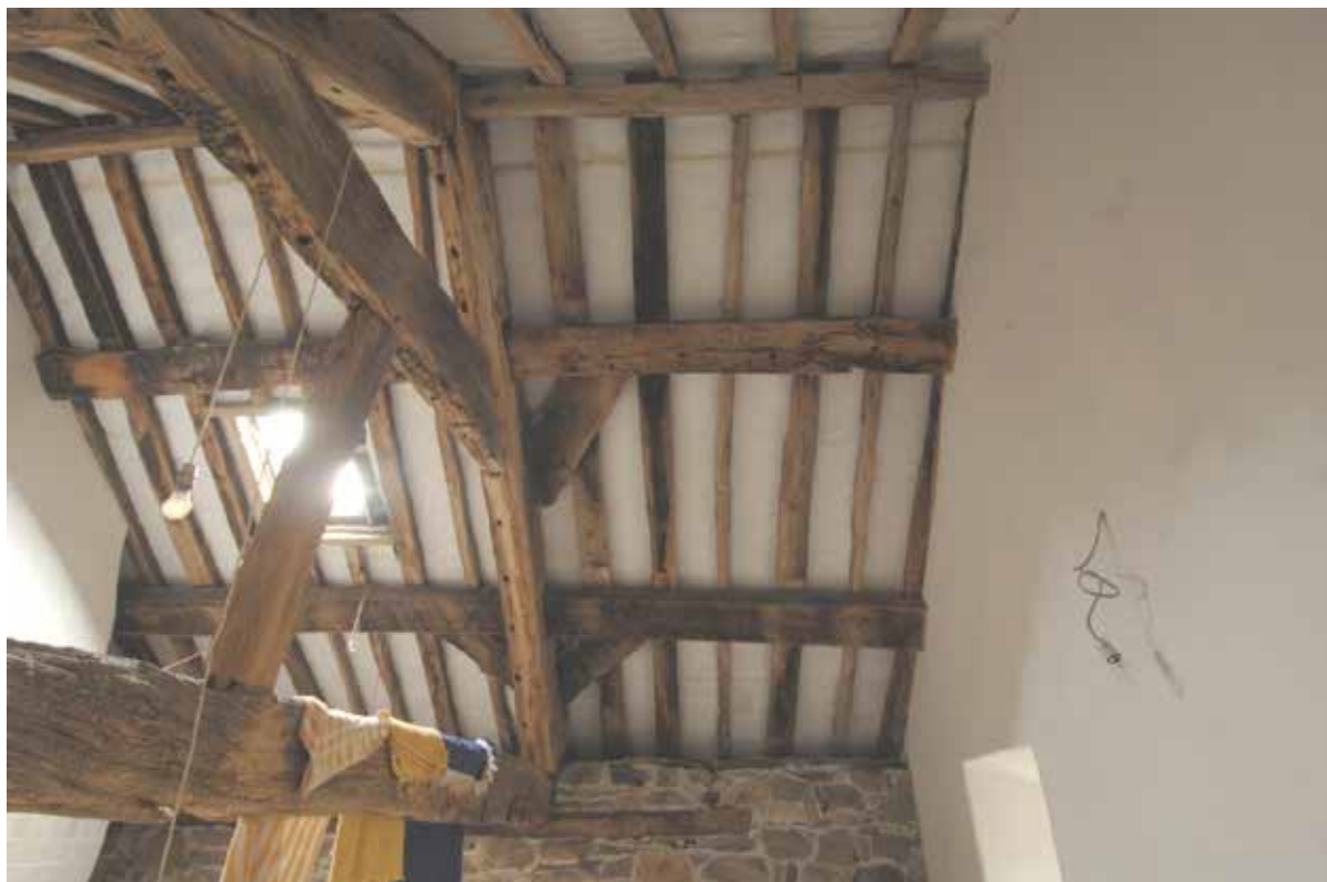
Plate 33: T3: rafters & wind braces
