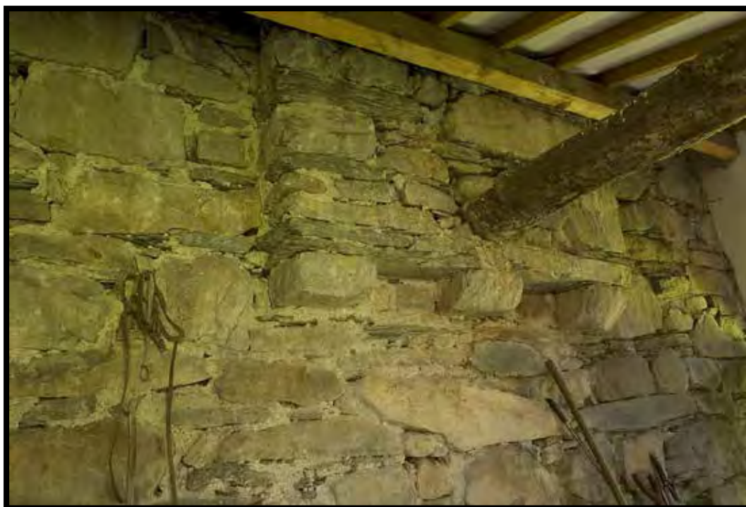
Plate 6: NE gable – corbelled external chimney breast
