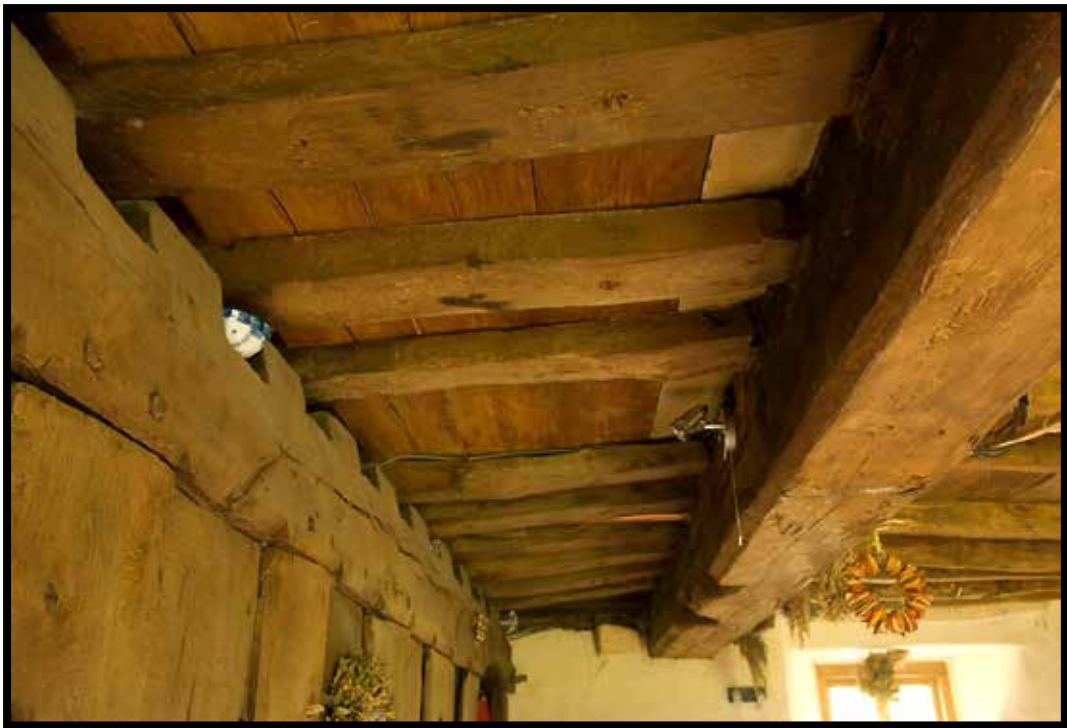
Plate 17: Dais canopy, screen and later pine beam
