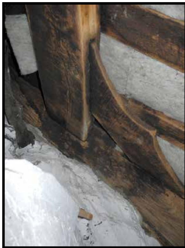
Plate 27: T2E: eastern principal -wind brace detail
