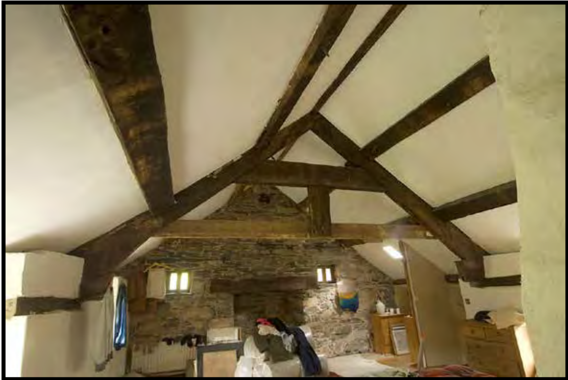
Plate 19: Truss 1. Lost tie beam to collar, post and tie beam truss.
