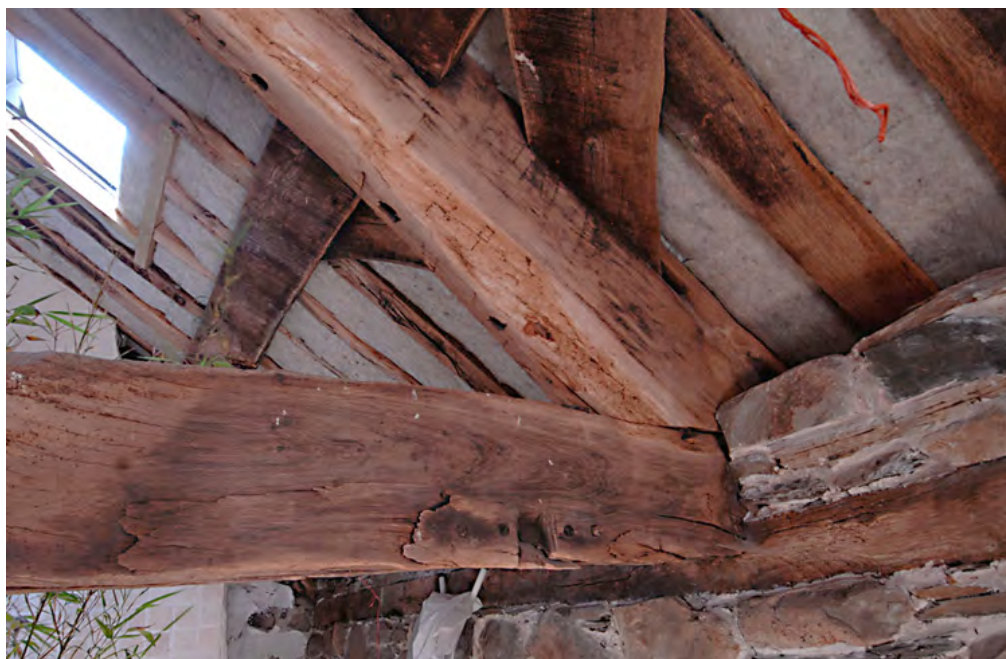
Plate 31: T3: base of principal and tie-beam; housing & peg holes?
