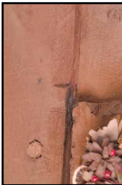
Plate 16: Screen detail – nailhead stop & chamfers
