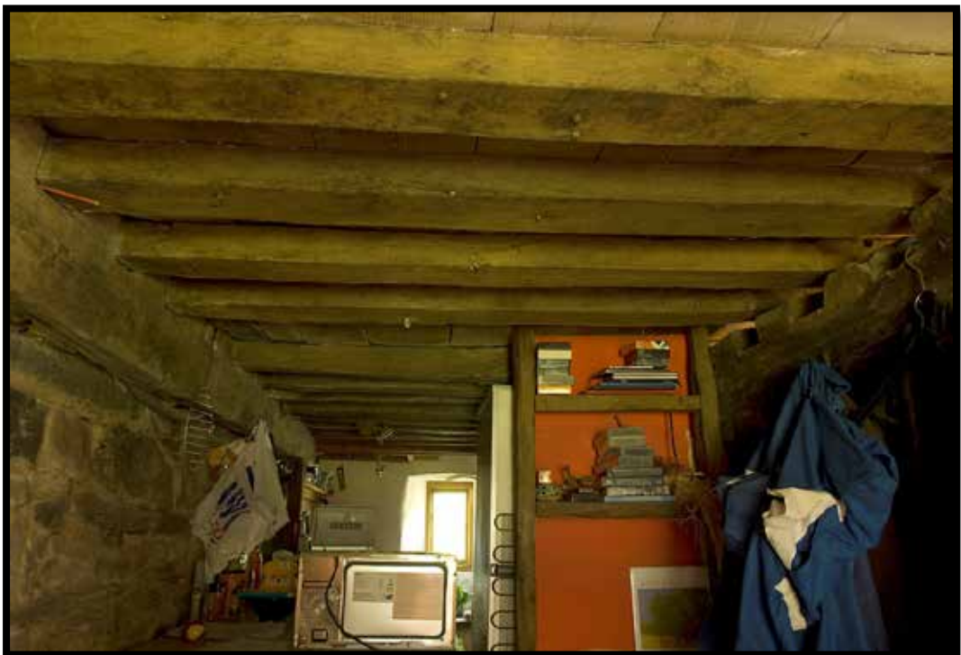
Plate 18: Joists over inner room with supporting beam to left
