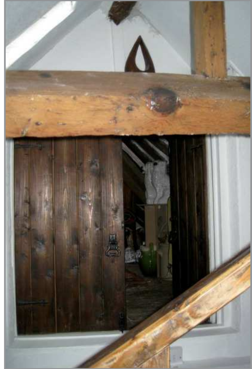
Plate 18: Door leading into bathroom showing blocked window. Facing north-west
