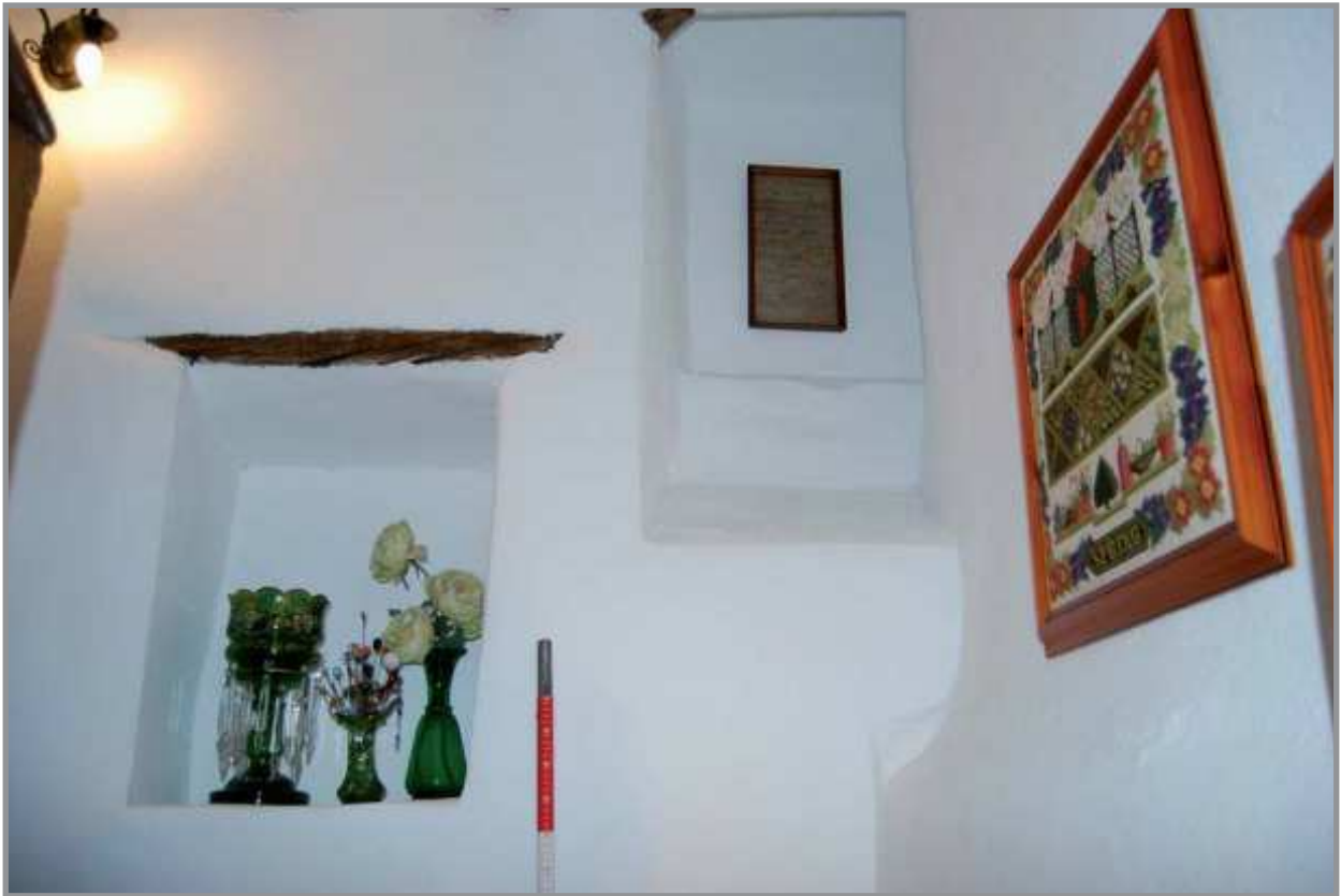
Plate 9: Stairway, showing blocked window. Facing south-west
