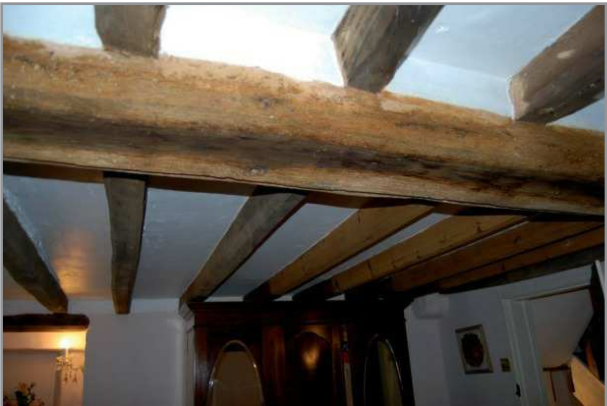
Plate 16: Front bedroom, showing chamfered beam. Facing south
