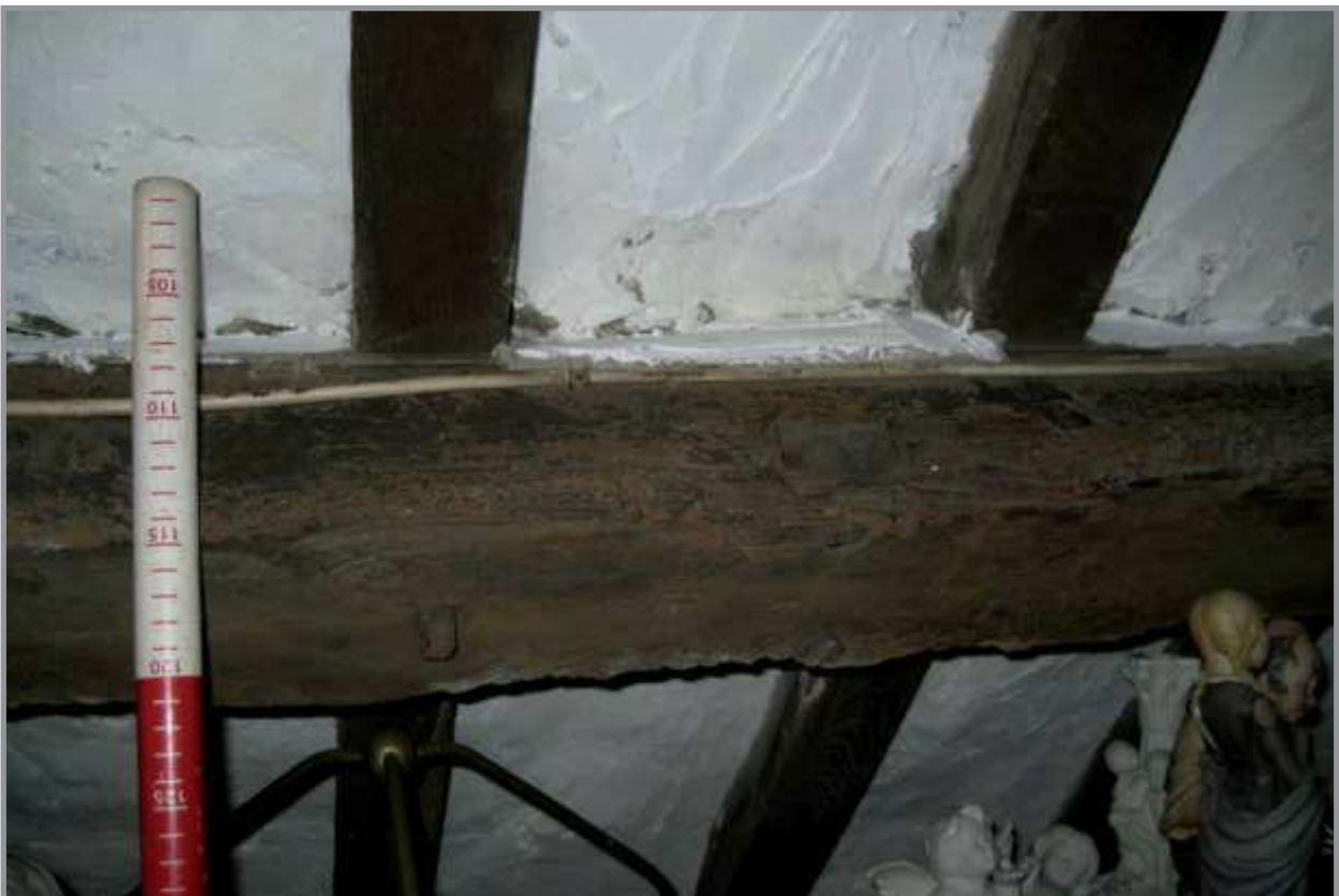
Plate 24: Attic room, showing timber detail. Facing north-west
