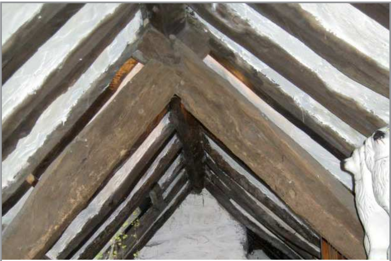
Plate 22: Truss 2 in attic room. Facing south-west
