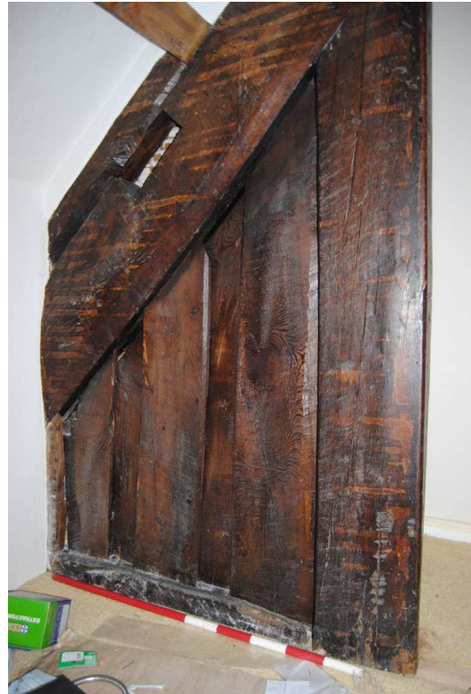
Plate 39: T1 (E), in-situ planking panel infill.
