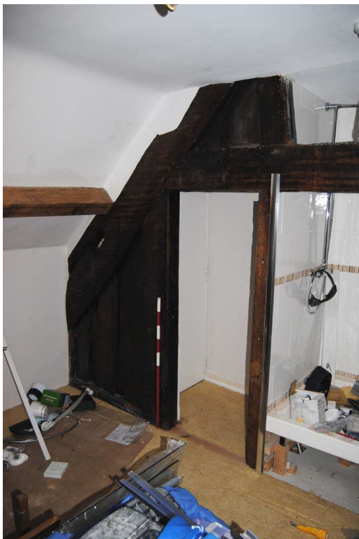
Plate 36: Room [2F01] ('Artro'); detail of Truss T1 (E).
