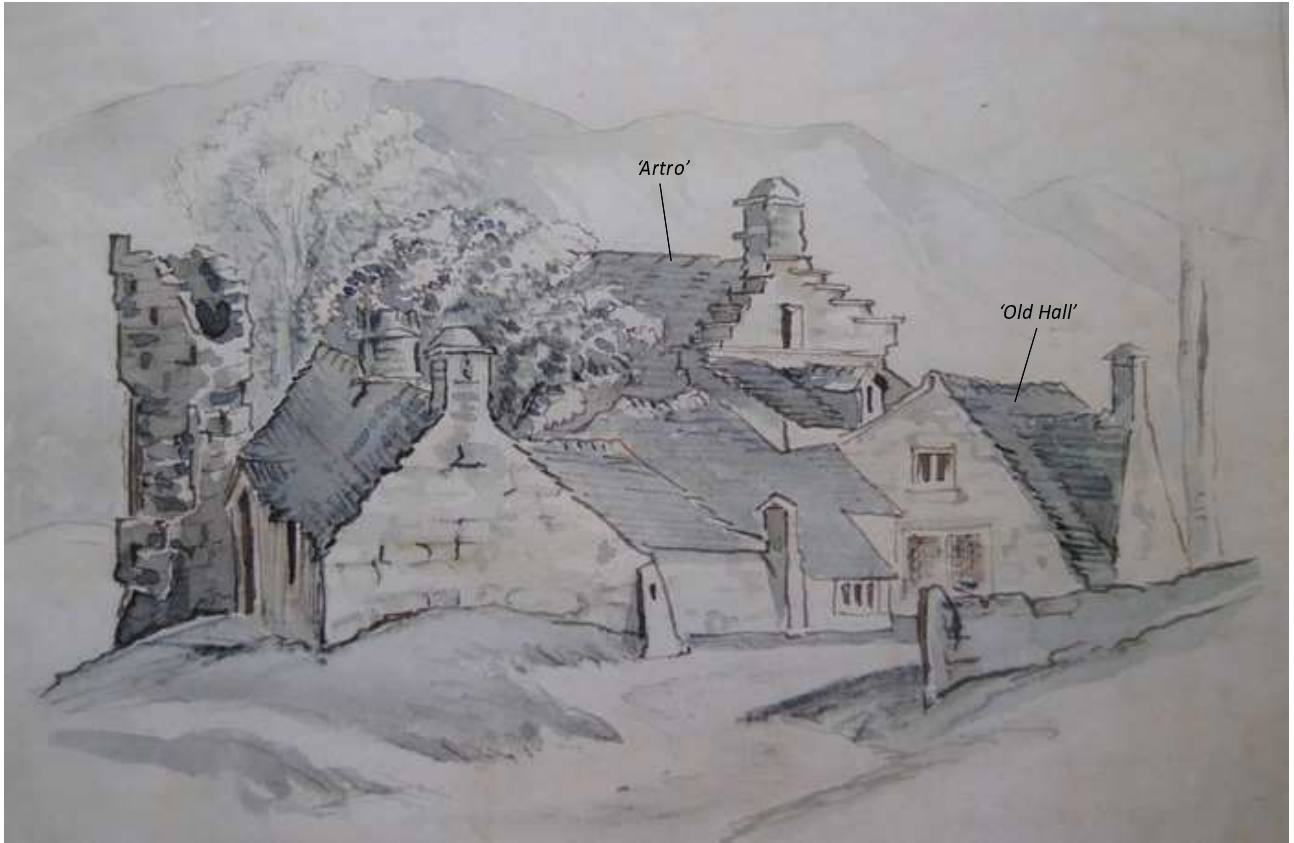
(a) General view of Dolmelynlyn Hall from north-west (compare Plate 3).
