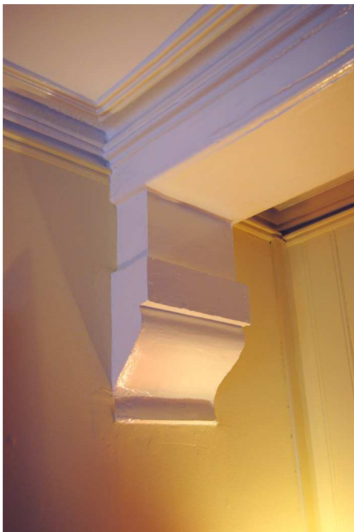
Plate 32: Ceiling beam on corbel, [1F02].
