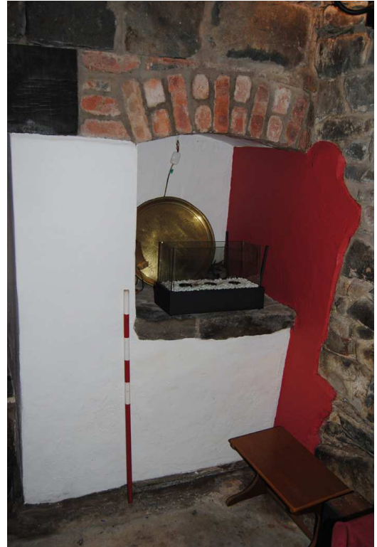
Plate 12: Bread oven inserted into primary FP recess.
