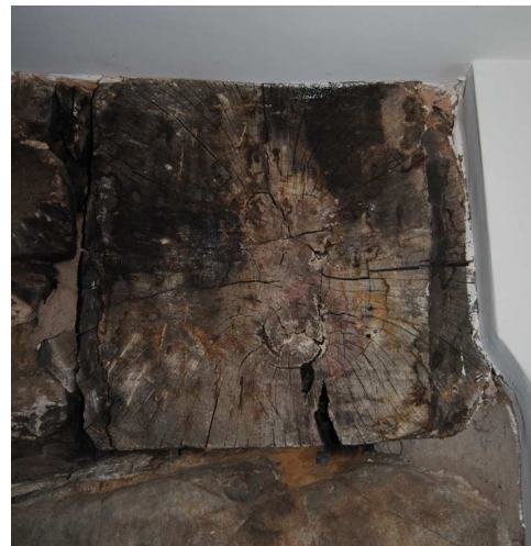
Plate 27: Detail of former FP bresummer, (NB: chamfered ariss to bottom right).
