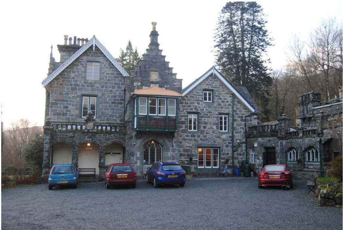
Plate 1: Principal elevation to north, 'Arthro' range to right of crow-stepped entrance (compare Figure 4b).
