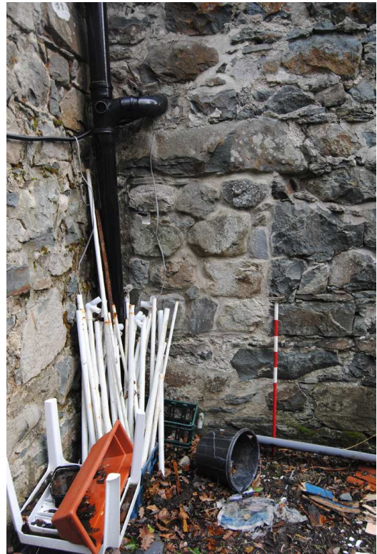
Plate 6: Blocked window to west elevation.
