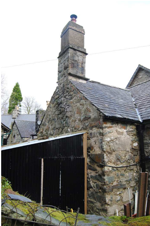
Plate 5: 'Old Hall', detail of lateral stack projection.
