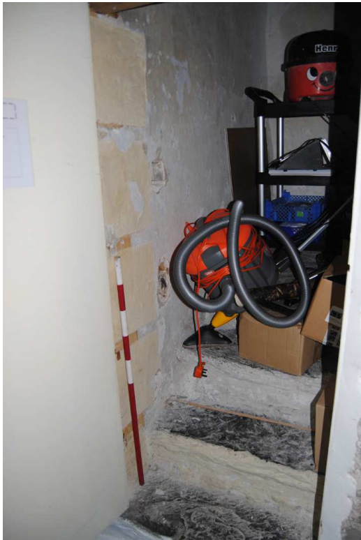
Plate 28: Stone winder stair (A) rises from south wall of passage.
