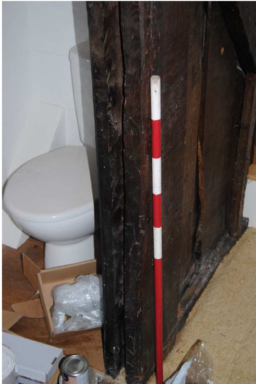
Plate 38: T1 (W): stud grooved to receive planking panels.
