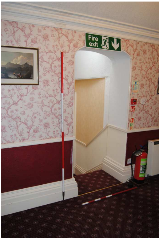
Plate 29: Doorway at E end corridor [1F01] (former window).
