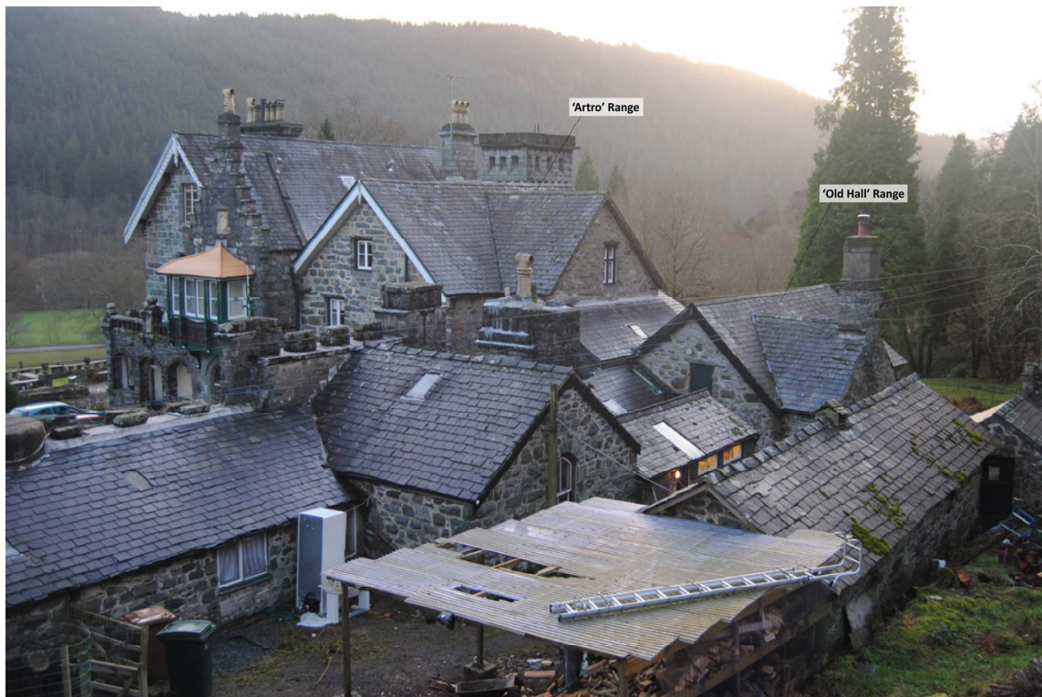
Plate 3: General view of complex from north-west with 'Arthro' range to centre, 'Old Hall' to right (compare Figure 3a).
