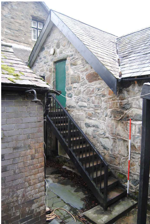
Plate 7: 'Old Hall', north elevation (oblique).
