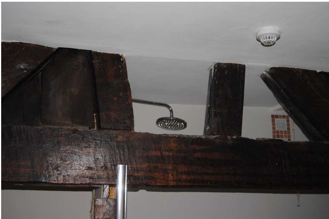
Plate 40: Room [2F01] ('Arthro'); truss T1 - angled struts above collar.
