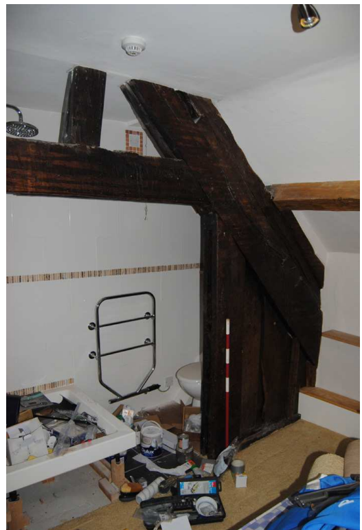
Plate 37: Room [2F01] ('Artro'); detail of Truss T1 (W).
