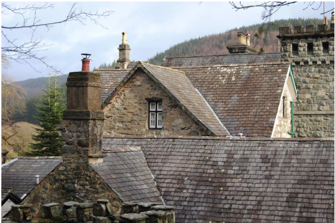
Plate 19: 'Arthro' range with gabled stair/stack (removed) projection, viewed from west.
