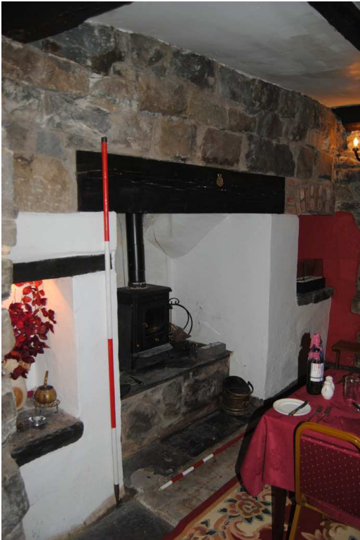
Plate 11: [GF01]: inserted FP within primary recess at north end of west wall.
