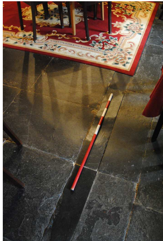
Plate 10: [GF01]: patching in slate floor beneath beam C.
