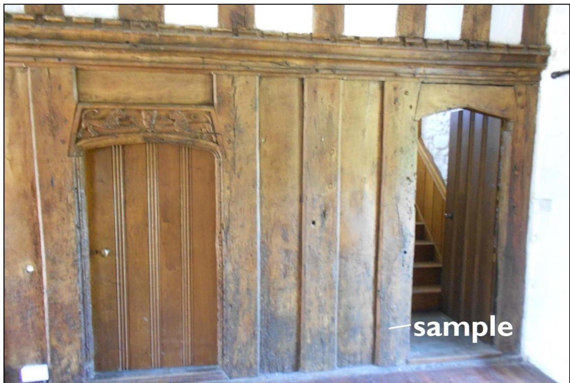
Figure 1: View of the screen, showing the approximate position of the sample taken for future radiocarbon analysis.
