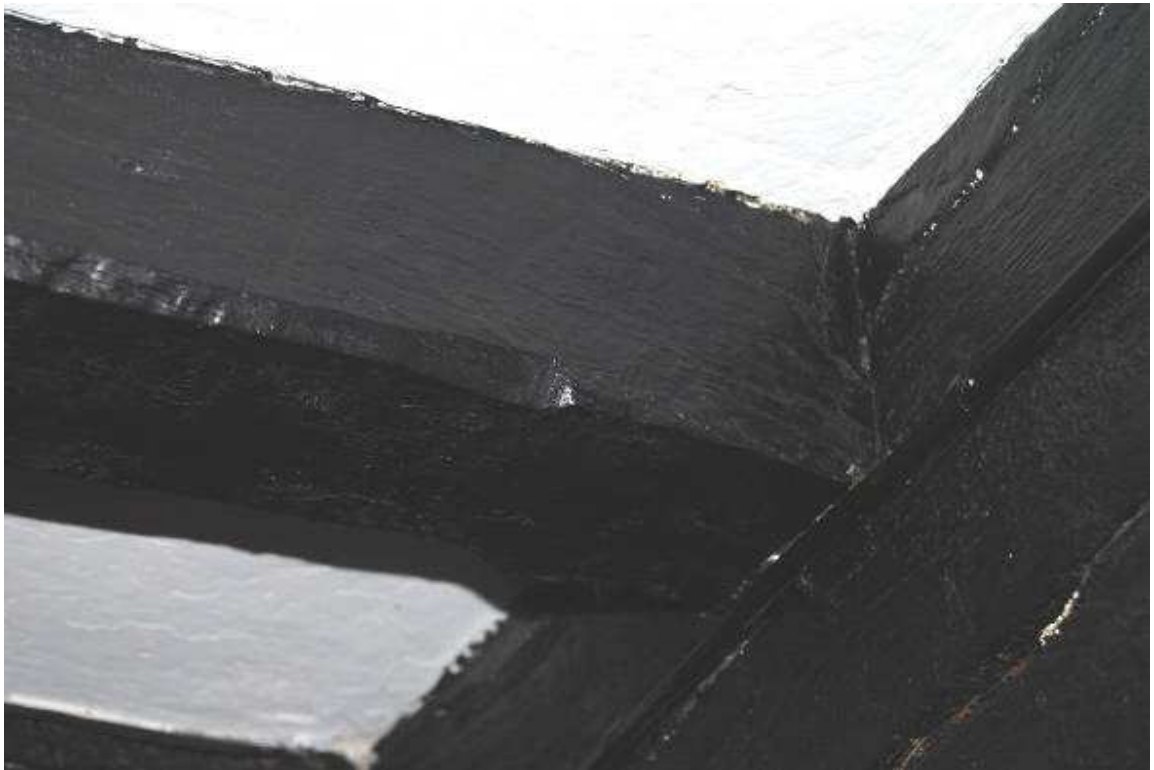
Plate 12: [GF01]; detail of main beam / common joist. NB; fine chamfer, stop and bare-faced soffit tenon joint.
