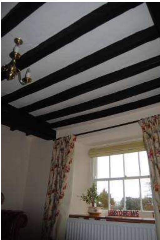
Plate 10: [GF01] ceiling structure, looking east.
