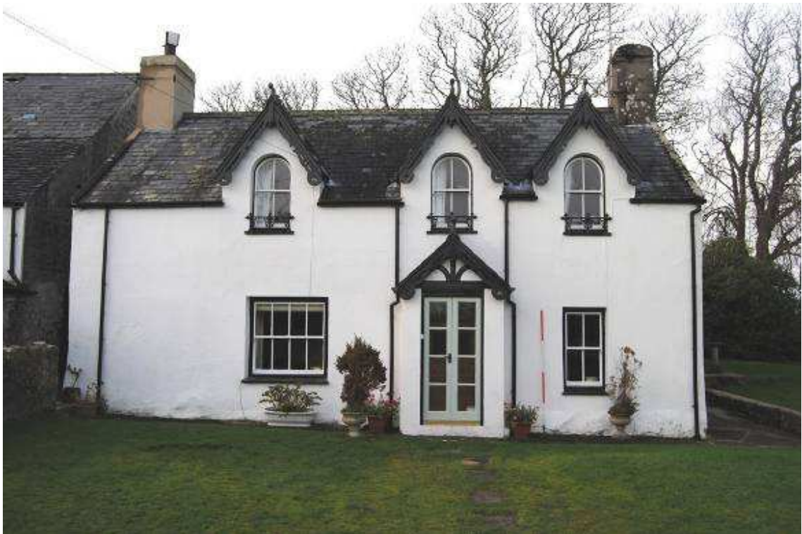
Plate 2: Principal range, east elevation.
