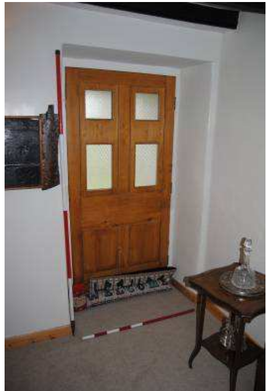
Plate 16: Room [GF02]; door in east wall.
