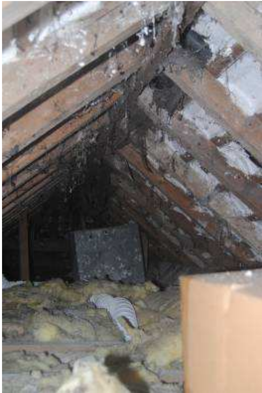
Plate 32: Common rafter roof over NW extension.
