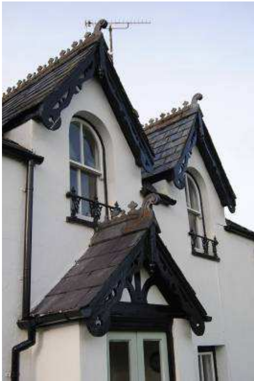
Plate 3: Principal range; detail of porch gable and dormers.
