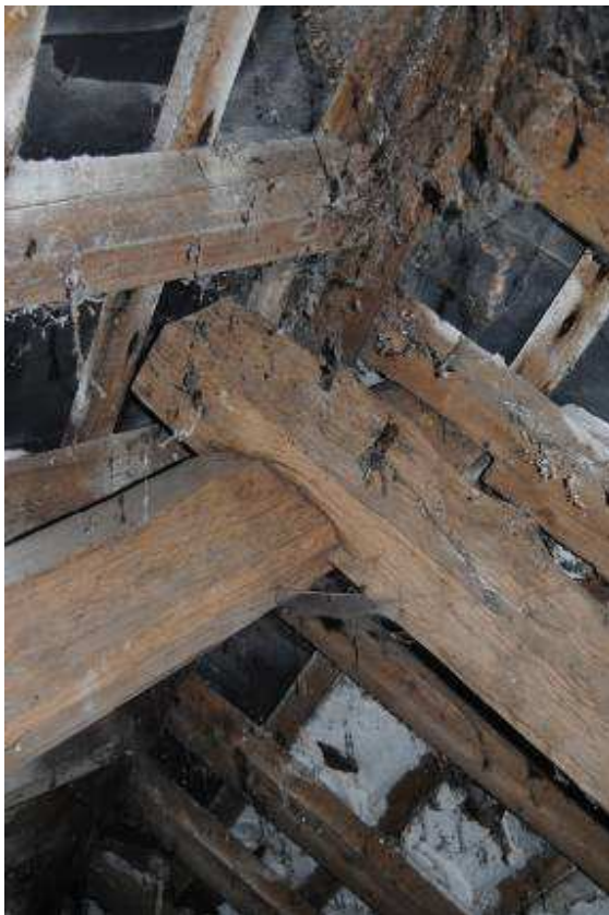
Plate 25: Principal range roof; apex detail
