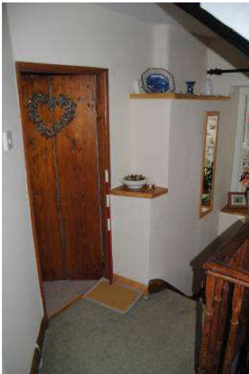
Plate 19: Head of inserted stair (note stack).
