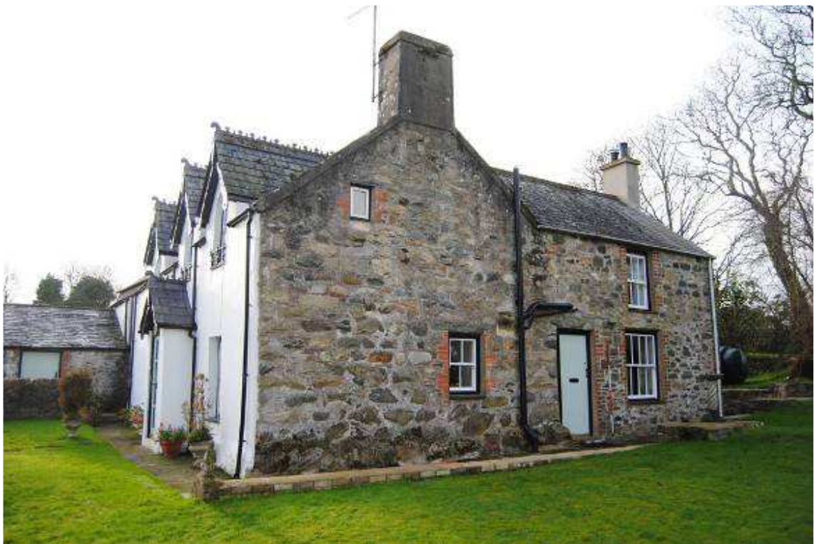
Plate 8: General view of north elevation; principal range (left) and north-west extension (right).
