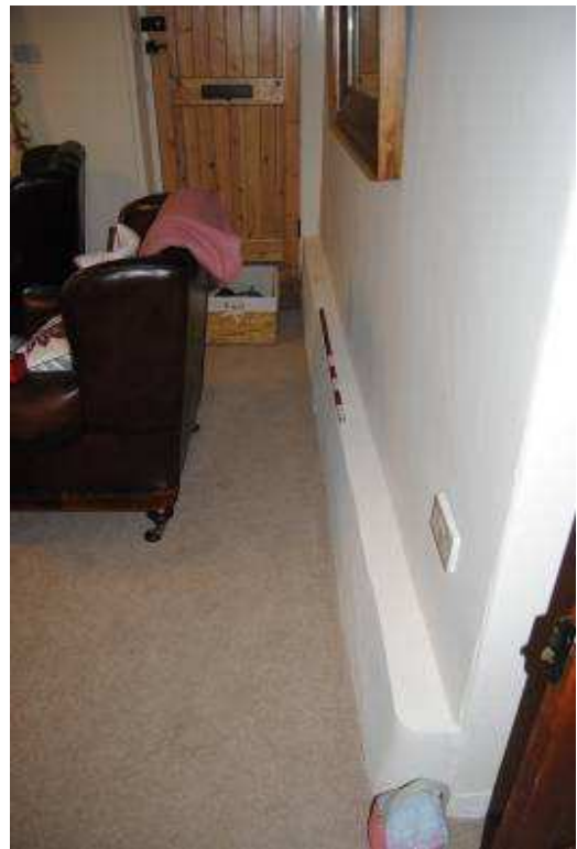
Plate 31: [GF03]; offset at base of east wall (ie. western exterior wall of primary range).
