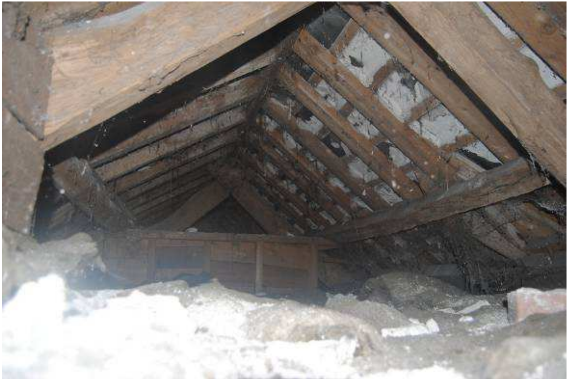
Plate 24: Roof of principal range observed from hatch within [1F02].
