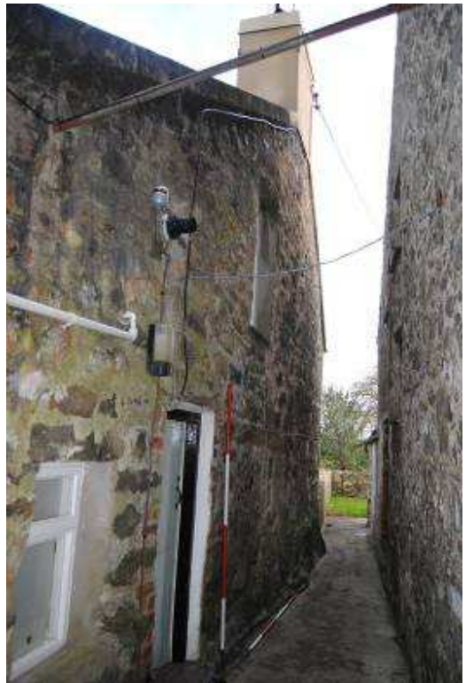
Plate 6: Principal range, south elevation (oblique).
