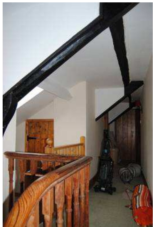
Plate 20: Lateral corridor [1F01] to west side of principal block, note principal rafters.
