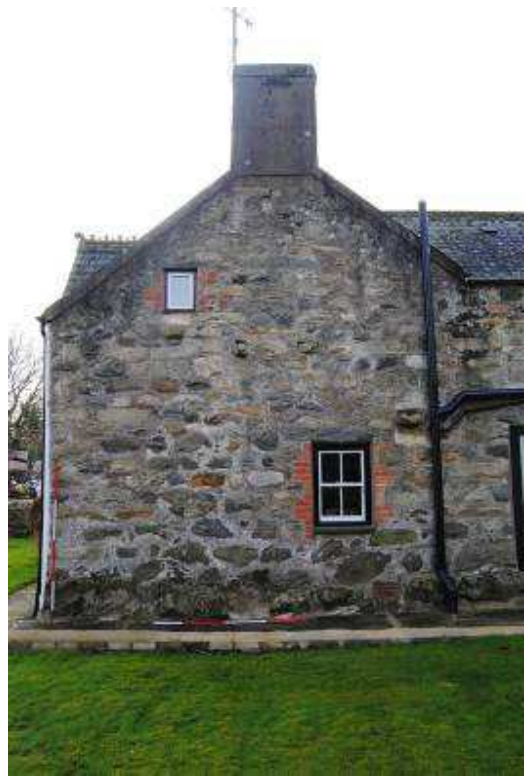
Plate 4: Principal range; north elevation.
