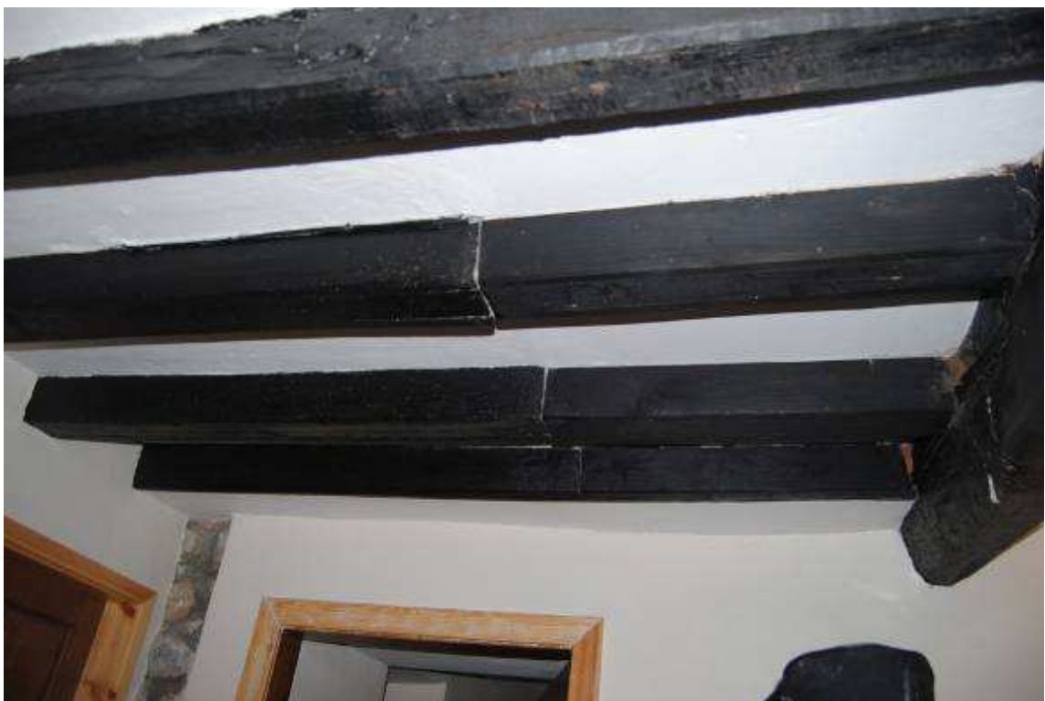
Plate 17: Room [GF02]; renewed ceiling joists to west.
