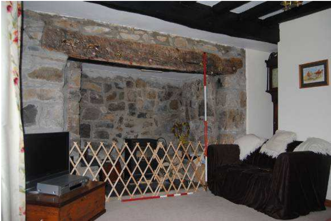
Plate 9: Room [GF01]; principal FP to south wall.
