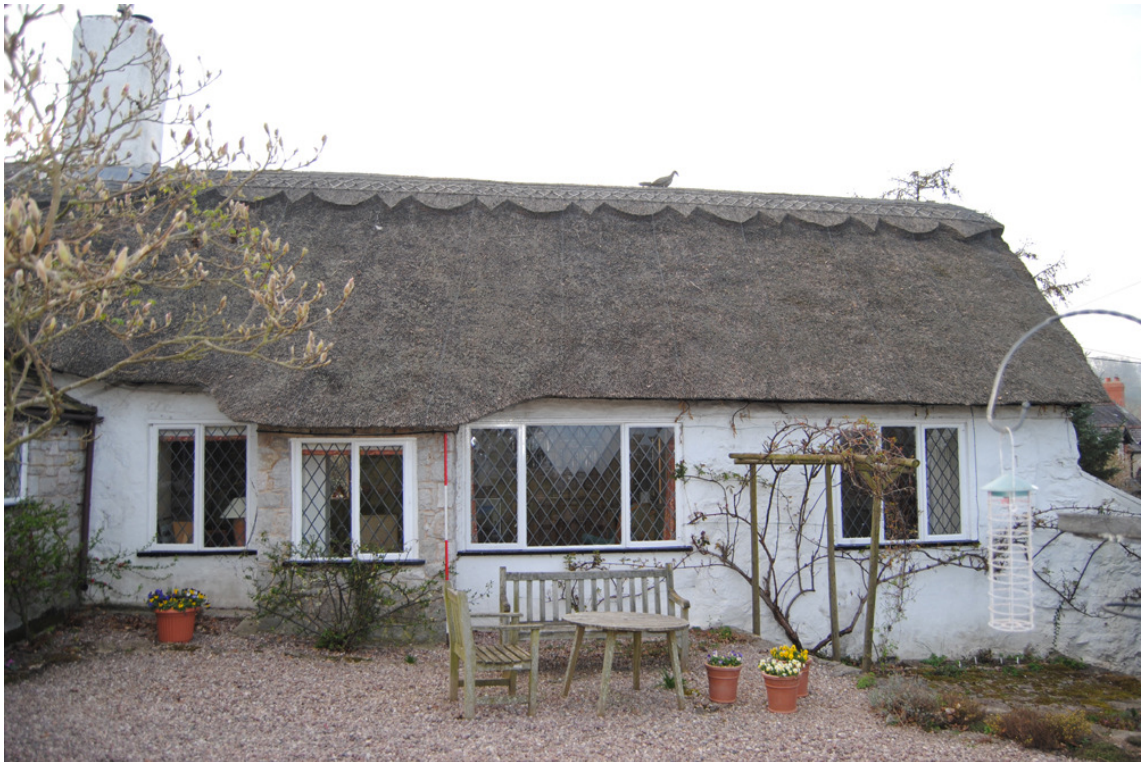
Plate 6: North end of east elevation; inserted windows and window projection.
