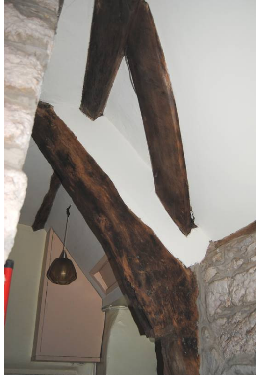
Plate 15: Cruck [T2] (E); wind-bracing to lower purlin.
