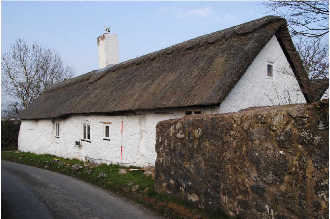
Plate 2: West elevation, oblique, looking north-east.
