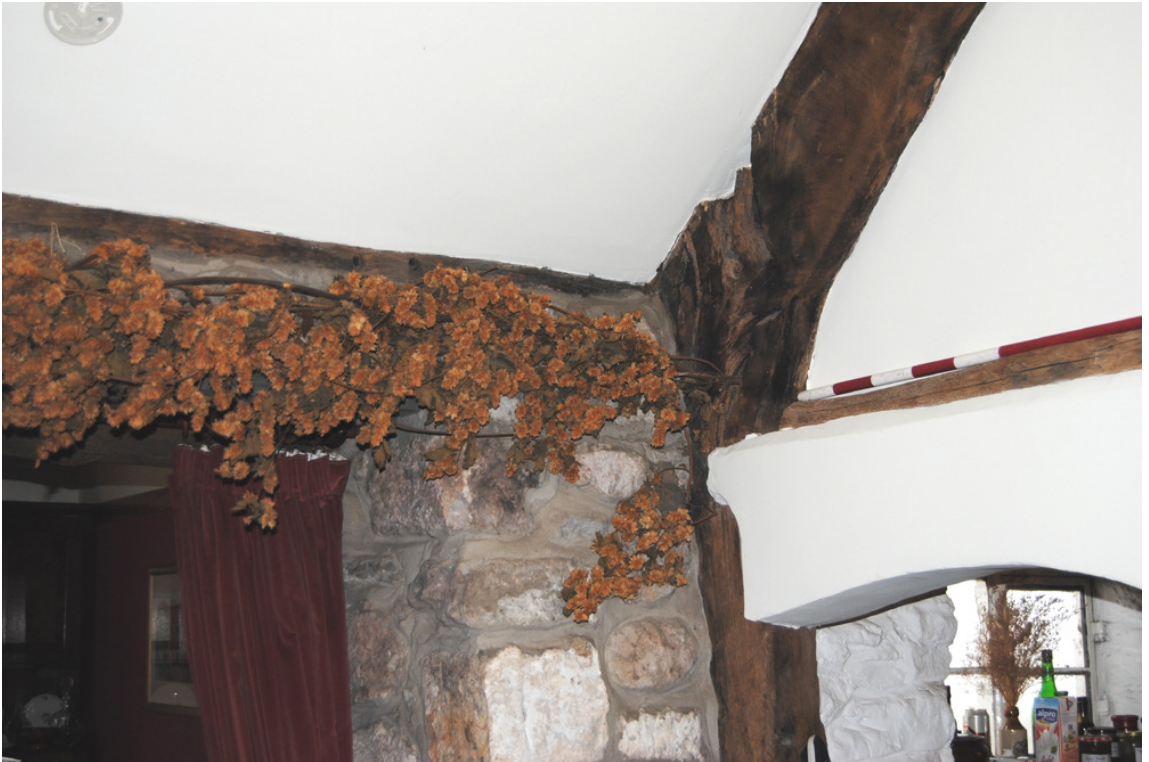
Plate 18: Cruck [T1] (E) NB: section of primary wall plate to left.
