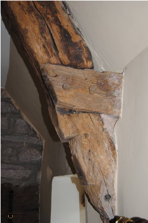
Plate 12: Cruck [T3] (W); truncated tie.
