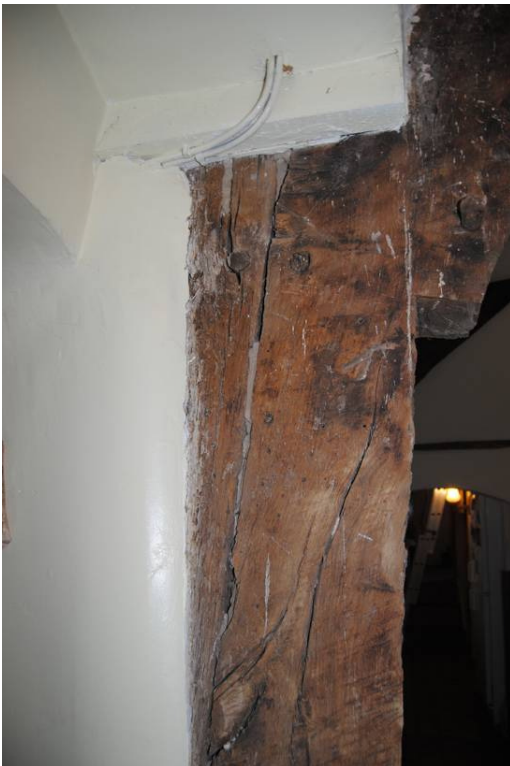
Plate 14: Cruck [T2] (E); detail of post.
