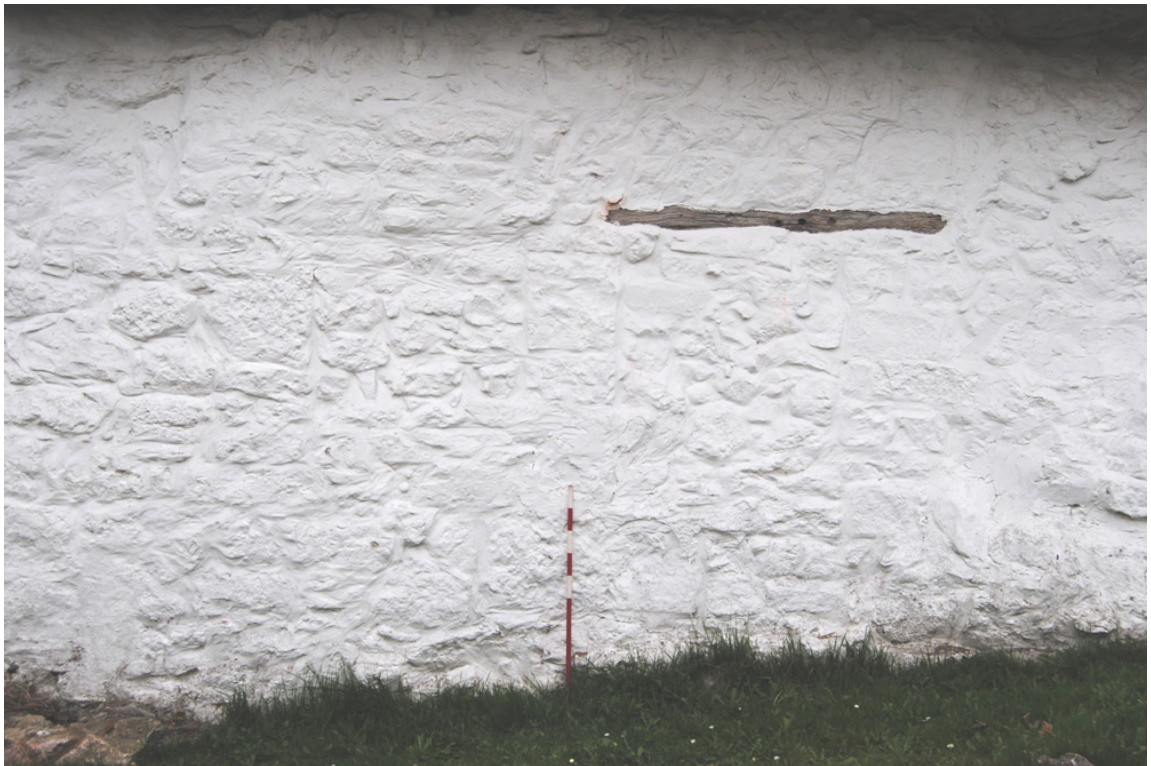
Plate 5: Blocked window (left) and doorway (right with lintel) at north end of west elevation.
