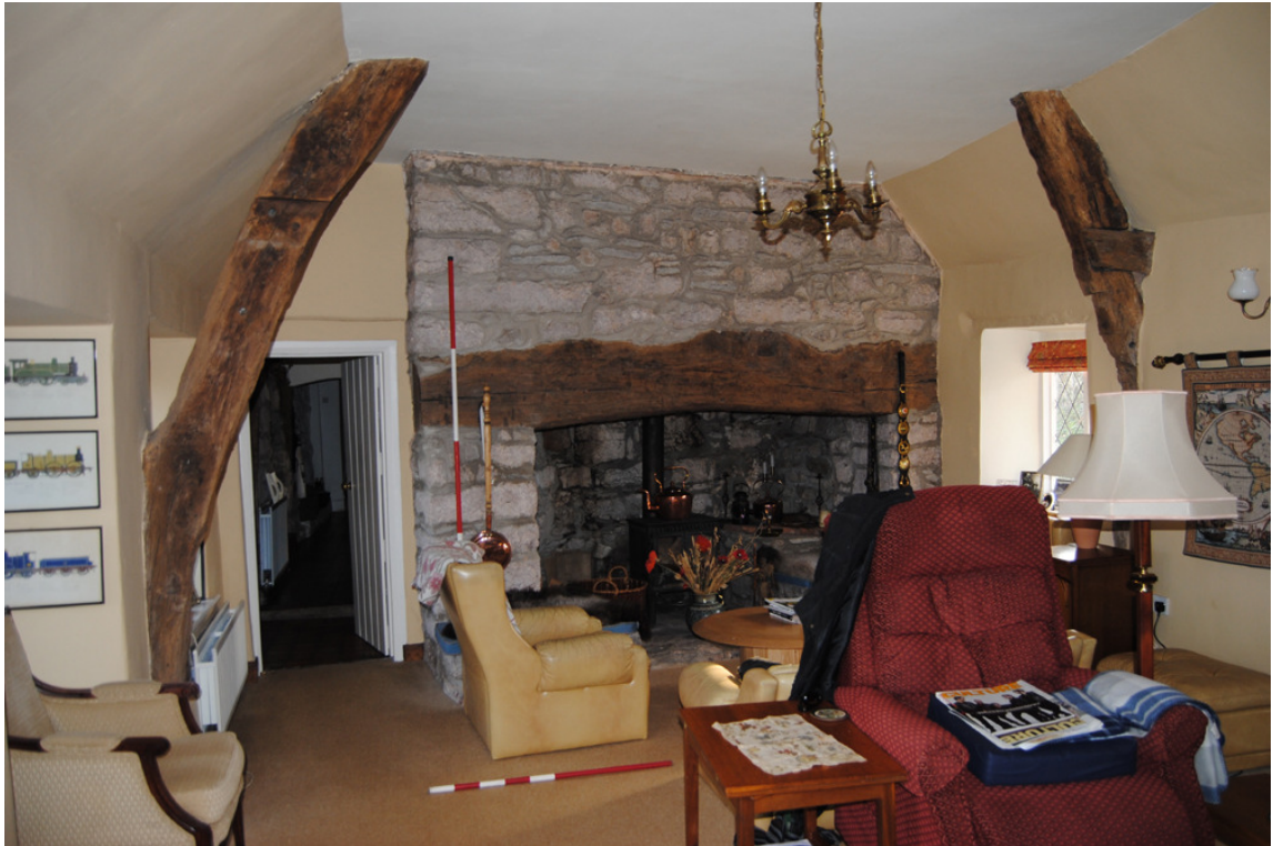
Plate 10: Cruck [T3] looking south towards inserted stack.
