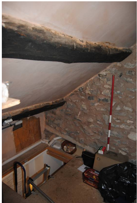
Plate 21: Bay 1 western roofslope showing two tiers of purlins.
