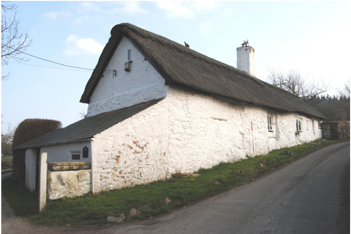
Plate 1: West elevation, oblique, looking south-east.
