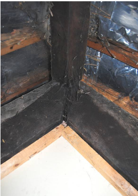
Plate 20: Cruck [T1], apex detail.
