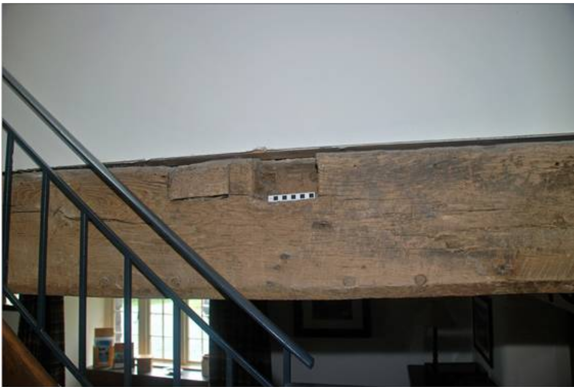
Plate 16: Mortise for an original joist.
