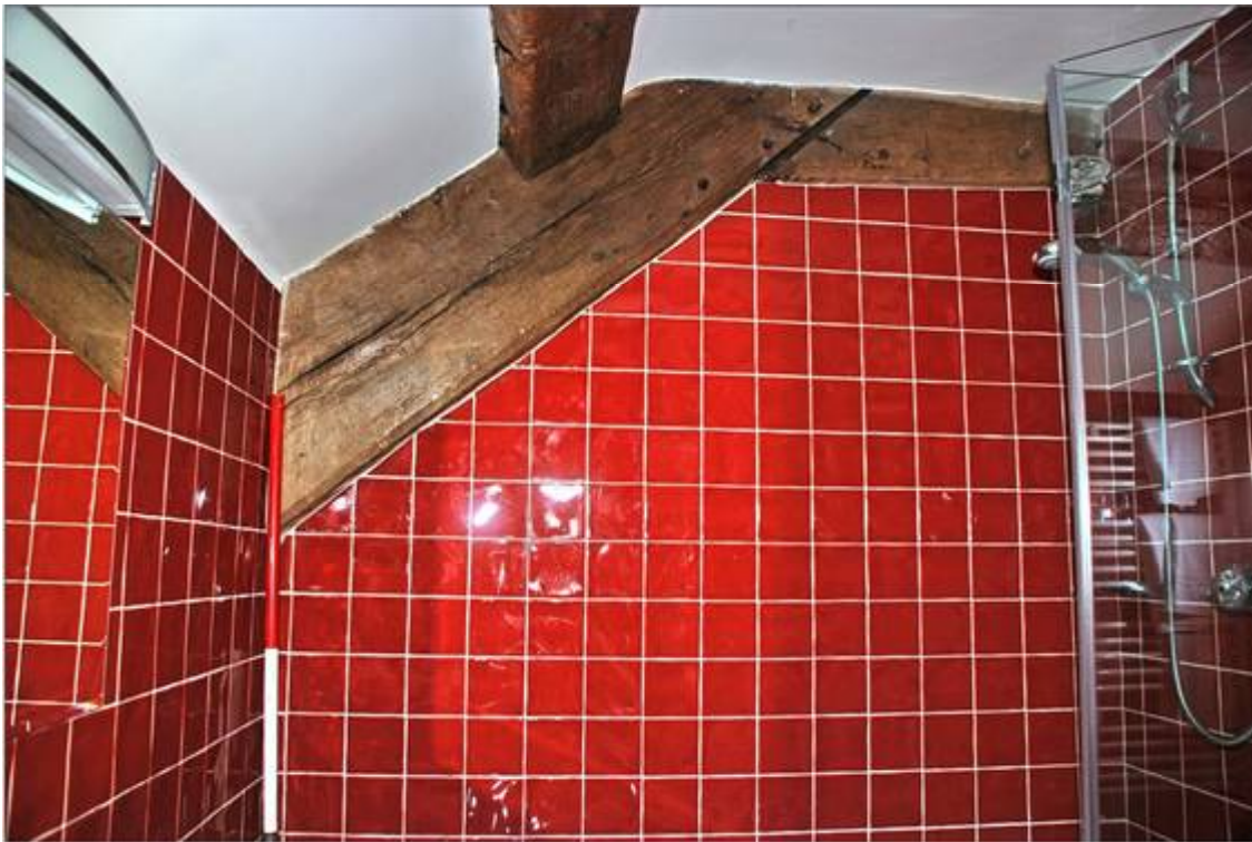
Plate 18: Truss 1 in bathroom
