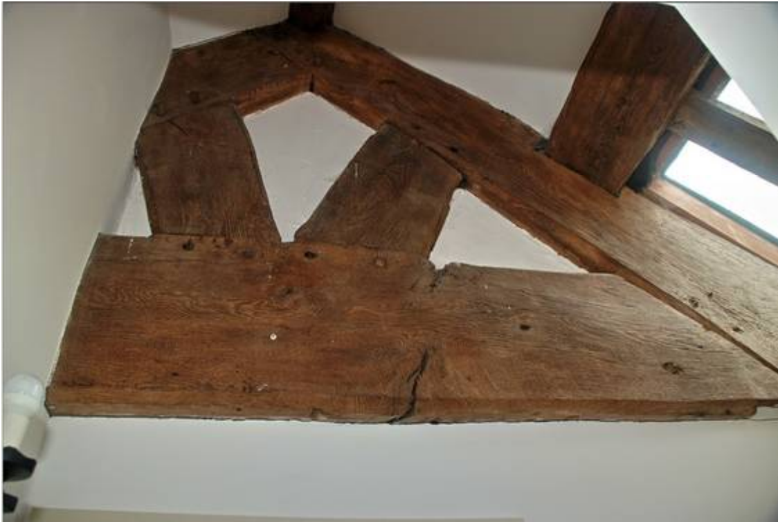
Plate 17: Truss 1 over the stairwell
