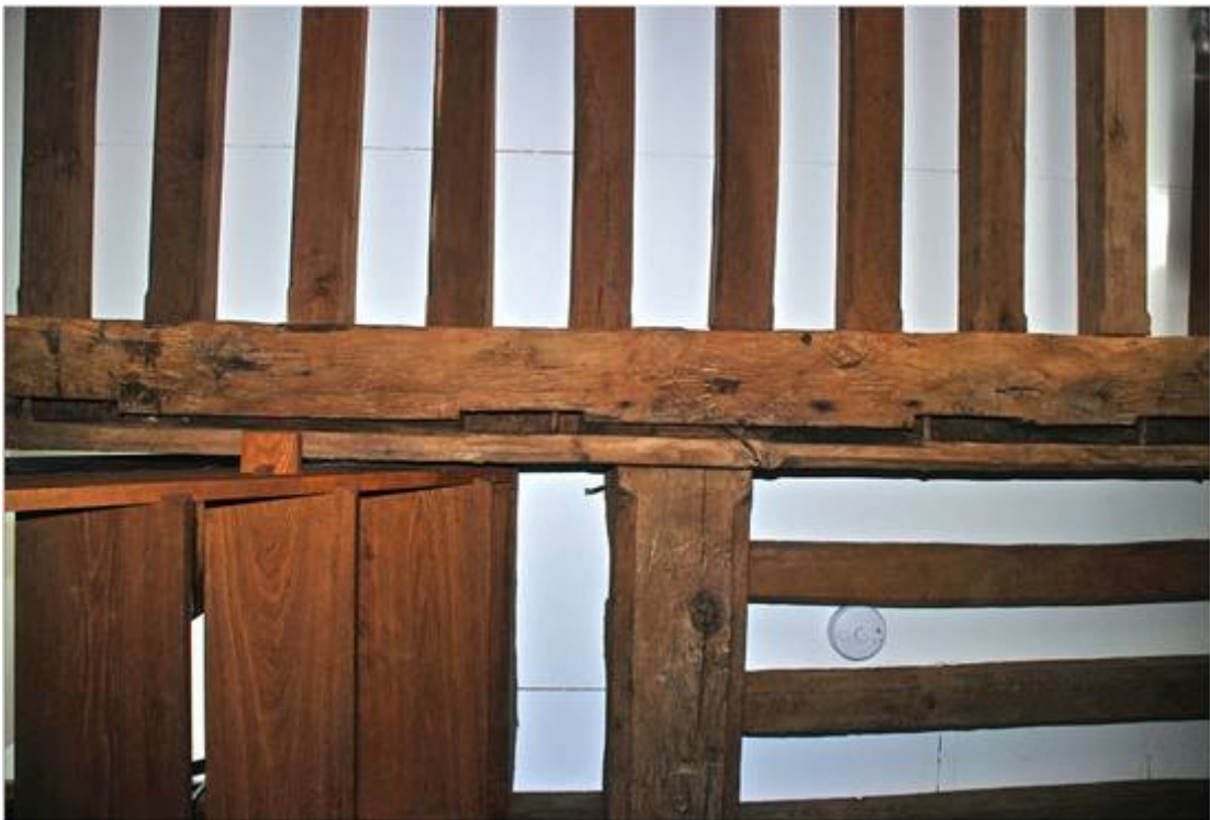
Plate 14: Evidence for the post and plank partition
