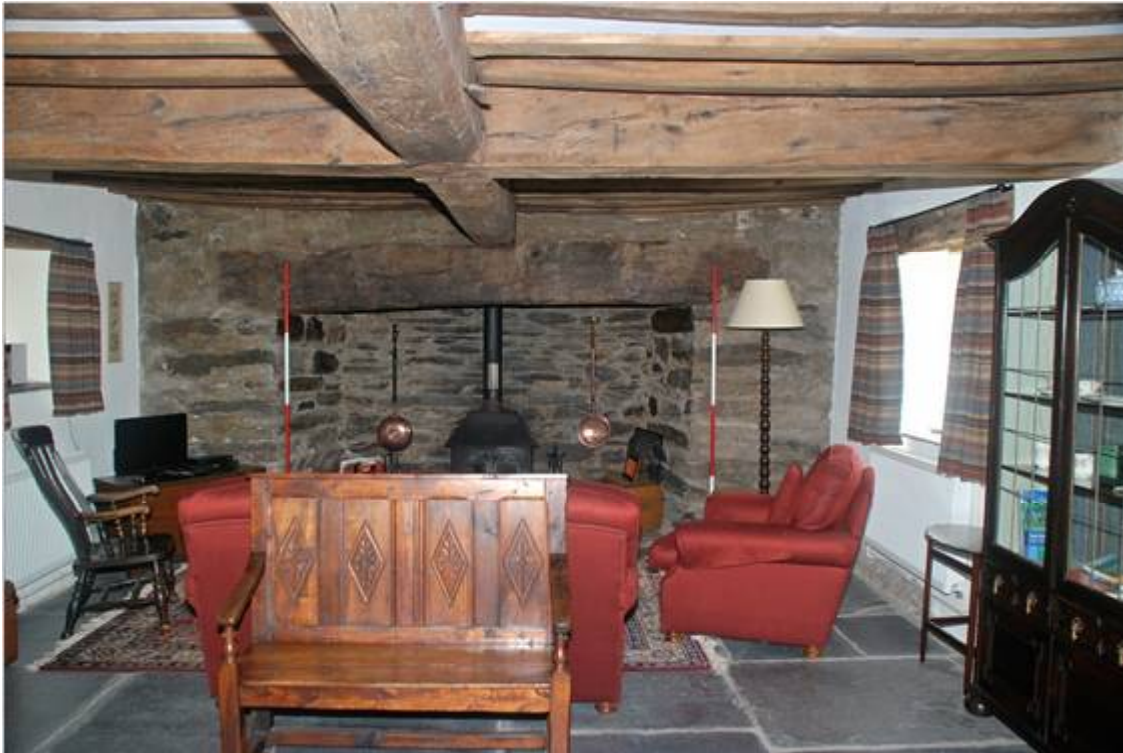
Plate 12: Bressumer and main longitudinal beam
