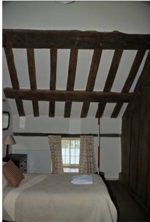
Plate 23: Common rafters and wall rail looking south east
