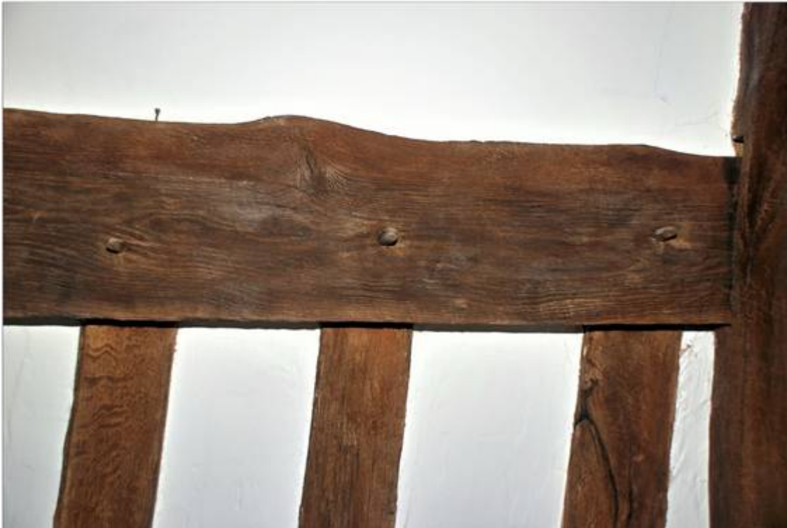
Plate 24: Detail of relationship between the purlins and common rafters
