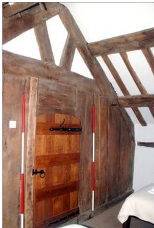
Plate 20: Plank and post partition looking west
