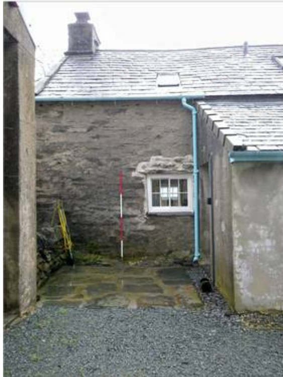
Plate 4: Rear elevation of original building
