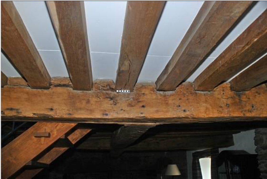
Plate 15: Ceiling joists
