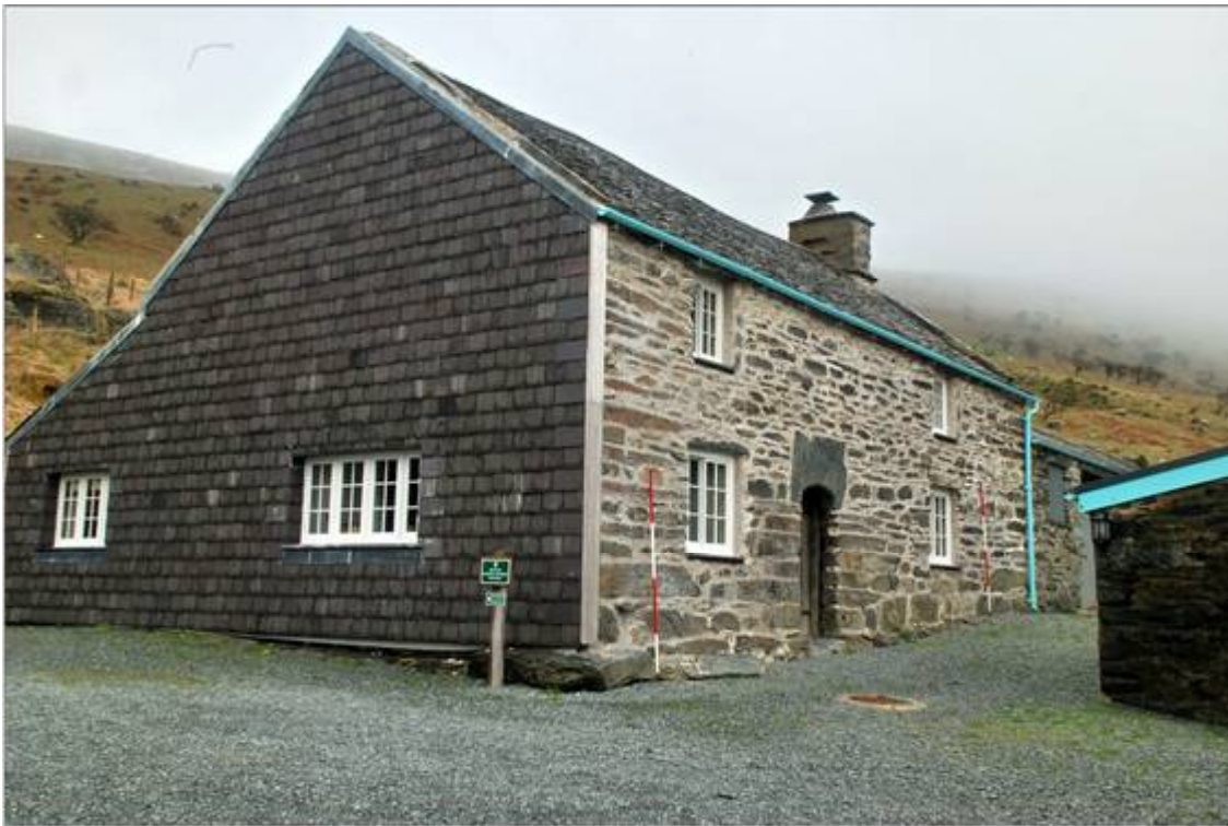
Plate 2: Front elevation looking north
