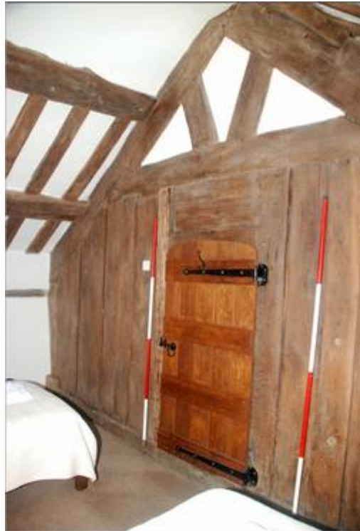
Plate 21: Plank and post partition looking south
