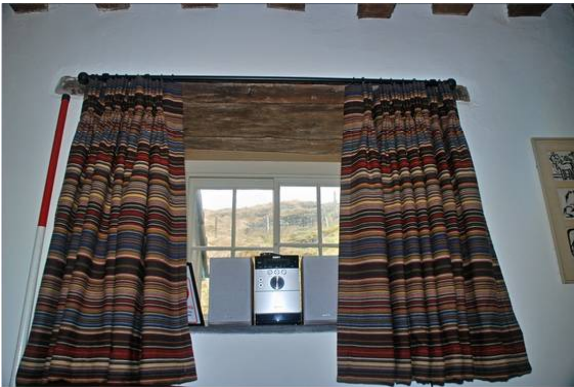
Plate 8: North eastern window showing wooden lintel
