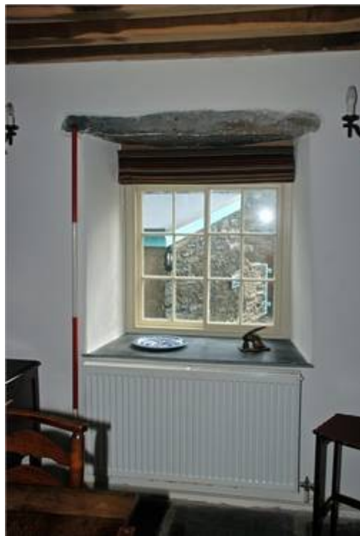
Plate 10: South eastern window showing slate lintel
